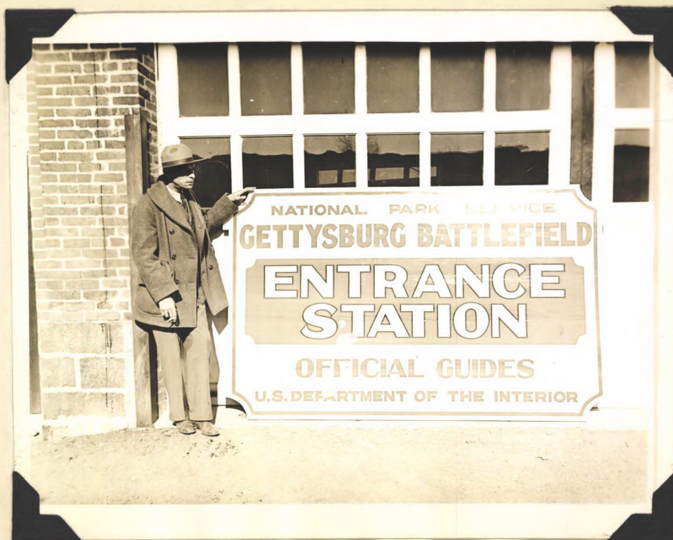
ENTRANCE STATION Sign after Alteration
