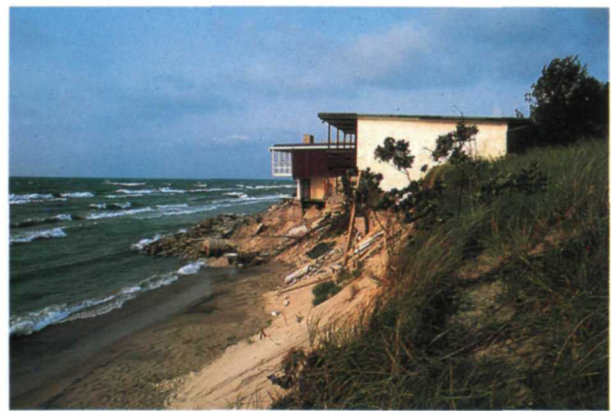
Coastal erosion causes large amounts of public and private property damage every year. This house was built close to a Lake Michigan beach that was eroding quickly.
