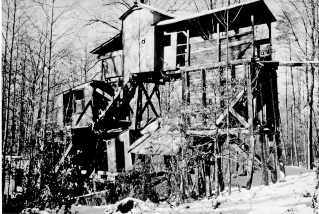
FIGURE 5.—Ruins of assay laboratory and mill. A , Ruins of assay laboratory at the Ford mine, about 100 feet east of No. 2 shaft. Brick structure in foreground was the furnace; cement tables in the background held analytical balances used for precise weighing. B , Ruins of mill at the Maryland mine. Ore cars entered on trestle at a , and dumped into ore bin ( b ). Ore was fed into primary jaw crusher located on concrete foundation at c , where the ore was crushed to fragments about 3 inches in diameter. It was then hoisted by bucket elevator to a second jaw crusher ( d ). From there, the ore passed through a 10-stamp mill ( e ) and ball mill ( f ). Finely crushed ore then passed through an impact amalgamator where free gold combined with mercury; it then passed over concentrating tables where gold-bearing sulfide minerals were recovered.
