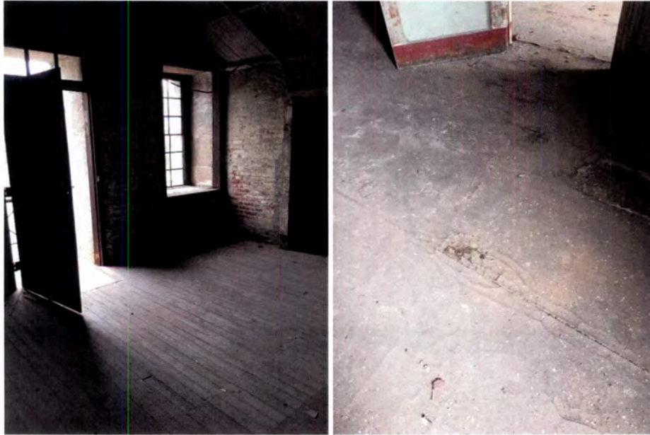
Figure 66: Wood flooring (left) and composite sheet flooring (right).
