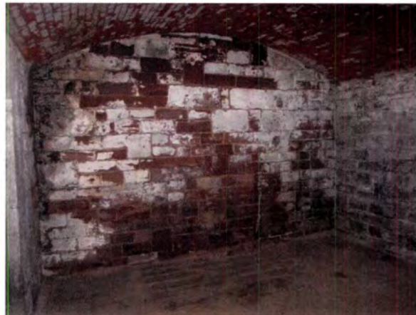
Figure 49: Brick arched ceiling in Room 112.
