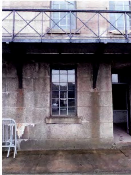
Figure 26: Typical biological staining and efflorescence on granite walls of Parade Ground.
