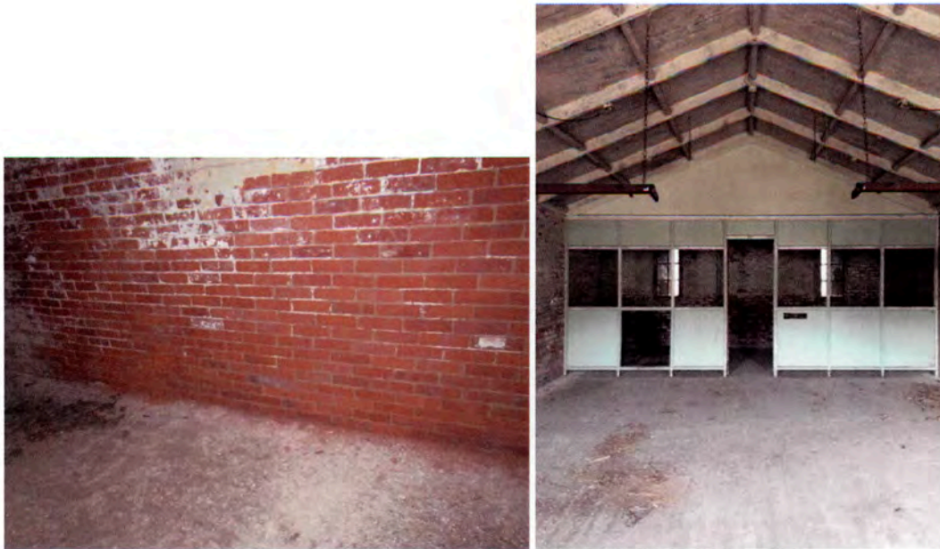
Figure 68: Typical brick walls (left) and added partitions (right) on the second floor.
