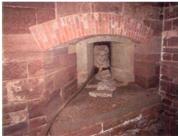
Figure 96: Infilled Gun Port in Counterscarp.
