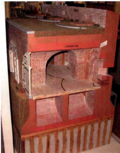
Figure 5: Model of Fort Pulaski, showing similar construction of the East Casemates at Fort Tompkins with cisterns below. 12
