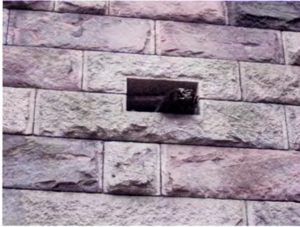
Figure 20: Rectangular masonry openings in upper level of granite counterscarp walls.
