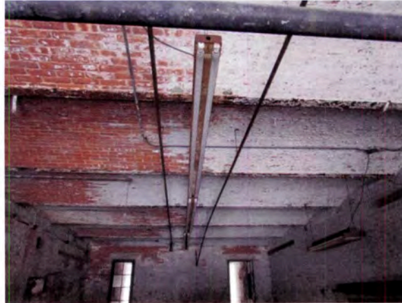
Figure 33: Typical arched, brick ceilings with exposed steel joists.
