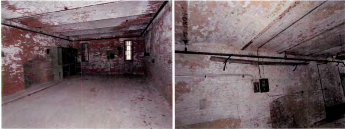
Figure 43: Typical ceiling conditions of first floor.
