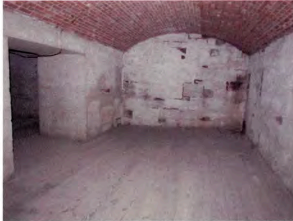
Figure 57: Granite and sandstone walls in Room 149.
