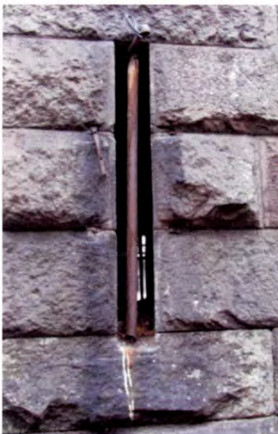
Figure 5: Detail of embrasure with metal pole at south end of west elevation (left) and embrasures at north end of east elevation (right).
