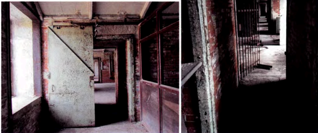
Figure 73: Sliding metal door in Room 211 (left) and iron gate in Room 212 (right).
