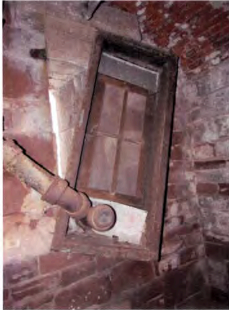
Figure 55: Modified window in corner section of first floor.
