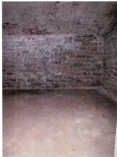
Figure 43: Typical concrete floor in corner of first floor.
