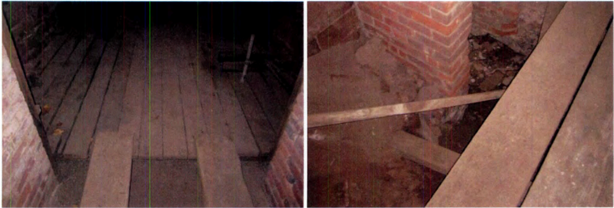
Figure 99: Wooden platform (left) and excavation of Counterscarp (right).
