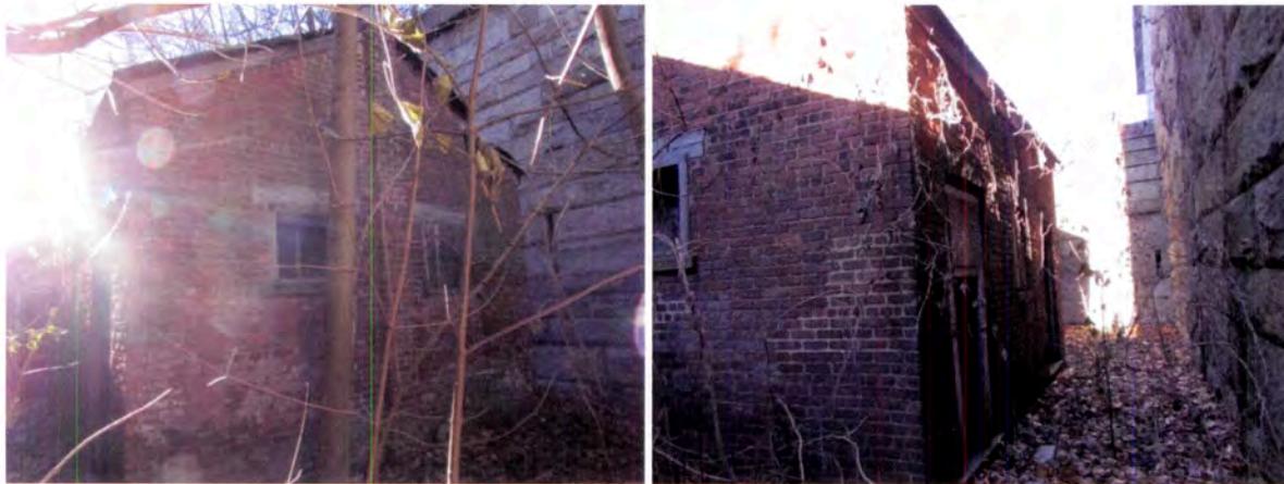
Figure 103: East elevation (left) and south elevation (right) of Building 139.
