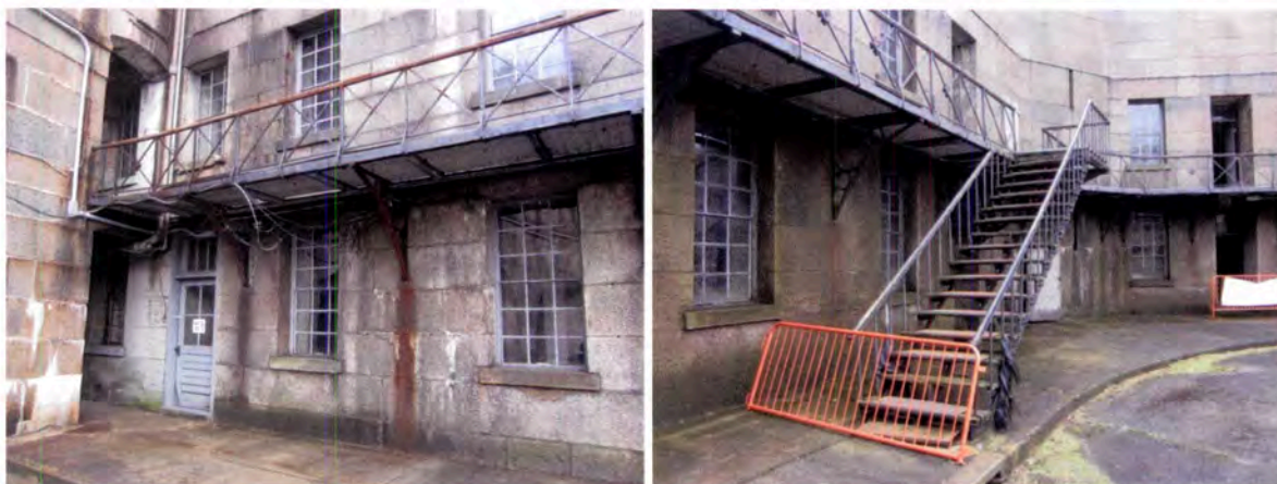
Figure 27: Typical gallery framing (left) and staircase (right) in Parade Ground.
