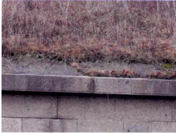
Figure 16: Top of masonry wall and vegetative roof.
