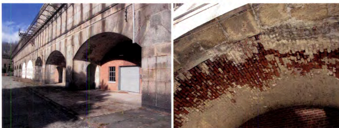
Figure 28: Brick arches of East Casemates (left) and the underside of the brick arches of the East Casemates (right).
