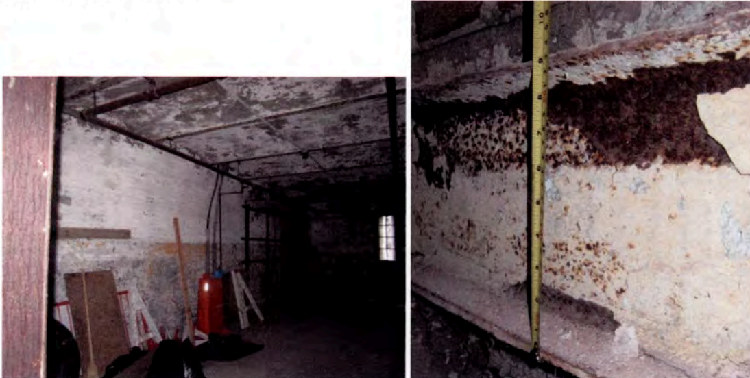
Figure 41: Overview of typical first floor room (left) and detail of typical beam (right).
