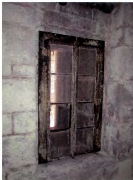
Figure 83: Four-light steel French casement window in Room 227A.
