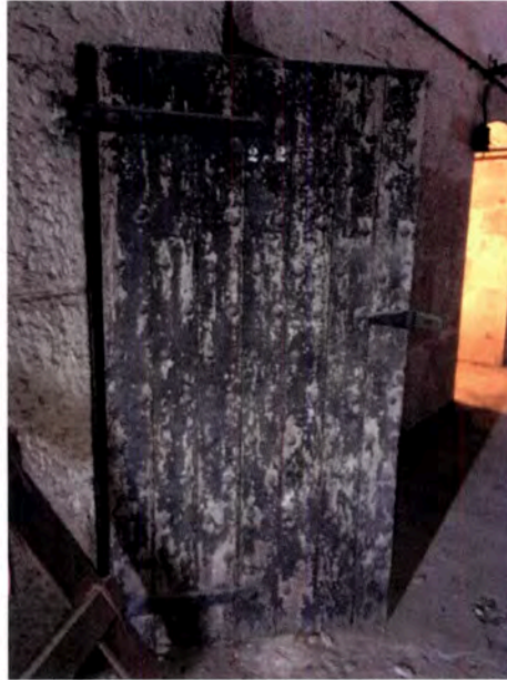
Figure 92: Wood door with metal strap hinges and lock in the south corner of the second floor.
