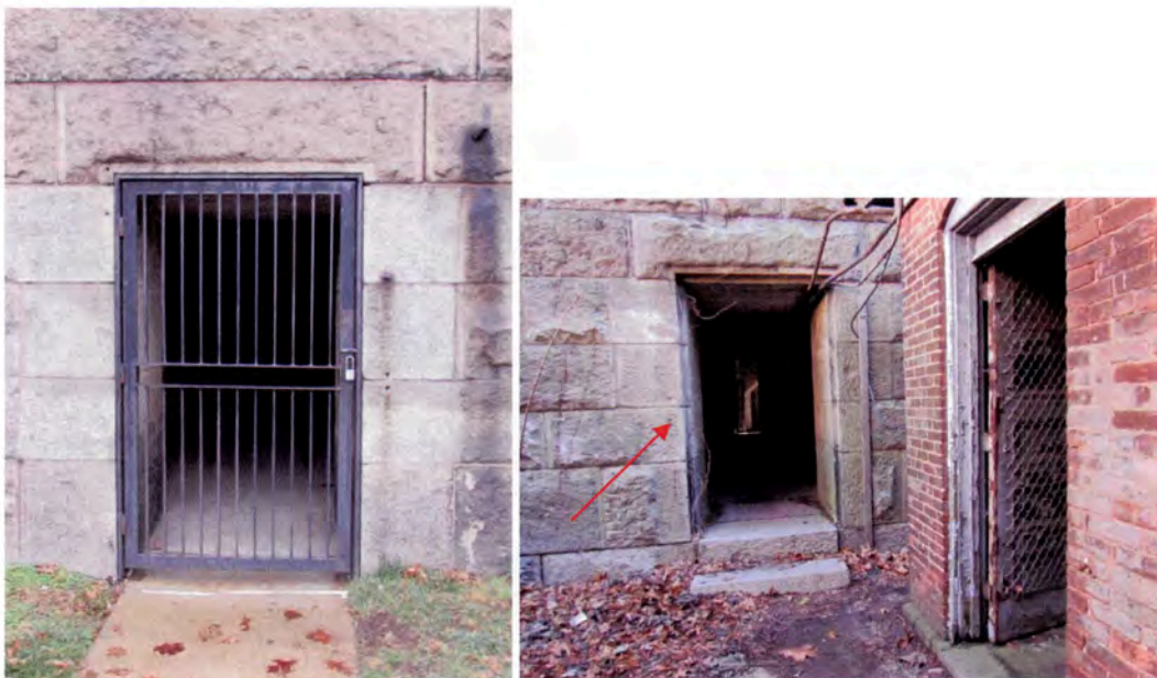
Figure 8: Masonry opening with metal gate at east end of south elevation and masonry opening at east end of north elevation (right).
