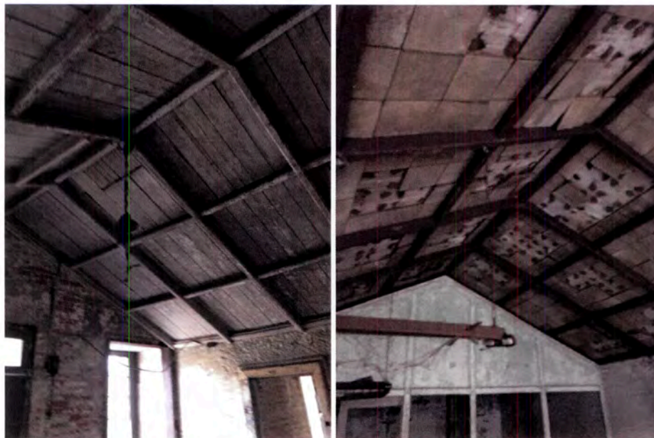
Figure 70: Wood bead board ceiling on exposed wood rafters (left) and acoustical ceiling tile on exposed wood rafters (right).
