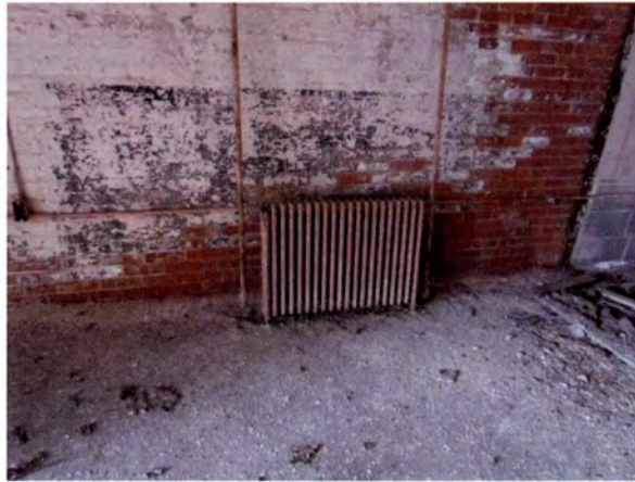
Figure 37: Typical radiator and pipes on first floor.
