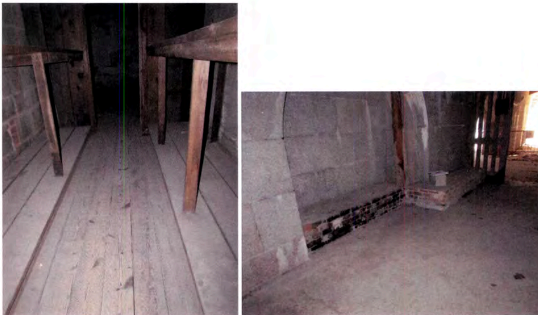
Figure 56: Wood board floors in Room 149 (left) and concrete floor in Room 150 (right).
