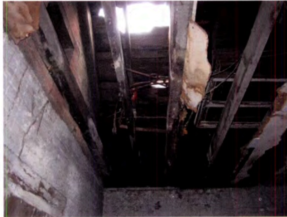
Figure 106: Roof structure of Building 139.
