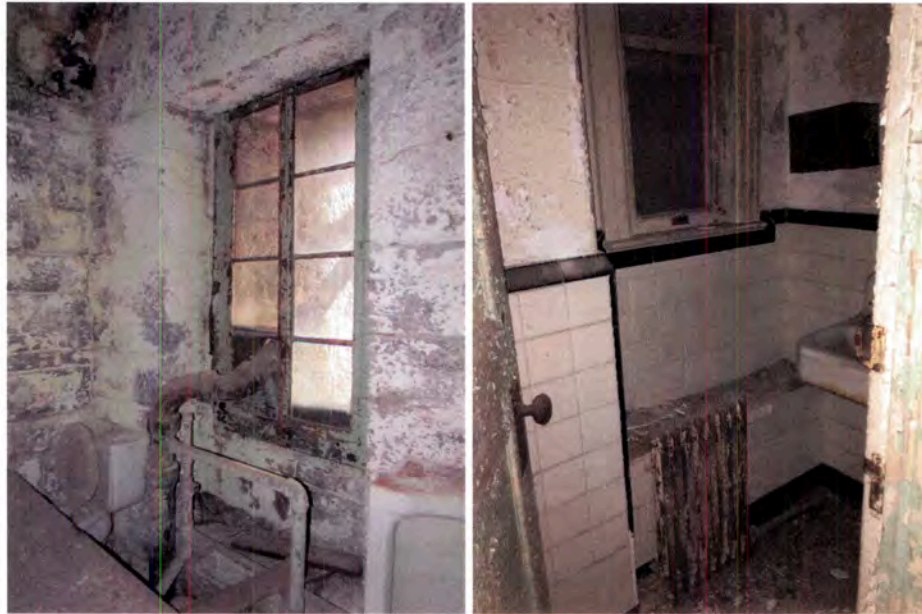
Figure 90: Modified French casement window (left) and one-over-one double-hung window (right).
