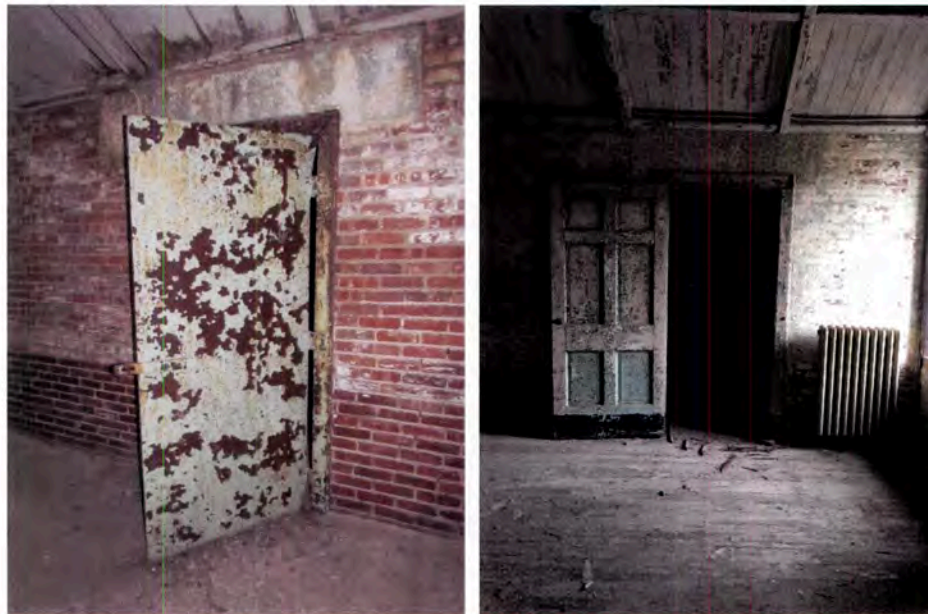
Figure 79: Typical conditions of second floor doors.
