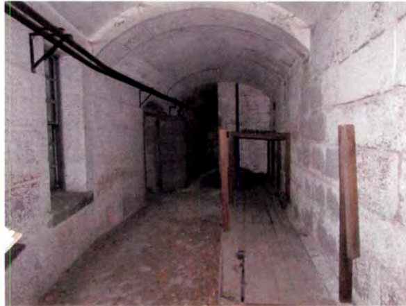
Figure 89: Granite walls in Room 236.
