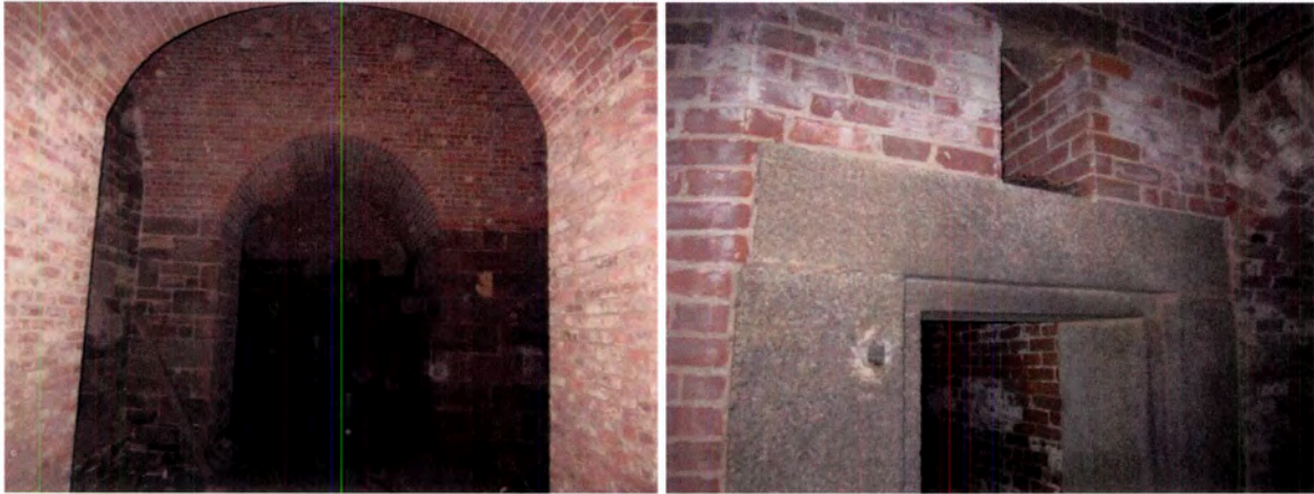
Figure 95: One of the larger casemates in counterscarp (left) and interior granite and brick interior wall in counterscarp (right).
