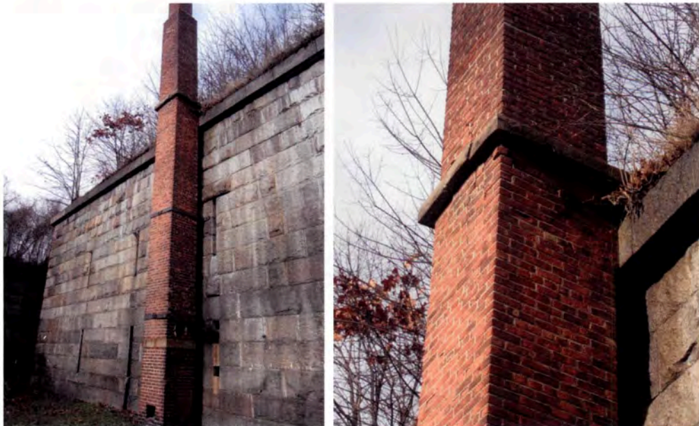
Figure 17: Overview and detail of west chimney on south elevation.
