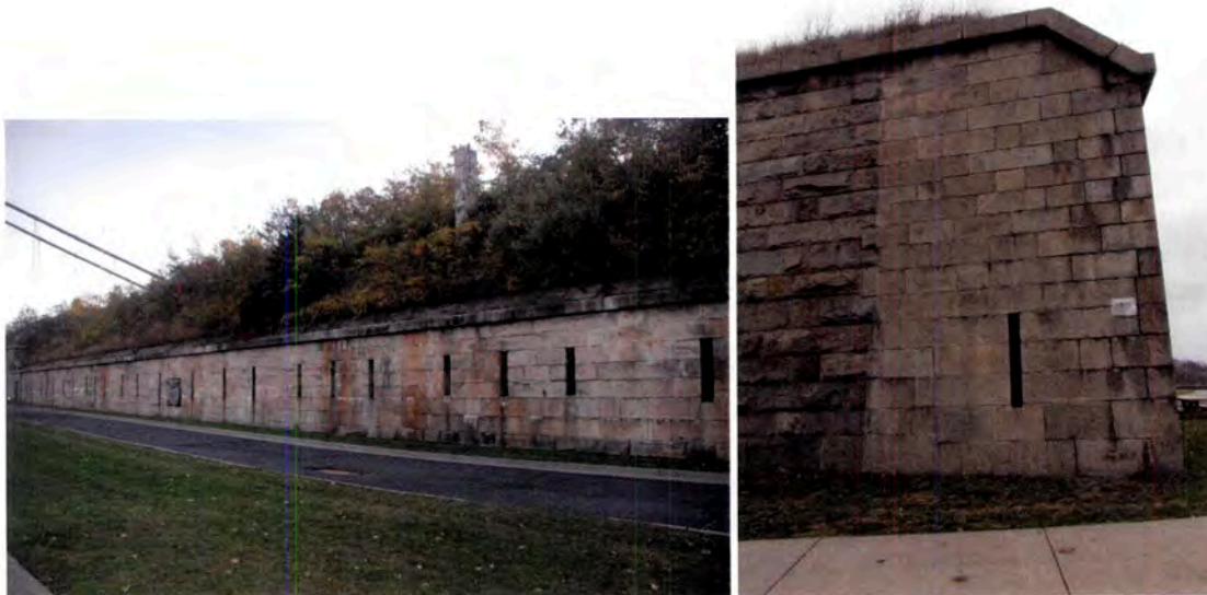
Figure 3: Smooth-faced granite walls of east curtain (left) and east end of south elevation where the rough-hewn granite meets the smooth-face replacement granite where counterscarp was removed (right).
