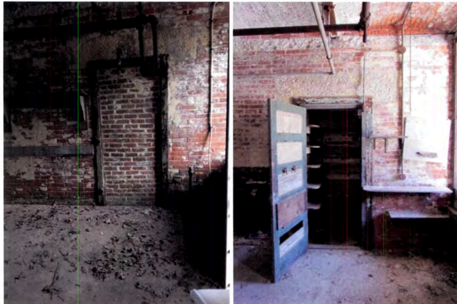
Figure 45: Brick infill in metal cased opening (left) and five-paneled closet door (right).
