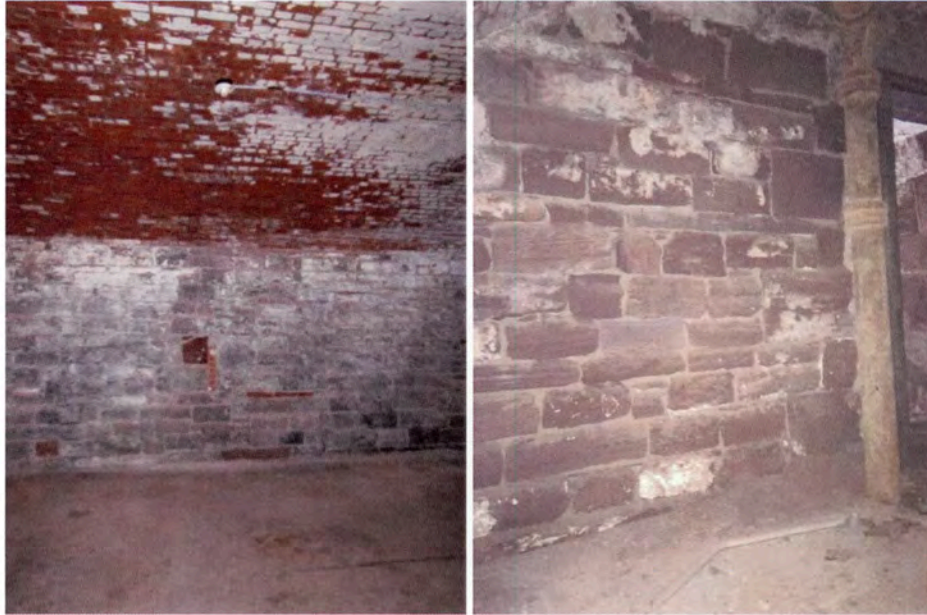
Figure 44: Granite walls (left) and sandstone walls (right) in corner sections of the first floor.
