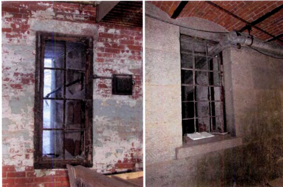
Figure 34: Typical eight-light steel casement windows (left) and nine-over-nine single-hung steel window (right).
