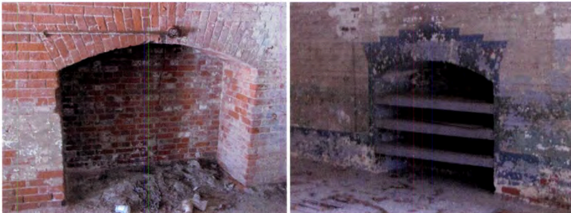
Figure 40: Typical fireplace on first floor (left) and fireplace with wooden shelves in Room 102 (right).
