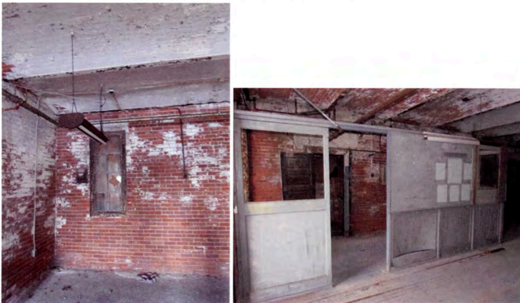
Figure 32: Original brick walls (left) and plasterboard partitions that were likely added during the 1930s (right).
