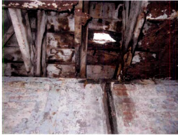
Figure 101: Framing of roof structure in Building 138.
