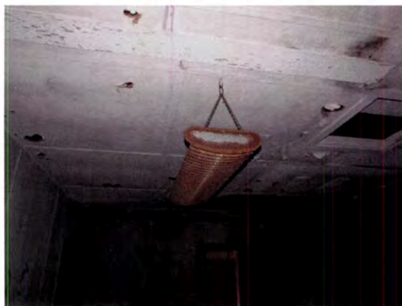
Figure 71: Plywood and batten ceiling in Room 201.
