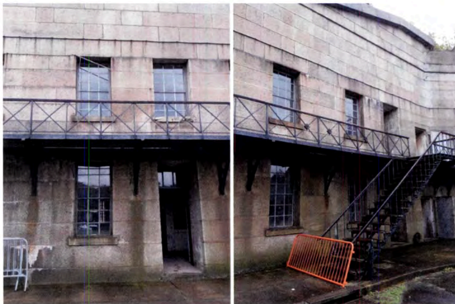
Figure 25: Steel gallery in Parade Ground (left) and stair in southwest corner (right).
