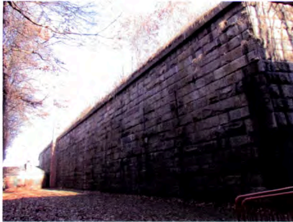
Figure 4: Rough-hewn granite walls on north escarpe wall (west wall similar).
