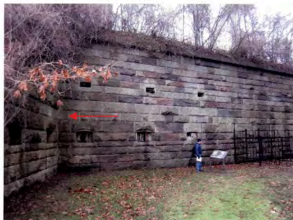
Figure 20: Overview of rough-hewn granite walls of the Counterscarp (arrow is pointing to north elevation).
