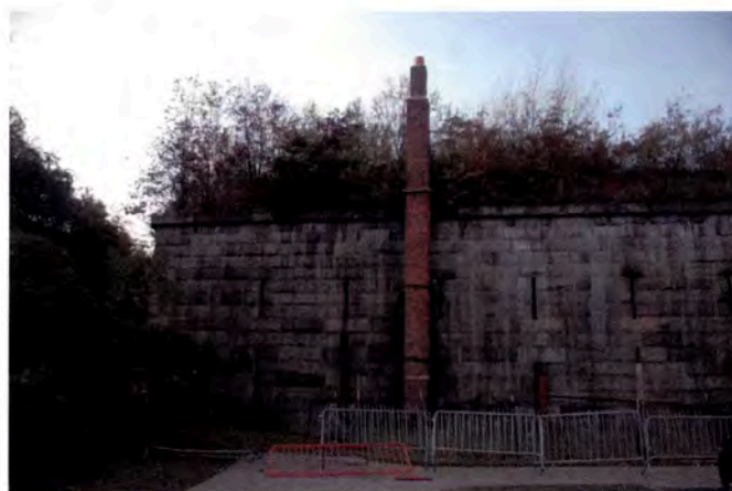
Figure 13: Brick chimney stack at west end of south elevation.
