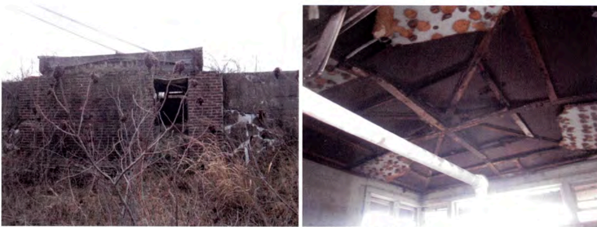
Figure 17: Structure on southeast corner of roof.
