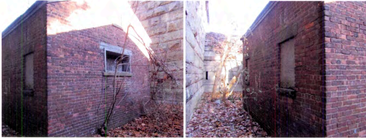
Figure 102: West elevation (left) and north elevation (right) of Building 139.
