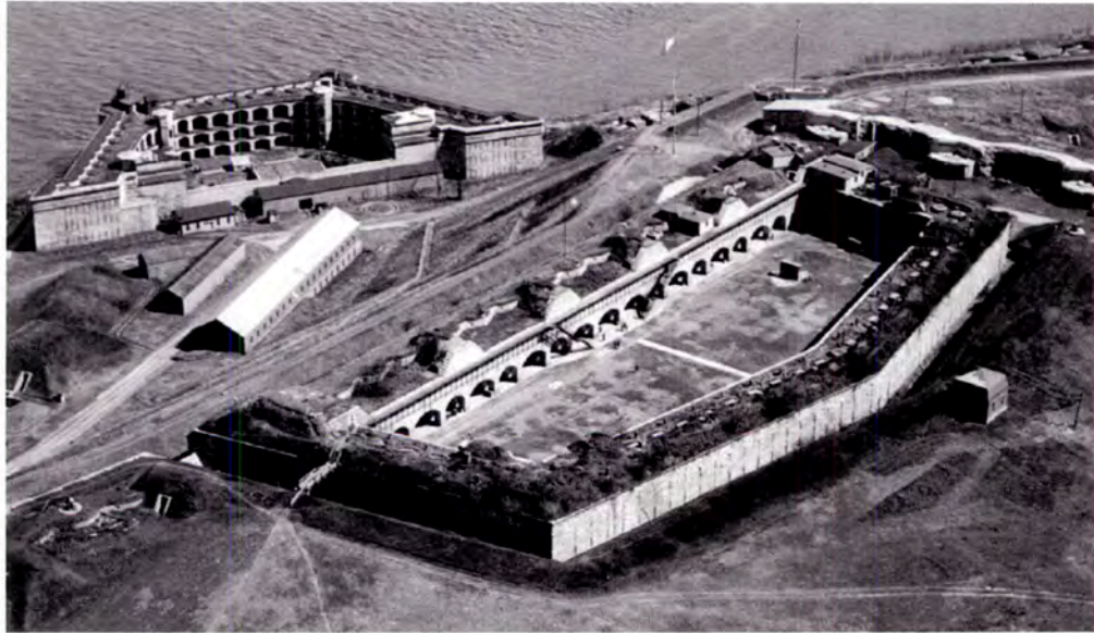
Figure 10: Aerial view of Fort Tompkins, likely dating to the 1930s, showing elements of the rampart including the barbettes, terreplein, and parapet wall. Many roof structures are present, however are currently inaccessible.
