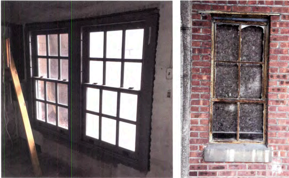
Figure 64: Range of conditions at west end windows at the casemates.
