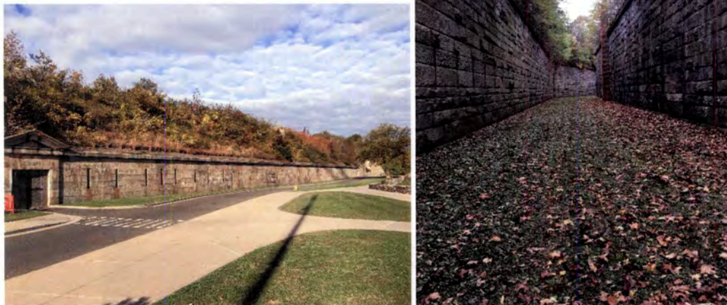
Figure 2: East, main facade of Fort Tompkins (left) and view of counterscarp from southwest corner (right).
