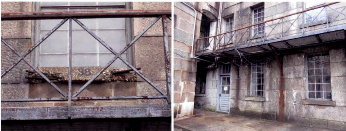
Figure 27: Modified door opening with deteriorating sill and exposed rebar on second story (left) and rust stains on granite walls of Parade Ground (right).
