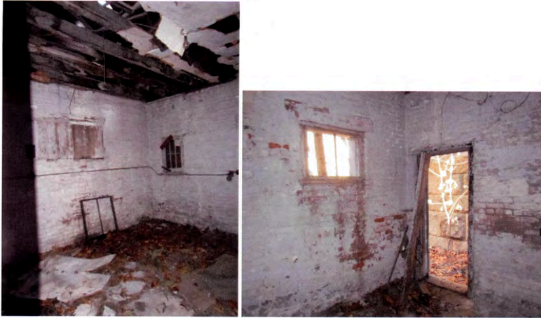
Figure 104: Interior finishes of Building 139.
