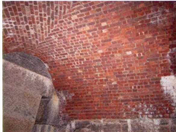
Figure 87: Brick arched ceiling and granite walls in Room 226B.
