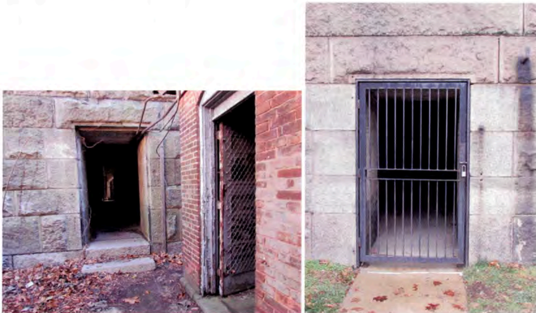
Figure 10: Masonry opening on north elevation (left) and masonry opening with metal gate on south elevation.
