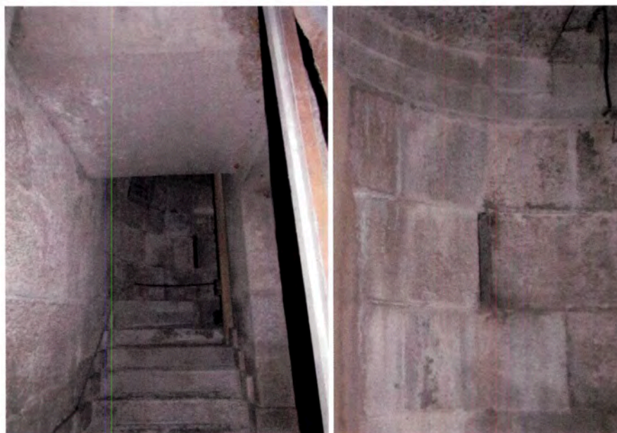
Figure 62: Detail of granite finishes in north stair (left) and typical embrasure in granite wall (right).
