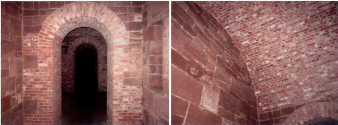
Figure 94: Brick archways in counterscarp (left) and brick arched ceiling with sandstone arched walls (right).
