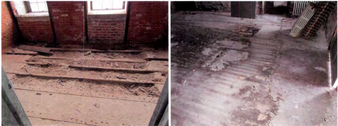
Figure 72: Typical floor conditions on the second floor.
