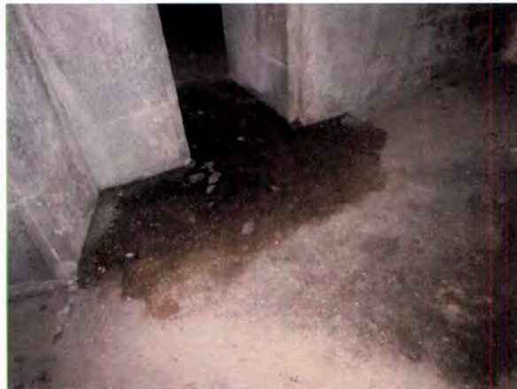
Figure 80: Typical concrete floor in corner section of second floor.
