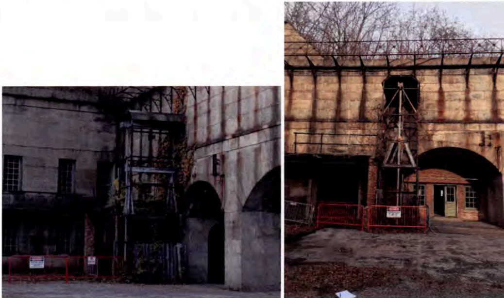
Figure 26: Overviews of Lift Structure in northeast corner of Parade Ground.
