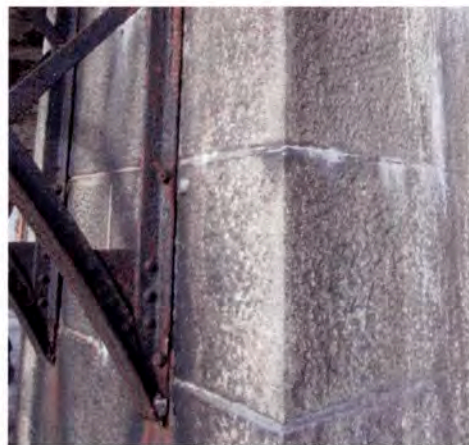
Figure 34: Framing for landing at south stair on east elevation.
