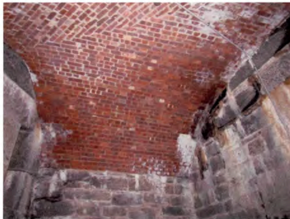
Figure 82: Typical brick arched ceiling and granite walls in corner.
