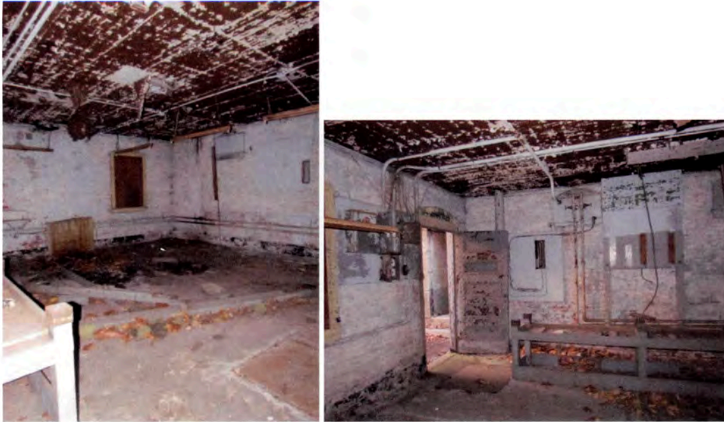
Figure 99: Interior finishes of Building 138.
