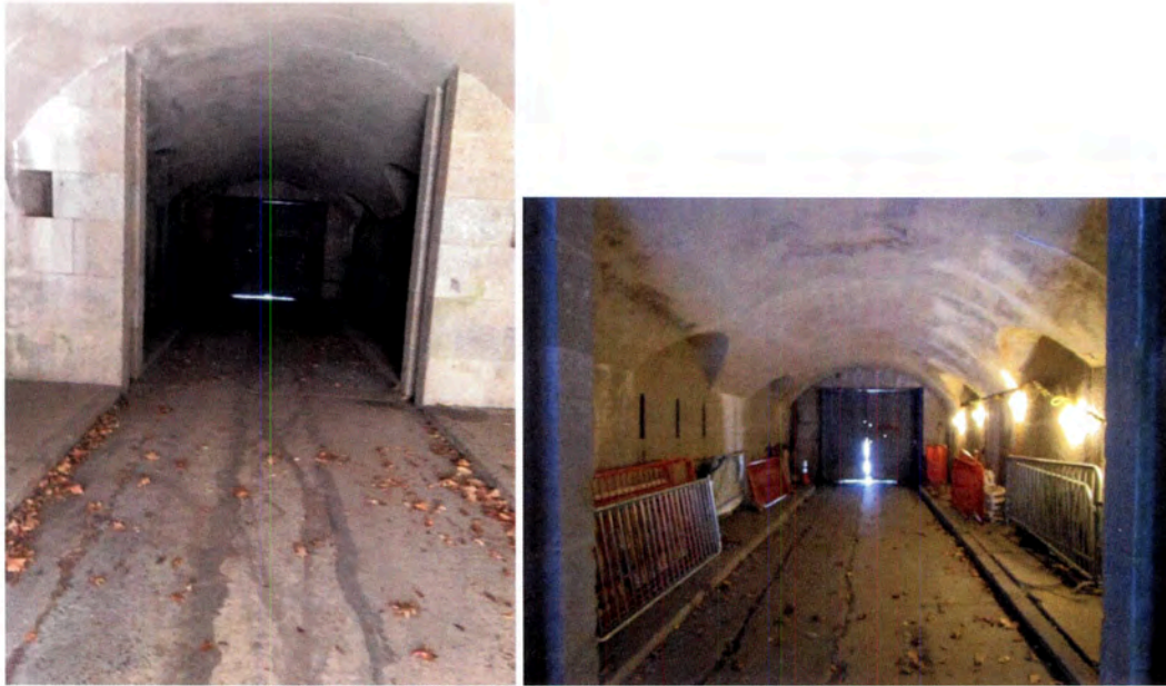
Figure 50: North sally port (left) and south sally port (right).
