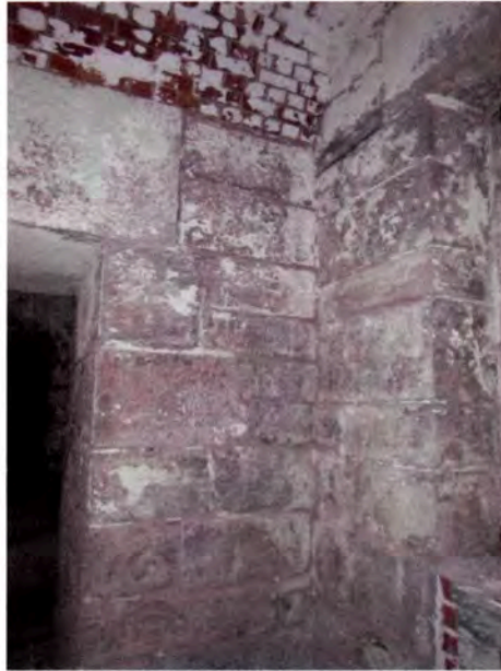
Figure 81: Typical granite walls in the corners of the second floor.
