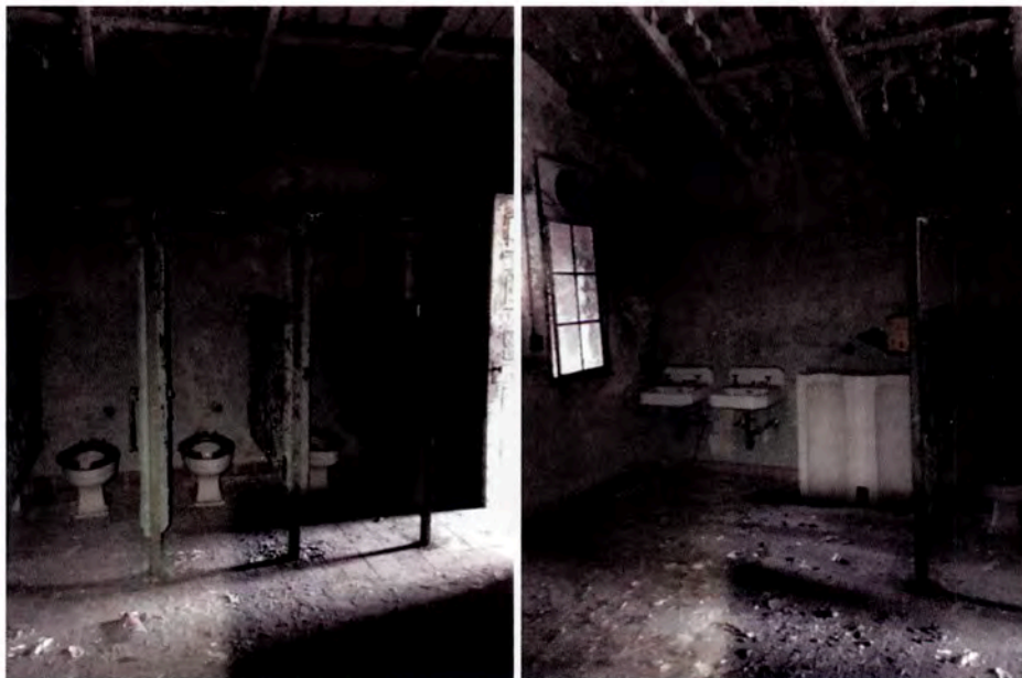
Figure 76: Typical plumbing fixtures and metal partitions in lavatories on second floor.
