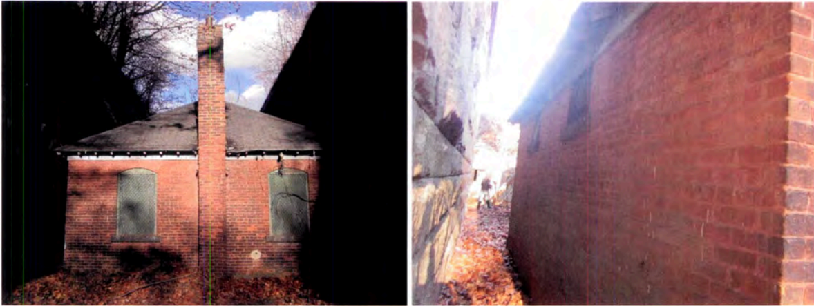
Figure 97: West elevation (left) and north elevation (right) of Building 138.
