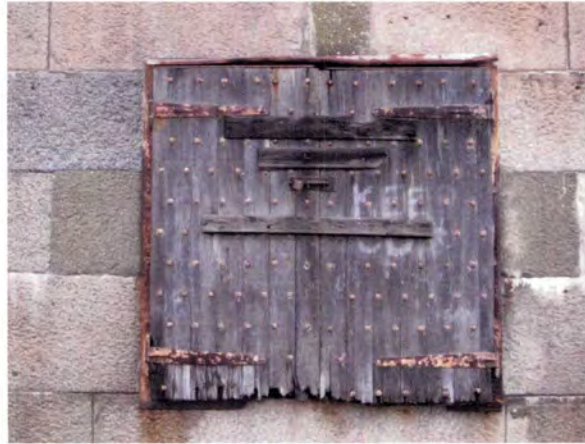
Figure 6: Square, masonry opening on east faced with metal frame and wood security panel.
