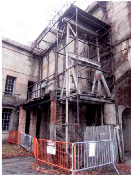
Figure 30: Lift structure in northeast corner of Parade Ground.
