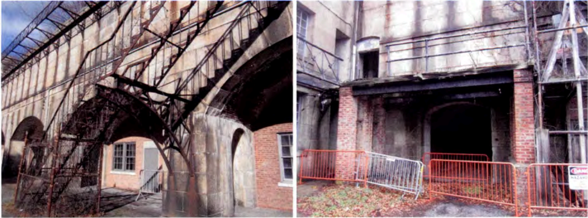
Figure 29: Stairs located on east elevation (left) and walkway at lift structure (right).
