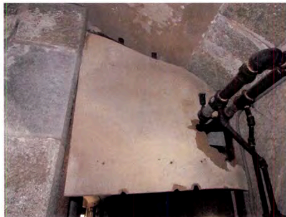
Figure 93: Pipes in north corner of second floor.
