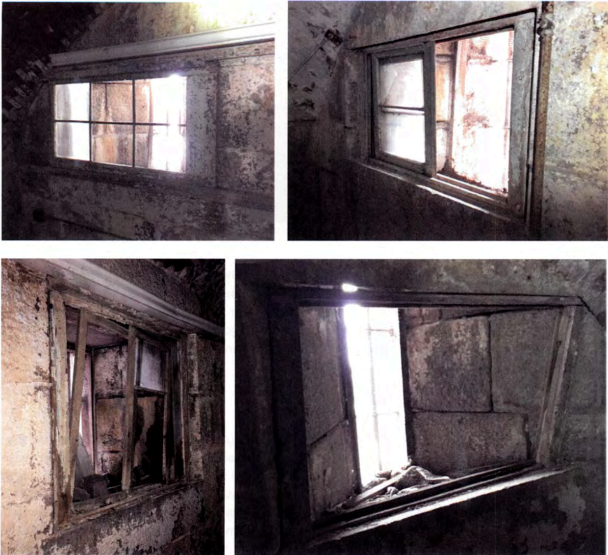
Figure 65: Range of conditions at east end windows at the casemates.
