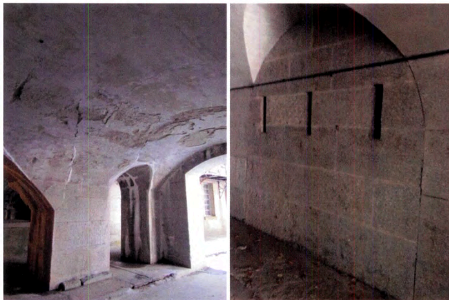
Figure 51: Ceiling in south sally port (left) and typical embrasures found in both sally ports (right).
