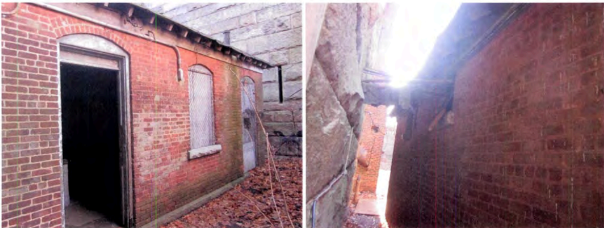
Figure 98: East elevation (left) and south elevation (right) of Building 138.
