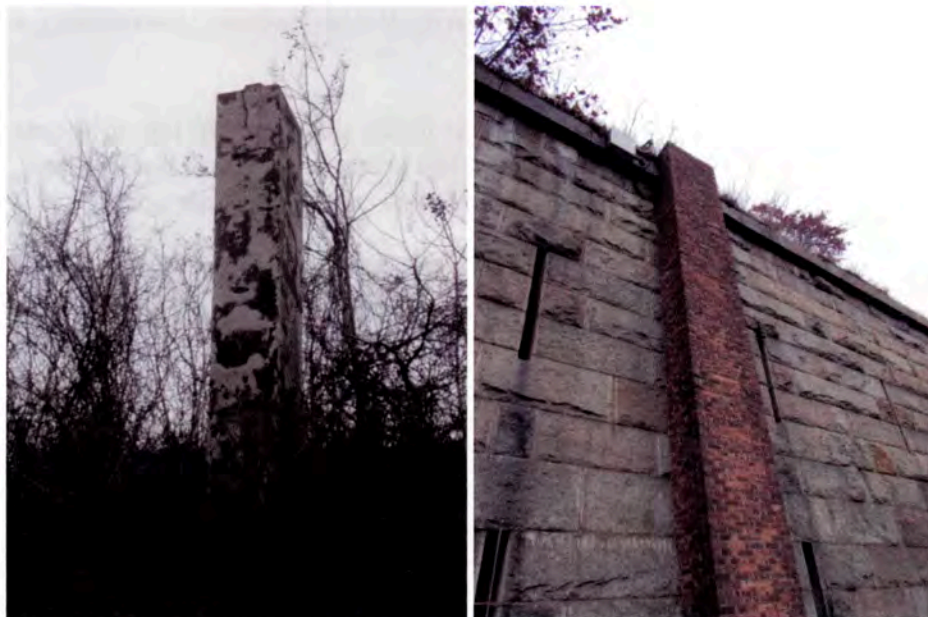
Figure 12: Stuccoed CMU chimney at center of east elevation (left) and brick chimney at east end of south elevation (right).
