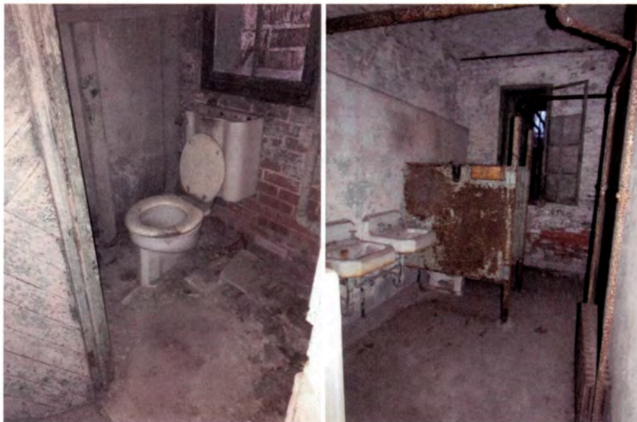
Figure 38: Plumbing fixtures in Room 122 (note wood door herringbone pattern) (left) and lavatories and metal partitions in larger restroom on first floor (right).
