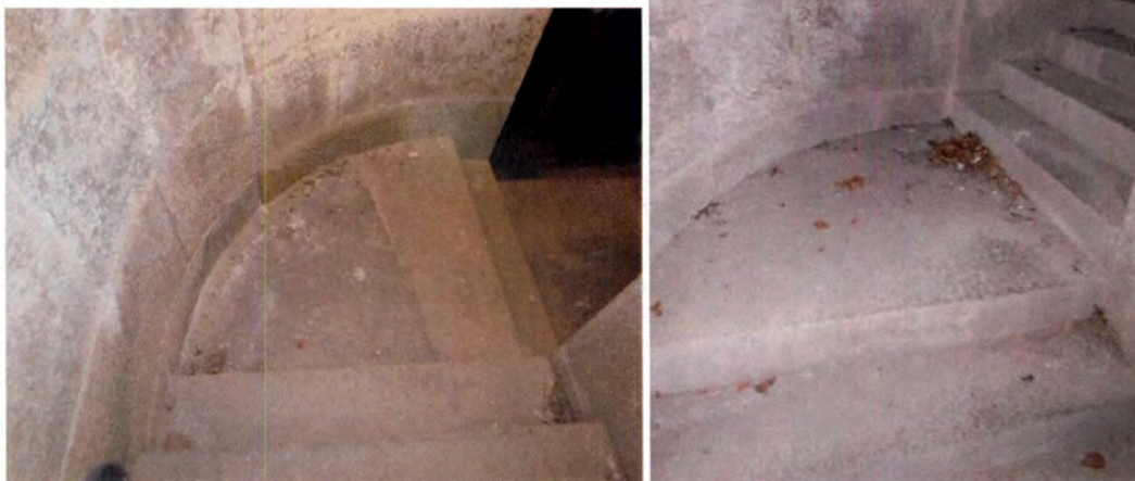
Figure 61: Honed granite stairs and smooth-face granite walls in south stair (left) and north stair (right).
