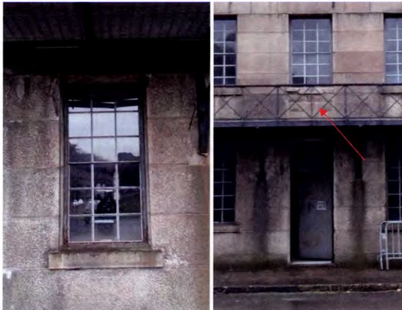
Figure 23: Typical nine-over-nine steel single-hung window (left) and evidence of former door infilled with CMU and steel window.
