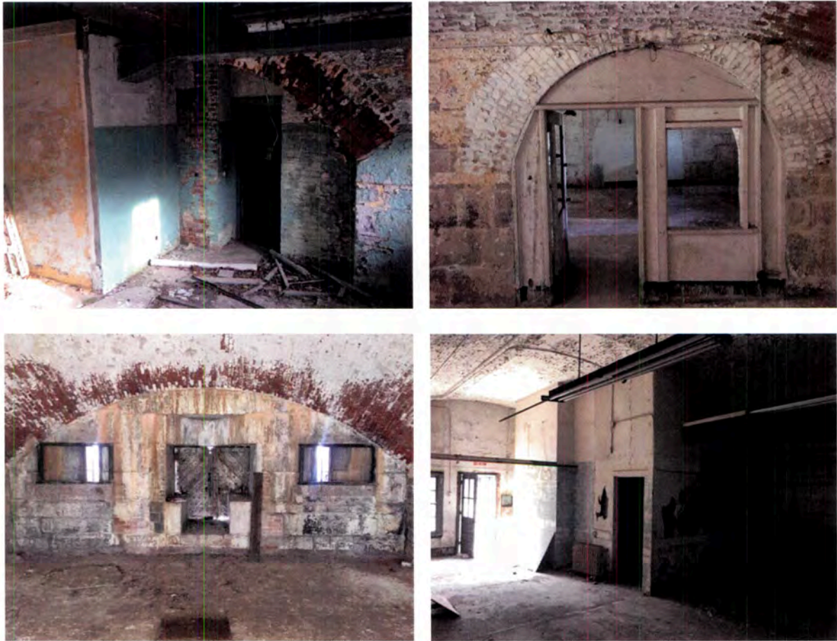
Figure 62: Various wall conditions at the east casemates. Clockwise from upper left: Casemates N, C, E, L.
