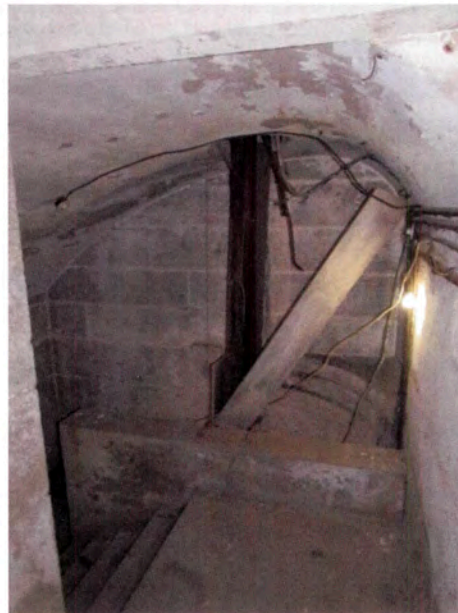
Figure 65: Stair leading to roof.
