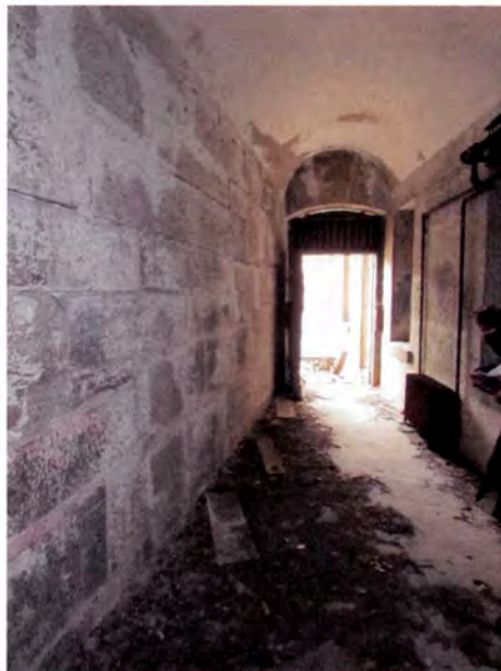
Figure 88: Concrete Floor in Room 236.
