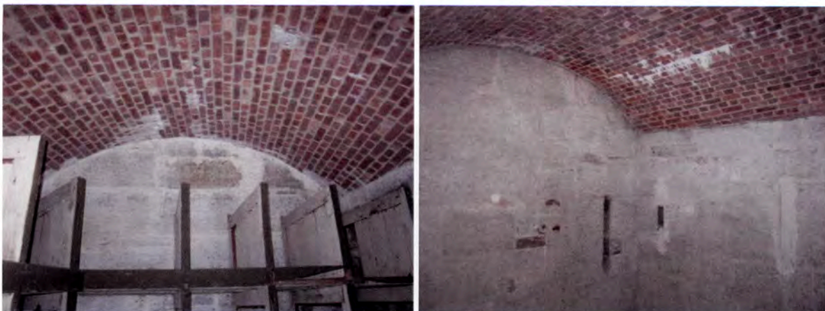
Figure 60: Granite walls and brick arched ceilings.
