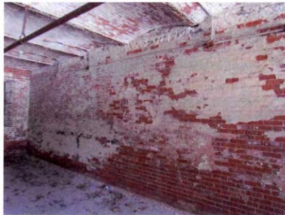
Figure 42: Typical conditions of first floor brick walls.
