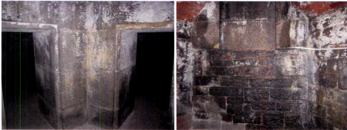
Figure 48: Granite walls in Room 112.
