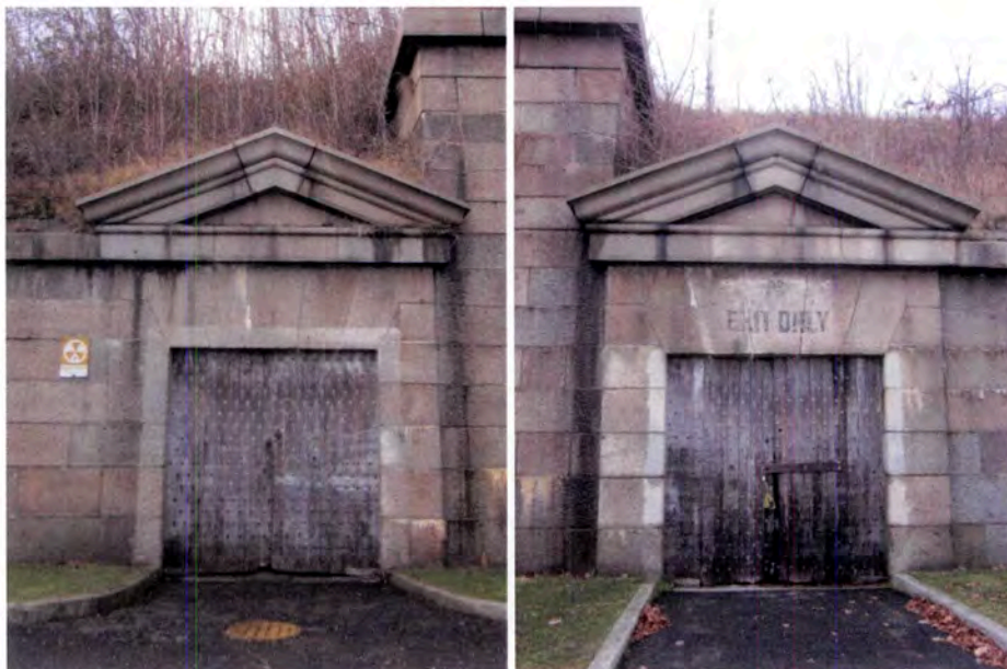
Figure 7: Doors at north end of east elevation (left) and south end of east elevation (right).
