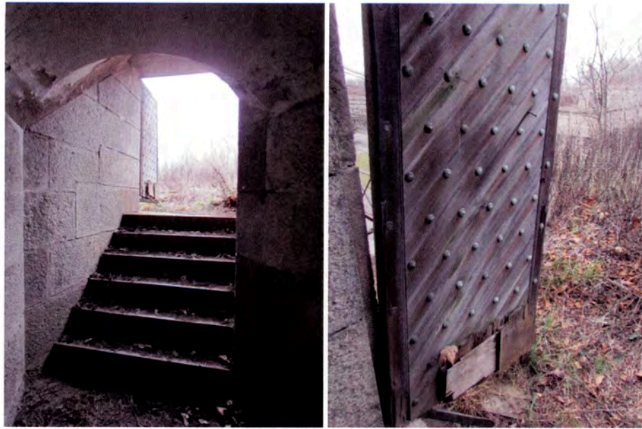
Figure 63: Stairs leading to doorway at roof (left) and detail of door at roof (right) in north stair.
