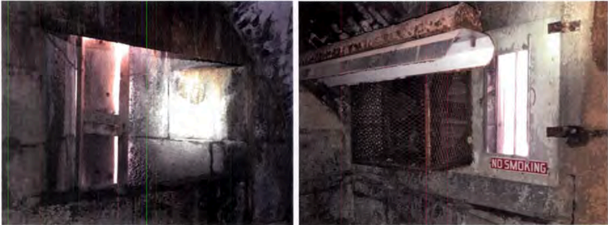
Figure 66: Modern plywood infill at embrasure (left) and older plywood infill fitted with mechanical equipment at Casemate O (right).
