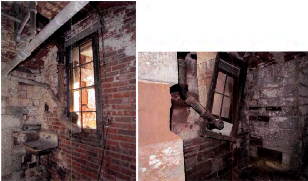
Figure 46: Typical eight-light steel casement window (left) and four-light sash in modified metal frame (right).
