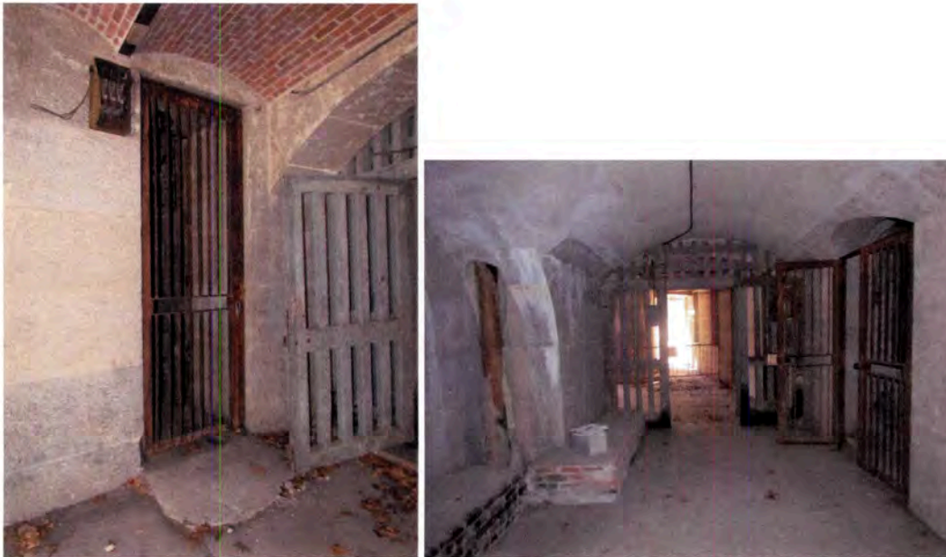
Figure 59: Metal security gate (locked) to Room 147 (left) and open timber lattice frame and door in Room 150 (right).
