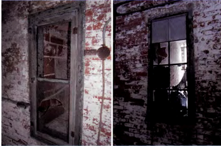
Figure 44: Wood framed window with wood storm panel (left) and typical eight-light steel casement window (right).
