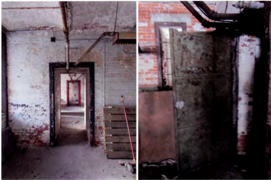
Figure 35: Typical cased metal opening on first floor (left) and thin metal paneled door (right).
