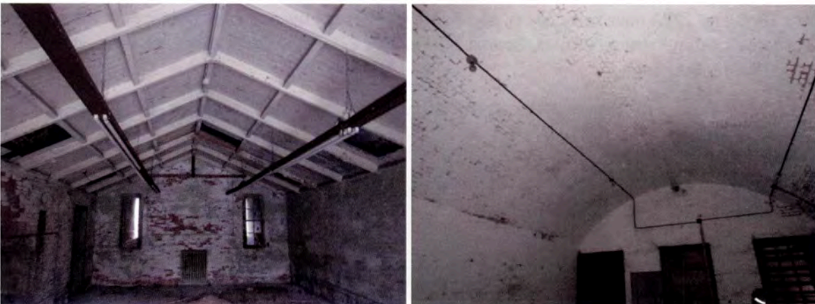
Figure 79: Bead board ceiling with exposed wood rafters (left) and barrel vaulted ceiling (right).
