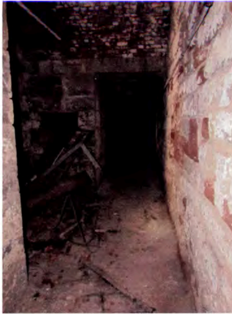
Figure 47: Typical granite doorway in corner section of first floor.
