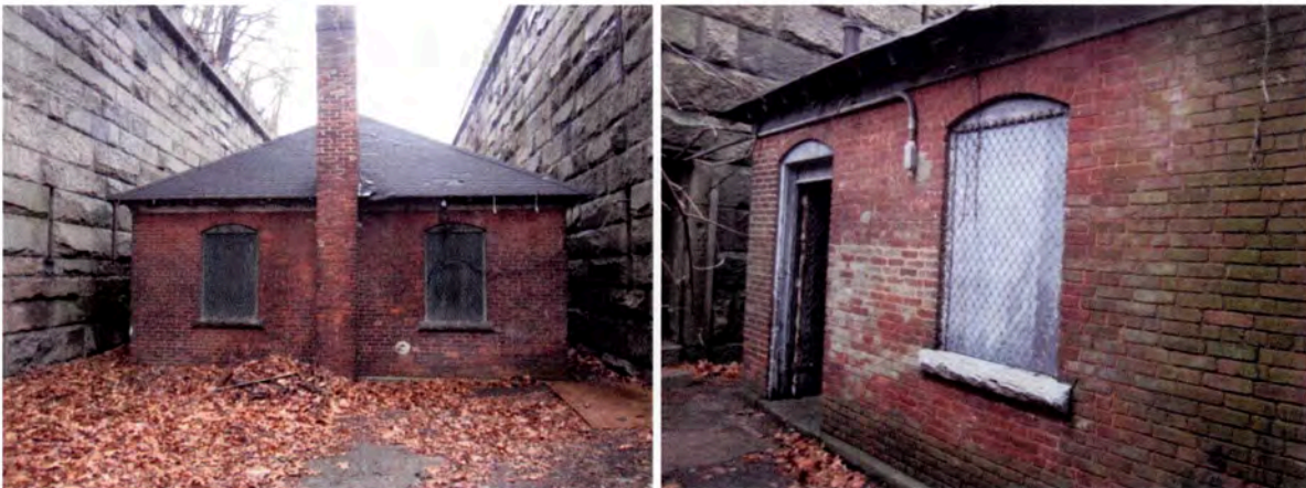
Figure 100: West elevation (left) and east elevation (right) of Building 138.
