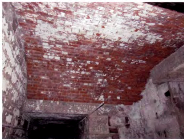
Figure 54: Typical brick arched ceiling in corner sections.
