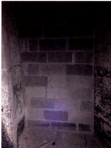
Figure 45: CMU infill in first floor corners.
