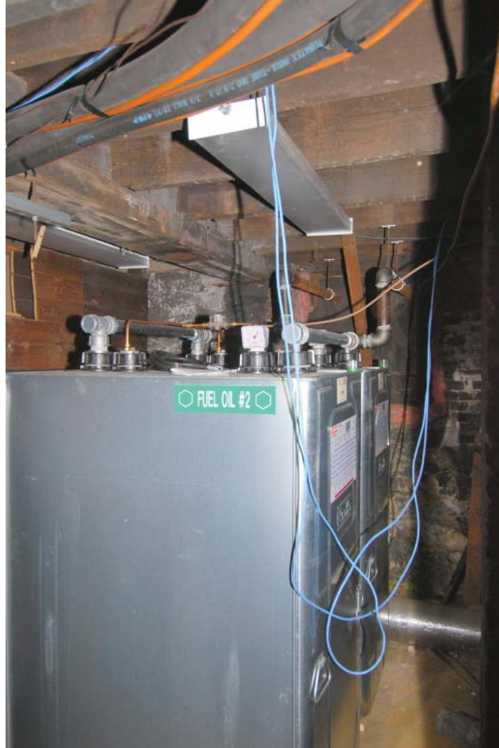
Photo 51. Coal Bin looking northwest (JMA, October 2009)
