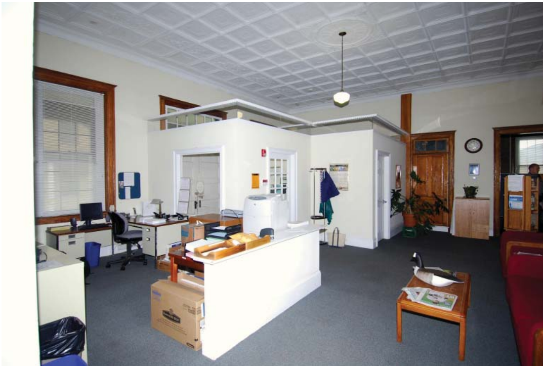
Photo 85. View of the main entrance foyer from public lobby looking northwest. The central space has smooth and continuous circulation spaces (JMA, October 2009).
