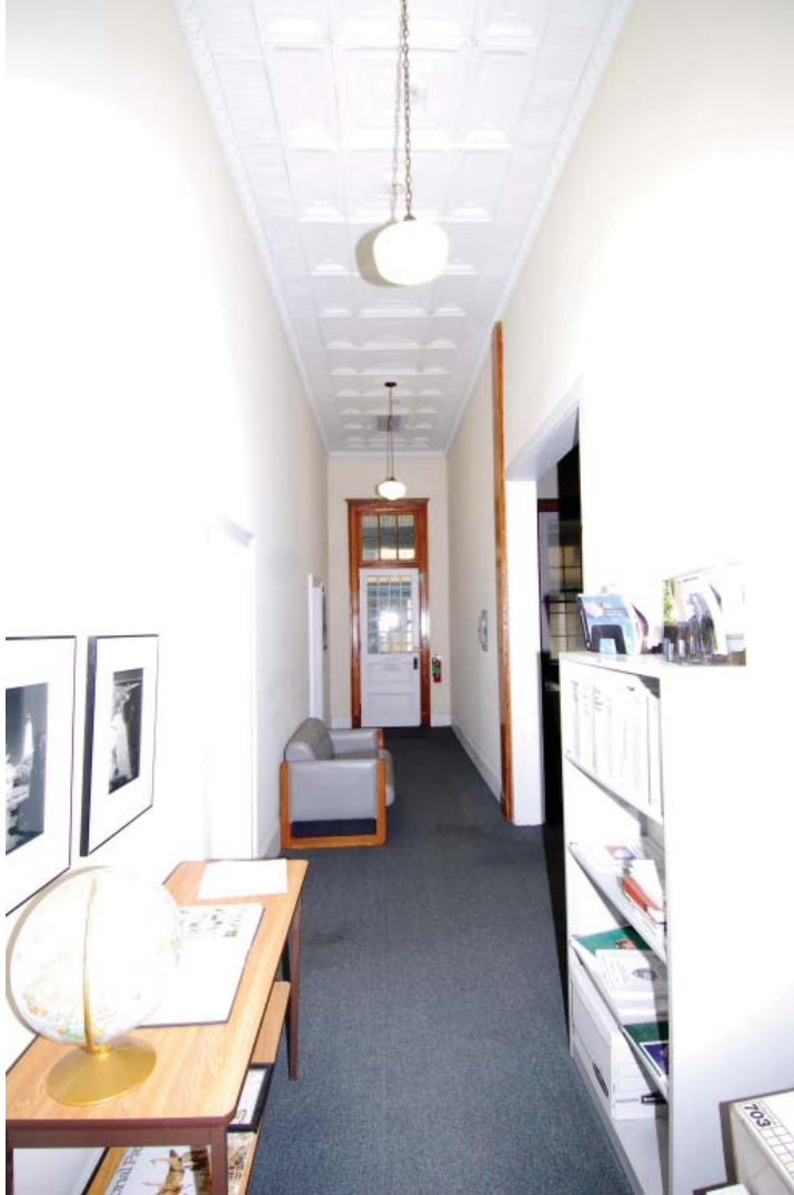
Photo 86. View of southern hall looking west. The existing Hall provides an accessible circulation path. Existing furniture currently located along the Hall should be relocated to keep the path open (JMA, October 2009).
