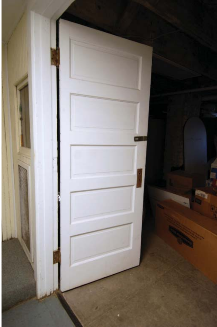
Photo 80. One leaf of the double doors to the Boiler Room. These doors may be historic but are not in their original location. (JMA, October 2009)
