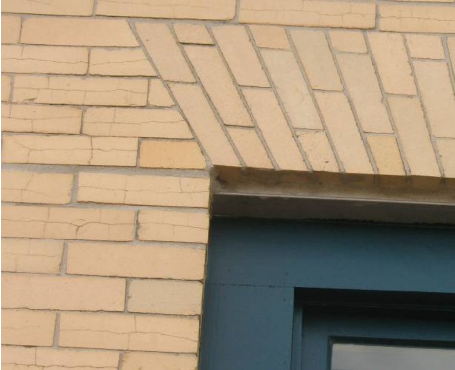
Photo 3: Lintel Replacement. Notice distortion of wall due to rust jacking from previous lintel.
