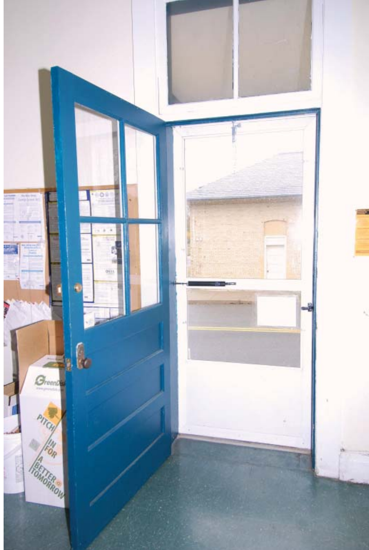
Photo 91. Entrance door from east porch has ADA compliant width but retains original hardware (JMA, October 2009).
