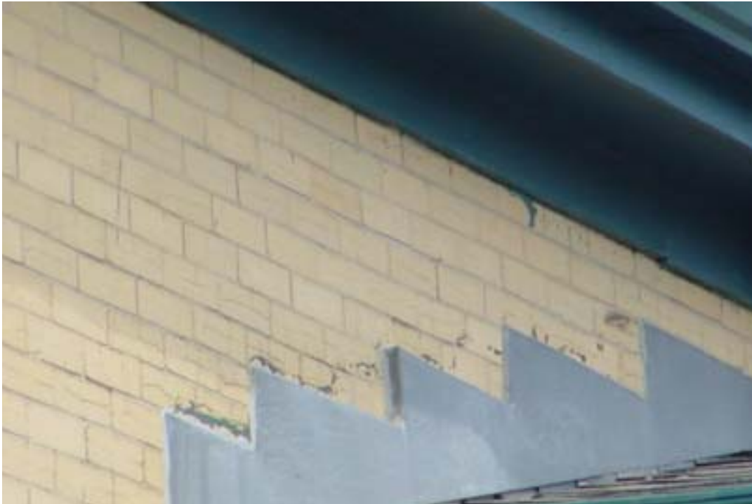
Photo 27. Detail of stepped terne-coated flashing at the east porch roof (JMA, August 2010)
