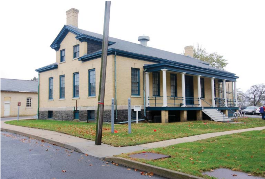
Photo 26. View of Building #58 looking southeast (JMA, October 2009)
