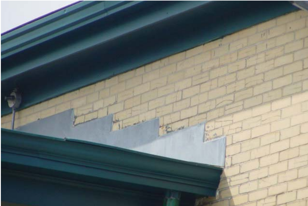
Photo 73. Detail of the stepped flashing at the east porch roof. (JMA, August 2010)
