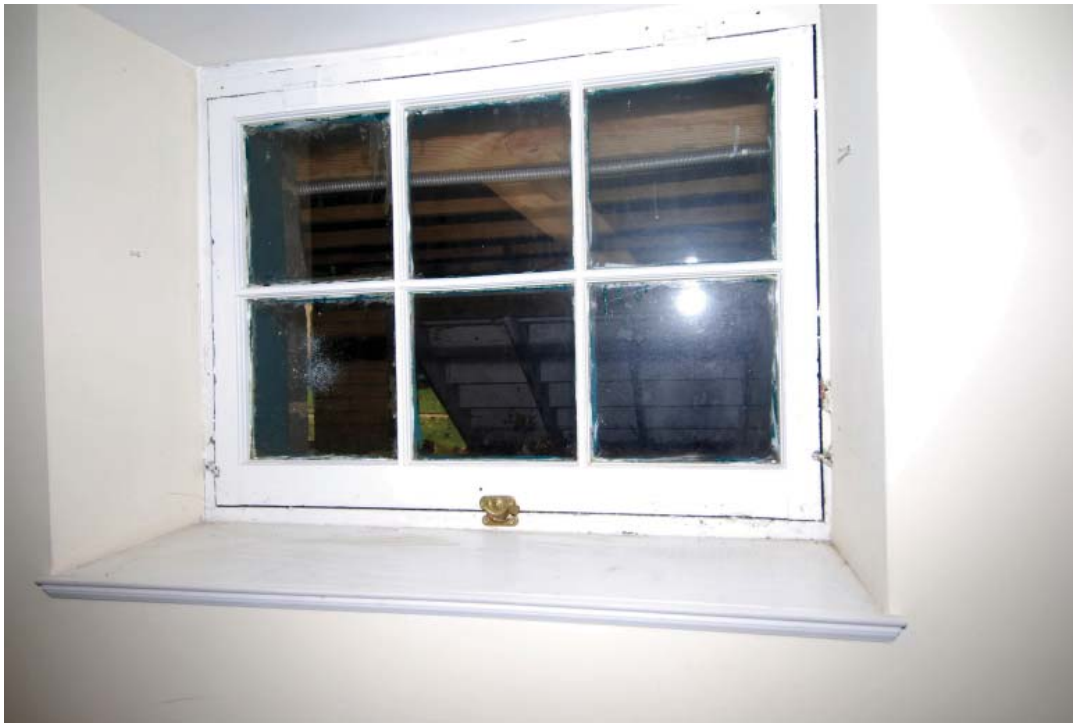
Photo 71. Interior side of a typical awning window at the basement level. (JMA, October 2009)
