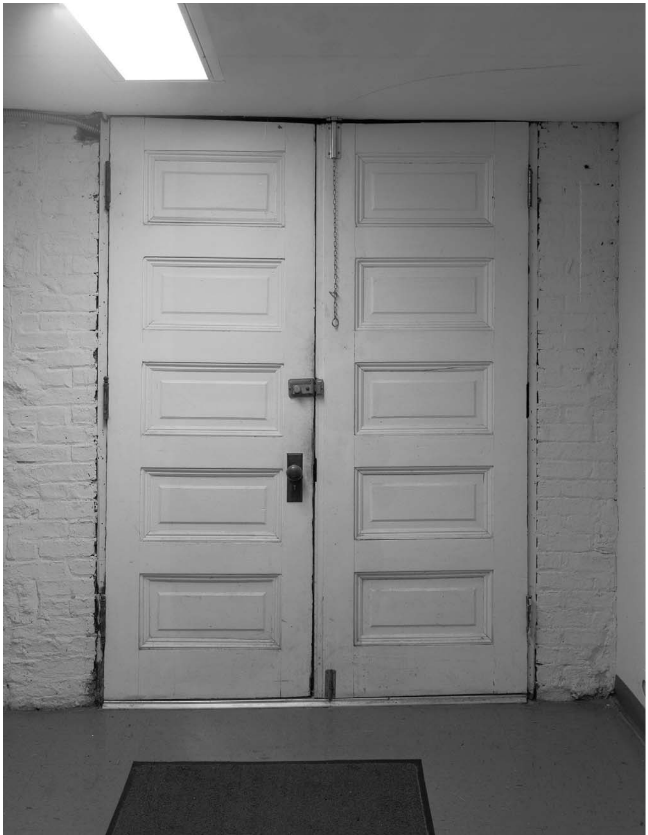
Photo B-27. Building #58, basement interior, original double leaf basement entry doors on west. Fort Hancock, Sandy Hook Unit, Gateway National Recreation Area. Sandy Hook, New Jersey. Photographer: Doug Harnsberger. September 2010.
