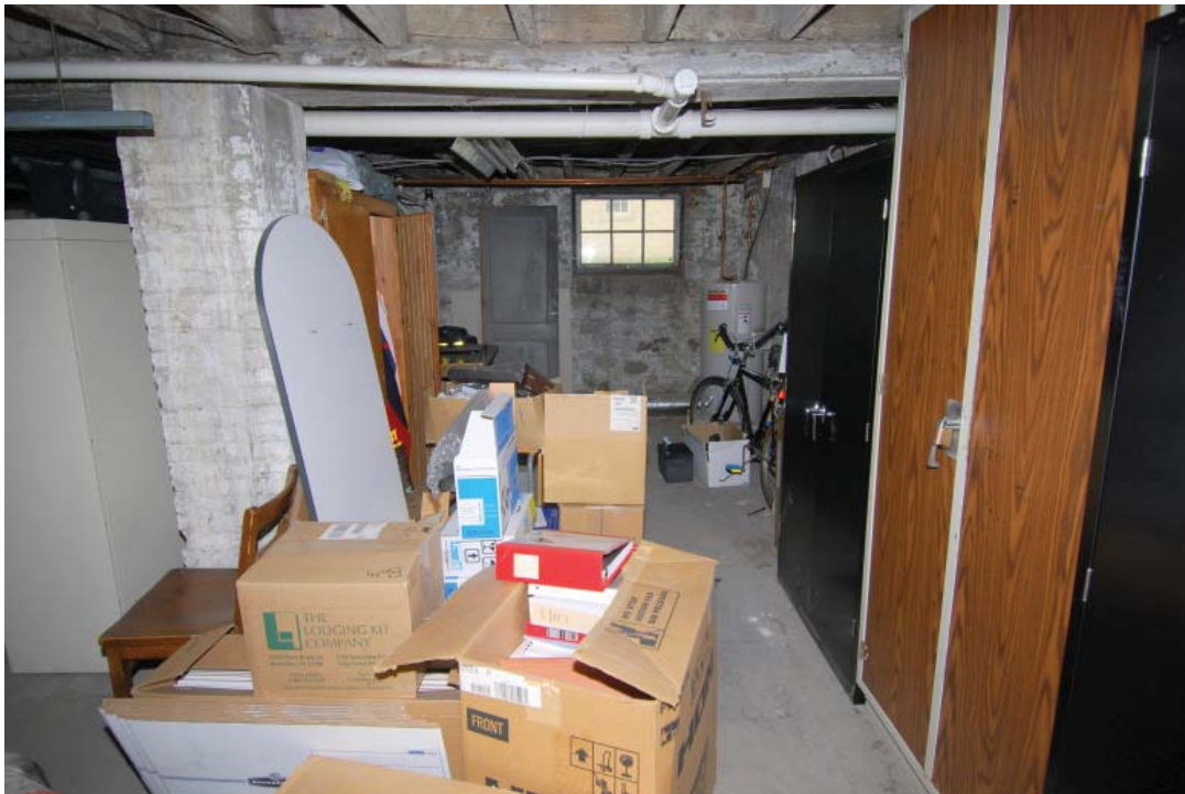
Photo 47. Boiler Room, south end looking east (JMA, October 2009)
