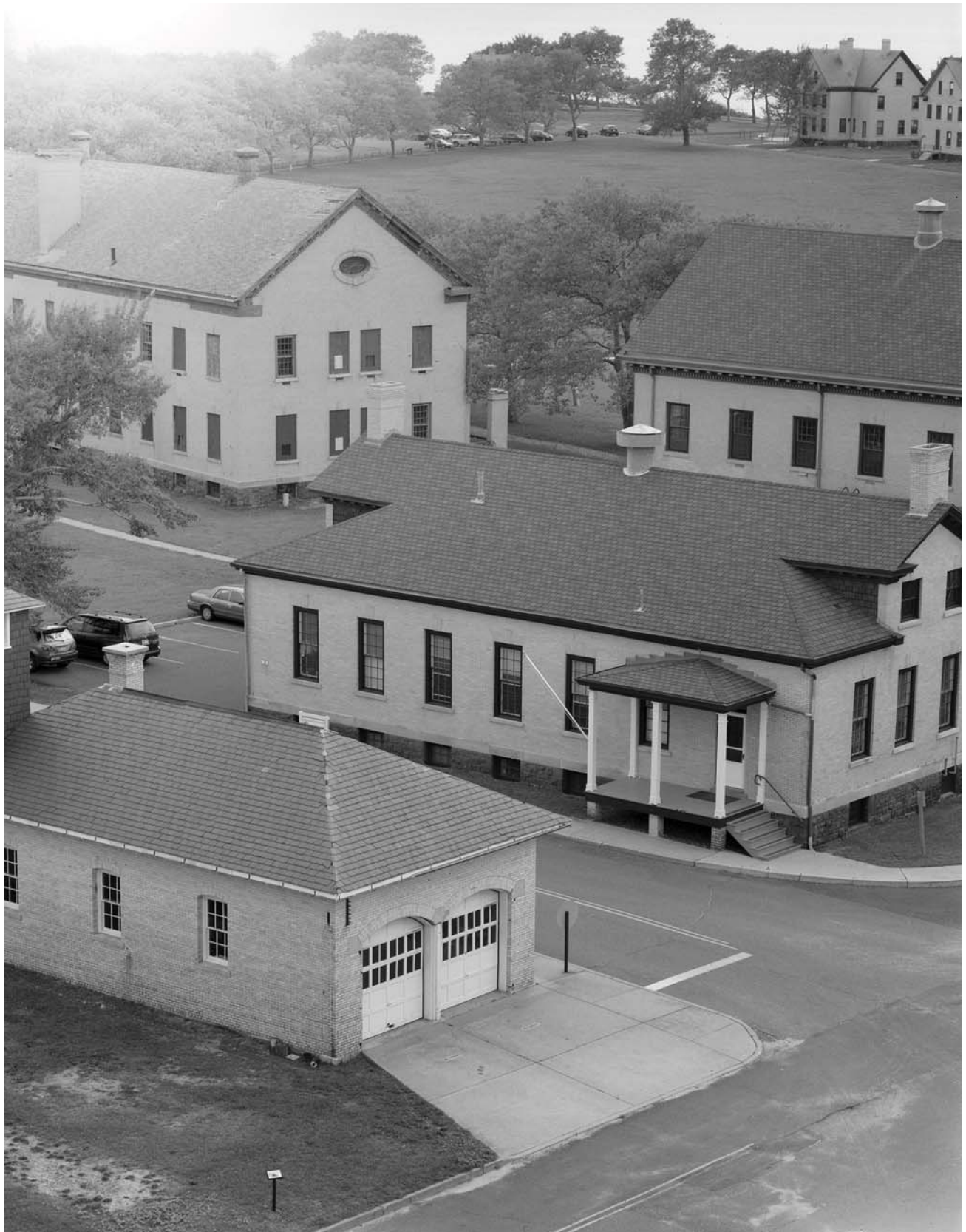
Photo B-11. Detail view of Building #58 from Sandy Hook Lighthouse. Fort Hancock, Sandy Hook Unit, Gateway National Recreation Area. Sandy Hook, New Jersey. Photographer: Doug Harnsberger. September 2010.
