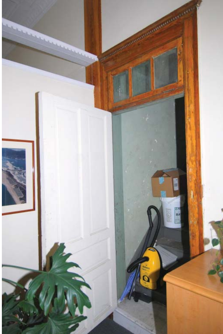
Photo 45. Door at northwest corner of the mess hall space leads to the attic stair (JMA, October 2009)
