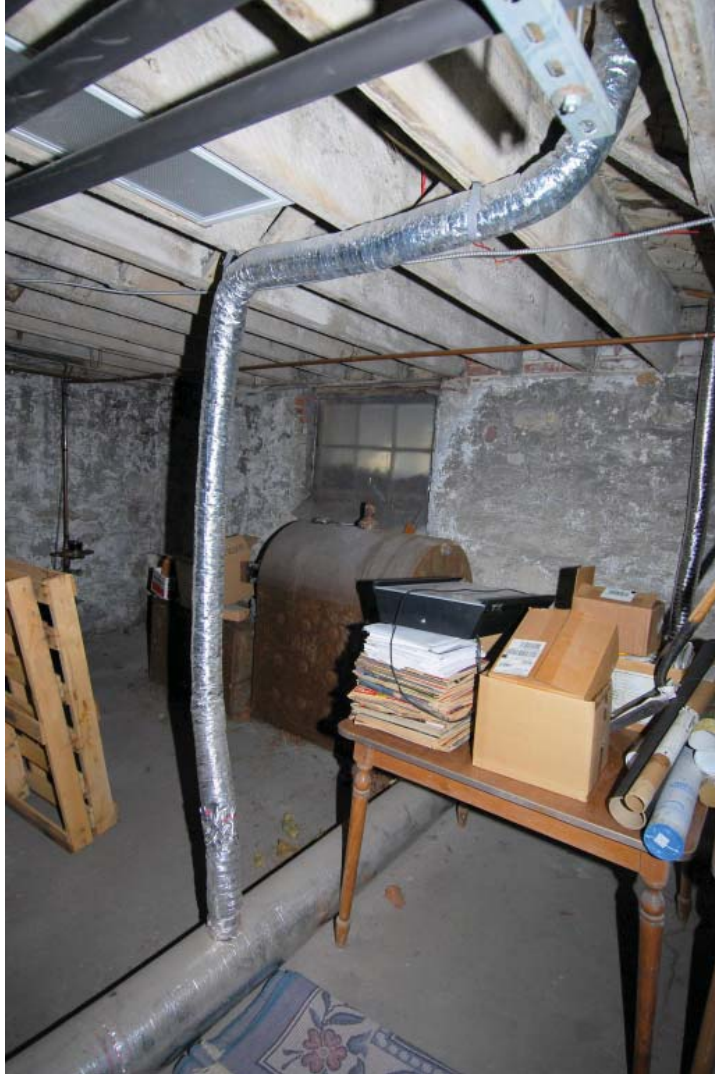
Photo 48. Boiler Room looking northeast. Note oil tank no longer in use (JMA, October 2009).
