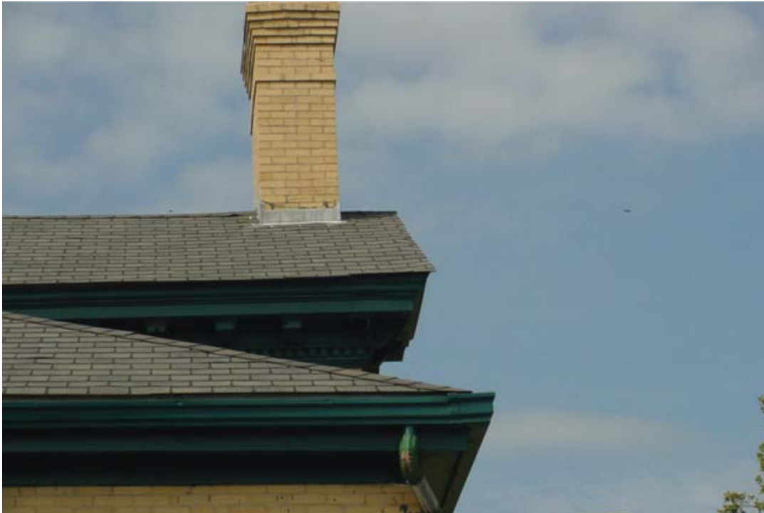
Photo 75. The dormers at Building #58 retain the original dentils at the cornice. The lower roof edge has a fascia mounted molded metal gutter. (JMA, August 2010)
