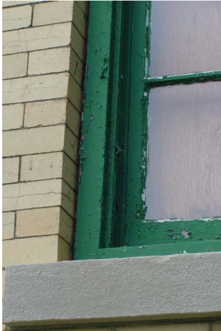
Photo 69. Detail of the original window at Building #57. Note the thinner casing and original hardware. (JMA, August 2010)
