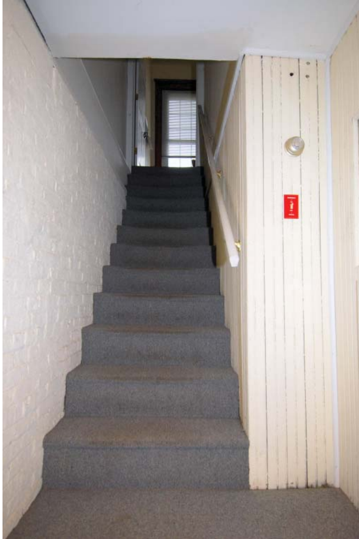
Photo 44. Stairs from the basement to first floor, looking north (JMA, October 2009)
