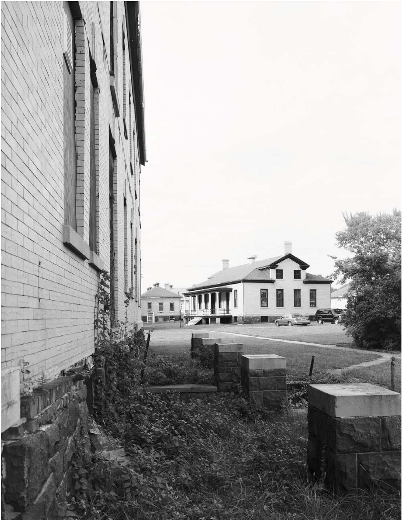
Photo B-13. Building #58, looking northeast from missing rear porch at Barracks Building #24. Fort Hancock, Sandy Hook Unit, Gateway National Recreation Area. Sandy Hook, New Jersey. Photographer: Doug Harnsberger. September 2010.
