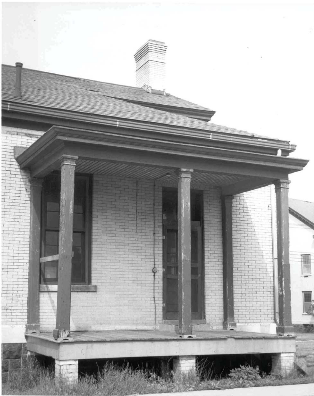
5. Undated photograph showing rear east kitchen porch of unidentified mess hall. Note concrete topping at door threshold. Photo #7915, Gateway National Recreation Area Archives.
