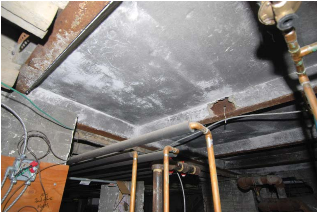
Photo 49. Boiler Room concrete and metal ceiling at north end (JMA, October 2009)
