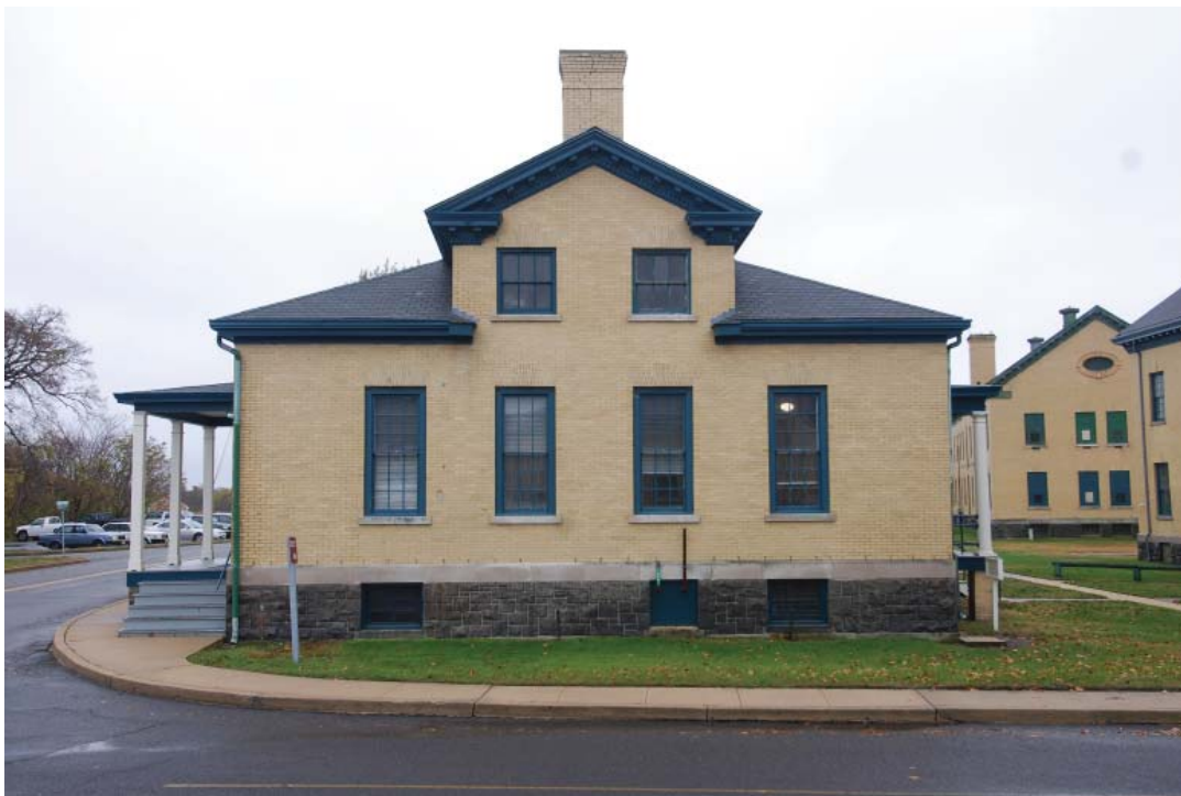
Photo 70. North elevation of Building #58. Note the three-over-three attic windows, nine-over-nine first floor windows, and variety of basement windows and grates. Basement window 001A appears to be a six-over-six top sash from a double hung wood window. (JMA, October 2009)
