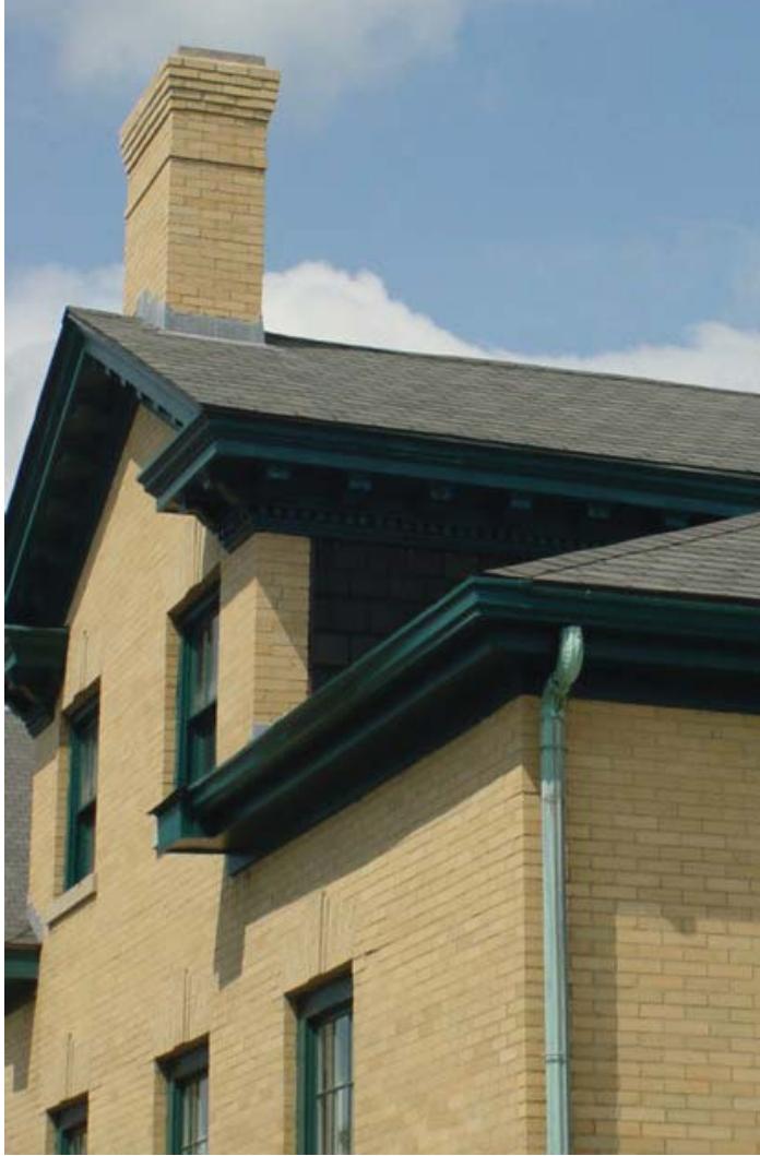
Photo 28. Detail of southeast roof with the historic metal cornice at the dormer and simpler replacement metal box gutter at the lower roof (JMA, August 2010)
