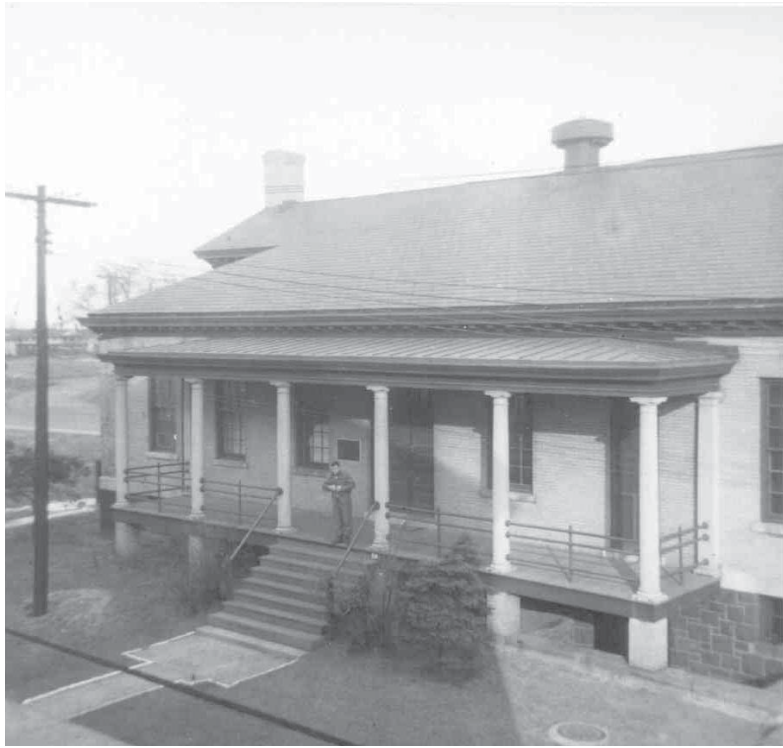
Photo 11. West façade of Mess Hall #57 looking toward northeast, c. 1956. Note porch columns painted white. (#11210, Gateway National Recreation Area Museum archives)
