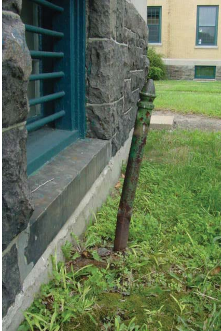
Photo 14. Historic cast iron bollard located on the north side at the foundation (JMA, August 2010)
