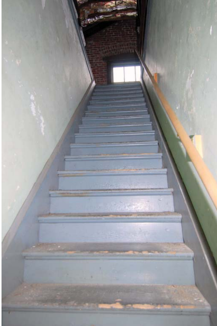
Photo 46. Stairs from the first floor to the attic, looking north (JMA, October 2009)
