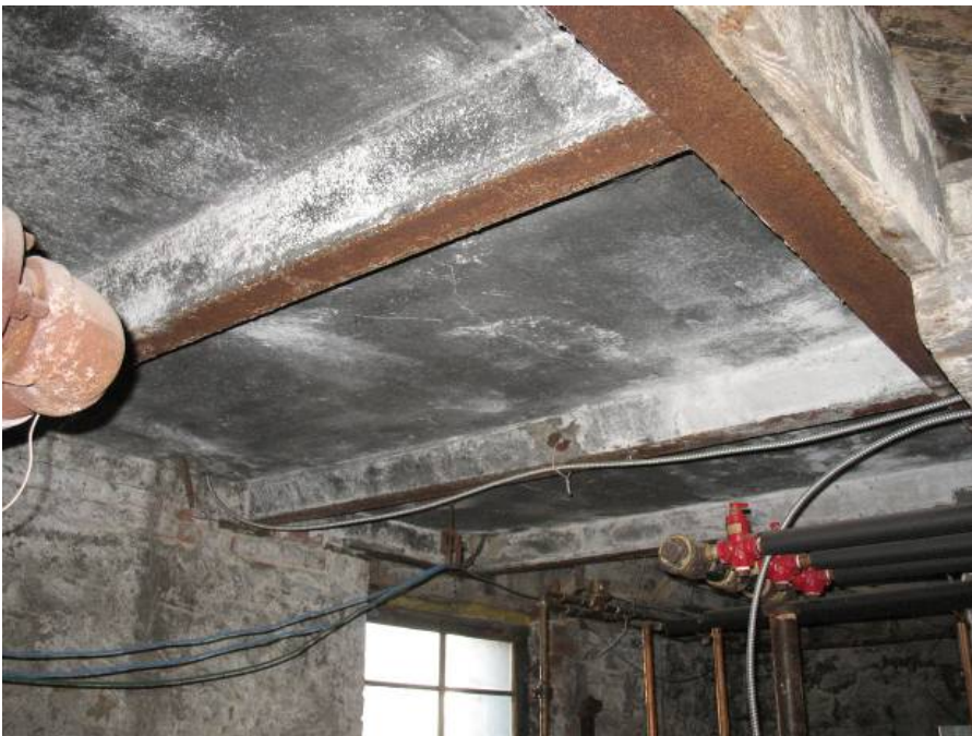
Photo 4: Steel and concrete framing at north end of first floor.
