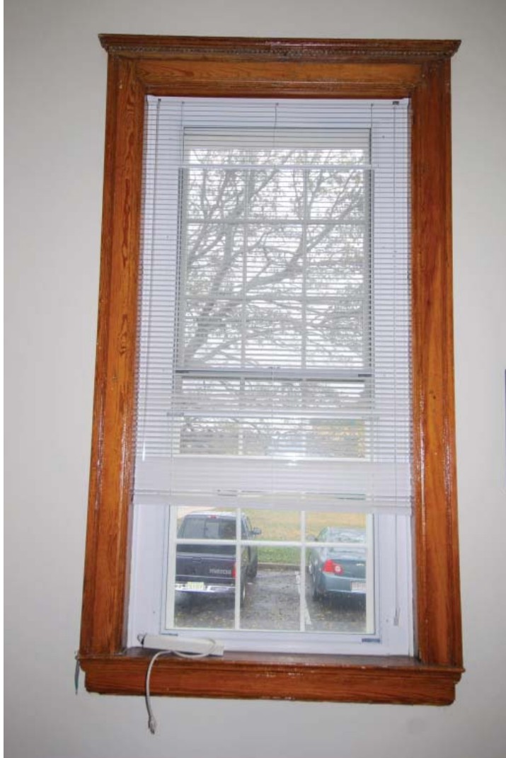
Photo 78. Interior view of a typical first floor replacement window. Note the wide casing and the interior trim, which has been stripped of its paint. (JMA, October 2009)
