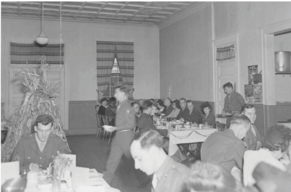
Photo 7. Interior view of typical mess hall room looking towards northwest corner. Five-panel door to attic and framed opening to kitchen on the right (#4629, Gateway National Recreation Area Museum archives)
