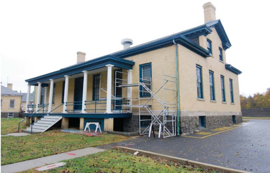
Photo 20. View of Building #58 looking northeast (JMA, October 2009)
