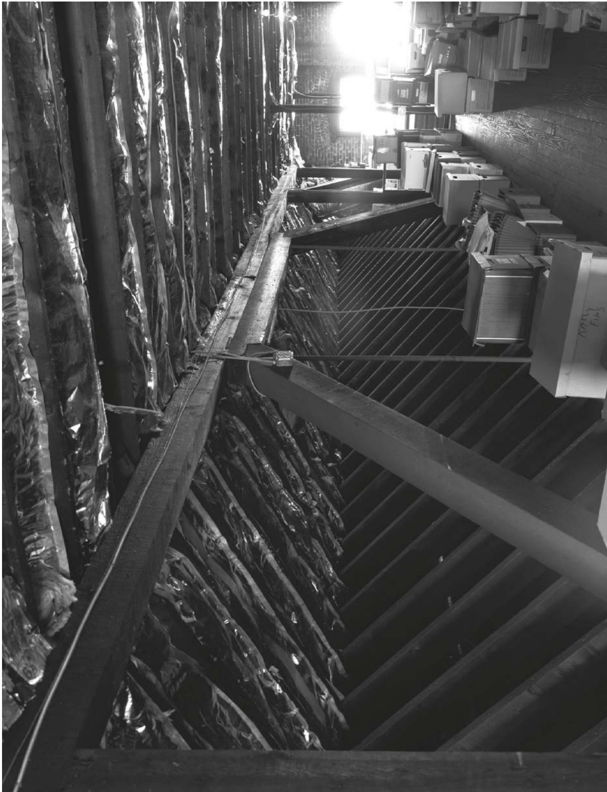
Photo B-31. Building #58, attic interior looking north. Fort Hancock, Sandy Hook Unit, Gateway National Recreation Area. Sandy Hook, New Jersey. Photographer: Doug Harnsberger. September 2010.
