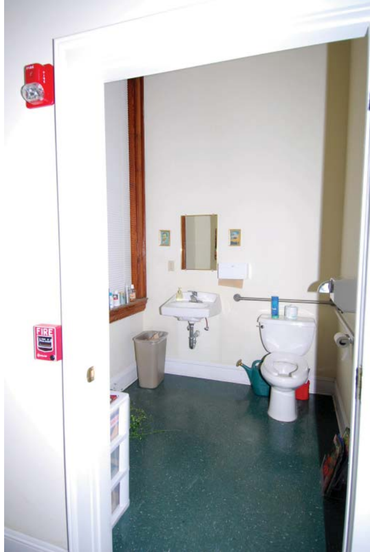
Photo 95. View of eastern ADA compliant toilet. These bathrooms show inconsistent efforts to address accessibility needs on the interior (JMA, October 2009).
