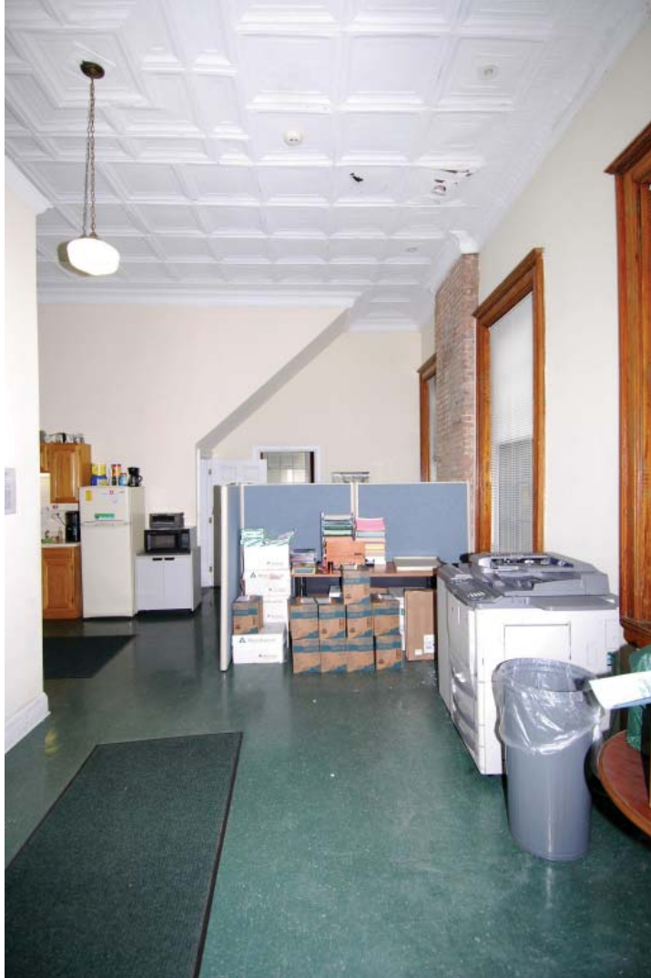
Photo 39. Historic kitchen area looking west (JMA, October 2009)
