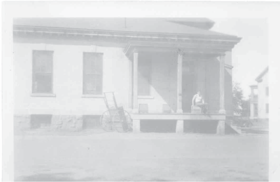
Photo 9. Mess Hall Building #56 showing the rear east kitchen porch. Some historic aerial images show the rear porch of Building #58 as partially enclosed, though the extent of the enclosure is not clear (#759.9, Gateway National Recreation Area Museum archives).
