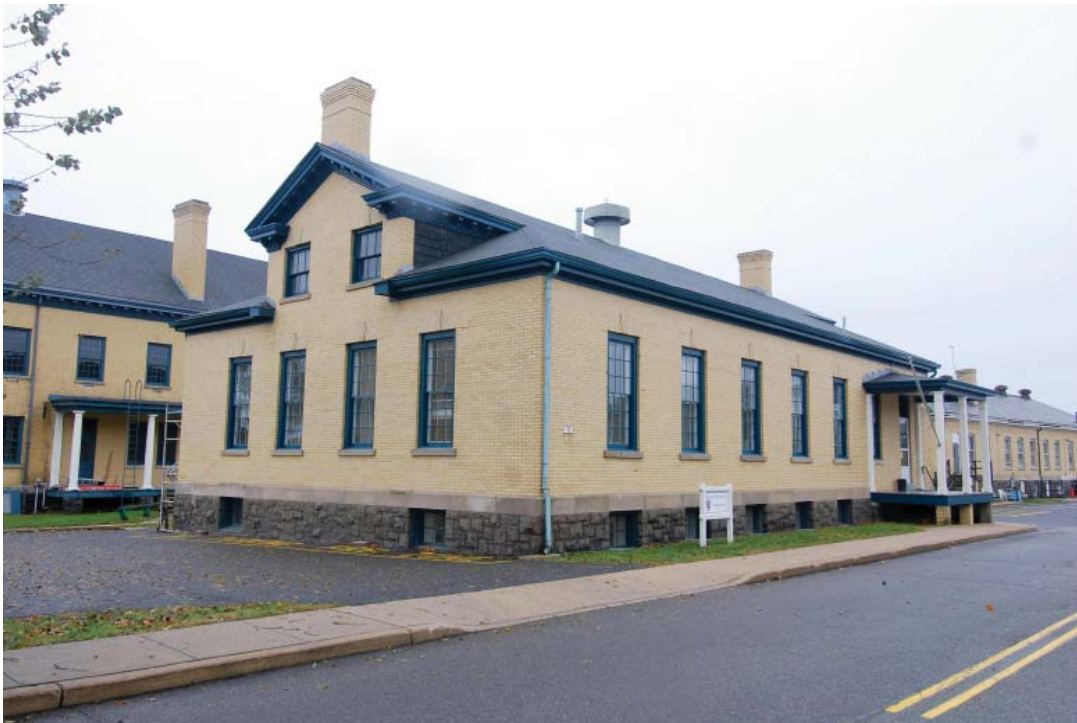
Photo 21. View of Building #58 looking northwest (JMA, October 2009)
