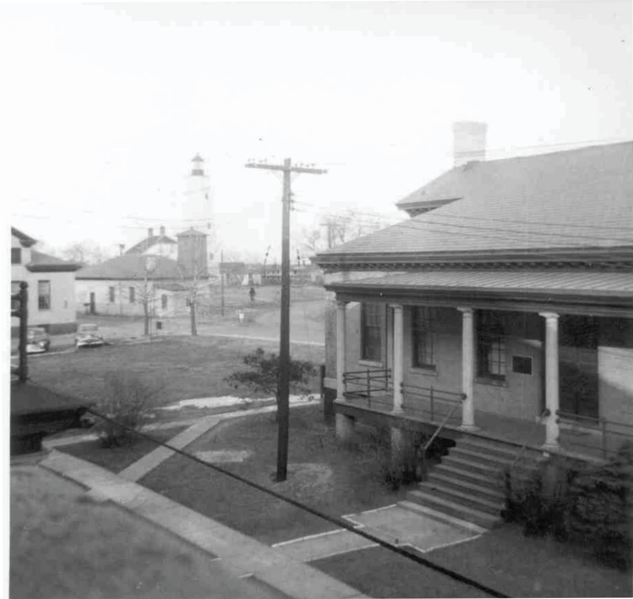
3. General view of mess halls toward northeast, c. 1956. Mess Hall #58 cut off on far left. Mess Hall #57 at far right. Photo #11209, Gateway National Recreation Area Archives.
