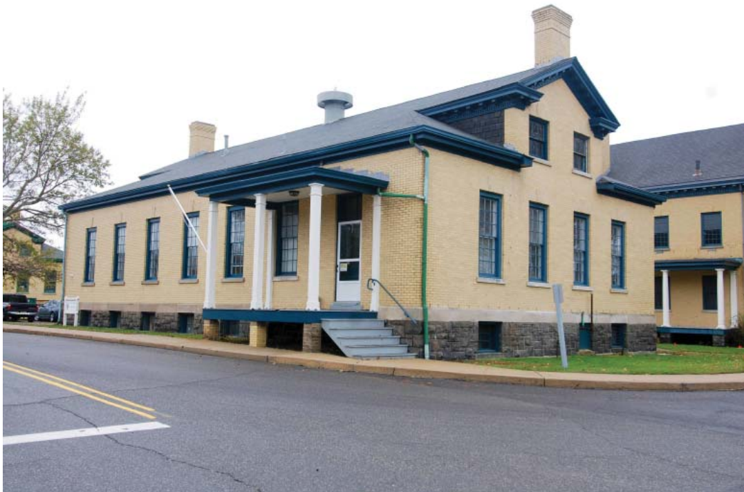
Photo 24. View of Building #58 looking southwest (JMA, October 2009)
