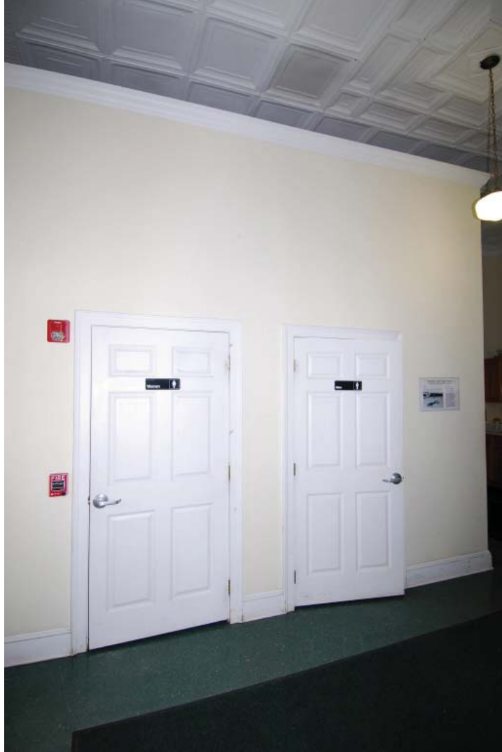
Photo 93. View of ADA compliant toilets located to southeast of historic kitchen area. The most recently built accessible toilet facilities have the required ADA compliant door hardware (JMA, October 2009).
