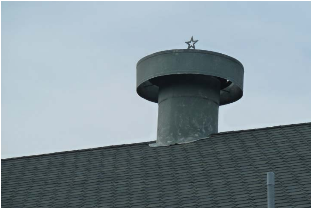
Photo 74. Detail of the central ridge ventilator. (JMA, April 2009)
