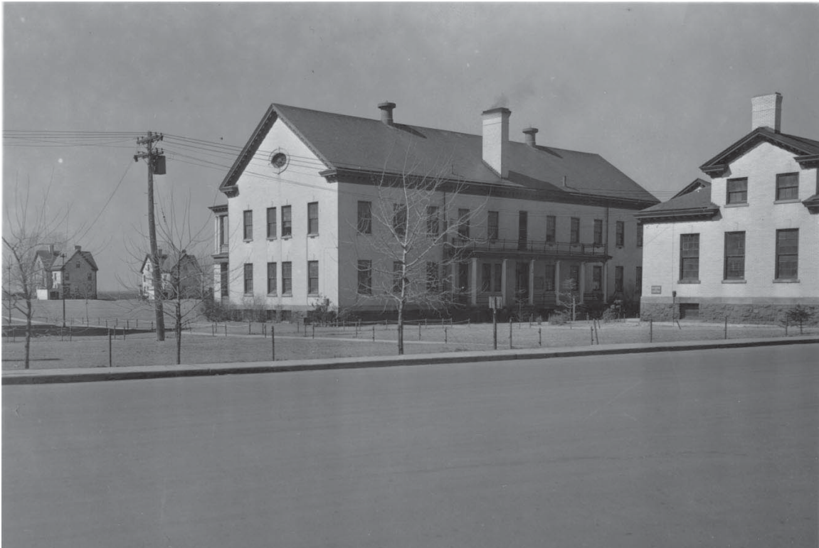
Photo 4. General view from south showing Enlisted Men's Barracks #24 at left and Mess Hall #57 at right (#30432, Gateway National Recreation Area Museum archives)
