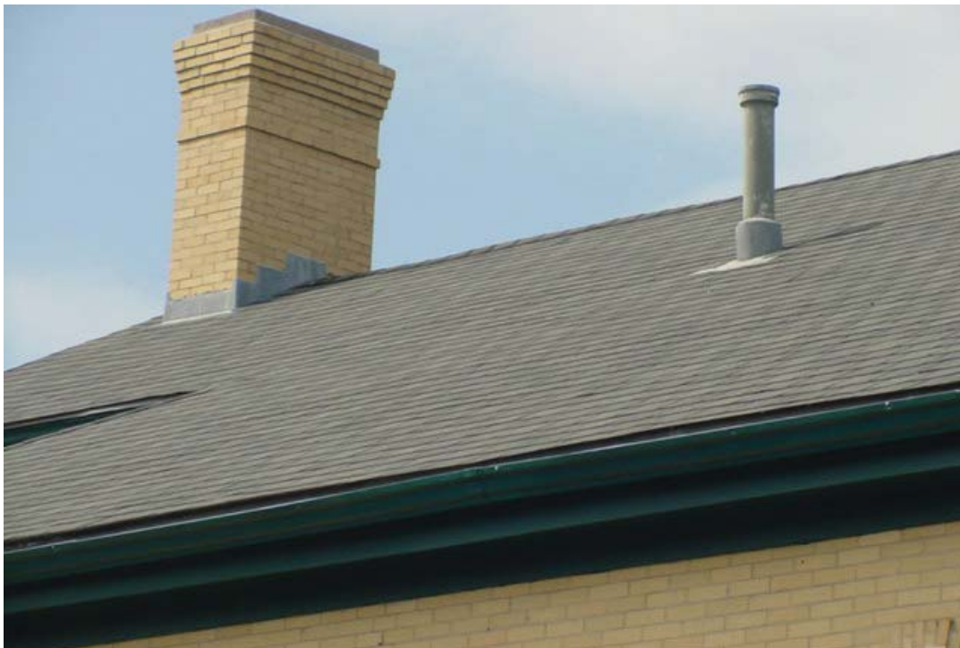
Photo 72. Detail of the roof at Building #58. Note the stepped flashing at the chimney and roof vent. (JMA, August 2010)
