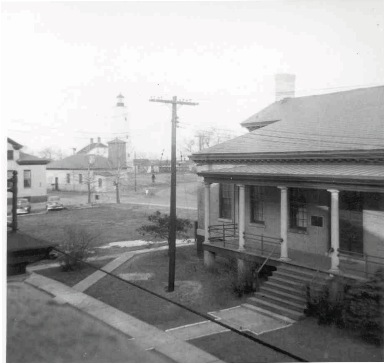
4. Undated photograph showing a portion of the main porch of Mess Hall Building 57. Photo #11209, Gateway National Recreation Area Archives.
