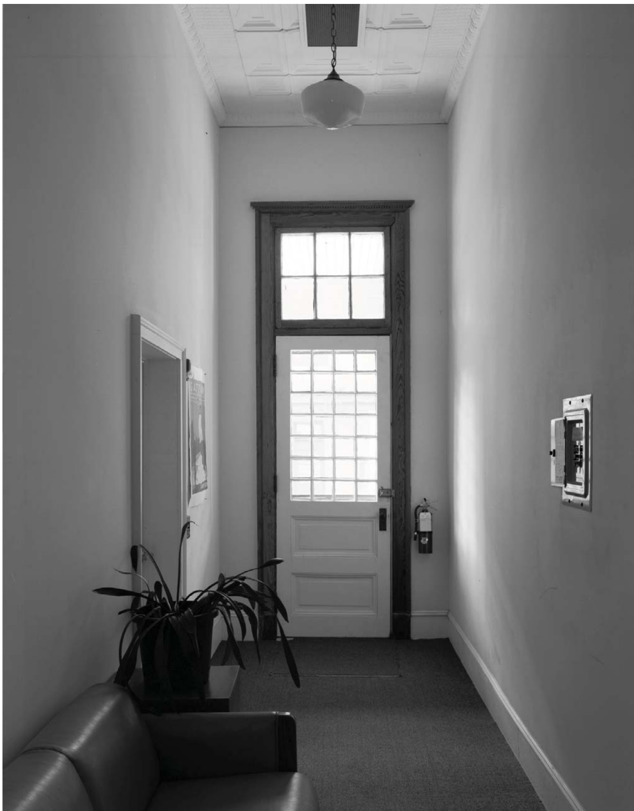
Photo B-24. Building #58, first floor interior of south hall looking west towards single door entry. Fort Hancock, Sandy Hook Unit, Gateway National Recreation Area. Sandy Hook, New Jersey. Photographer: Doug Harnsberger. September 2010.
