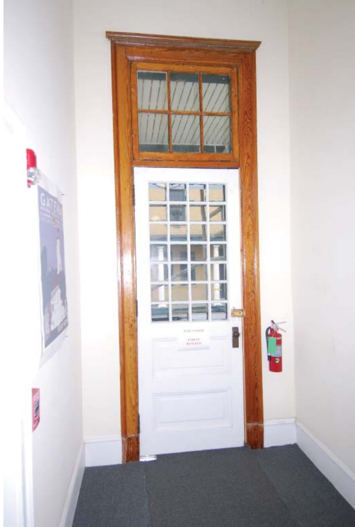
Photo 92. The single leaf entrance door from the west porch has ADA compliant width but retains original hardware (JMA, October 2009).
