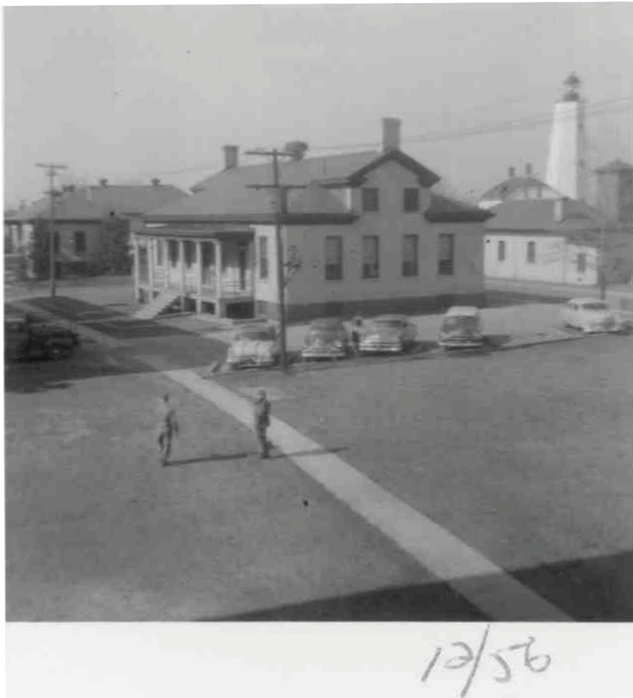
6. Photograph of south end and west side of Mess Hall Building #58 (December 1956). Photo #11212, Gateway National Recreation Area Archives.
