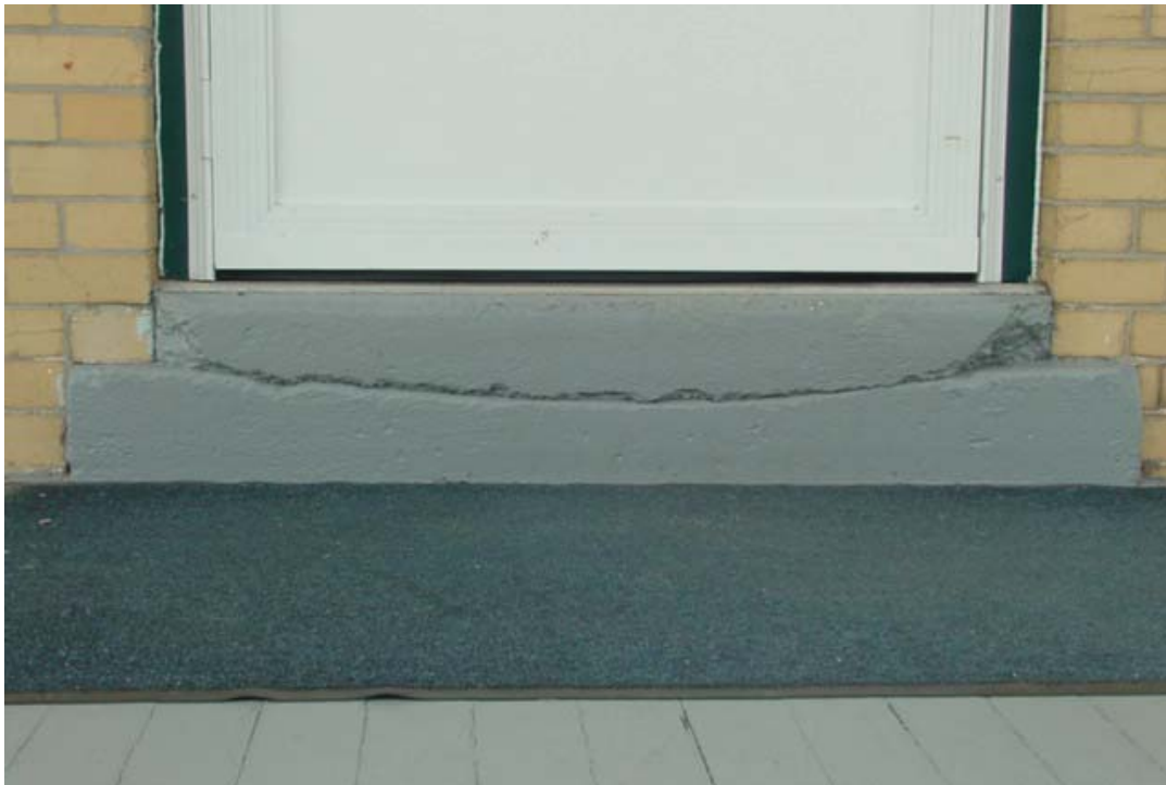
Photo 64. Detail of the east entrance door sill. Note the thick concrete topping, which extends across the kitchen and pantry floors. The concrete topping was placed on top of a well worn door sill. The gray paint is recent. (JMA, August 2010)
