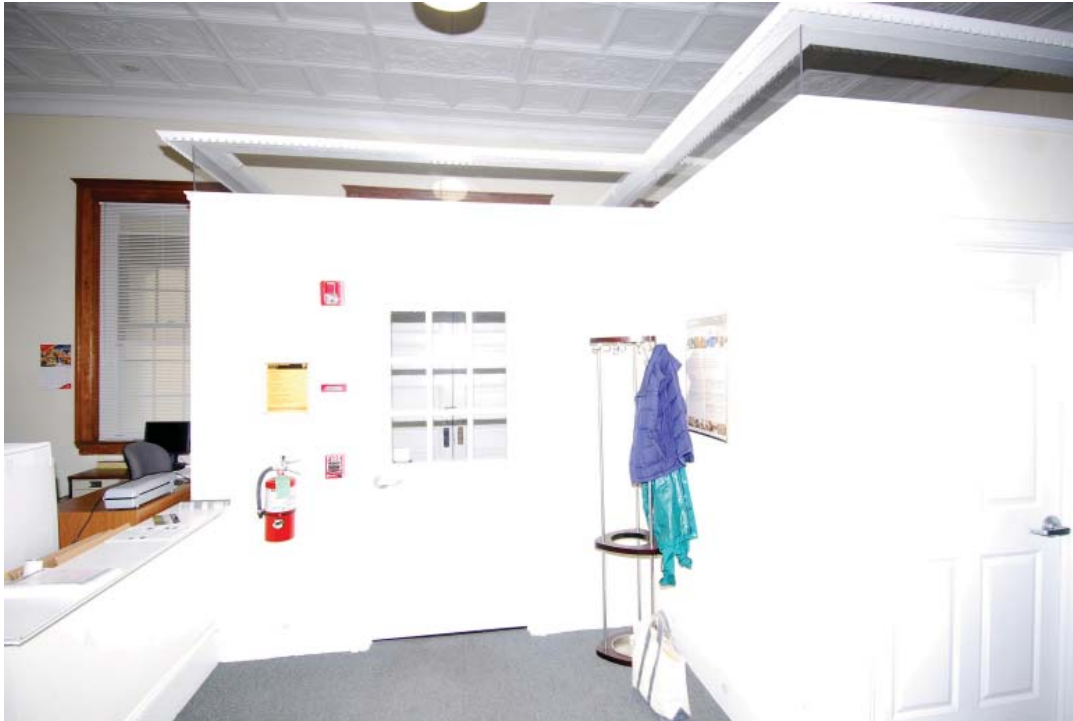
Photo 90. The single leaf door from the foyer (114-1) is appropriately sized and has ADA compliant hardware (JMA, October 2009).
