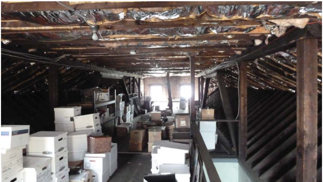
Photo 54. Attic overview looking south. Note opening for stair to first floor at lower right. (JMA, October 2009)
