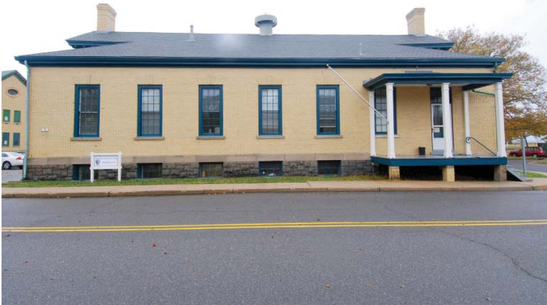
Photo 22. East elevation (JMA, October 2009)
