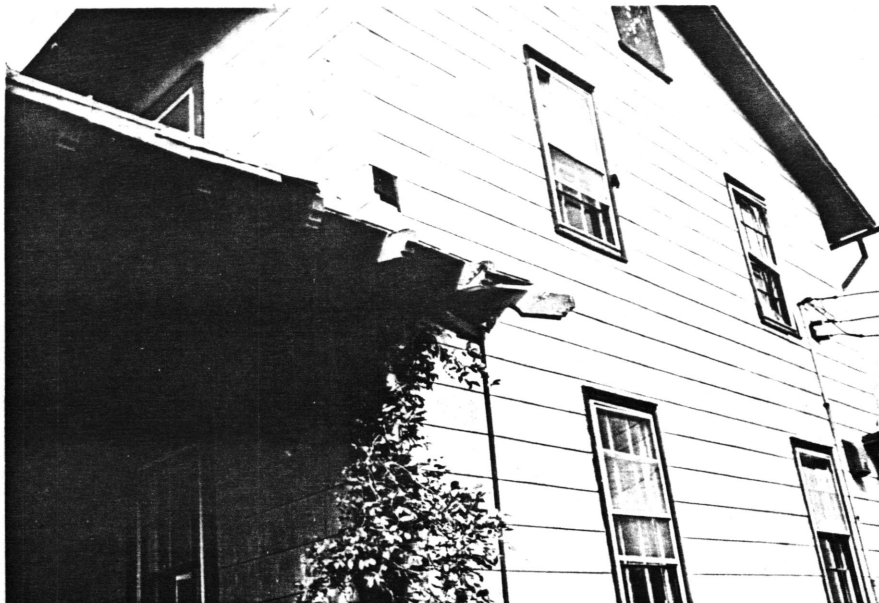
Building 75, Duplex N.C.O. Quarters, detail of front porch eave damage. Note also typical condition of aluminum storm sash, installed circa 1973. S-79
