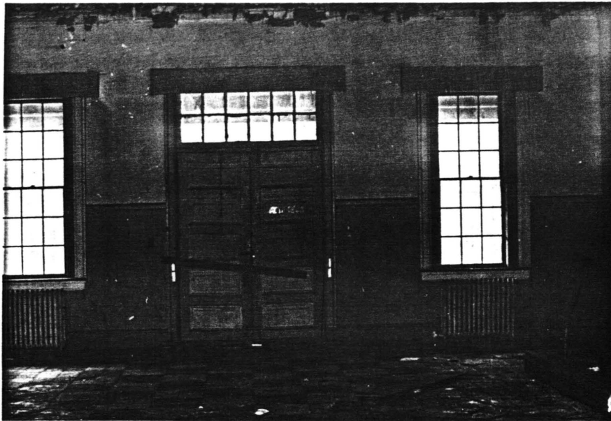
Building 58, Mess Hall, interior.
