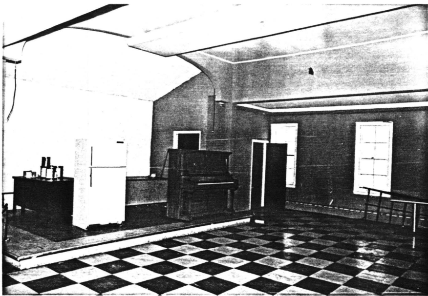
Building 123, St. Mary's Chapel, interior. Dropped panel on ceiling and room cornice conceal lighting. 4/79 FH4
