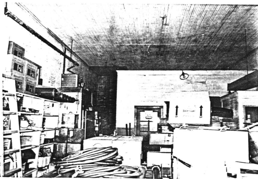
Interior, showing beaded ceiling and partition. Hose tower is above rear corner. 4/79 FH2
