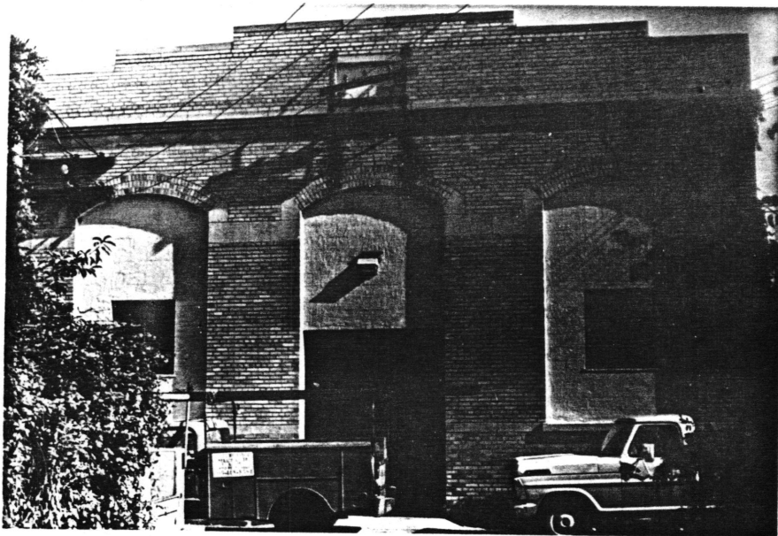
Building 341, Pump House, front. FH 9/78 B-17 17
