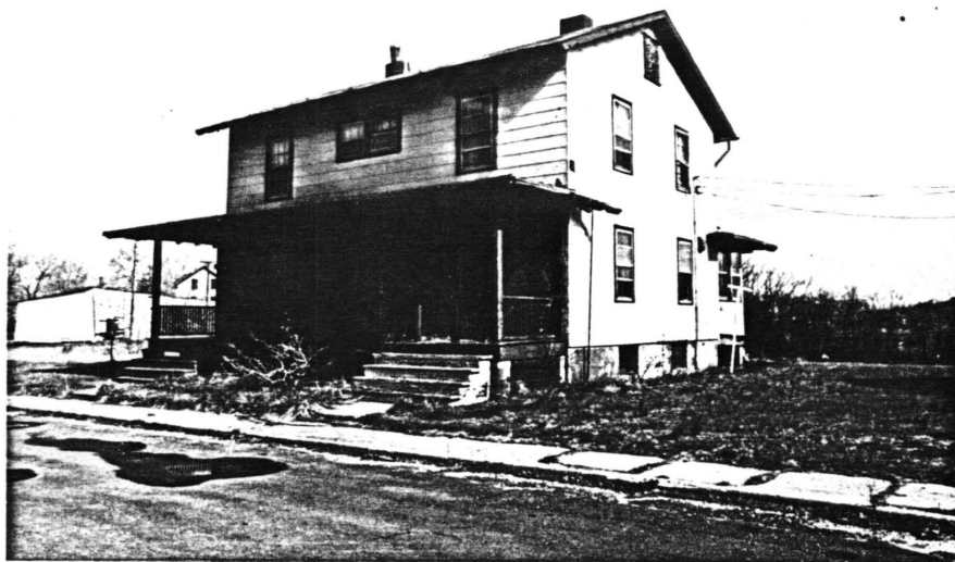
Building 75, Duplex N.C.O. Quarters, southwest view. Asbestos shingles hide earlier clapboard walls. Army logs describe the building as stucco, so this may be the third wall material. 4/79 FH2
