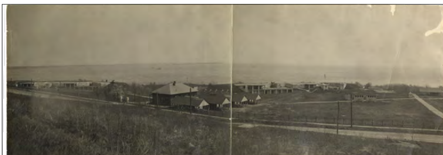
Figure 4.26. Historic photograph illustrating the extensive vegetation clearing south of the battery control structures and north of Battery Road. This historic view had a significant and specific function in the historic military landscape. The battery control structures supported the Endicott batteries to the south (Gateway National Recreation Area Collection, Photo 20618 (2
