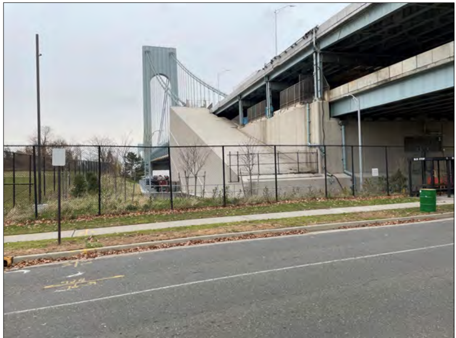
Figure 4.27. Photograph of the western anchor for the Verrazzano-Narrows Bridge, facing southwest (PaleoWest 2021).
