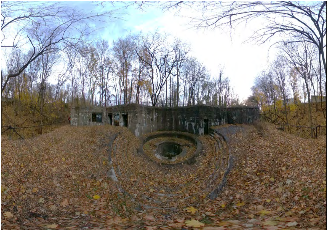
Figure 3.13. 360-degree photograph of the interior of Battery Dix. Note the existing chain link fencing (PaleoWest 2021).
