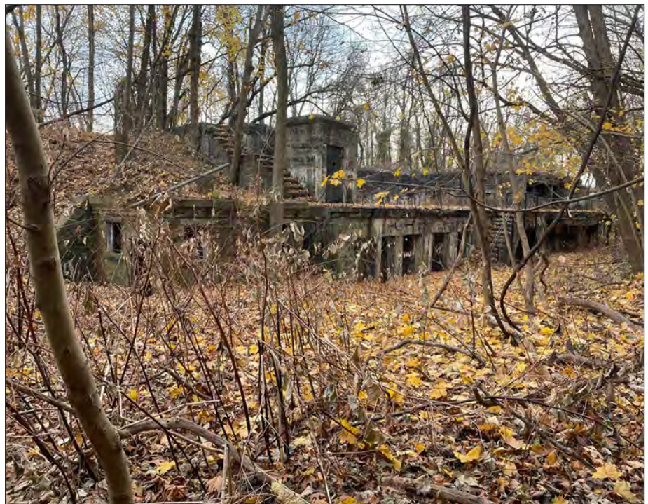
Figure 2.94. Figure 2 94. Photograph of Battery Dix, the least deteriorated of the Endicott Era batteries, December 2021 (PaleoWest).
