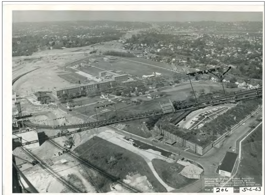
Figure 2.69. Aerial photograph depicting excavation for the bridge anchorage and clearing for the bridge approaches, May 1963 (Courtesy of MTA Bridges and Tunnels Special Archive, Photo NB-3-206).
