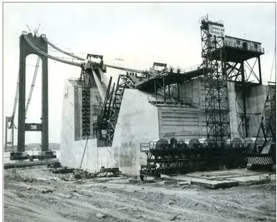
Figure 4.28. Historic photograph of the west anchor for the Verrazzano-Narrows Bridge, 1963, facing southeast (Metropolitan Transit Authority Bridges and Tunnels Archives, Photo NB_3_209).
