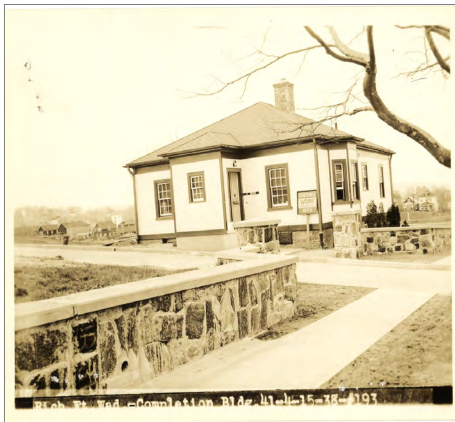
Figure 2.51. Photograph depicting an example of support buildings constructed or renovated by the Works Progress Administration, 1930s. Note the stone wall which is a similar type installed along the Battery Weed overlook, later National Park Service Terrace (Gateway National Recreation Area Collections, Image 20605).
