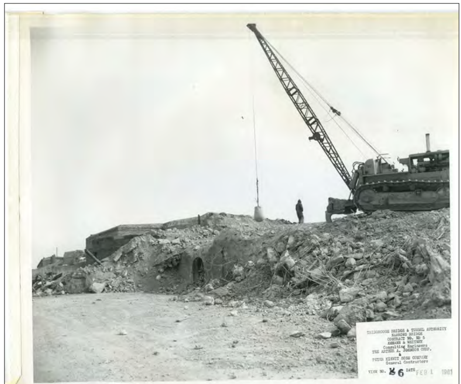
Figure 2.72. Photograph of the partial demolition of Battery Duane, February 1961 Courtesy of MTA Bridges and Tunnels Special Archive, Photo NB-5-26).
