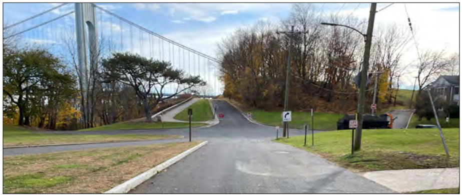
Figure 4.2. Photograph of Battery Weed Road, looking south (PaleoWest 2021).
