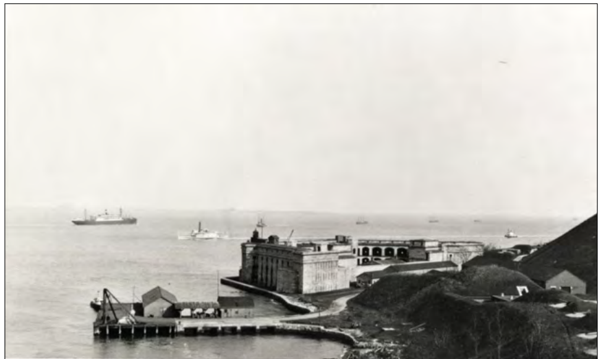
Figure 4.14. Historic photograph of Battery Weed and the North Dock, facing southeast, circa 1915 (Gateway National Recreation Area Collections, Photo 19431).
