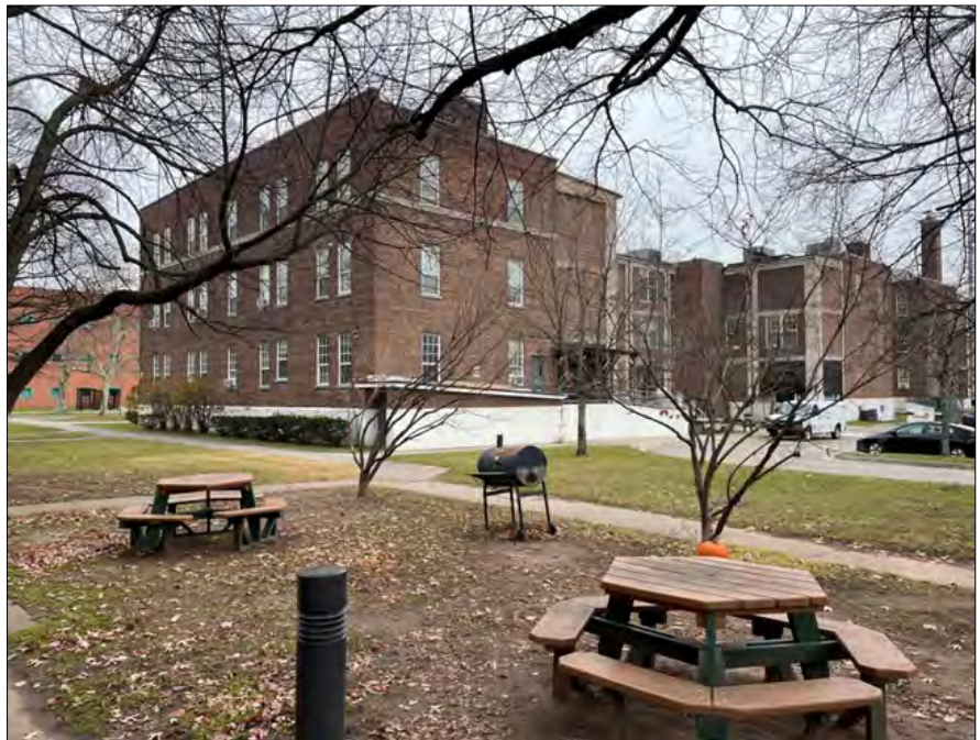
Figure 4.24. Photograph of rear of Building 210, facing southeast (PaleoWest 2021).
