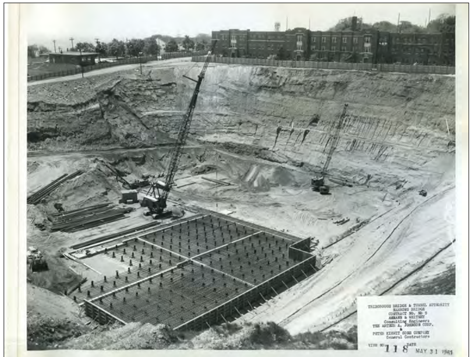
Figure 2.70. Photograph of excavations for the bridge anchorage, May 1961. Note the remaining 1931 Infantry Barracks are visible in the background (Courtesy of MTA Bridges and Tunnels Special Archive, Photo NB-5-118).
