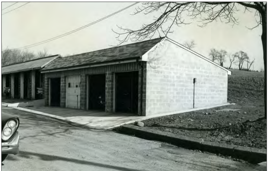
Figure 4.21. . Historic photograph of garages for Officer Residences, New Building No. 116, photographed January 5, 1961 (Metropolitan Transit Authority Bridges and Tunnels Archives).
