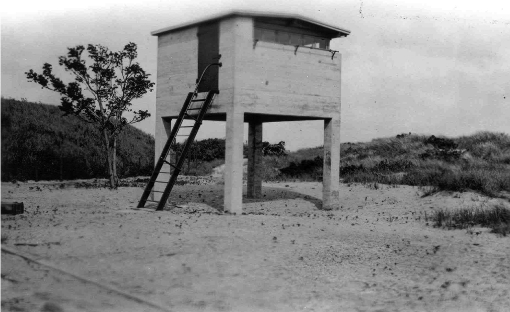
Figure 12. View looking northwest at coincidence range finding station east of Battery Morris, circa 1921. (GATE 7893)
