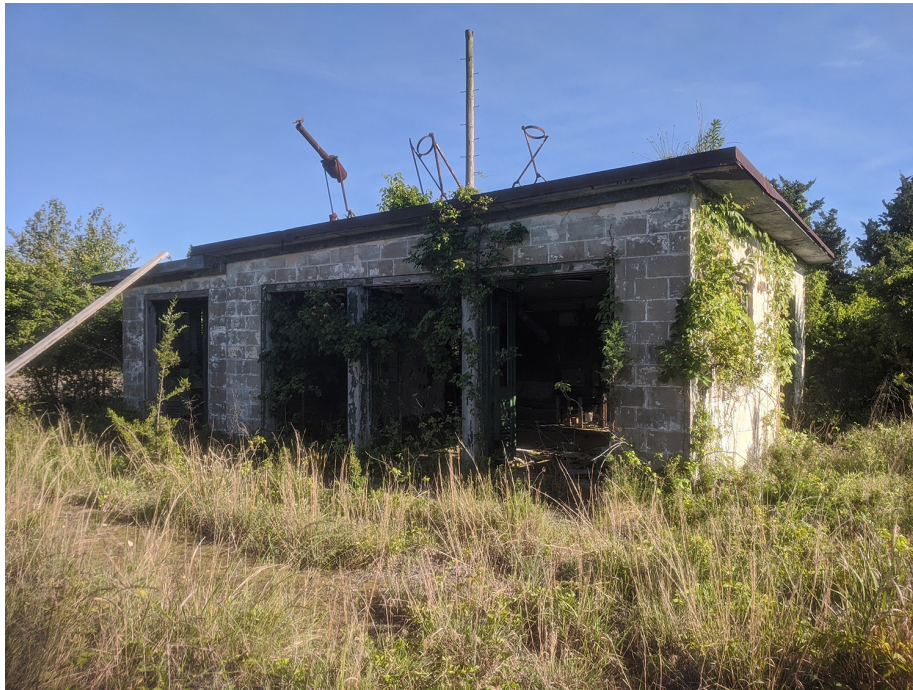
Figure 21. View looking southeast at the Generator Building (414), Control Area #2, at the NIKE Radar Site. (OCLP 2020, IMG-173852)
