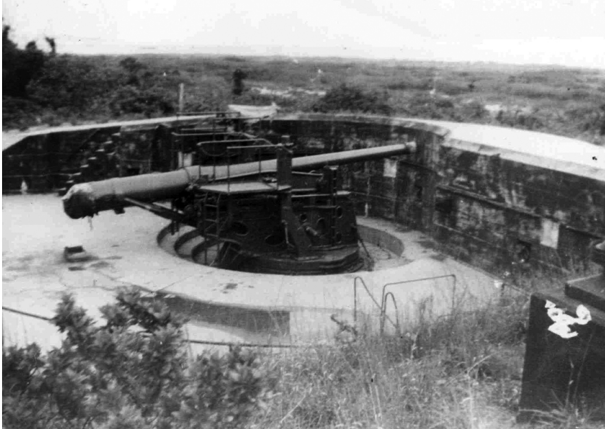
Figure 9. View looking northeast at Battery Gunnison's emplacement #2, circa 1936-1939. The Army replaced the pictured counterweight carriage guns with barbette-mounted guns in 1943. (GATE 7834)
