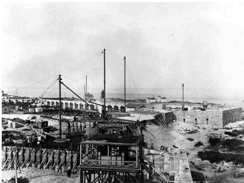
Figure 4. View looking northwest at construction of Nine Gun Battery over the east oceanside wall of the Civil War-era granite fort, 1897. (GATE 7880)
