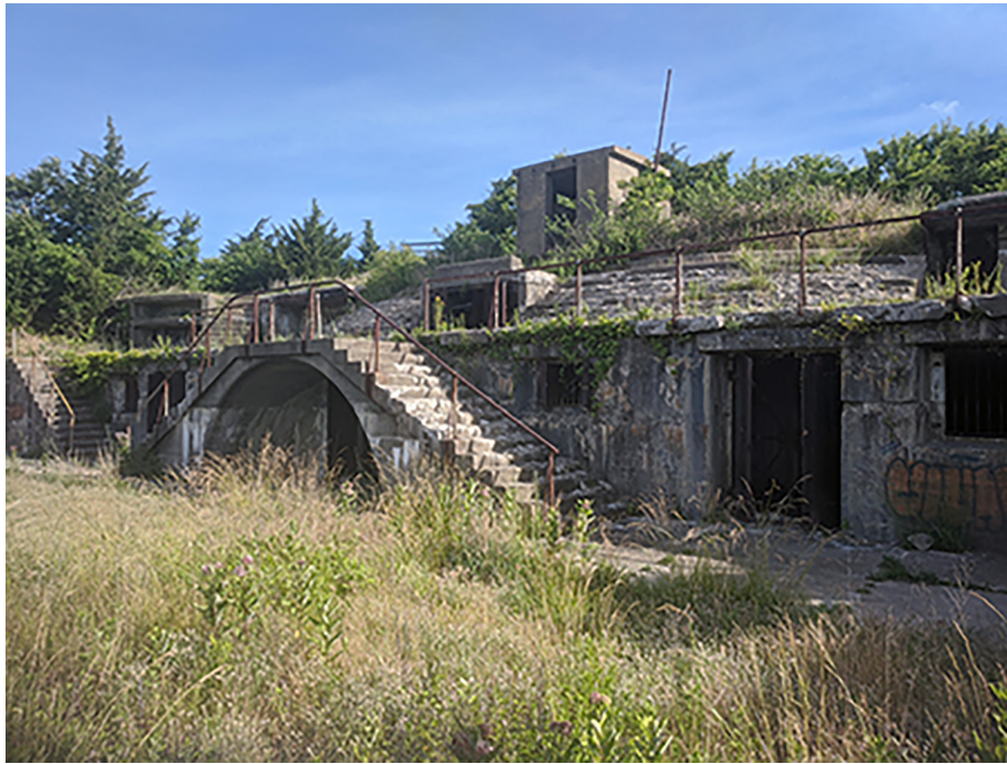
Figure 15. View looking northwest at the rear elevation of Battery Peck. (OCLP 2020, IMG-082853)
