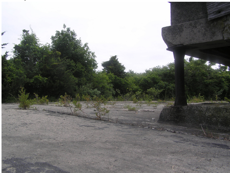
Figure 23. Blocked view looking east from the battery commander's station at Battery Granger. (OCLP 2020, P1010015)
