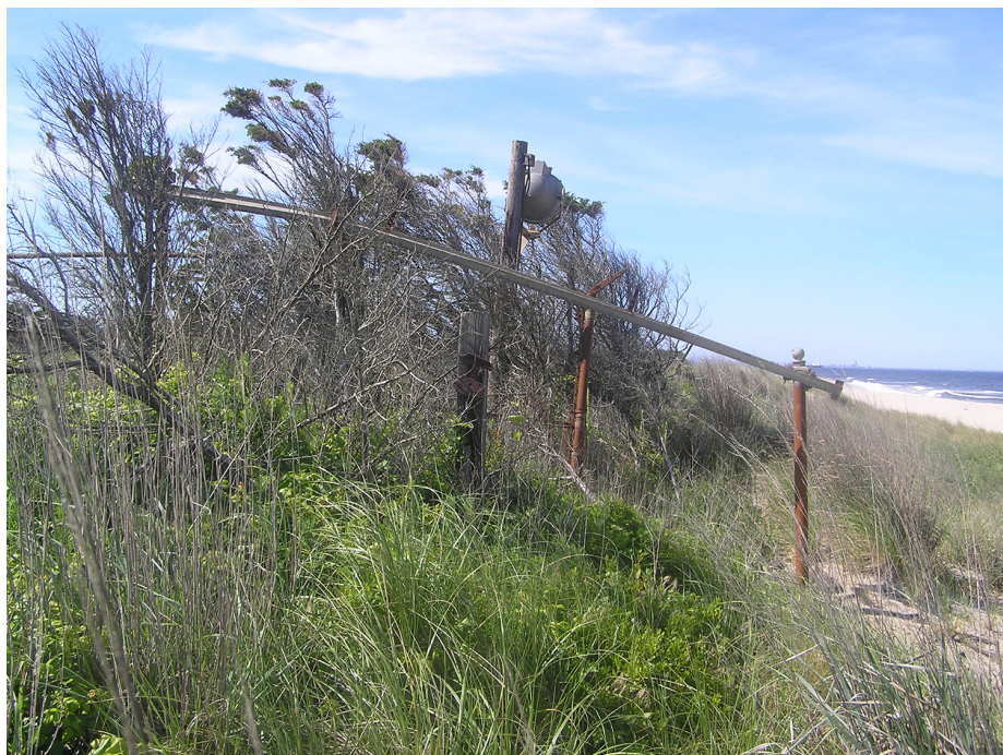
Figure 16. View looking north at fencing and a floodlight at the southeast corner of the NIKE Launch Site. Severe erosion of the engineered slope on the east, ocean beach side of the site has impacted both features. (OCLP 2020, P1010018)
