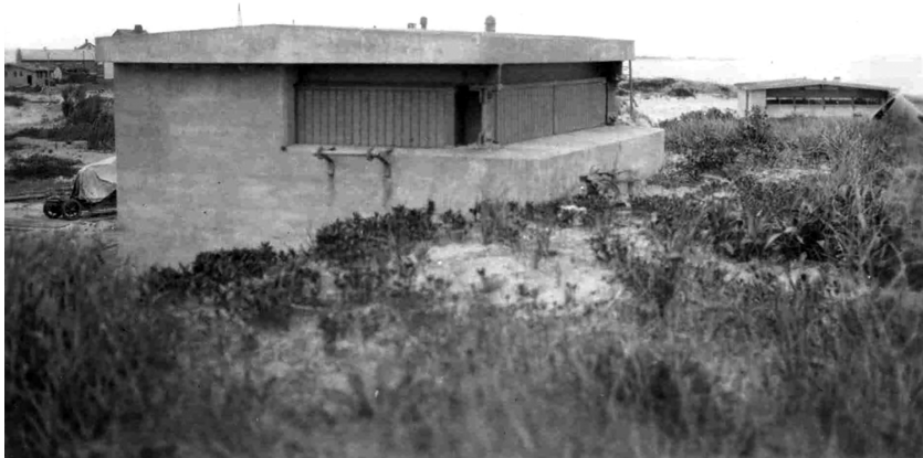
Figure 11. Covered battery commander's station at Battery Peck, foreground, and coincidence range finding station built over former Battery Engle's gun emplacement, right background, 1921. (GATE 7892)
