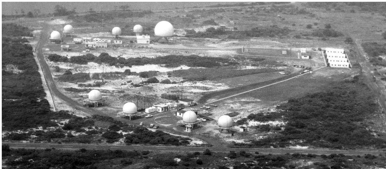
Figure 13. Oblique aerial view, NIKE radar site, circa 1965. Control Area #2 appears in the foreground with Control Area #1 in the background and the Ready Barracks to the right. (GATE 20818)
