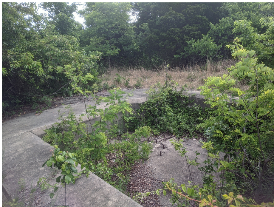
Figure 22. View looking north at the current view from Emplacement 4, Battery Urmston. (OCLP 2020, IMG-095656)
