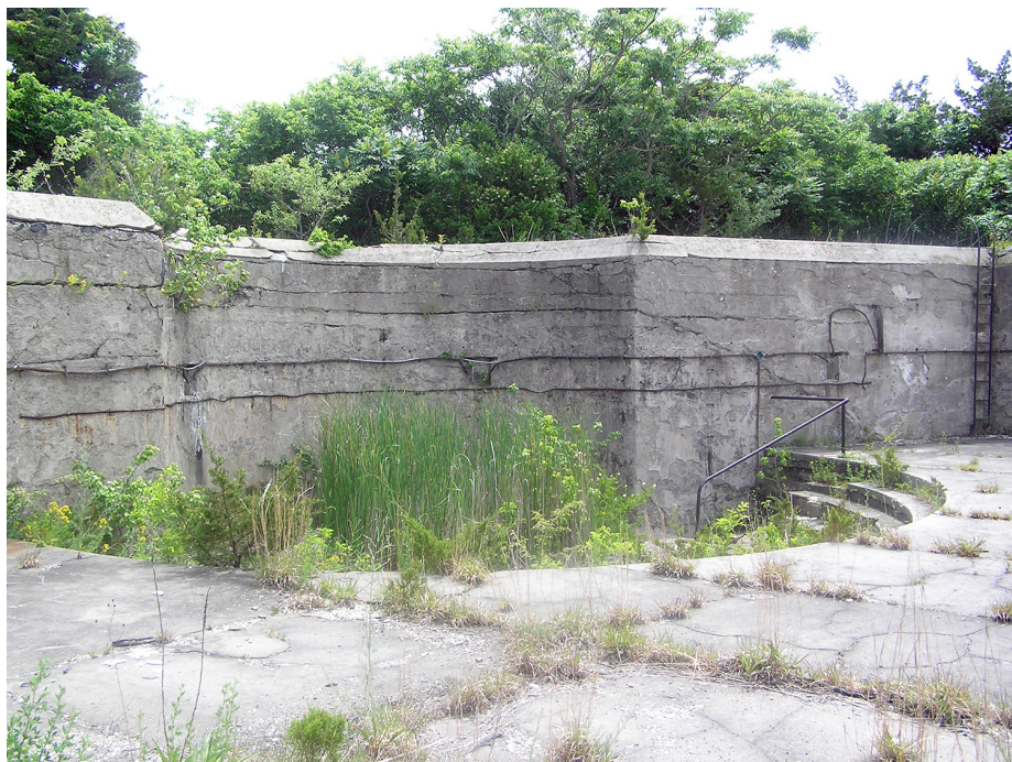
Figure 17. View looking east at vegetation growing in the gun pit and atop the parapet wall of Emplacement No. 1, at Battery Granger. (OCLP 2020, P1010011)
