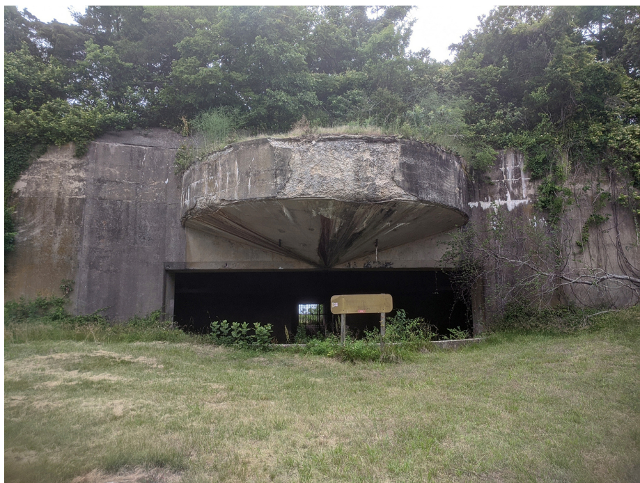
Figure 19. View looking west at Emplacement No. 1 at Battery Mills. (OCLP 2020, IMG-153044)
