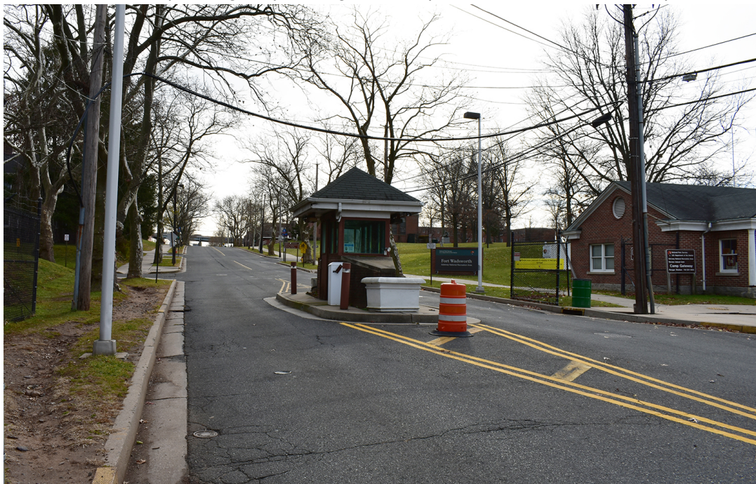
Figure 46. View looking south at the gate hut (Building 201) on New York Avenue, at the north boundary of Fort Wadsworth. The Gatehouse/Ranger Station (Building 220) is at image right. (PaleoWest 2021, DES-1779)
