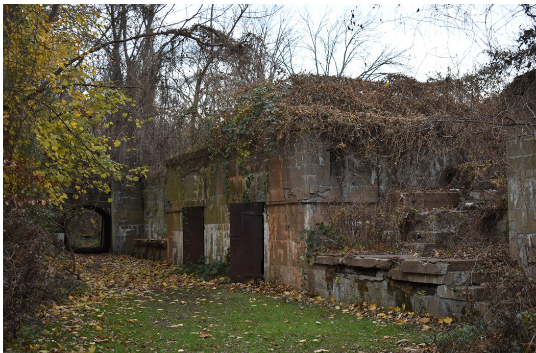
Figure 31. View of Battery Catlin. (PaleoWest 2021, DES-1886)
