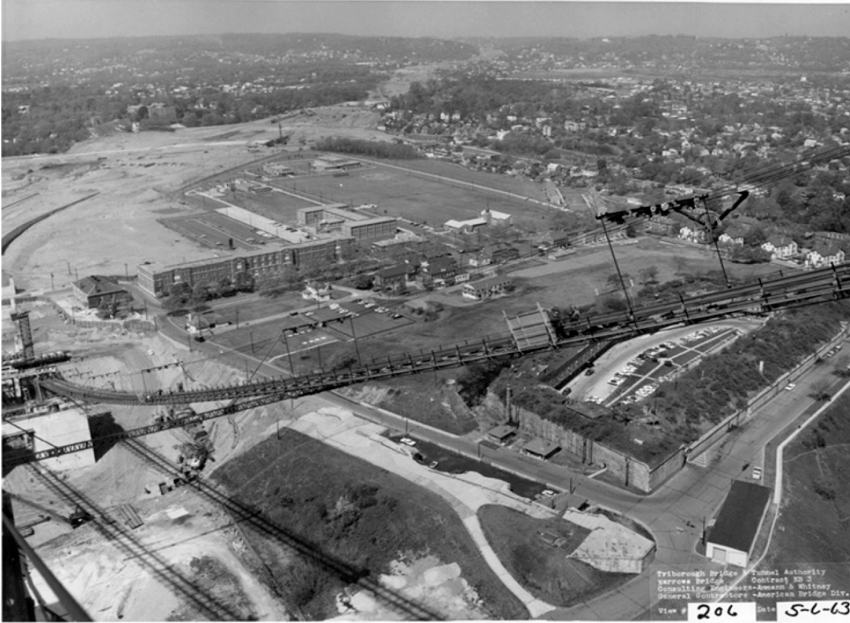
Figure 14. Aerial photograph depicting excavation for the bridge anchorage and clearing for the Verrazzano-Narrows Bridge approaches, May 1963. (Courtesy of MTA Bridges and Tunnels Special Archive, Photo NB-3-206, from CLR 2022: 108)
