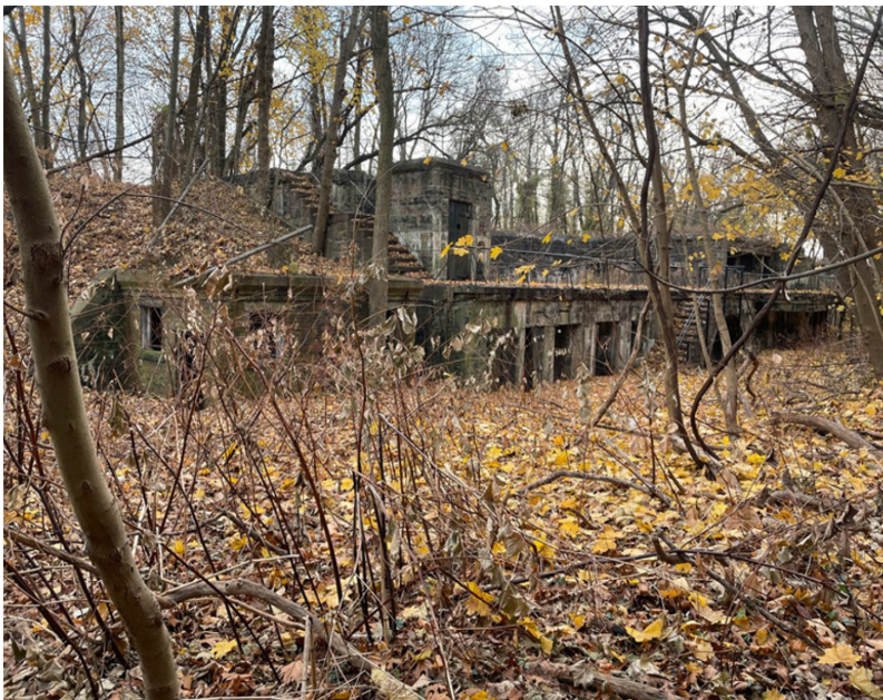
Figure 20. Photograph of Battery Dix, the least deteriorated of the Endicott Era batteries, December 2021. (PaleoWest, from CLR 2022: 150)
