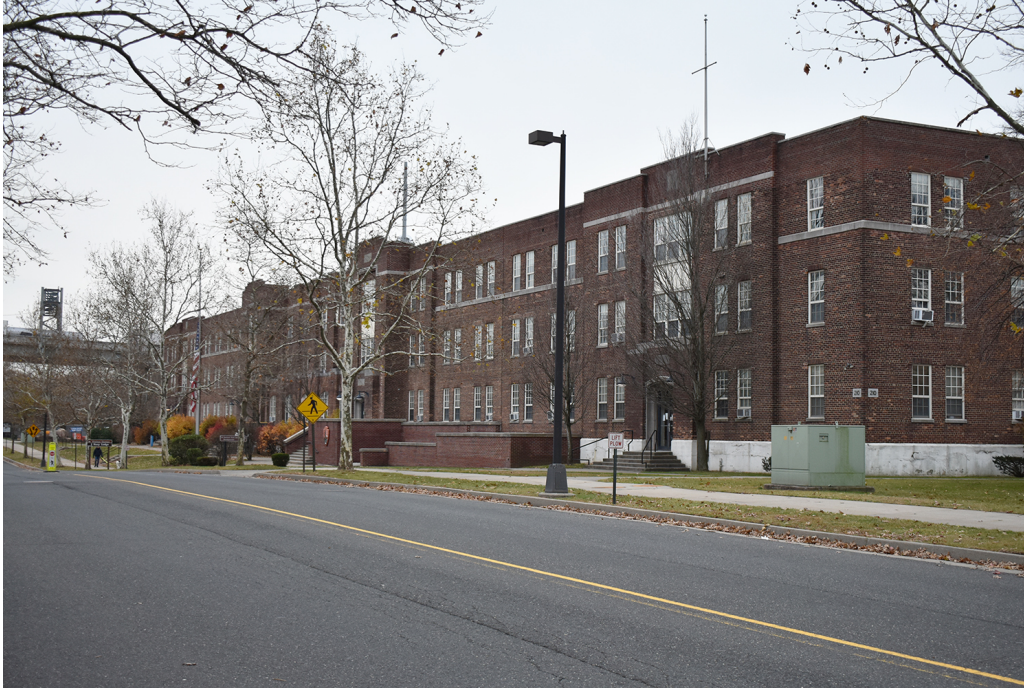
Figure 47. View looking south east at the former enlisted barracks (Building 210), now the headquarters of Gateway NRA. (PaleoWest 2021, DES-1914)
