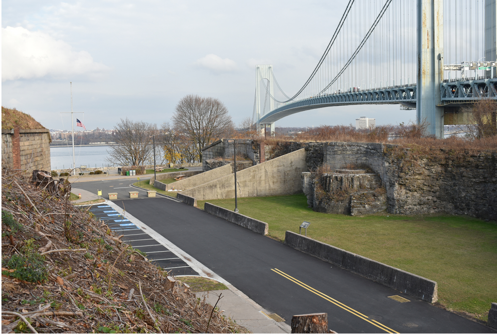
Figure 25. View looking southeast at recently cleared vegetation on the south side of Fort Tompkins and grass clearings at Battery Duane. (PaleoWest 2021, DES-1990)
