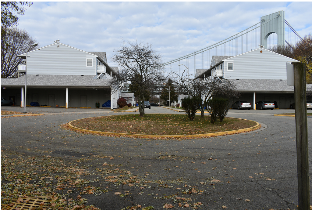
Figure 29. View looking northeast at USS New Mexico Court that accesses Junior Officers' Housing (Buildings 456 and 457). (PaleoWest 2021, DES-2262)
