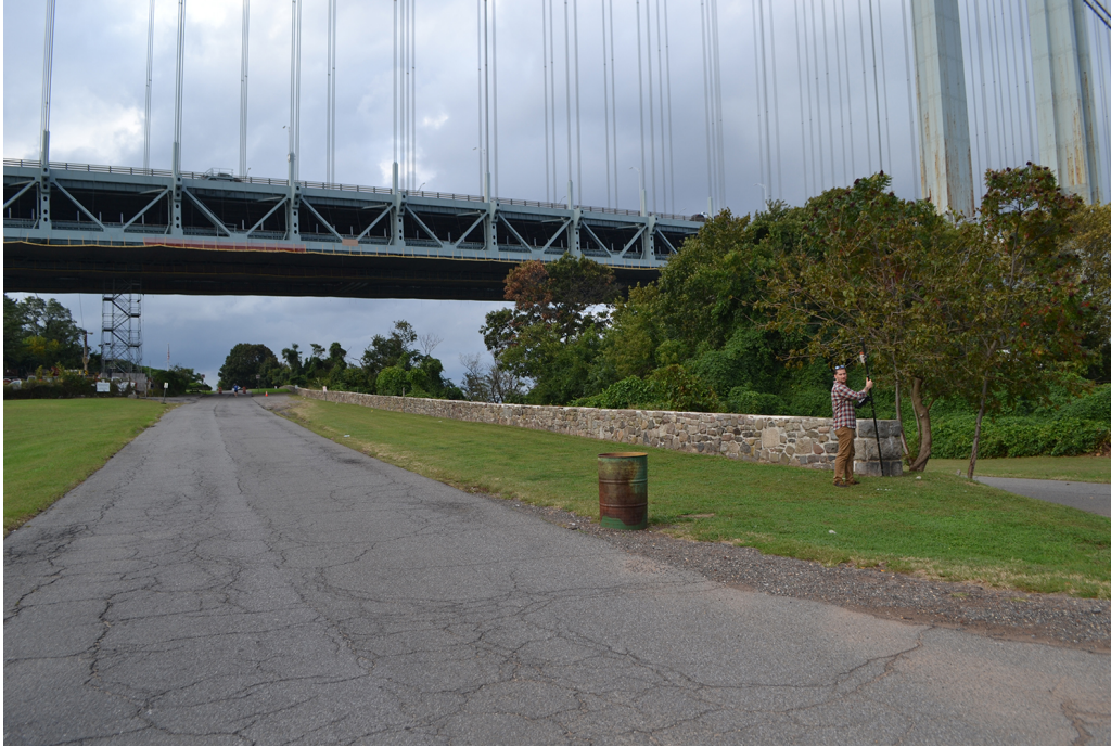
Figure 41. View looking north at the south end of the stone wall along Hudson Avenue. (OCLP 2021, DSC-0983)
