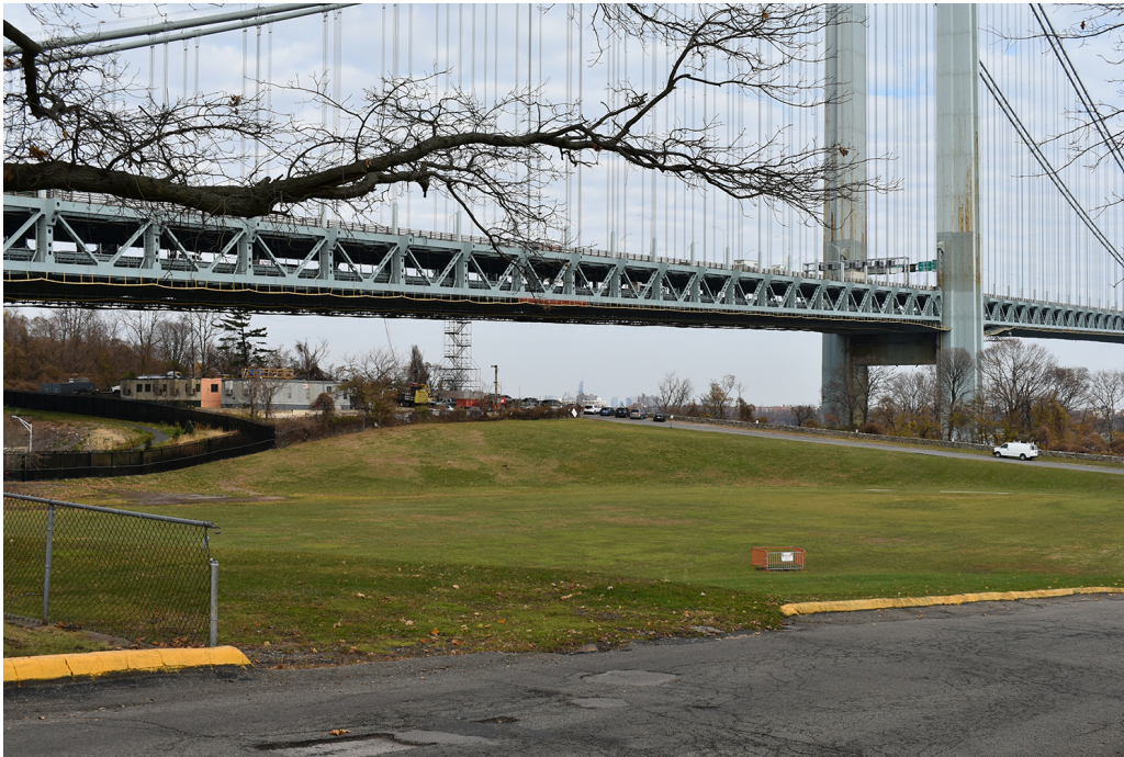
Figure 49. View looking northeast at the former track and athletic field space. (PaleoWest 2021, DES-2250)
