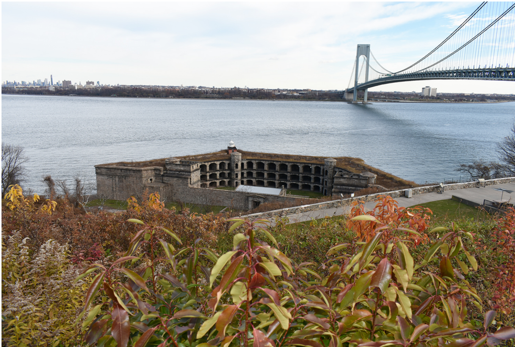
Figure 48. View looking east from the top of Fort Tompkins toward Battery Weed and the Narrows. (PaleoWest 2021, DES-1772)
