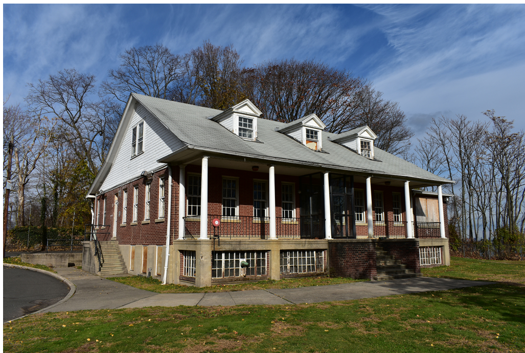
Figure 35. View looking north at the Administration/Officer's Club (Building 109). (PaleoWest 2021, DES-1797)
