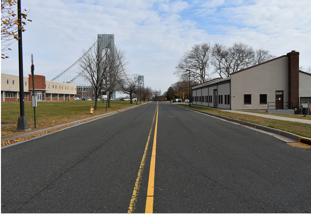
Figure 30. View looking east from Battery Road. An Army Reserve building is visible on the left. The building on the right is one of the motor pool buildings (Building 201). (PaleoWest 2021, DES-2228)
