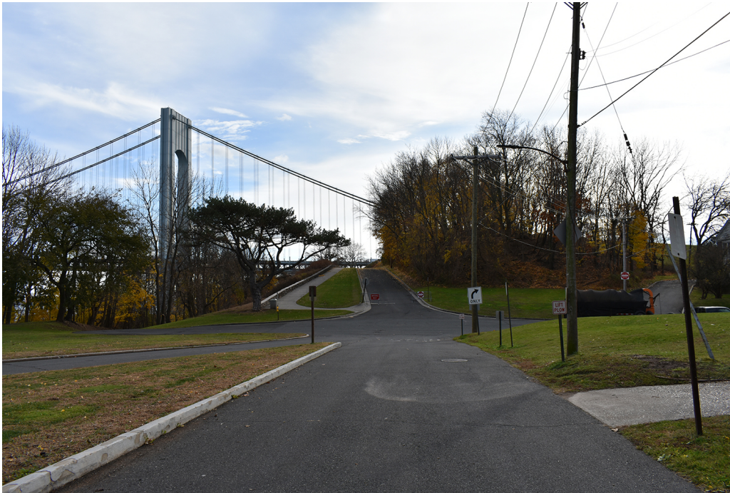
Figure 28. View looking south at the north end of Hudson Road, at intersection with the north end of Battery Weed Road (background left) and Mont Sec Avenue (background right). (PaleoWest 2021, DES-1794)
