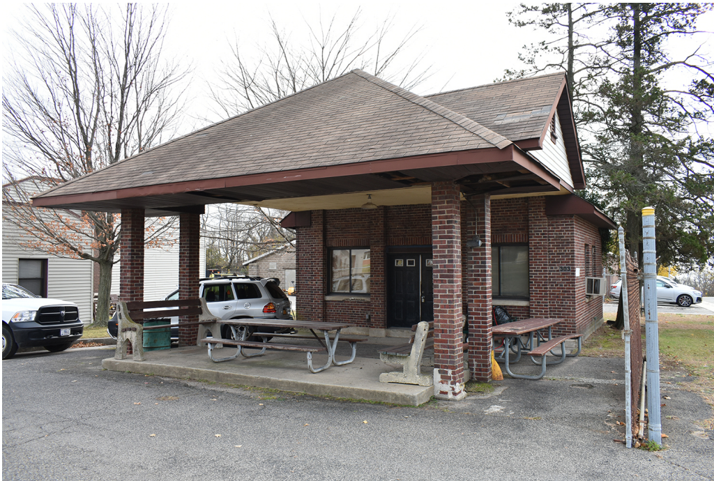
Figure 44. View looking south at the Motor Pool Office (Building 303/304). (PaleoWest 2021, DES-2211)
