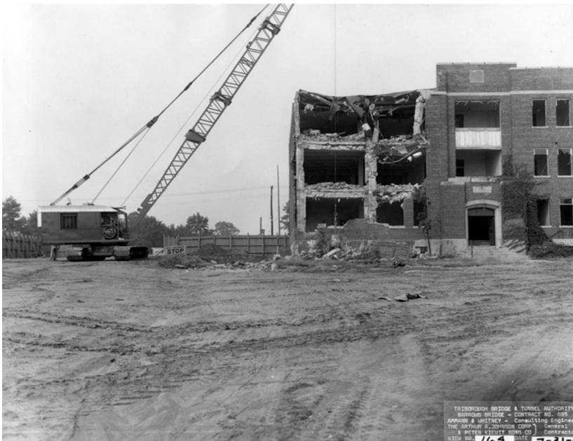
Figure 13. Photograph of the demolition of the 1931 Infantry Barracks at the southern end of Building 210, June 1961. (Courtesy of MTA Bridges and Tunnels Special Archive, Photo NB-5-164, from CLR 2022: 109)
