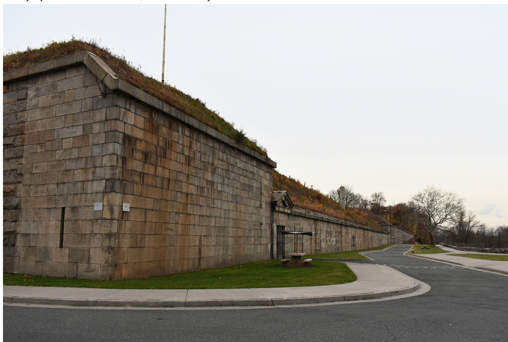
Figure 40. View looking west at Fort Tompkins. (PaleoWest 2021, DES-1983)
