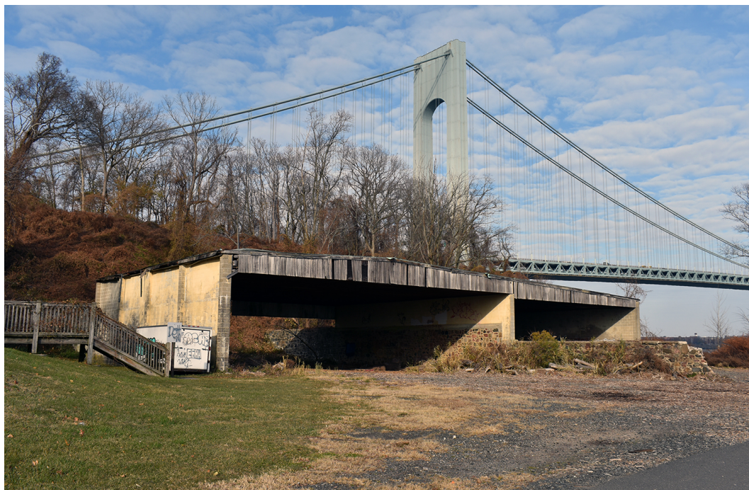
Figure 39. View looking northeast at the former Seaplane Hangar, then the Rifle and Pistol Range (Building 339). (PaleoWest 2021, DES-2268)
