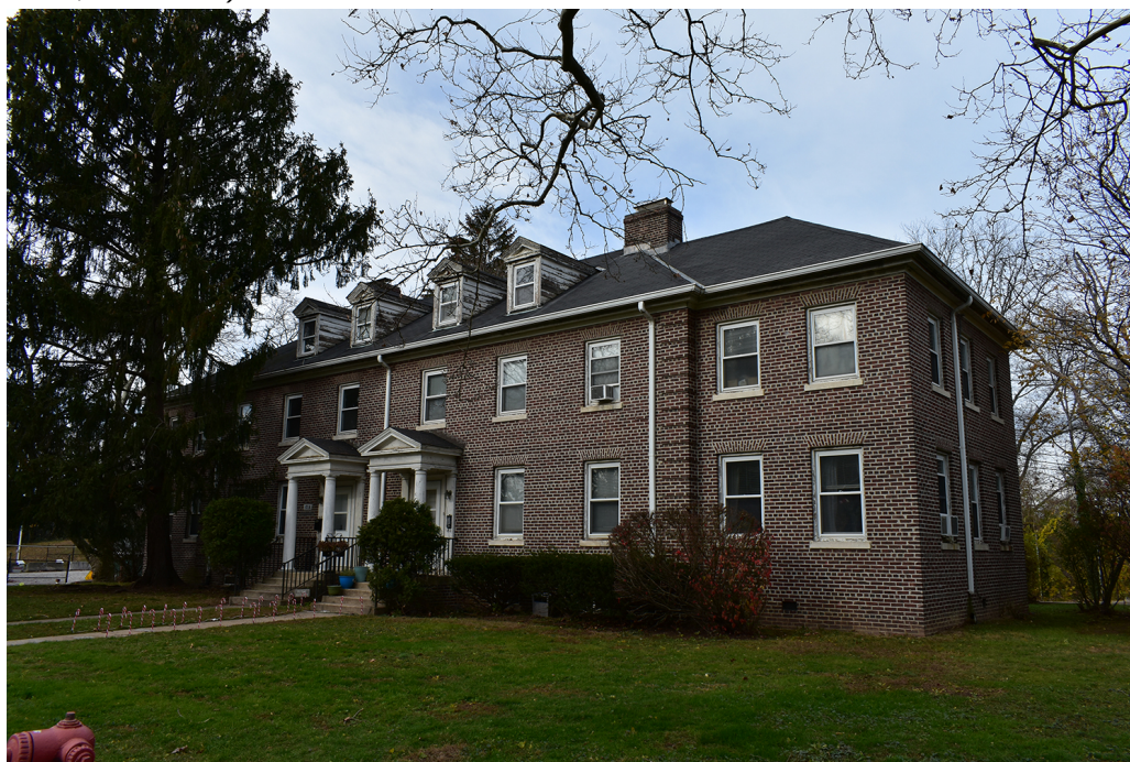
Figure 34. View looking at housing (Building 101) on Mont Sec Avenue. (PaleoWest 2021, DES-1782)
