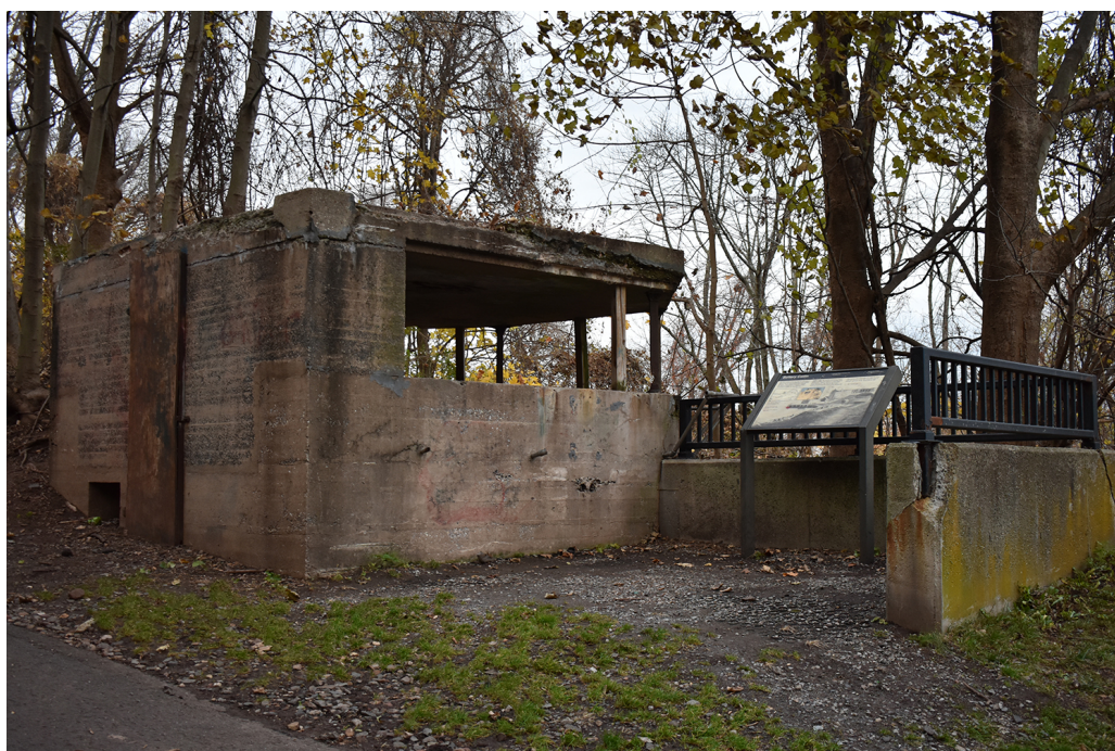
Figure 32. View looking north at the CRF station at Battery Catlin. (PaleoWest 2021, DES-2010)
