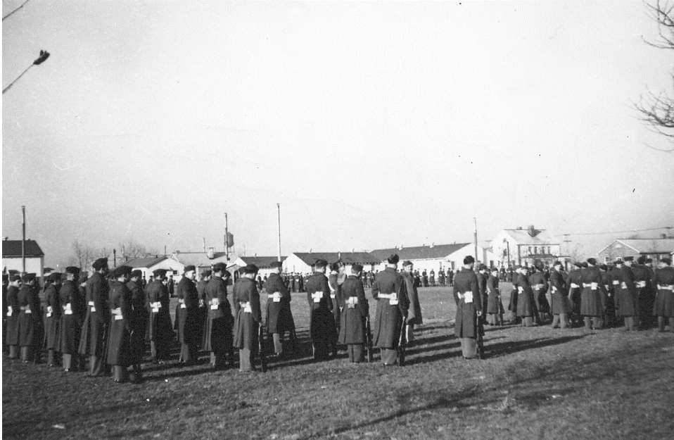
Figure 9. Soldiers drill on parade ground, view northwest, 1941. Buildings left to right: recreation hall (T-158), tailor shop (T-44), guest house (T-160), post restaurant (T-161), double NCO quarters, dispensary 10 (60 AB). (GATE Museum Collection 13105)
