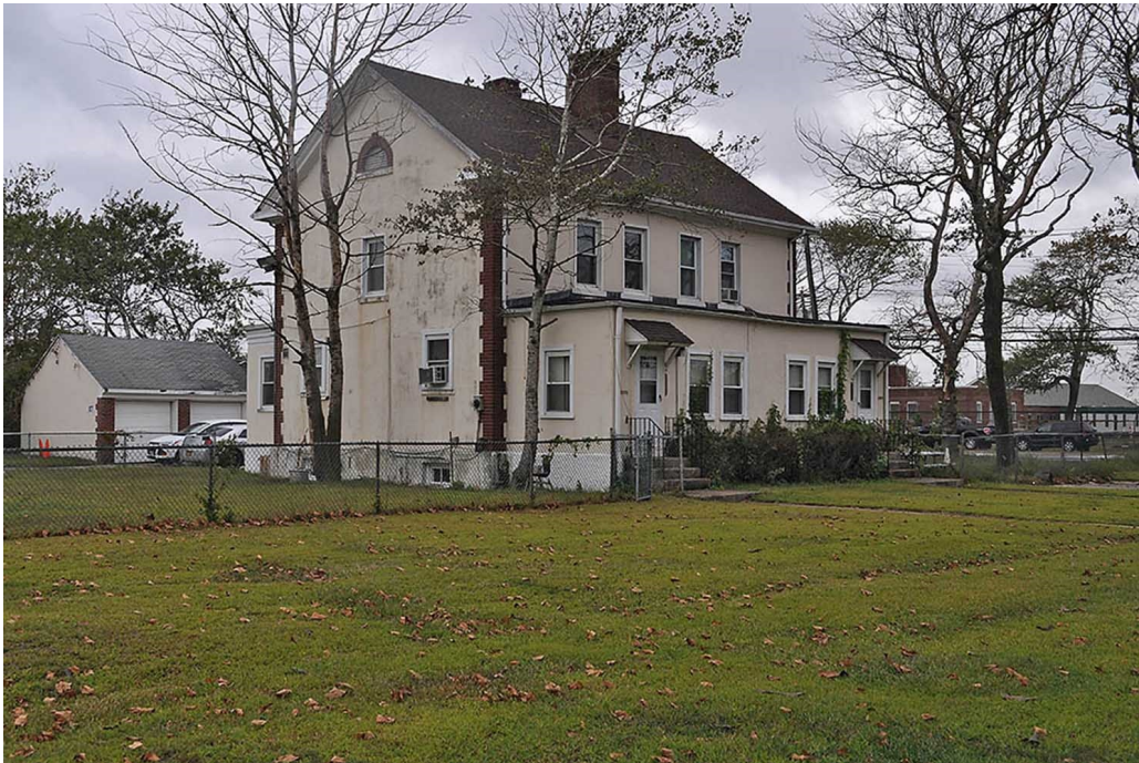
Figure 29. View northwest of officer quarters built in 1919 (former Double NCO, Bldg 106), 2014. Front porch was originally open; vinyl windows are recent addition. This is only remaining World War I-era building in post. (Olmsted Center)
