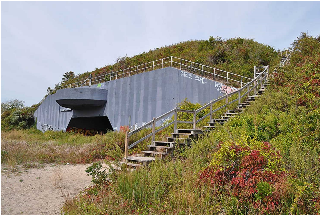
Figure 21. Wood stairway leading to Battery Harris Observation Platform, looking northeast from Range Road, 2014. (Olmsted Center)
