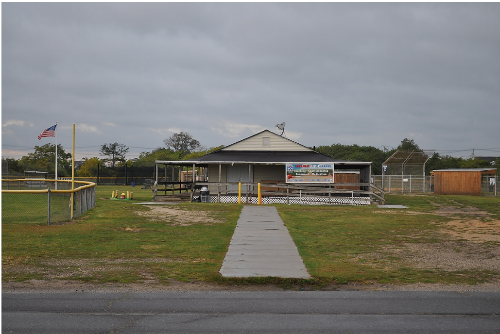
Figure 27. The Rockaway Little League clubhouse (T-162), the only remaining Series 700 building from the World War II-era barracks complex west of the parade ground, looking north, 2014. (Olmsted Center)
