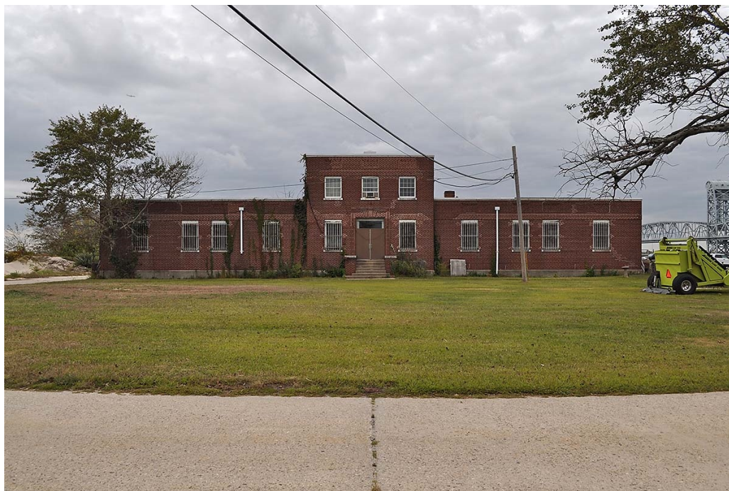
Figure 30. The WPA-built ordnance-administration building (Building 219, now storage) completed in 1937, looking north across Dunn Circle and lawn showing remnant ornamental plantings, 2014. (Olmsted Center)
