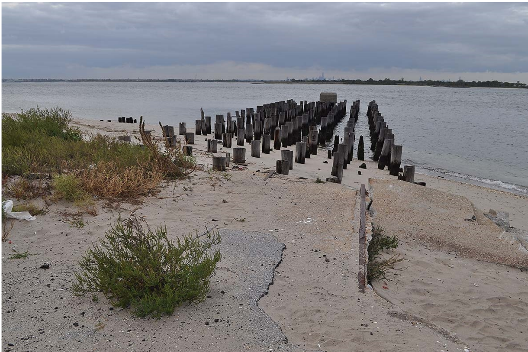
Figure 19. Remnant pilings from the Fort Tilden wharf (Building 209), looking northwest from Riis Landing parking area, 2014. (Olmsted Center)
