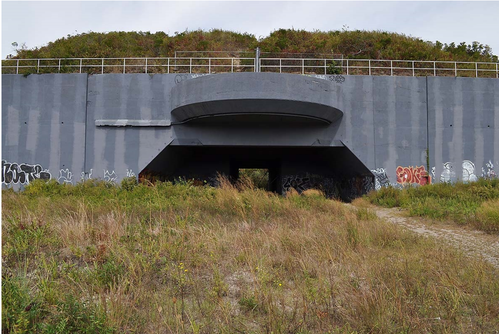
Figure 26. Battery Harris East Casemate (B-406), view north from Range Road showing protruding circular concrete hood and interior steel grill gates, 2014. The gun was removed in circa 1949 during the historic period. (Olmsted Center)
