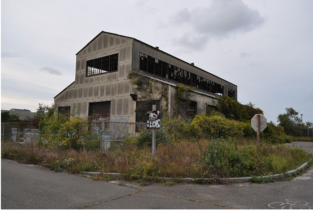
Figure 28. The World War II-era Ordnance Repair Shop (Building 9) with NPS parking area at right, 2014. This building, along with nearby warehouses (Buildings T-6, T-7) formed an industrial complex at the western side of the post. (Olmsted Center)
