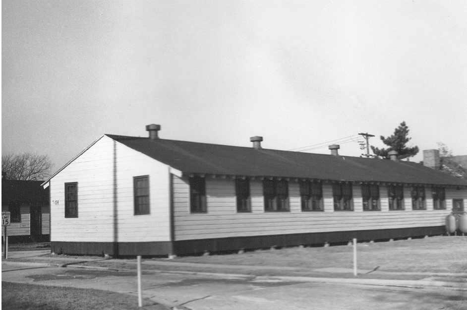
Figure 13. Former Provost Marshall building (T-128) on parade ground, typical of many Series 700 Army buildings of World War II era at Fort Tilden, circa 1974. This and most other frame buildings were razed in 1980s. (GATE Museum Collection 20980)
