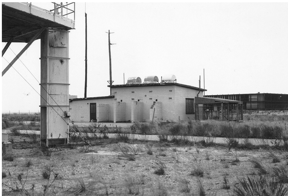
Figure 15. HIPAR station (Bldg 526) and radar platform of Nike tracking station #2, circa 1974. In 1980s, NPS redeveloped tracking station site as Fisherman's Parking Area, retaining only the HIPAR station. (Gateway Museum Collection, GATE 21034)
