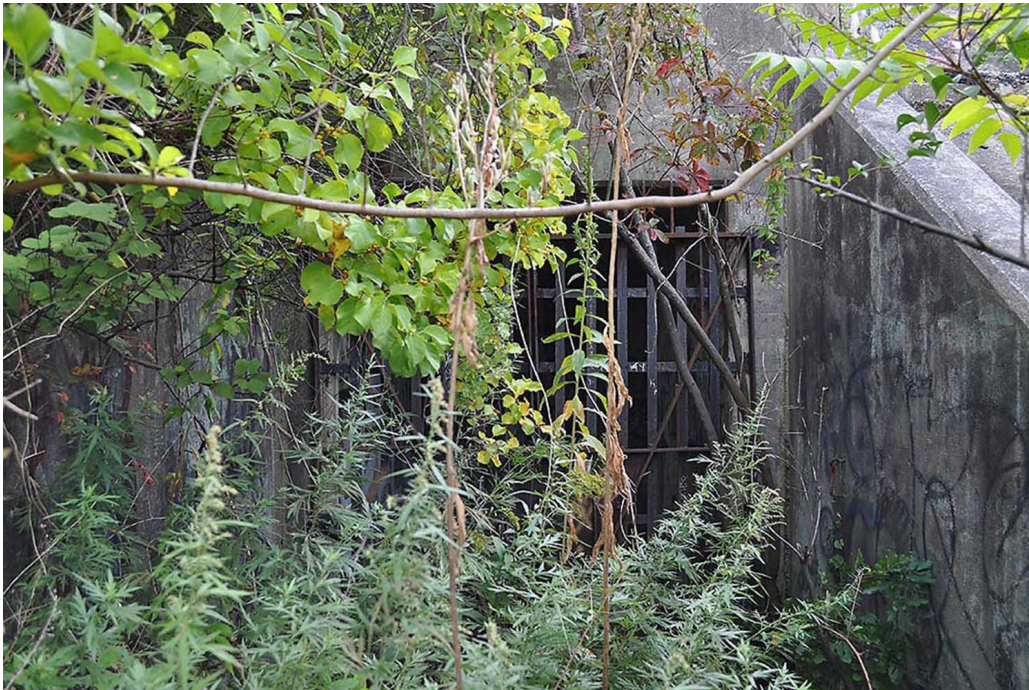
Figure 24. Gated entrance to earth-covered Mine Casemate and Plotting Room (B-511), 2014. (Olmsted Center)
