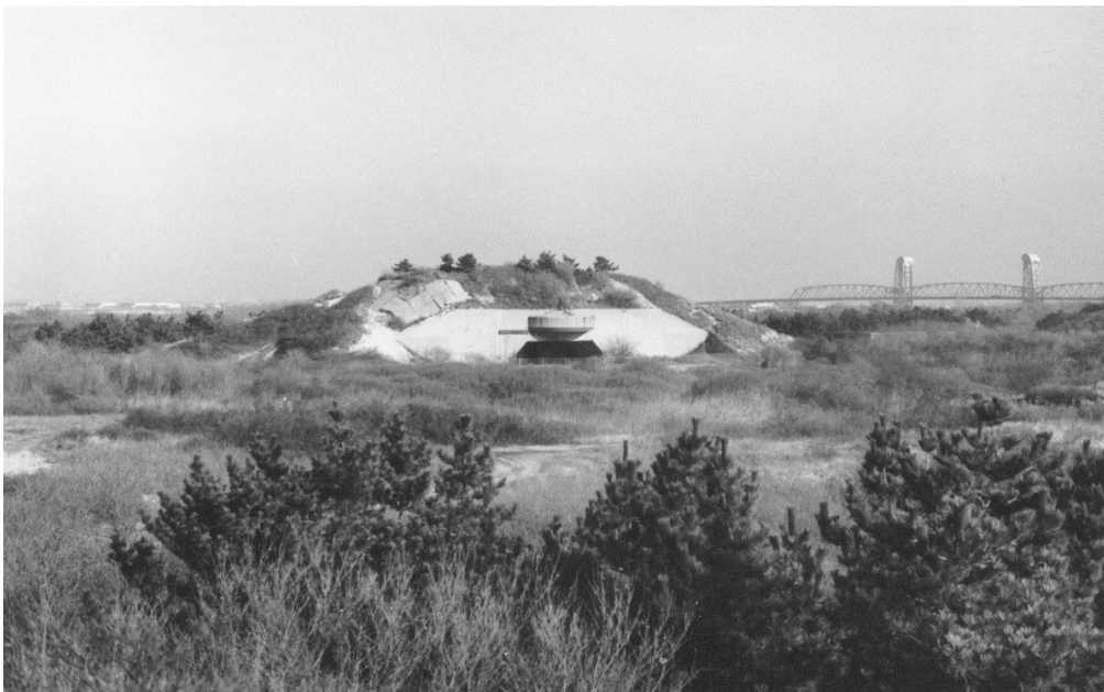
Figure 10. View northeast, ca. 1974, Battery Harris East (Bldg 406). Earthen/concrete casemate dates 1941-42. Army planted open grasslands and pines on casemate and in foreground during World War II. Gun removed ca. 1949. (GATE Museum Collection 21047)
