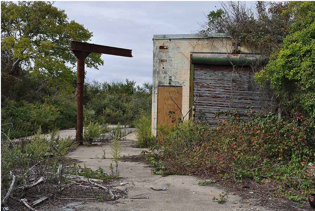
Figure 25. Park maintenance building (B-307), formerly the Nike missile warhead assembly building, looking northwest, 2014. (Olmsted Center)
