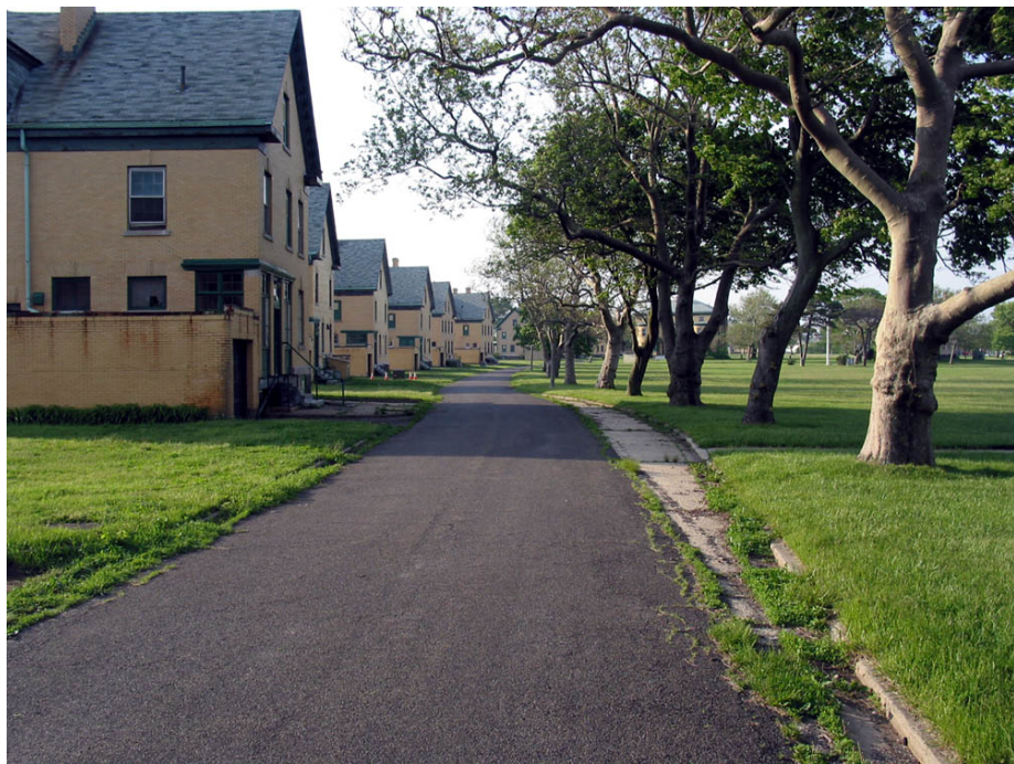
Figure 12. Kessler Road, looking north. The Parade Ground is to the right of the treeline (OCLP, 2007).
