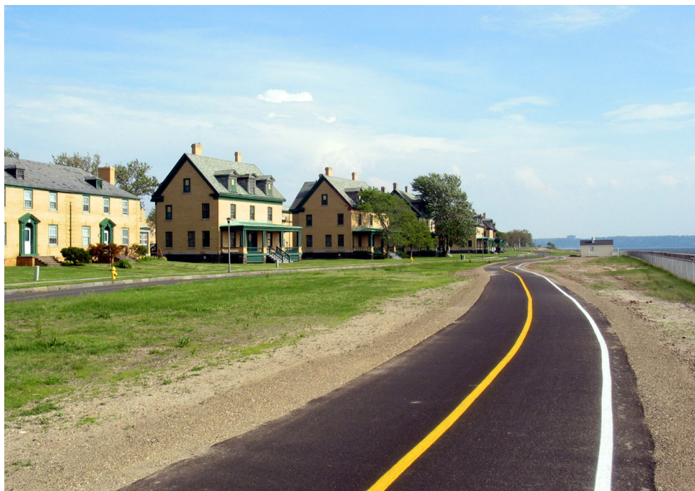
Figure 11. View of the multi-use path and Officer's Row, looking south (OCLP, 2007).
