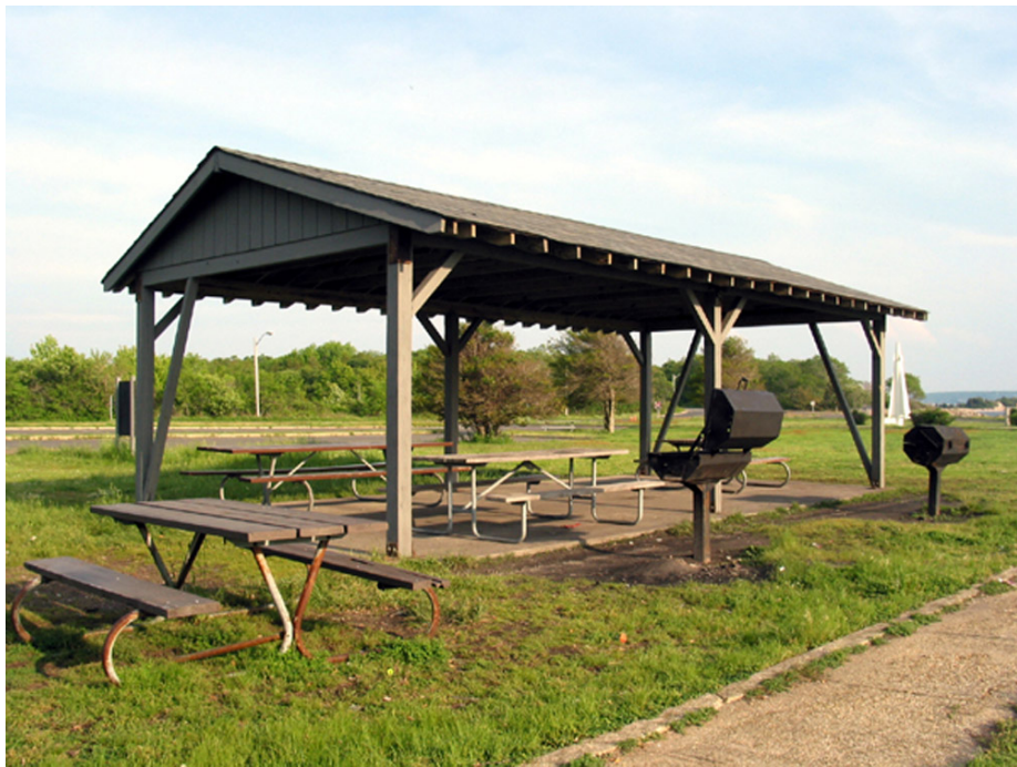
Figure 22. Several picnic shelters and barbecue pits are located in Guardian Park (OCLP, 2007).
