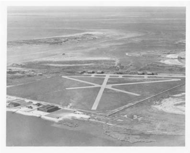
Figure 6. View of Floyd Bennett Field looking southwest, 1940. The 1940 Navy Seaplane Patrol Base and the Coast Guard Air Station are visible in the lower left side of the photograph (NPS Gateway NRA Museum Collection, Fort Wadsworth, photograph 18927).
