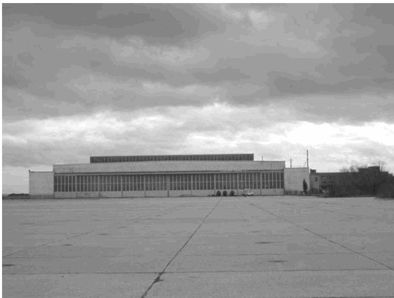
Figure 16. View looking south at Hangar B with the Navy Seaplane Patrol Base and apron. The design and construction of this World War II-era building contrasts with the municipal airport buildings of Hangar Row (see Fig. 13) (SUNY ESF, 2006).
