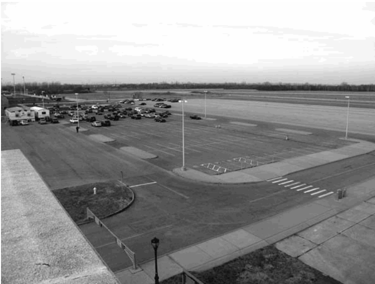
Figure 15. New parking lots were built on the apron and passenger loading area east of the Administration Building (SUNY ESF, 2006).
