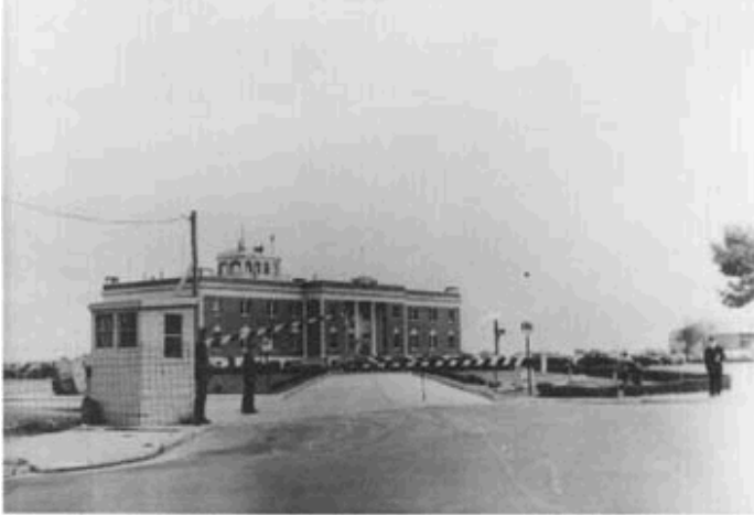
Figure 7. View of the airport entrance and Administration Building, 1942. The Navy installed the guard booths and gates to limit access ("Historic Structures Report," 251).
