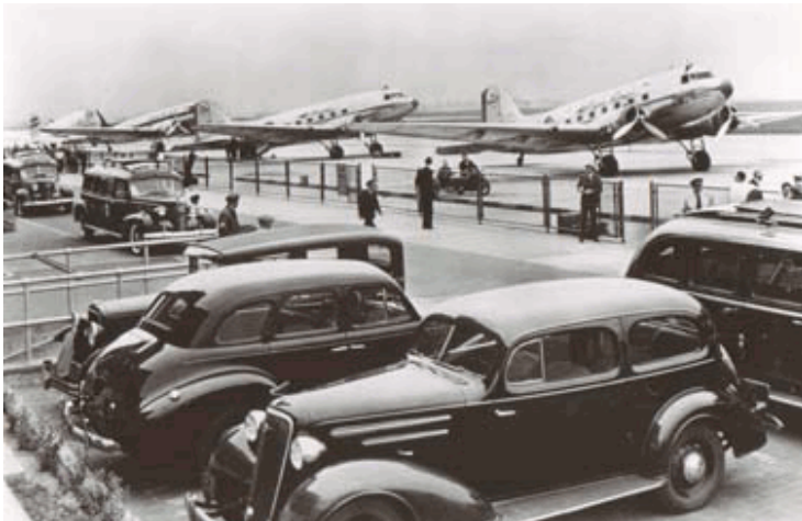
Figure 3. View of the airport looking northeast at the parking area north of the Administration Building, circa 1935-1940 (NPS Gateway NRA Museum Collection, Fort Wadsworth, photograph 18963).
