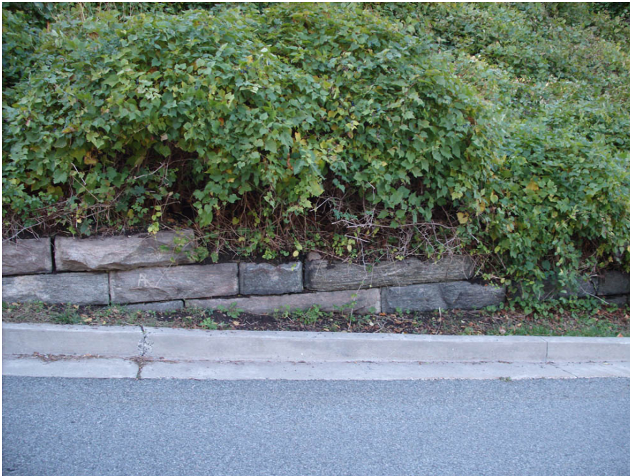
Figure 29. The slope retaining wall (BS-14), built in c.1848, view look west with Battery Weed Road in the foreground. (SUNY ESF, 2007)
