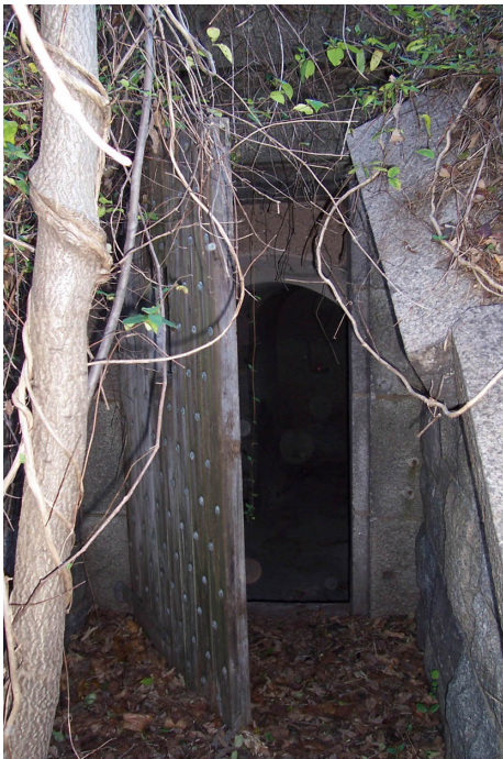
Figure 25. The exterior entry of the Battery Catlin parados (BS-8) built in c.1865, looking east showing granite cheek walls and overgrown conditions. (SUNY ESF, 2007)
