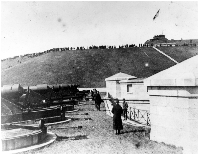
Figure 8. A photograph taken in 1902 looking southwest toward Fort Tompkins showing the barbette tier of Fort Wadsworth (Battery Weed) with its rotating guns still in place. (Photograph 19401, NPS/Gateway NRA Museum Collection)
