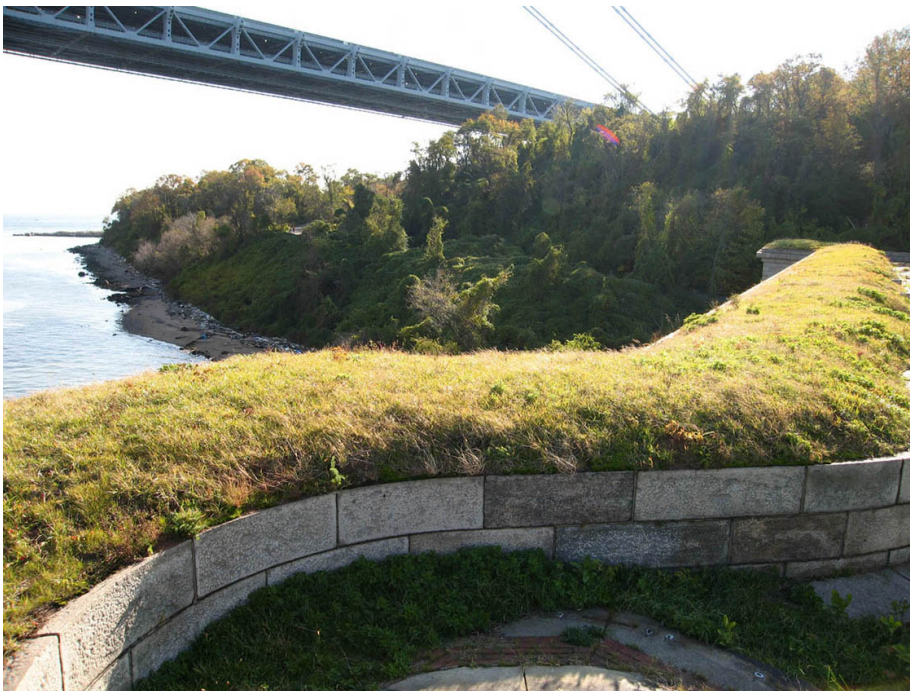
Figure 20. The vine and tree-covered Battery Bacon earthwork (T-3) built in c.1898 above the shoreline, looking southeast from the parapet of Battery Weed. The battery is the area above the shoreline. (SUNY ESF, 2007)
