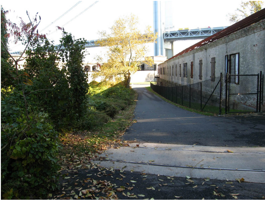
Figure 18. Battery Weed Road (C-1), looking southeast along the Torpedo Storage Building. The concrete surfaced track of the mine railway extends across the road from the rear of the building. (SUNY ESF, 2006)
