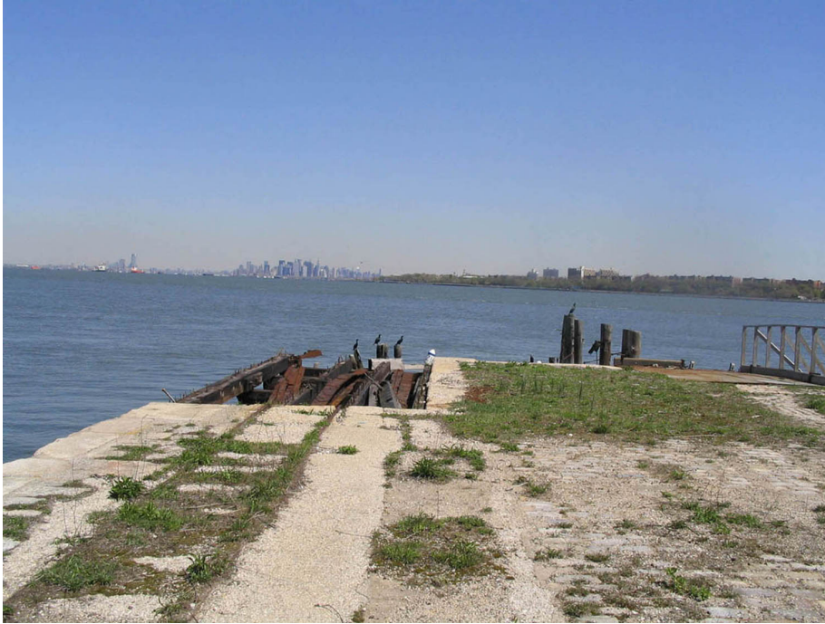
Figure 24. The north dock (BS-6), built in c.1859, view looking northeast showing granite and concrete surface, and remnants of the mine railway and timber extension dating to 1907. (SUNY ESF, 2007)
