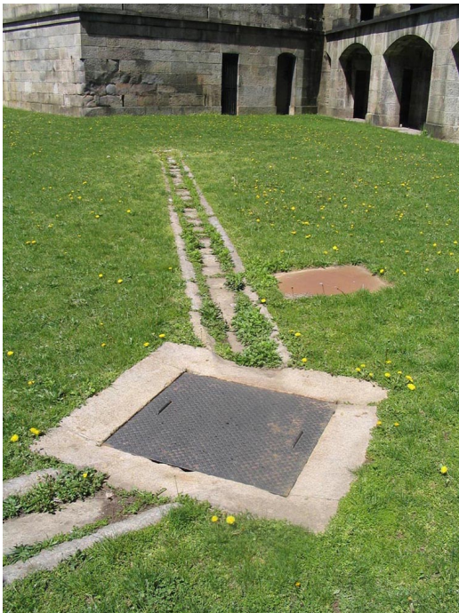
Figure 27. The stone gutters and cistern (BS-12), built c.1847-1864, looking west with contemporary cistern hatch in the foreground. (SUNY ESF, 2007)
