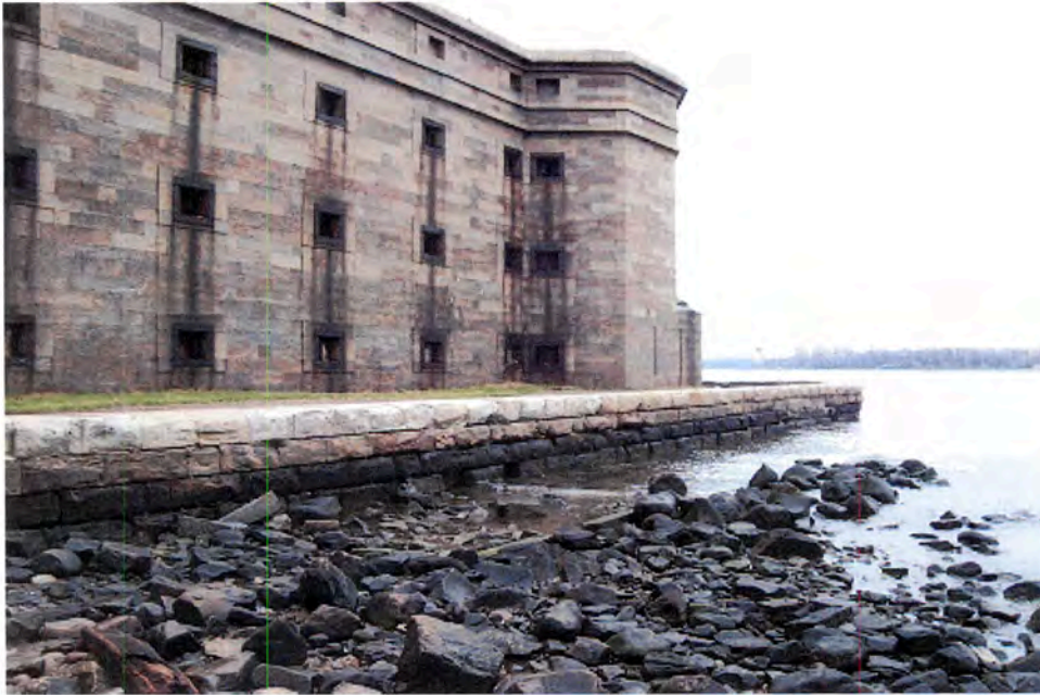
Figure 22. Battery Weed (BS-1), constructed between 1847 and 1864, and the seawall (BS-2) completed in c.1871, view looking northeast at section that forms the outer wall of the moat around Battery Weed. (SUNY ESF, 2007)
