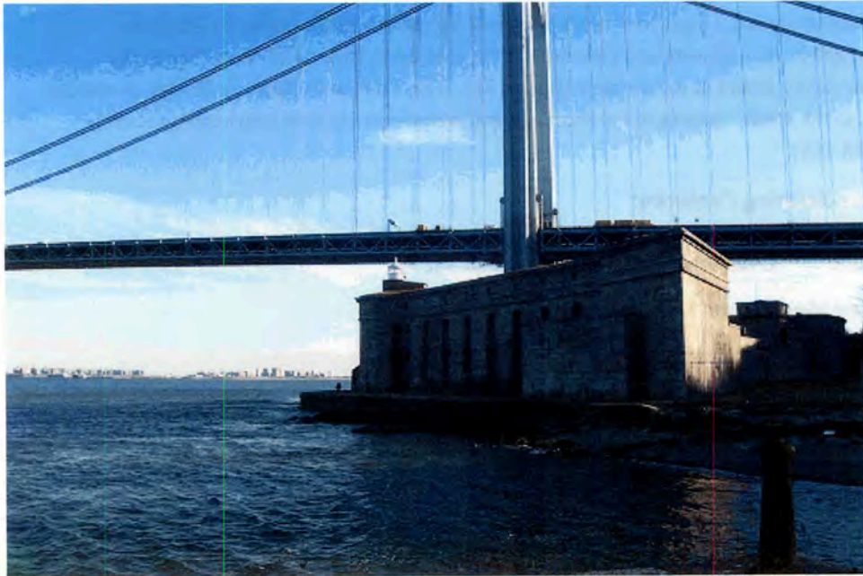
Figure 31. Water-level views (VV-2) looking southeast from the north dock with Coney Island (Brooklyn) in the distance. One of two iron dock bollards (SS-11) is in the foreground. (SUNY ESF, 2007)
