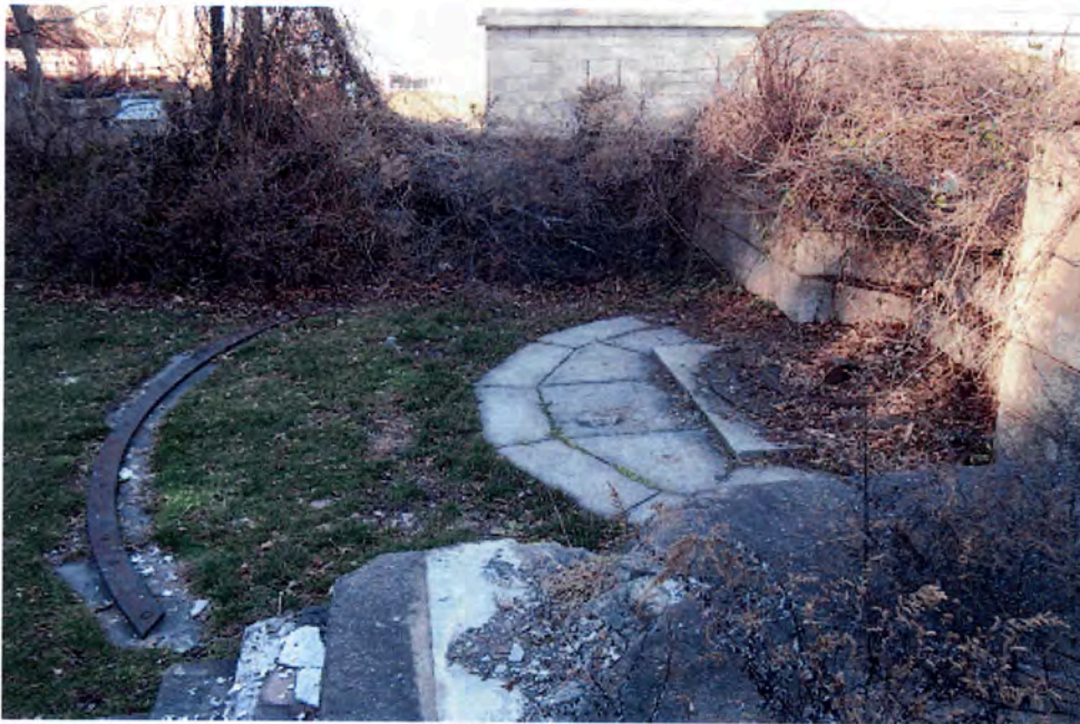
Figure 26. The gun emplacement (BS-9) at Battery Bacon (see T-3) built in c.1898 looking north showing concrete platform and parapet walls, iron pintle, and traverse circle. (SUNY ESF, 2007)
