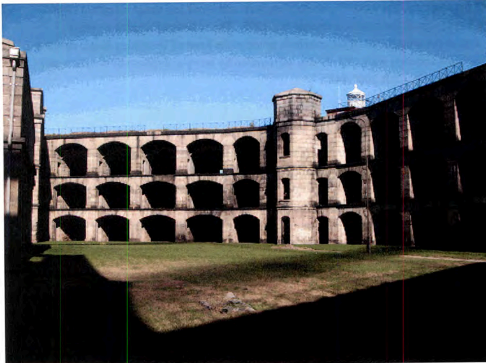
Figure 14. The parade ground (SO-1) view looking northeast, is enclosed by a half-hexagon of arched granite casemates with two four-story stair towers and guardhouse on the west side. (SUNY ESF, 2006)
