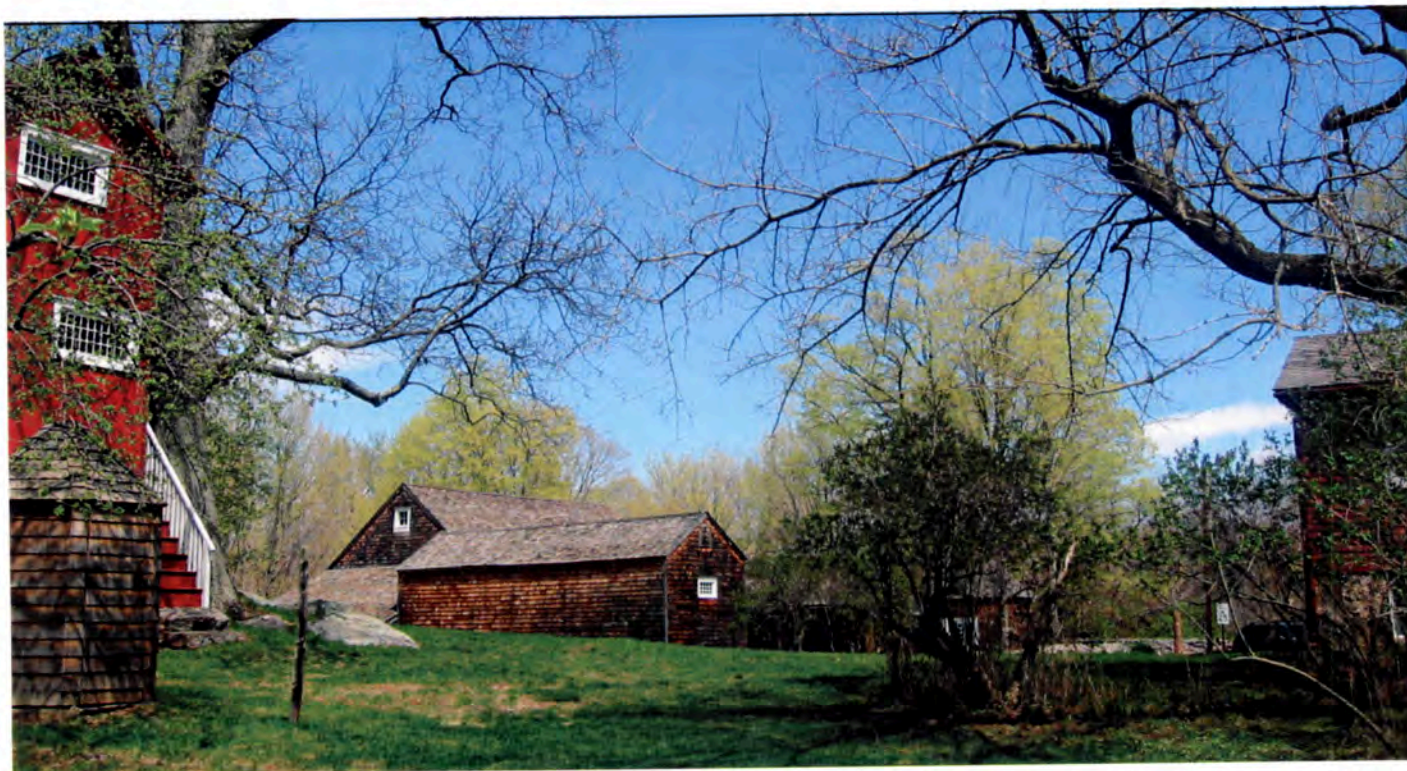
Documenting existing conditions at Weir Farm National Historic Site in Wilton, Connecticut (OCLP, 2003).
