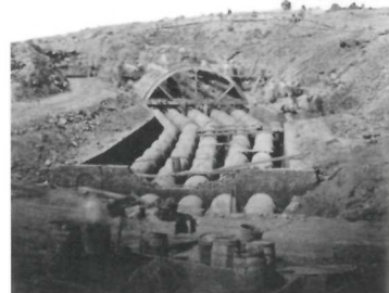
Workers install Central Park water system.
