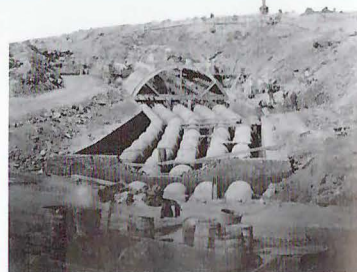
Workers install Central Park water system.
