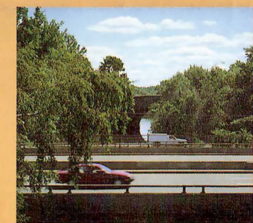
Boston roads have encroached on Olmsted's compositions, as shown at the entrance to Back Bay Fens.
