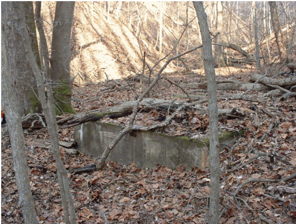
Concrete foundation of World War II era water pumping station in ravine north of Battery Wilkin, December 2004 (Laird).
