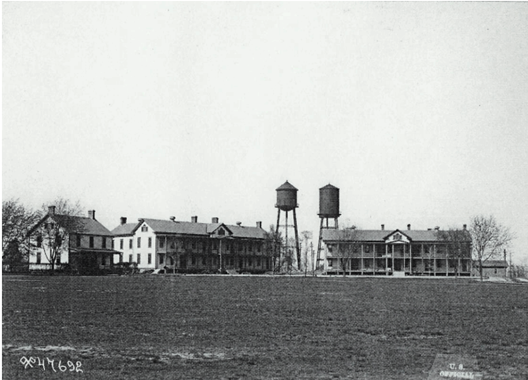
The former admin building, Coast Defense HQ (left) and large enlisted men's barracks, were located what is now a open field by east end of the Washington Dr. loop. (NARA RG 111-SC, Records of the Office of the Chief Signal Officer, Box 357, #47692).
