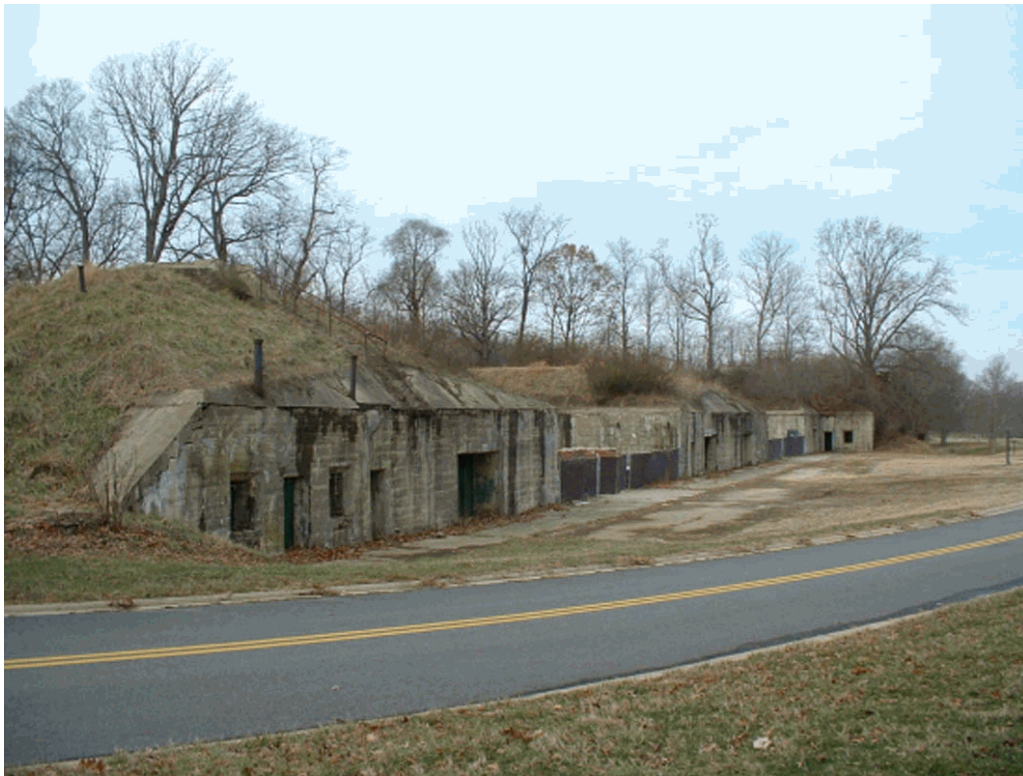
Battery Meigs, view to north, December 2005 (Laird).
