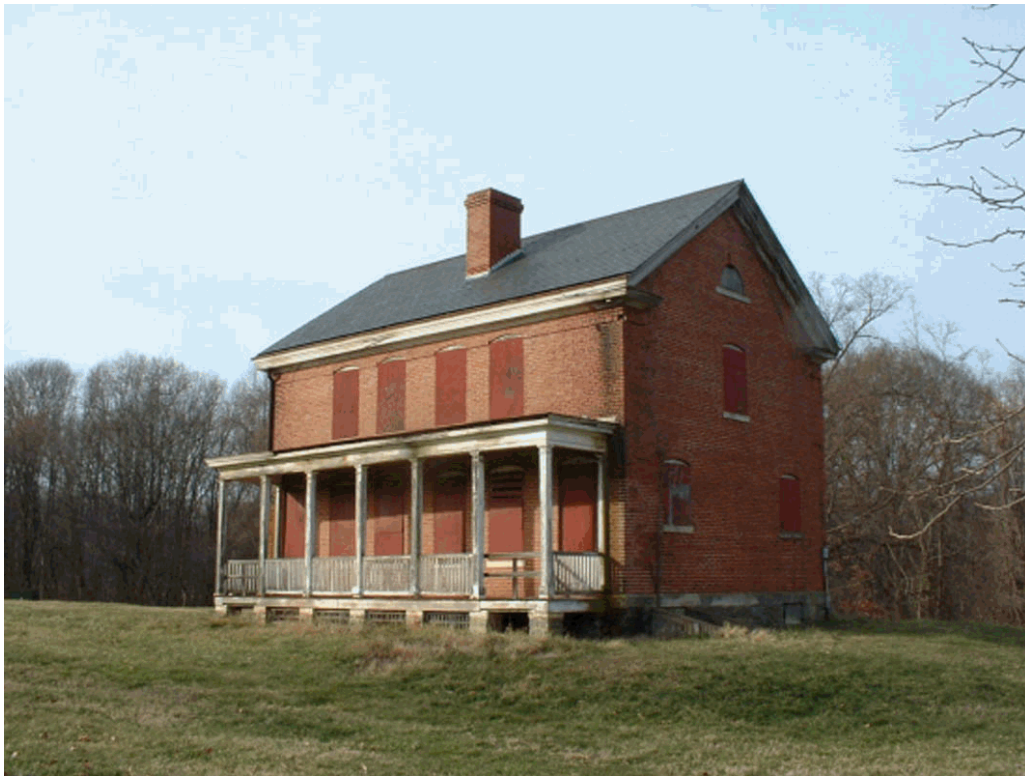
Bachelor NCO Quarters, view to southwest, December 2005 (Laird).
