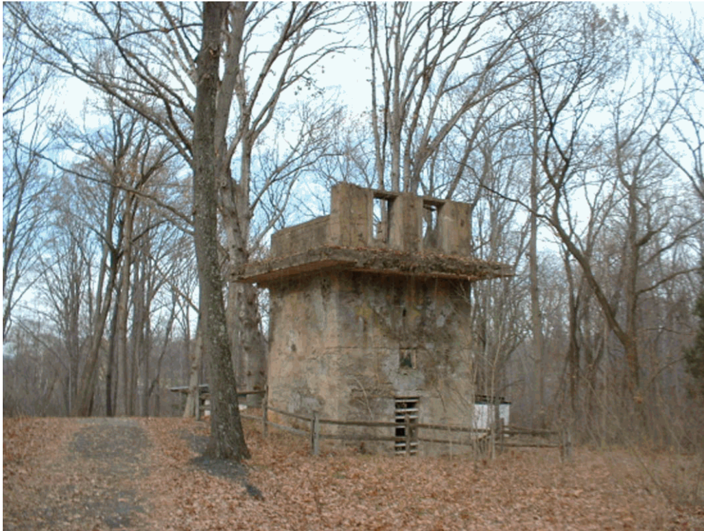
Southeast Fire Control Tower with Paint Shop Building in background, view to north, December 2005 (Laird).
