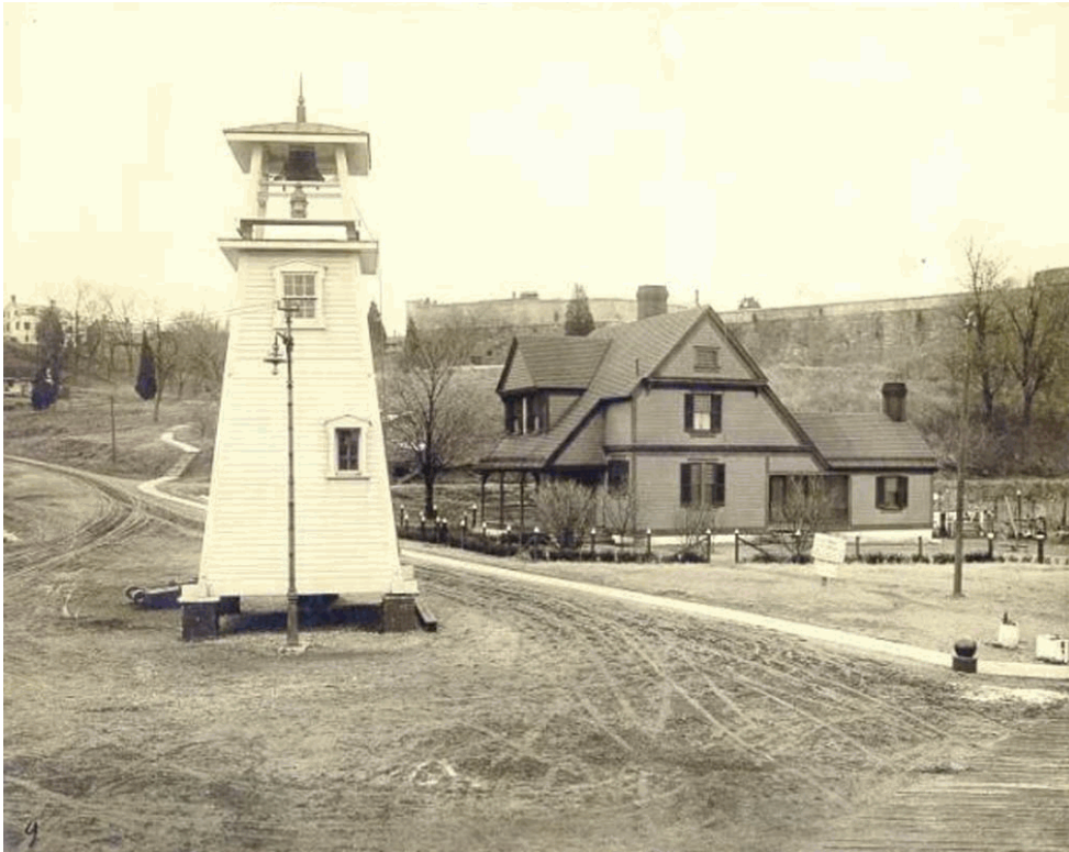
The Light 80 (originally built as a fog bell tower in 1882), and the ca. 1885 lighthouse keeper's house at Digges' Point shown in 1912. Note the Endicott period electric lamppost adjacent to the lighthouse. (Fort Washington photo files).
