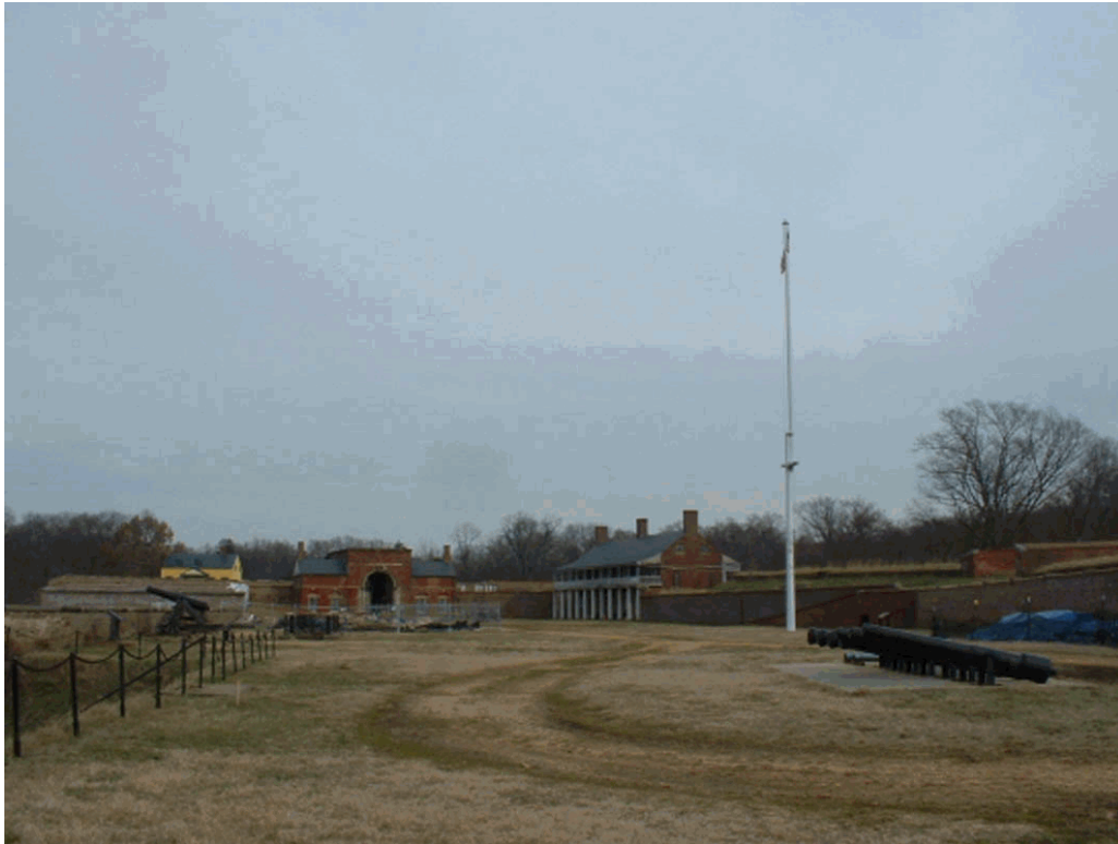
Fort Washington Parade, view to northeast, December 2005. Visible are the gatehouse, officers' quarters, flagstaff, artillery display, and 24-pounder cannon (Laird).
