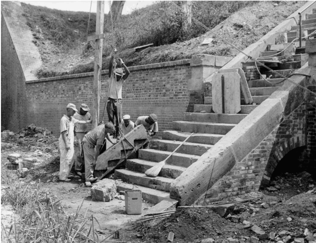
Stone coping is replaced on steps in the southwest demibastion in 1958. Rehabilitation efforts were funded under the Mission 66 program, but were halted the following year due to budget cuts (Fort Washington photo files).
