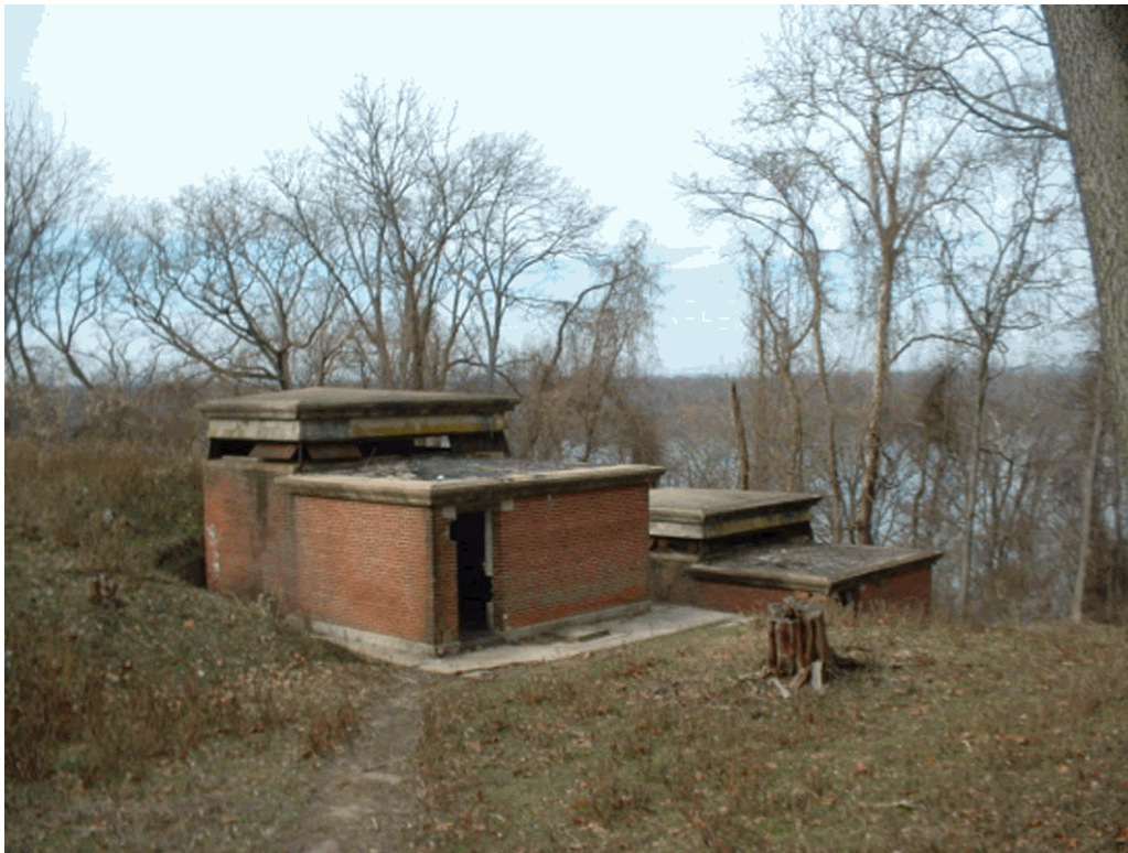
Command Structures, view to west, December 2005 (Laird).
