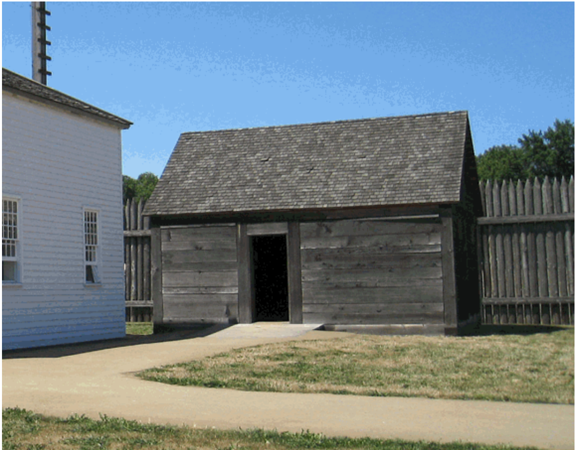
Jail, looking northwest (PWRO, 2009).
