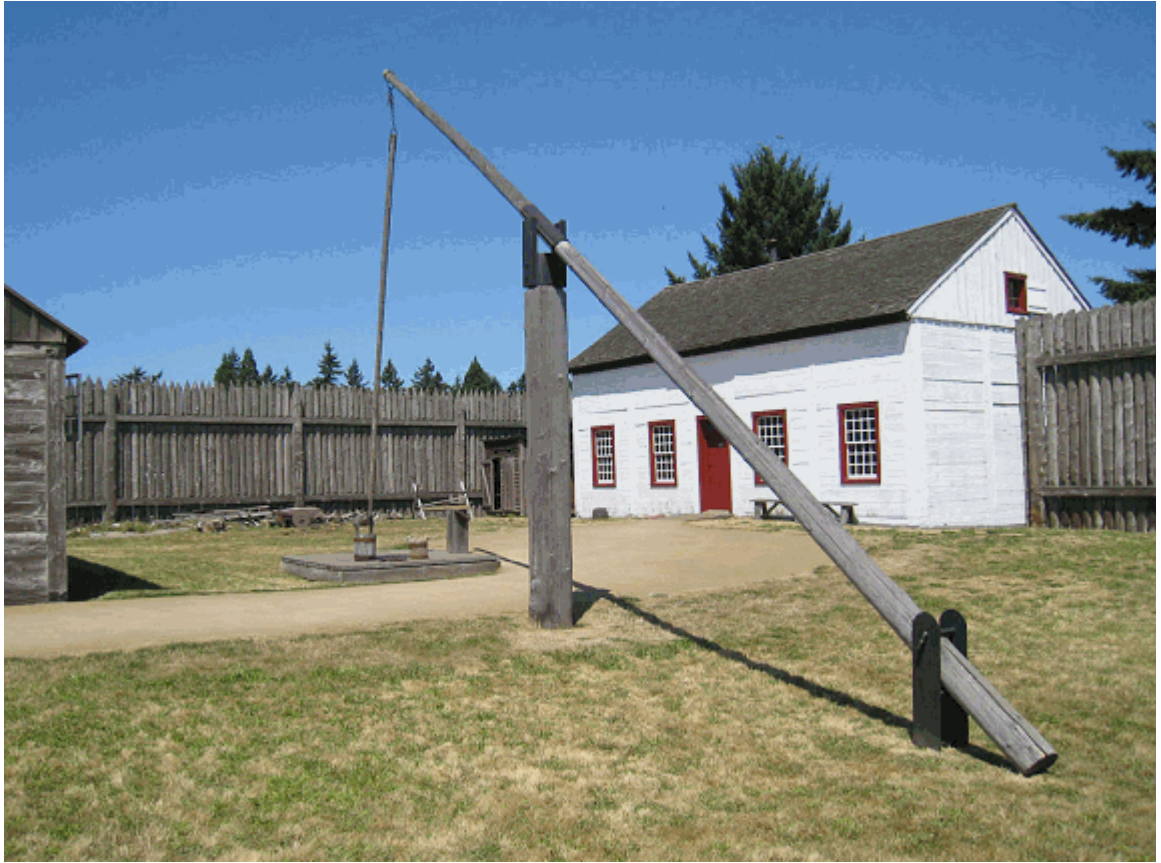
Restored well and reconstructed well sweep, looking northeast (PWRO, 2009).
