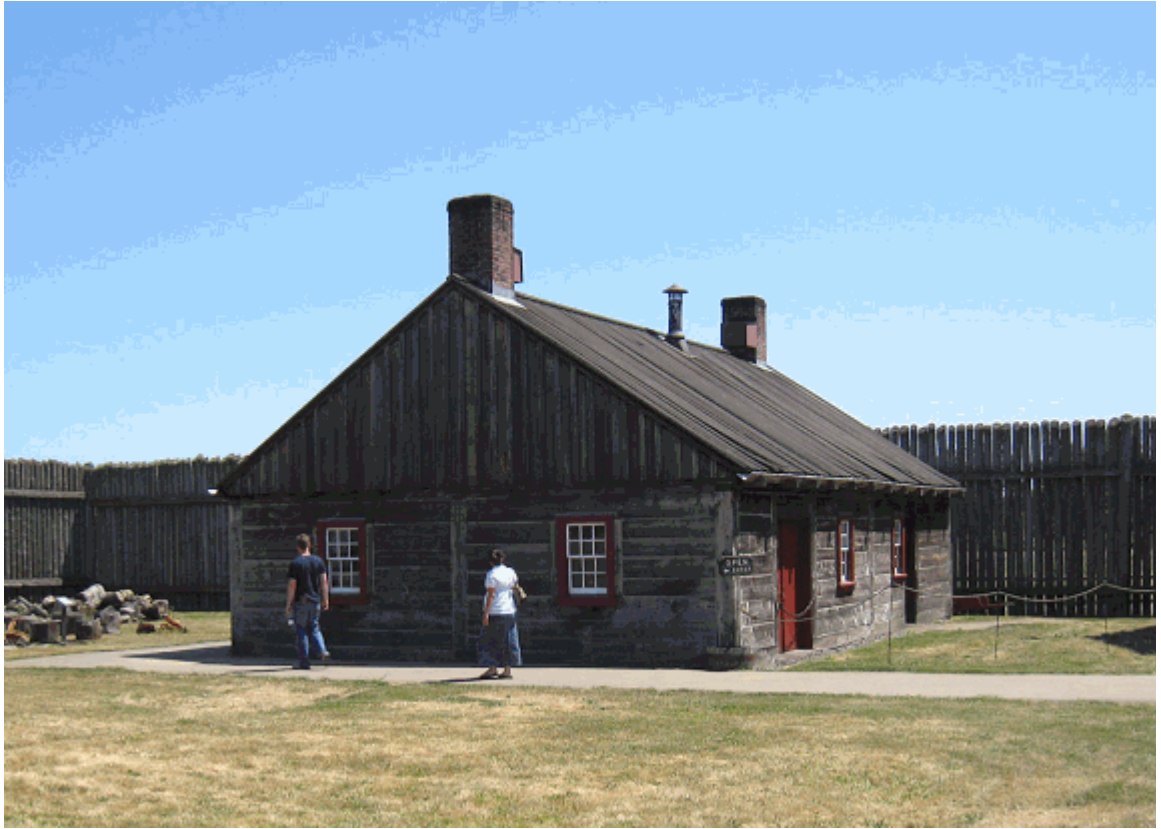
Blacksmith shop, looking southeast (PWRO, 2009).
