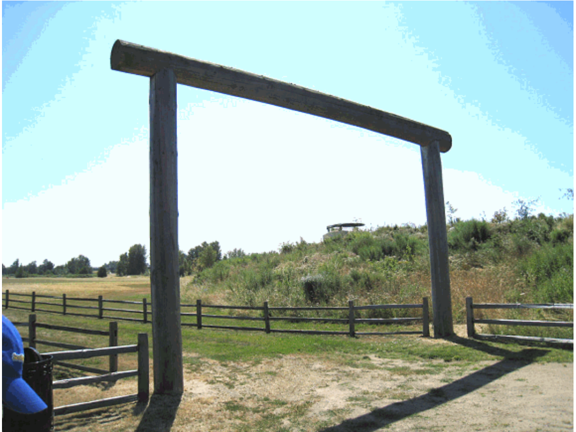
HBC Village Entrance Gate, looking southeast (PWRO, 2009). The base of the landbridge rises behind the gate and the hillside is planted with native vegetation.
