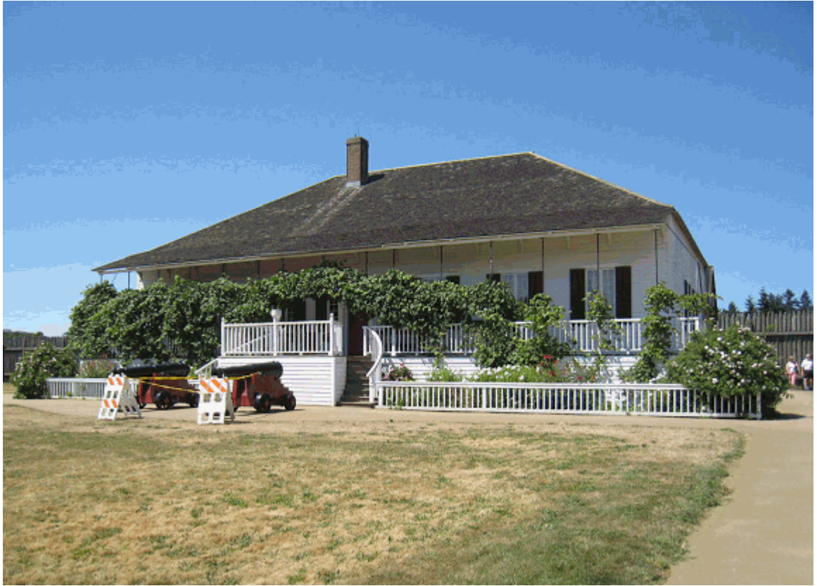
Chief Factor's House, looking northwest (PWRO, 2009).
