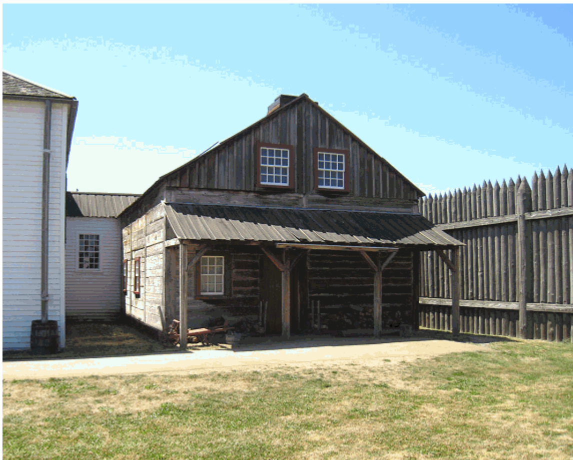
Kitchen, looking northwest (PWHO, 2009).
