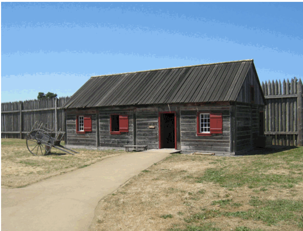
Carpenter shop, looking northwest (PWRO, 2009).
