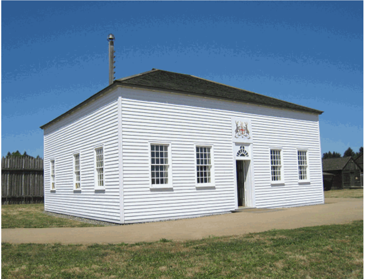
Counting house with belfry in background, looking northeast (PWRO, 2009).
