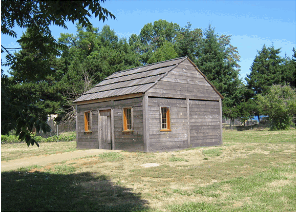
HBC Village house #1, looking northwest (PWRO), 2009).
