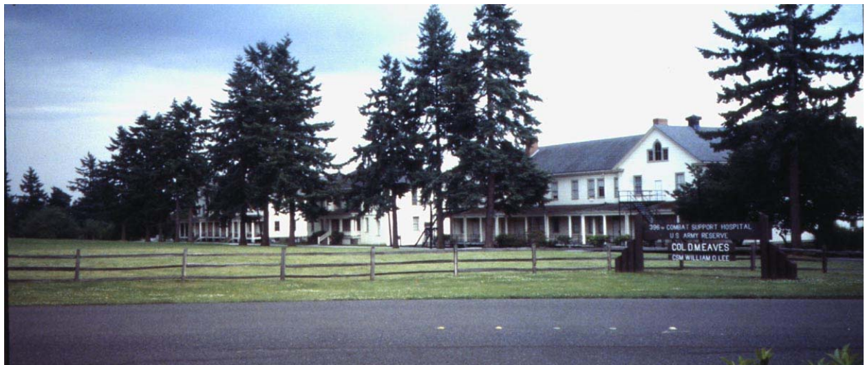
Historic barracks and headquarters buildings along the southern edge of the Parade Ground reflect the post's general development during the late nineteenth century. (PWRO, 2003)
