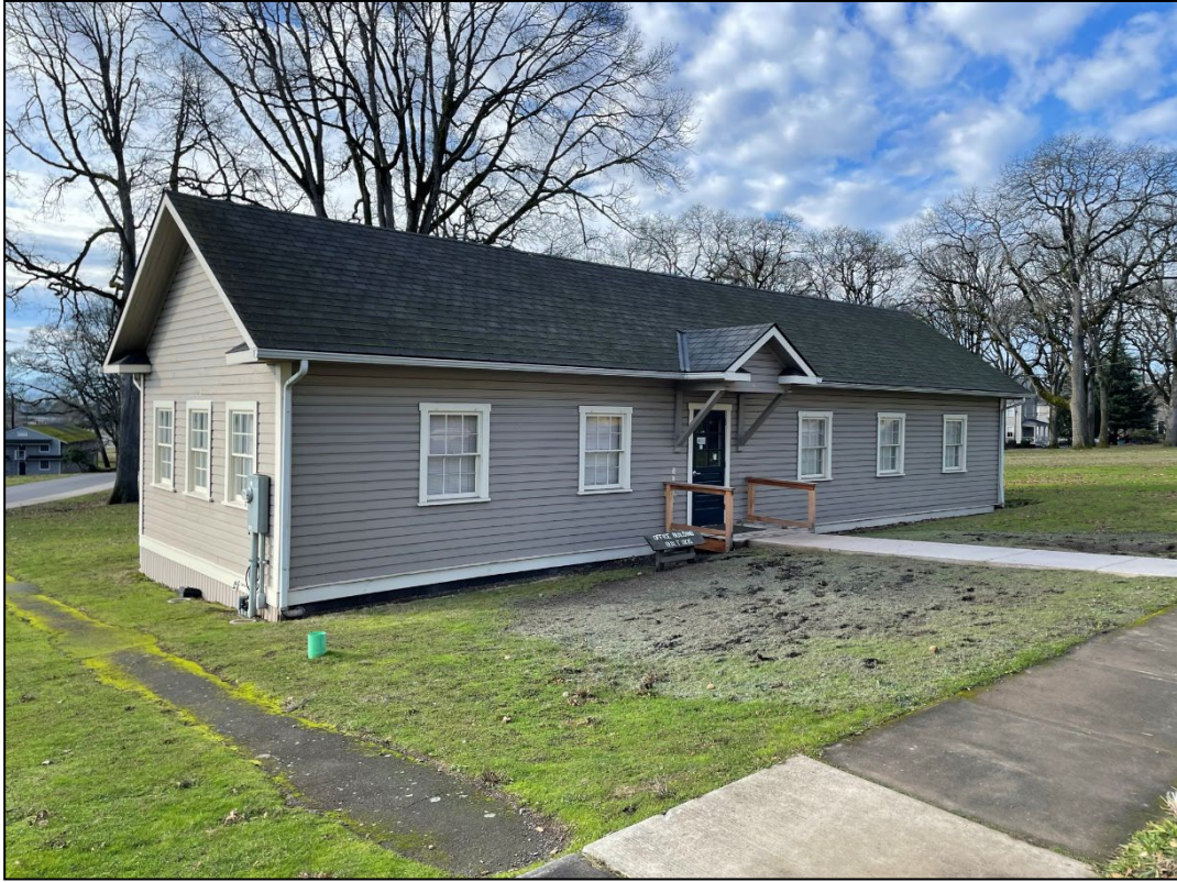
Figure 48. Building 704 (Contributing, CRIS CL ID 202902, CRIS HS ID 956505) (MIG January 2023)
