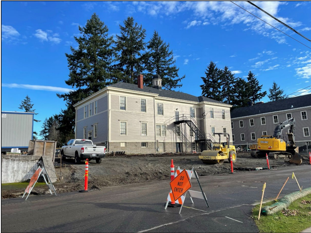
Figure 62. Building 991 (Contributing, CRIS CL ID 202918, CRIS HS ID 956538) (MIG January 2023)
