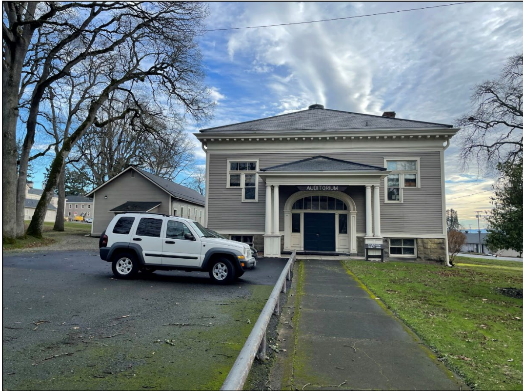
Figure 49. Building 721 (Contributing, CRIS CL ID 202905, CRIS HS ID 956509) (MIG January 2023)
