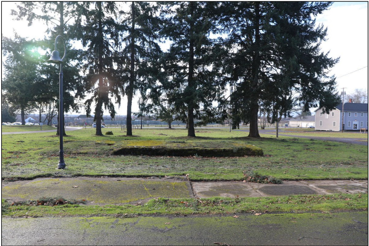
Figure 66. Historic Bakehouse Building Foundation. (contributing, CRIS CL ID 202921 (MIG January 2023))
