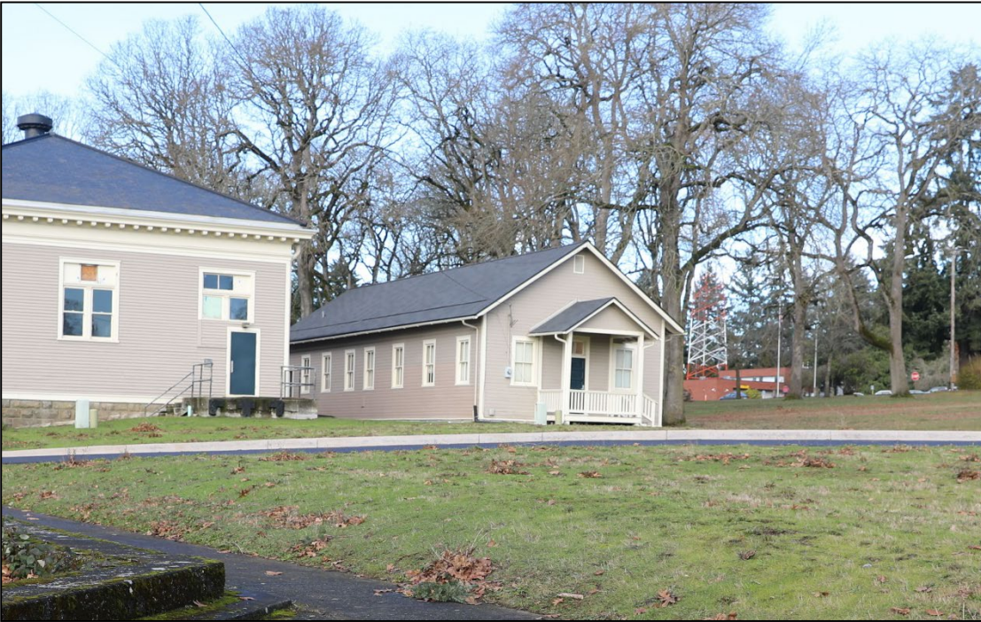
Figure 50. Building 722 (Contributing, CRIS CL ID 202906, CRIS HS ID 956512) (MIG January 2023)
