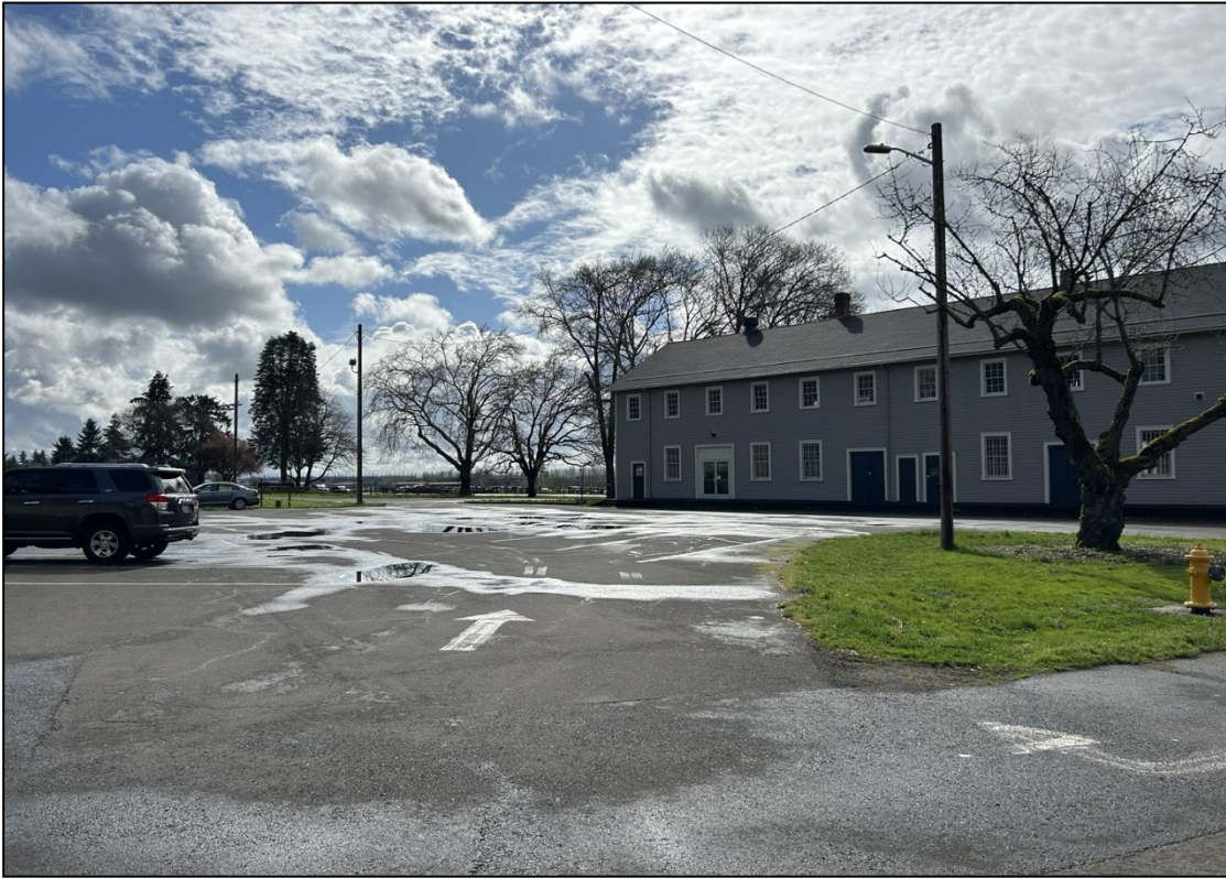
Figure 40. Central Lot Parking Area (Contributing, CRIS CL ID 202893) (NPS 2024)
