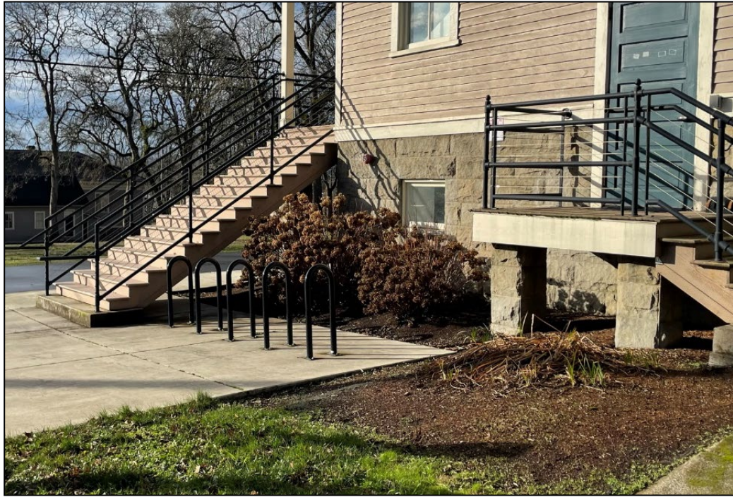
Figure 69. Bike rack next to building 987. (noncontributing, CRIS CL ID 202924) (MIG January 2023)
