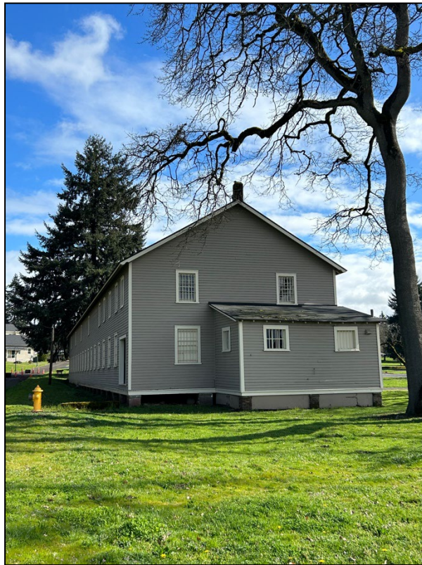
Figure 56. Building 752 (Contributing, CRIS CL ID 202912, CRIS HS ID 956534) (NPS, 2024)
