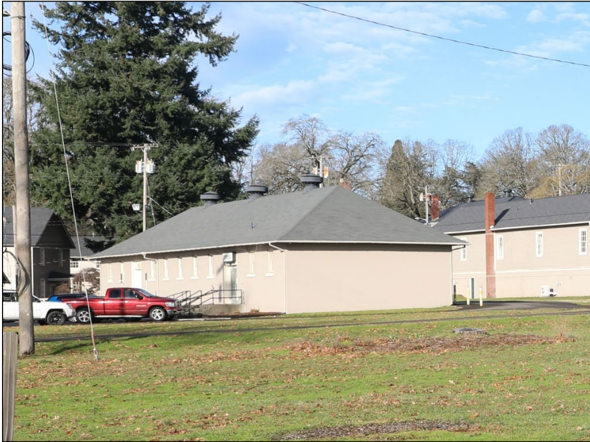
Figure 58. Building 754 (Contributing, CRIS CL ID 202914, CRIS HS ID 956531) (MIG January 2023)
