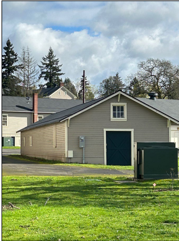
Figure 57. Building 753 (Contributing, CRIS CL ID 202913, CRIS HS ID 956533) (NPS, 2024)
