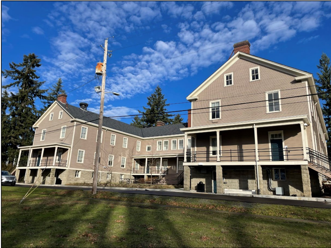
Figure 60. Building 987 (Contributing, CRIS CL ID 202916, CRIS HS ID 956907) (MIG January 2023)
