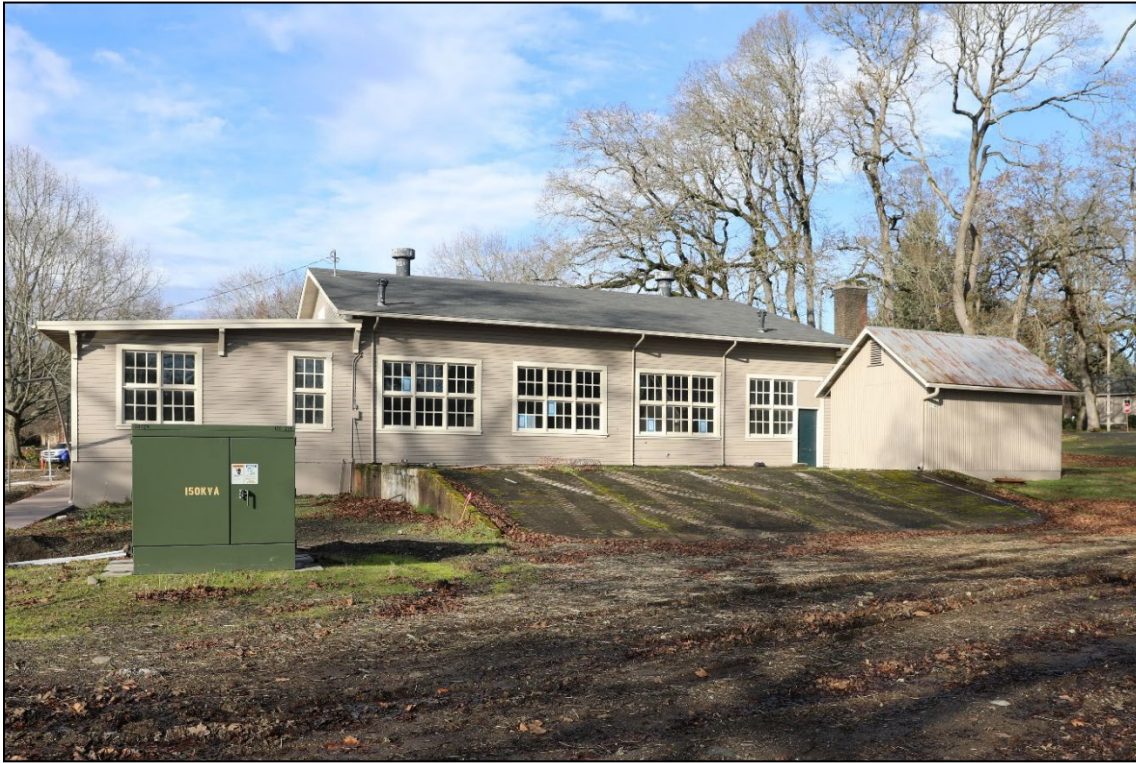
Figure 55. Building 748 (Contributing, CRIS CL ID 202911, CRIS HS ID 956528) (MIG January 2023)
