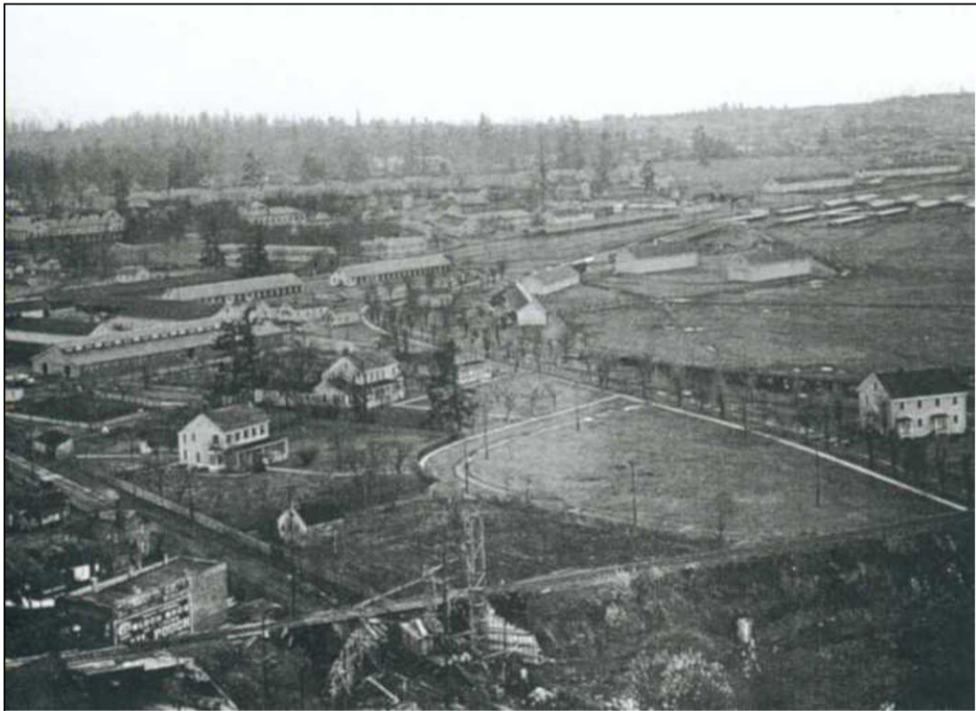
Figure 13. Photograph of Vancouver Barracks, circa 1917, looking northeast from the old Quartermaster's depot area, across East 5th Street to the Parade Ground beyond. (2018 East Barracks/Parade Ground Cultural Landscape Inventory)
