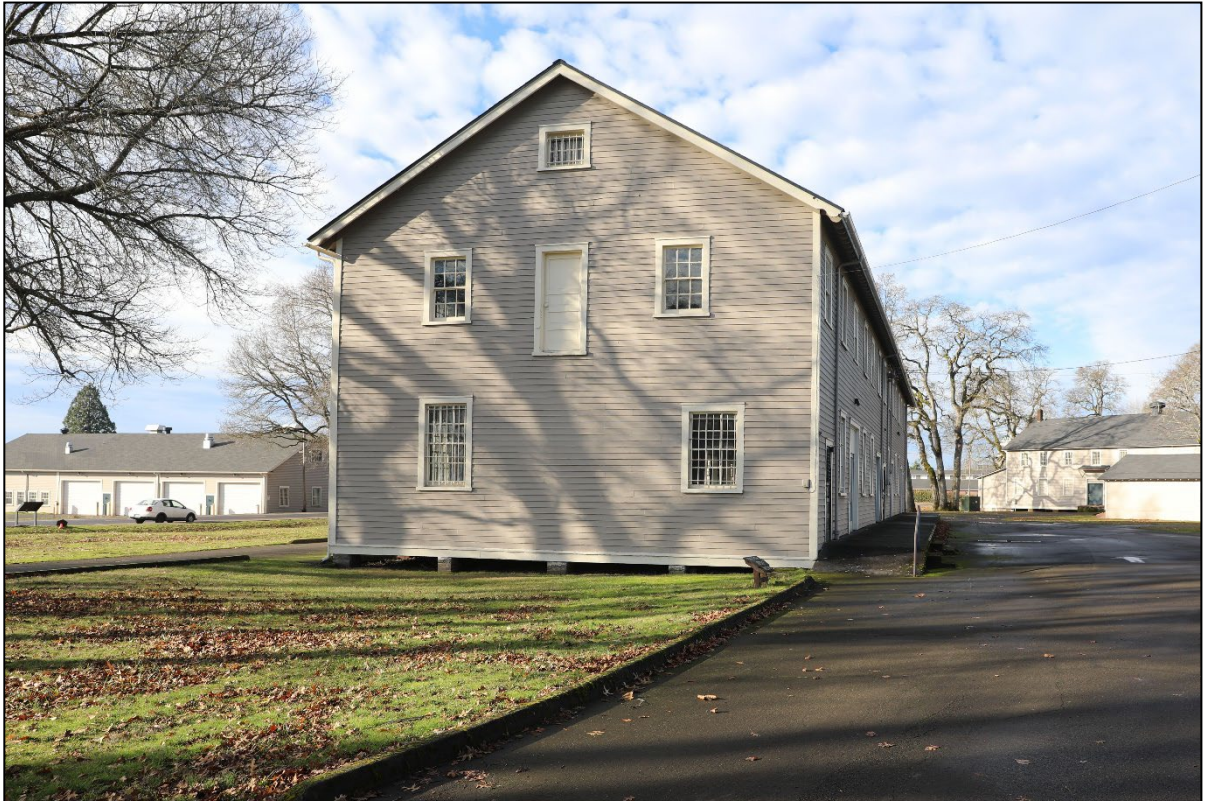
Figure 59. Building 786 (Contributing, CRIS CL ID 202915, CRIS HS ID 956535 (MIG January 2023))
