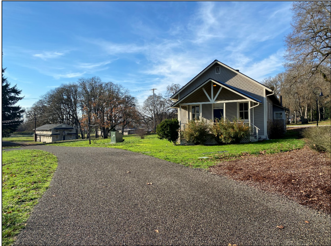
Figure 35. Alvord Road, looking southwest. (contributing, CRIS CL ID 202889) (MIG January 2023)
