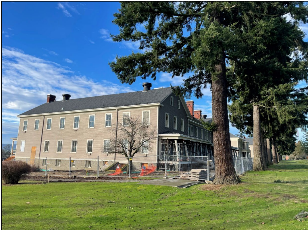
Figure 63. Building 993 (Contributing, CRIS CL ID 202919, CRIS HS ID 956537) (MIG January 2023)
