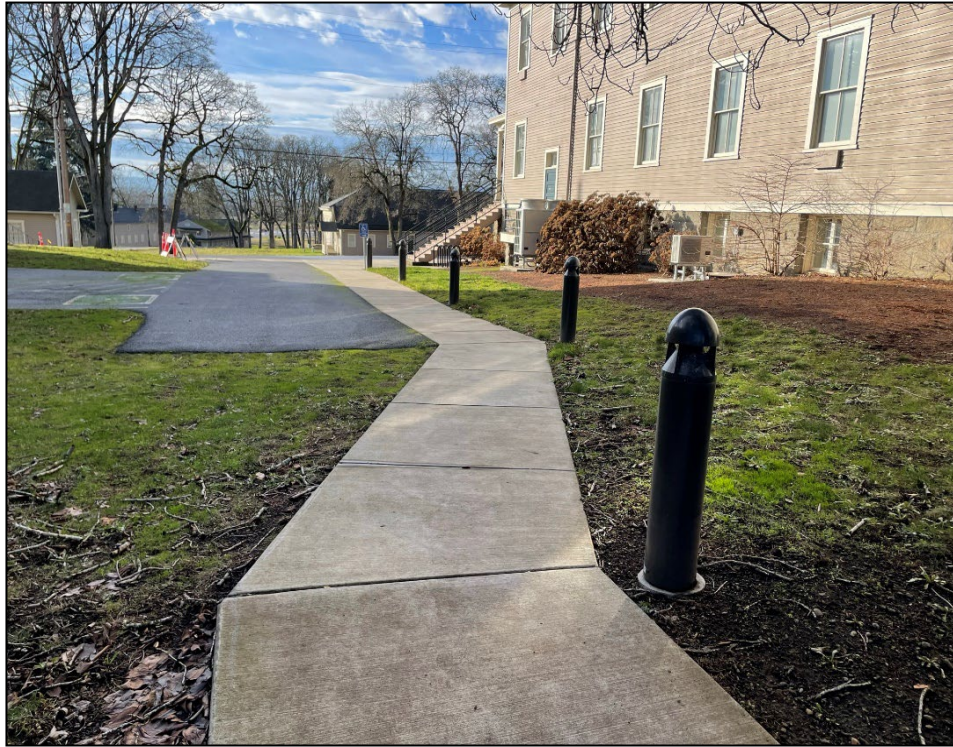
Figure 70. Lighted bollards between buildings 987 and 989. (noncontributing, CRIS CL ID 202925) (MIG January 2023)
