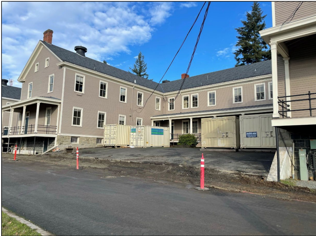
Figure 61. Building 989 (Contributing, CRIS CL ID 202917, CRIS HS ID 956536) (MIG January 2023)
