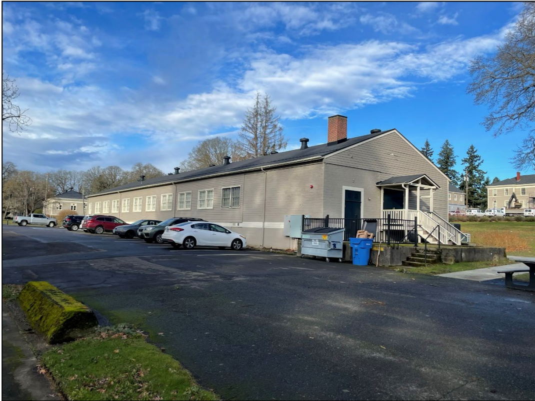
Figure 52. Building 728 (Contributing, CRIS CL ID 202908, CRIS HS ID 956519) (MIG January 2023)
