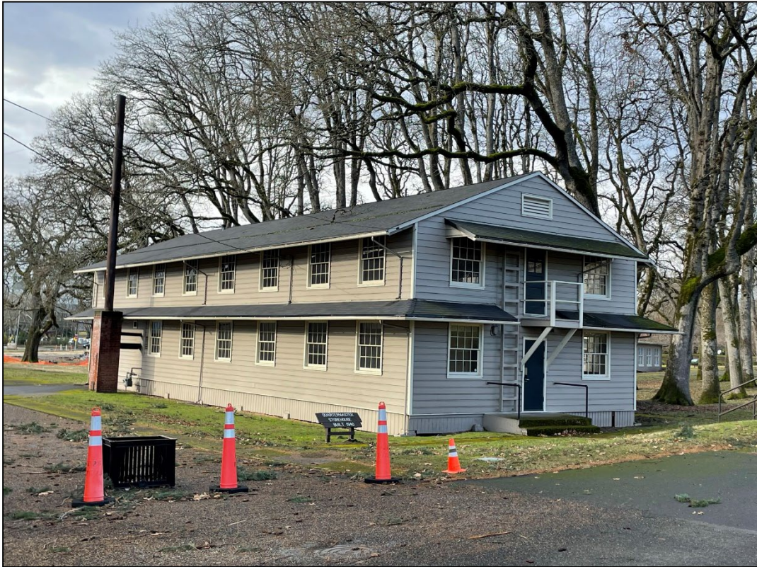
Figure 54. Building 746 (Contributing, CRIS CL ID 202910, CRIS HS ID 956524) (MIG January 2023)
