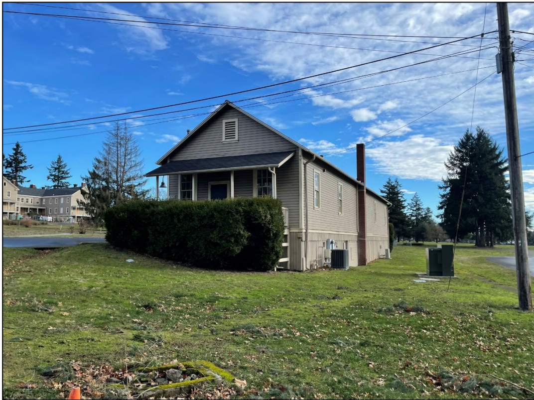
Figure 53. Building 733 (Contributing, CRIS CL ID 202909, CRIS HS ID 956521) (MIG January 2023)
