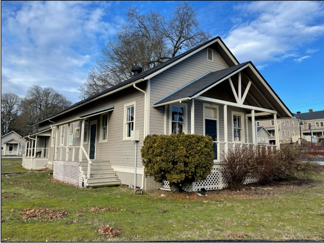
Figure 51. Building 725 (Contributing, CRIS CL ID 722907, CRIS HS ID 956515) (MIG January 2023)
