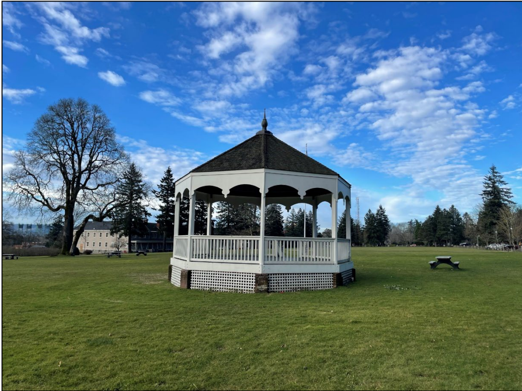
Figure 64. Bandstand on eastern edge of Parade Ground Bandstand (Noncontributing, CRIS CL ID 104880, CRIS HS ID 1170705) (MIG January 2023)
