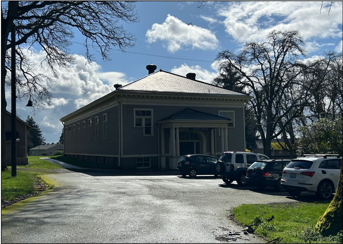
Figure 43. Gymnasium Lot Parking Area (Noncontributing, CRIS CL ID 202897) (NPS 2024)
