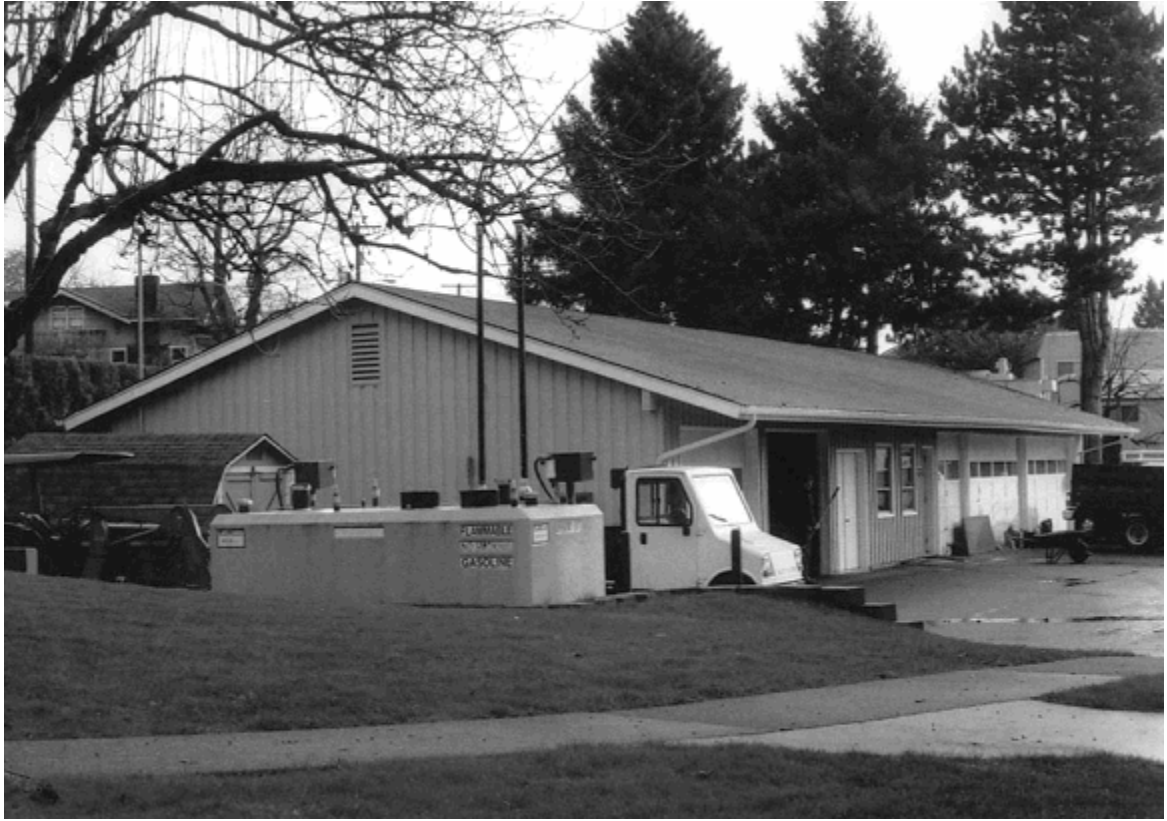
Contemporary photo showing the Mission 66 Maintenance Shop, looking northeast (PWRO, 2004).
