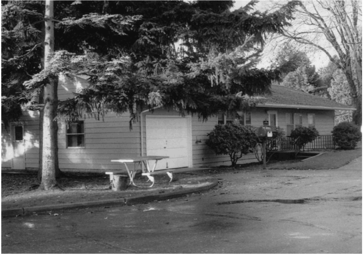
Contemporary photo showing Mission 66 Residence No. 1, looking southwest (PWRO, 2004).
