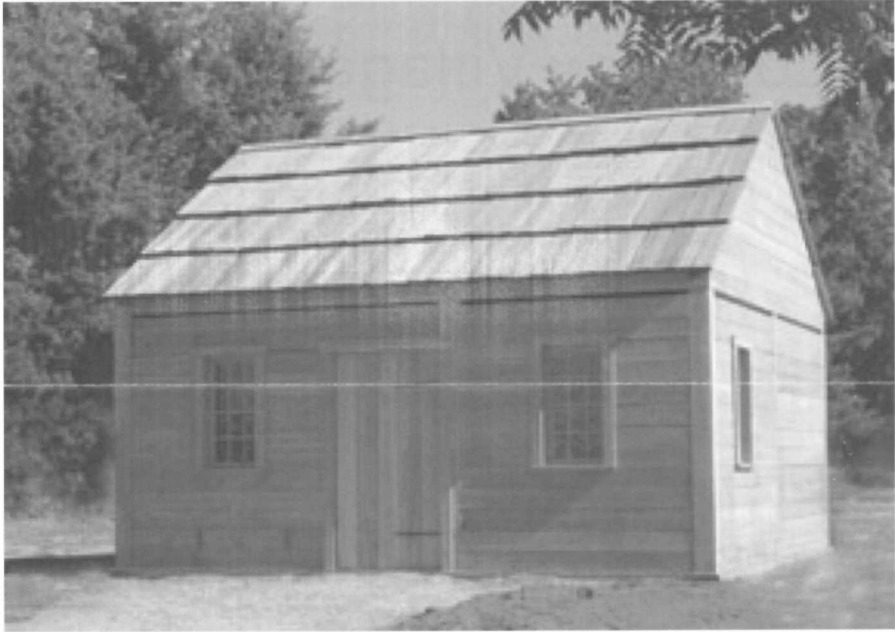
The reconstructed Engagé House, showing typical Canadian post-on-sill construction (National Park Service)
