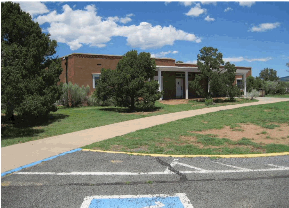
Front façade of the Visitor Center from the western parking area, facing northeast, July 2010. Source: National Park Service.
