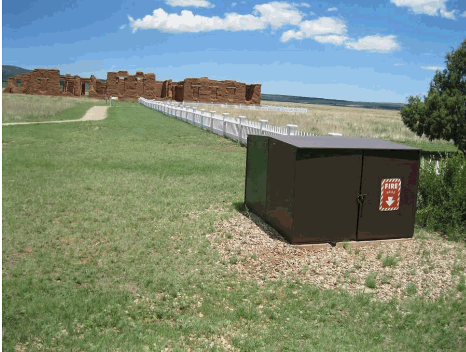
Large brown firebox located on the north side of the white picket fence on the eastern side of the Visitor Center, facing east, July 2010. Source: National Park Service.
