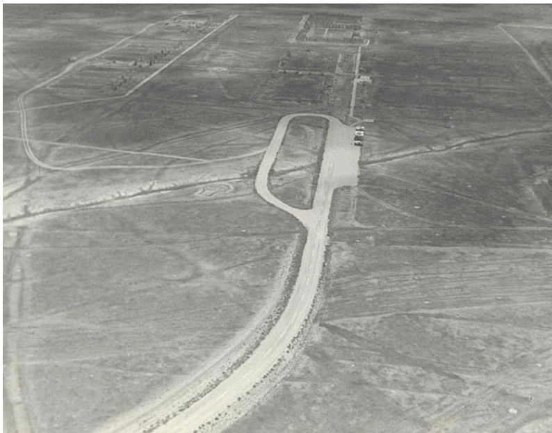
Aerial photo, circa 1954-57, showing parking area prior to visitor center construction, located directly south on the edge of the fort ruins. (Note location of major Santa Fe Trail rut). Source: Park photo files; taken from 2009 DOE.
