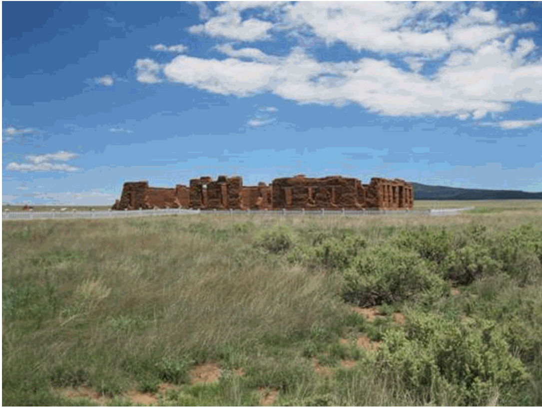
View from south of the Visitor Center to the Hospital ruins with grassy fields and mountains in the background, facing northeast, July 2010. Source: National Park Service.
