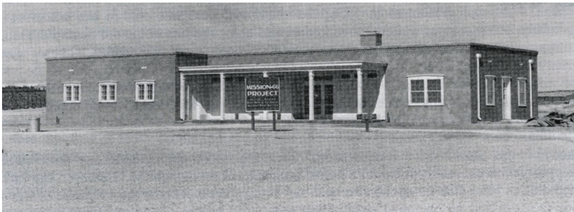
1959 photo of southern elevation. Source: Zhu 1992, 34; taken from 2009 DOE.
