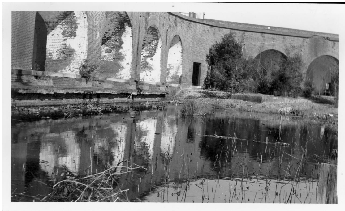
Figure 1. Flooded parade grounds of Fort Pulaski sometime during the CCC occupation (Box 82_397, Fort Pulaski National Monument Archives).
