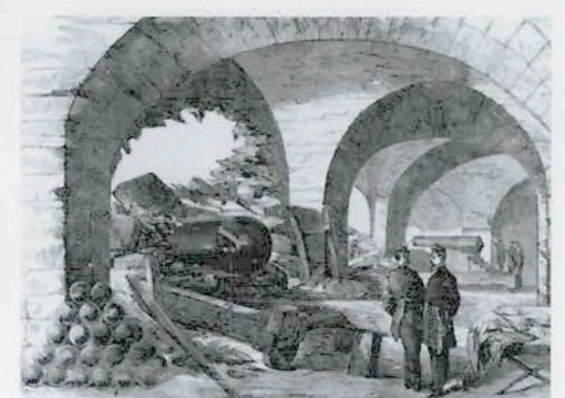
Interior view of Pulaski's southeast casemates showing the breach made by the Federal batteries
