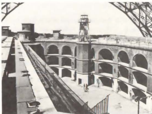
The handsome arched casemates with their intricate brickwork once housed the fort guns. There are thirty "gun rooms" on each floor.
