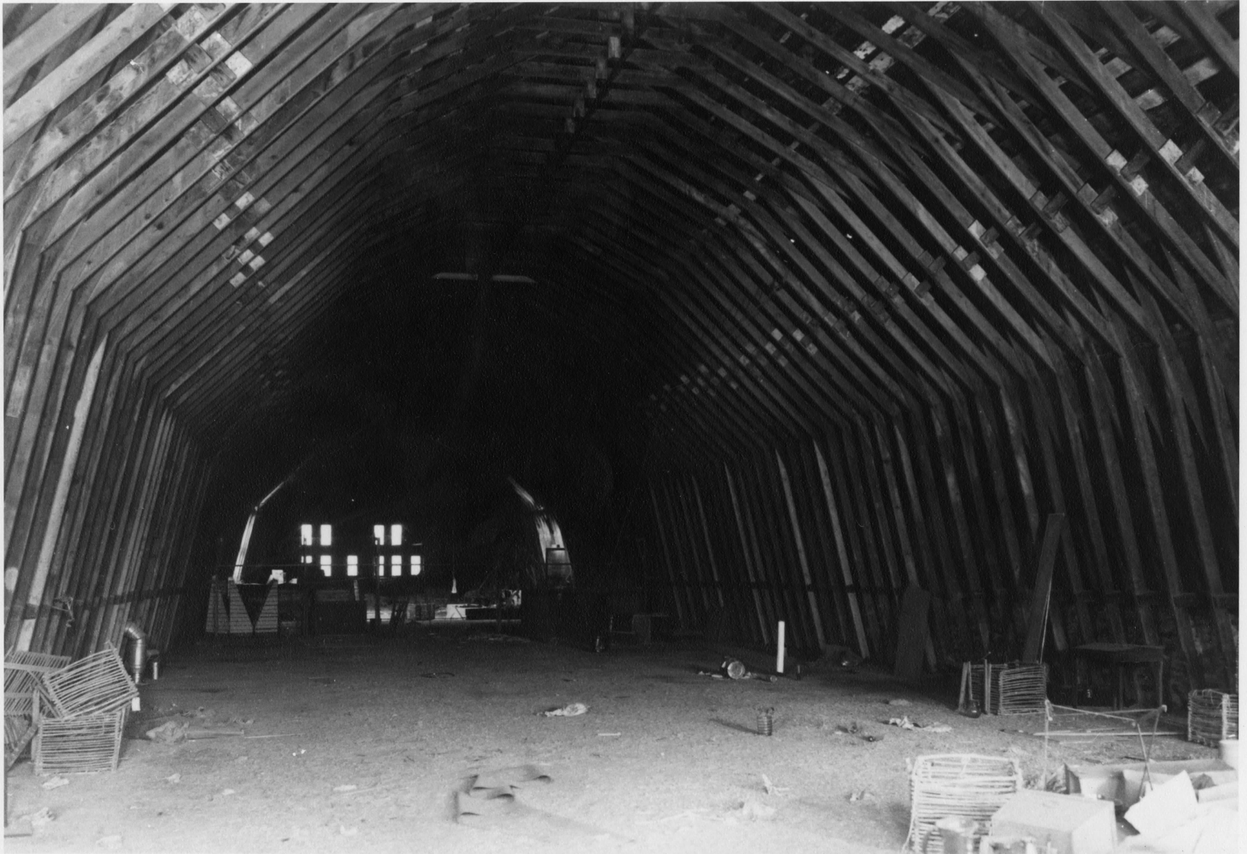
ILLUSTRATION NO. 6. Interior of Hay Loft to be removed.
