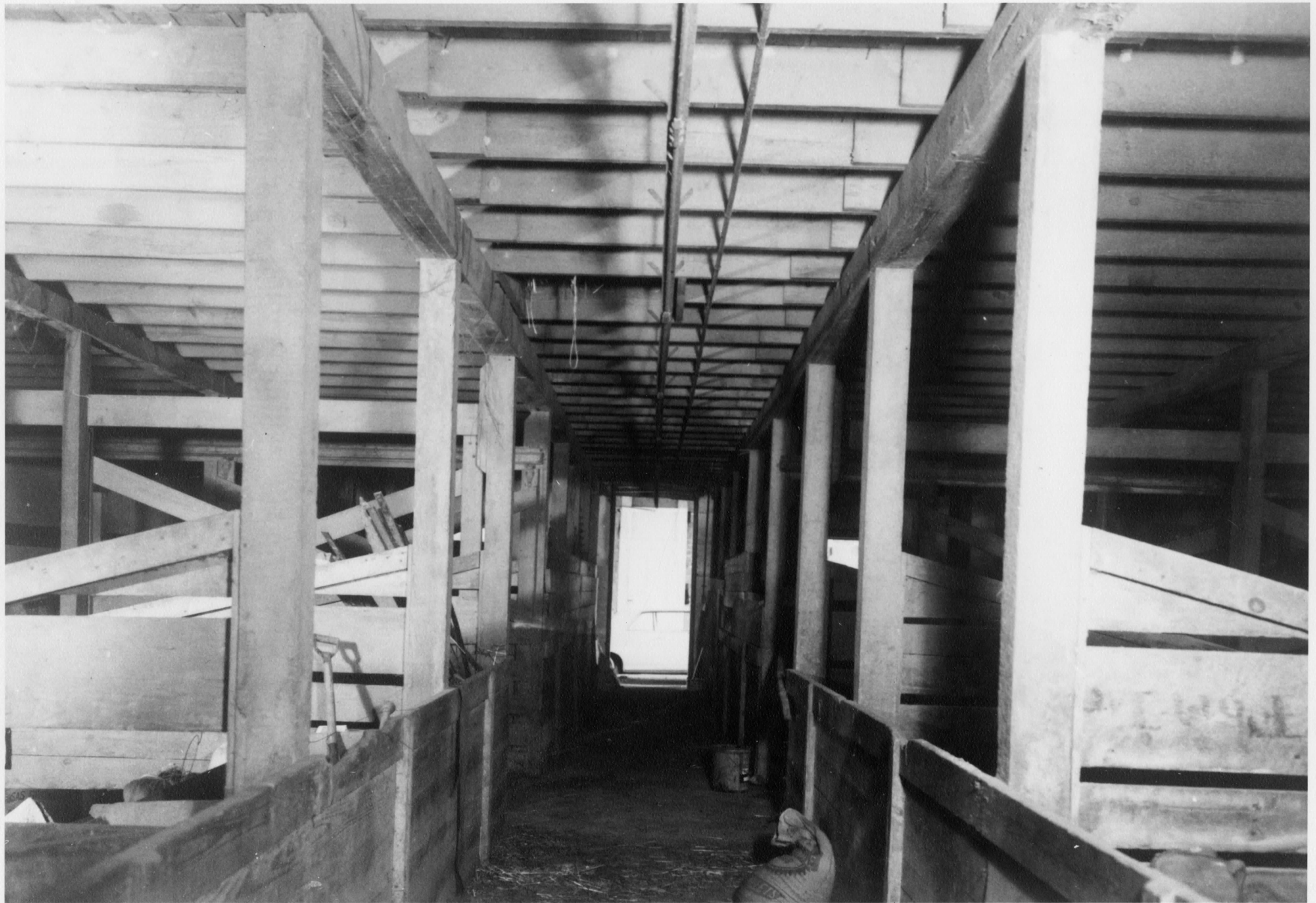
ILLUSTRATION NO. 7. Showing ceiling support, West End.
