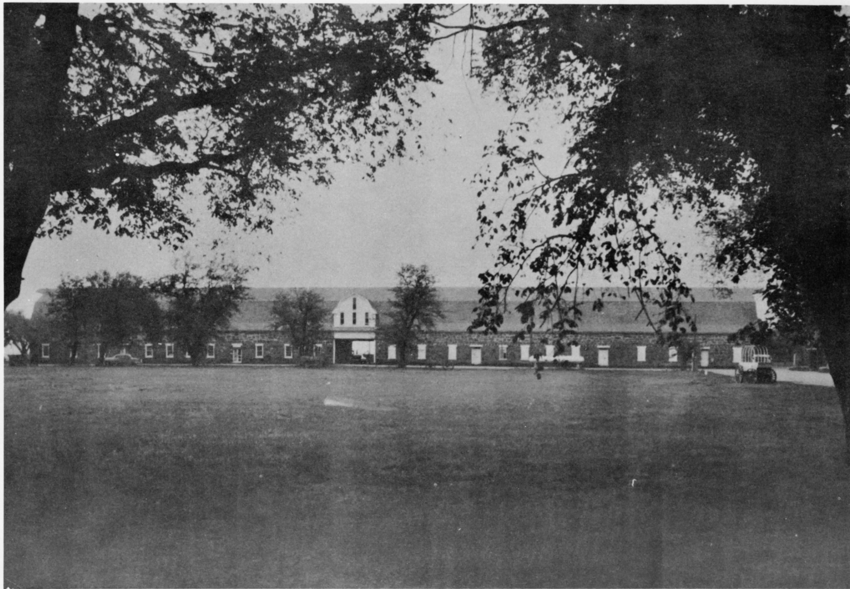
ILLUSTRATION NO. 4. Buildings No. 1 & 2, South Elevation, July 1965
