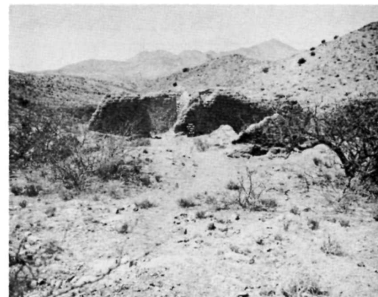
(C) HS 035 • EAST ELEVATION BEFORE 1967 STABILIZATION. SAME VIEW AS (B).
