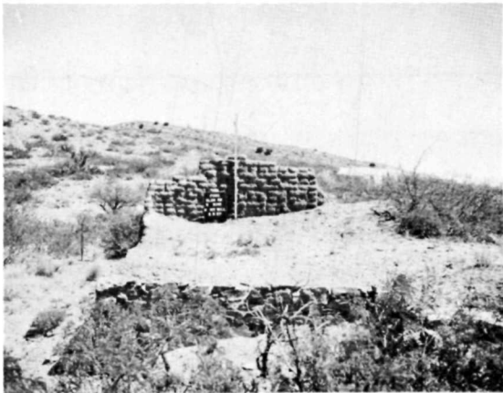
(A) HS 028 * SOUTH ELEVATION BEFORE 1967 STABILIZATION. SAME VIEW AS (P).
