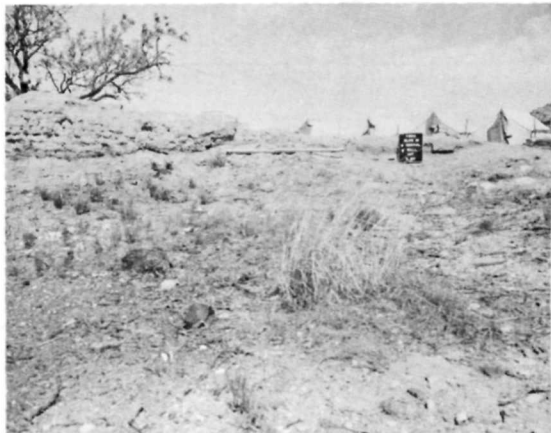
Ⓓ HS 010 • EAST ELEVATION BEFORE 1967 STABILIZATION SAME VIEW AS Ⓐ.
