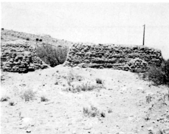
(D) HS 018 • SOUTH ELEVATION BEFORE 1967 STABILIZATION. SAME VIEW AS (P 55) (C)
