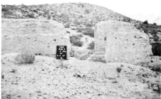
(D) HS 000 • WEST ELEVATION BEFORE 1967 STABILIZATION, SAME VIEW AS (E) 36 & (F) 36
