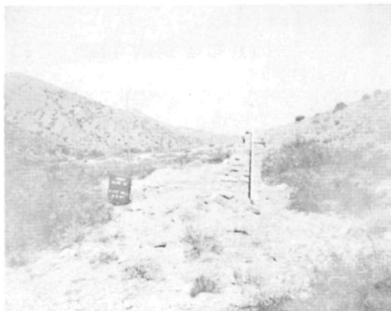
Ⓓ HS 037 • EAST ELEVATION BEFORE 1967 STABILIZATION, SAME VIEW AS Ⓒ.
