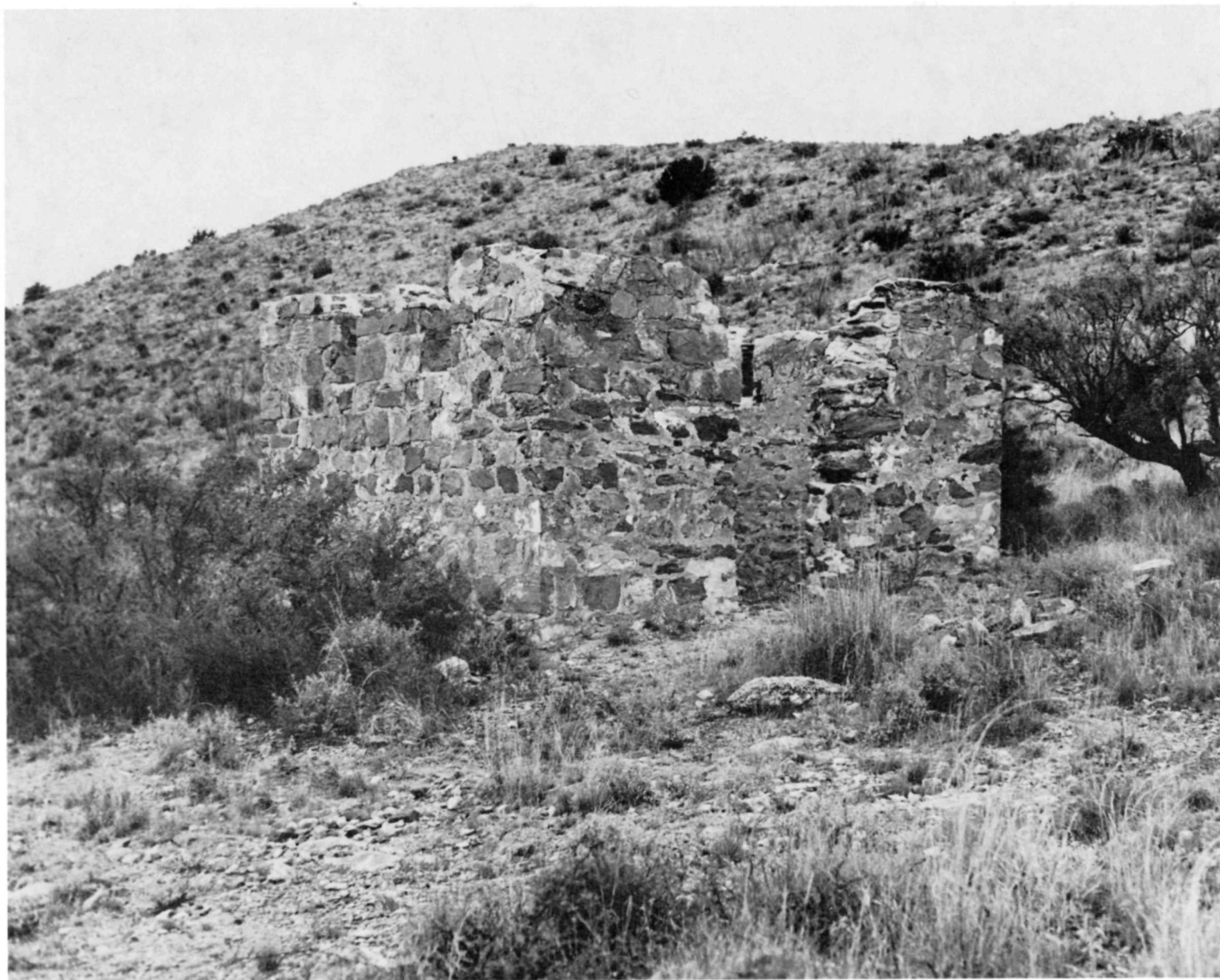
HS 036: View looking northwest.
