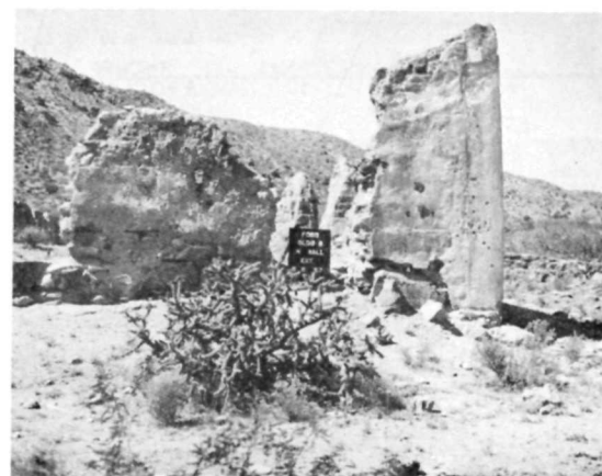
Ⓕ HS 008 • NORTH ELEVATION BEFORE 1967 STABILIZATION.
