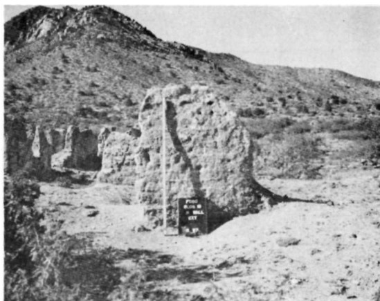
(A) HS 010 • WALL B • NORTH ELEVATION BEFORE 1967 STABILIZATION, SAME VIEW AS (B)
