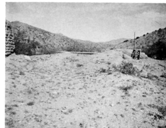
(C) HS 010 - EAST ELEVATION BEFORE 1977 STABILIZATION. SAME VIEW AS (B) & (D).
