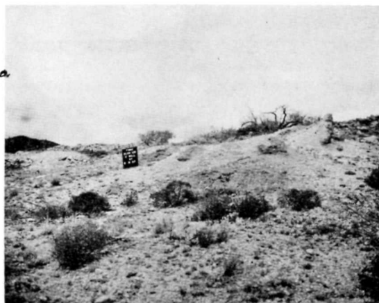
Ⓔ HS 106 • WALLS C & D • EAST ELEVATION BEFORE 1967 STABILIZATION.
