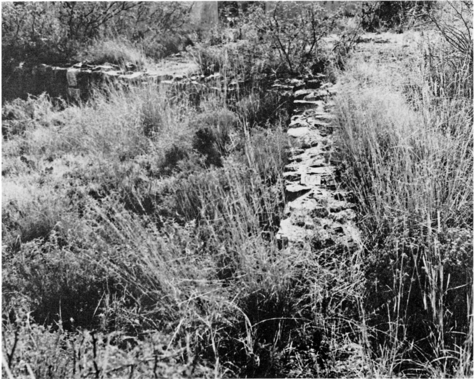
HS 064: View looking southeast.
