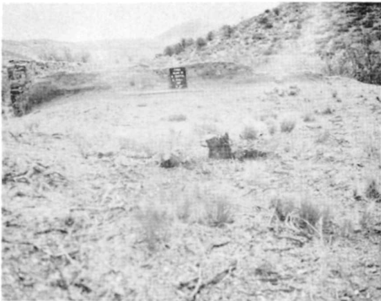
Ⓓ HS 010 • WEST ELEVATION BEFORE 1967 STABILIZATION. SAME VIEW AS Ⓒ.
