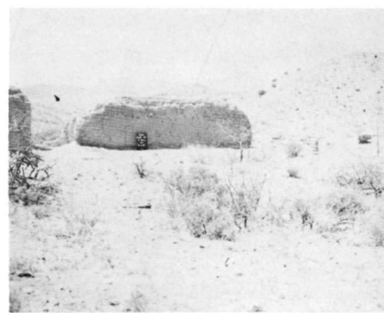
(F) HS 035 • EAST ELEVATION BEFORE 1967 STABILIZATION. SAME VIEW AS (B).
