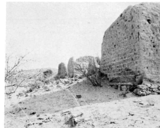
Ⓒ HS 035 • NORTH ELEVATION BEFORE 1967 STABILIZATION.
