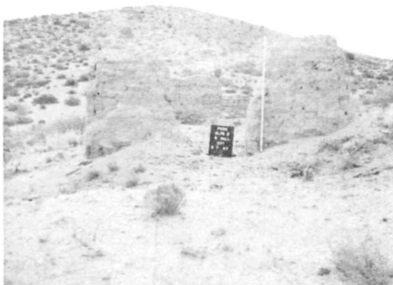
Ⓐ HS 004 & 005 • WEST ELEVATION BEFORE 1967 STABILIZATION.
