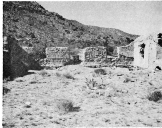
Ⓑ HS 008 • NORTH ELEVATION BEFORE 1967 STABILIZATION, SAME VIEW AS Ⓐ
