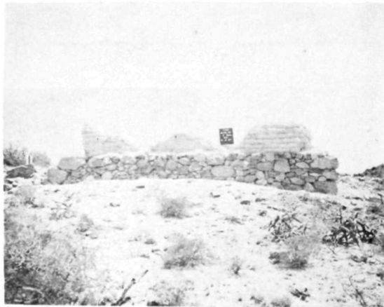
Ⓓ HS 101 • WEST ELEVATION BEFORE 1967 STABILIZATION, SAME VIEW AS Ⓐ & Ⓑ.
