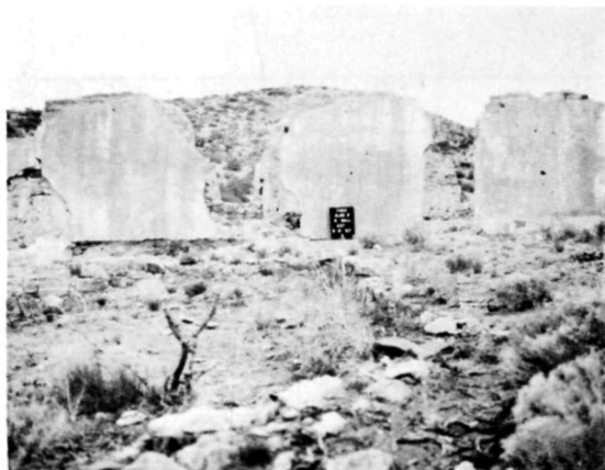
(A) HS 008 • WEST ELEVATION BEFORE 1967 STABILIZATION. SAME VIEW AS (A) (B) (C) (D)
