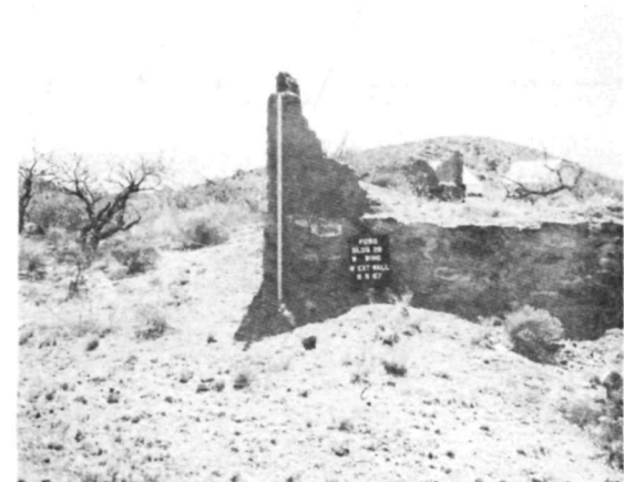
(F) HS 028 * WEST ELEVATION BEFORE 1967 STABILIZATION. SAME VIEW AS (E).
