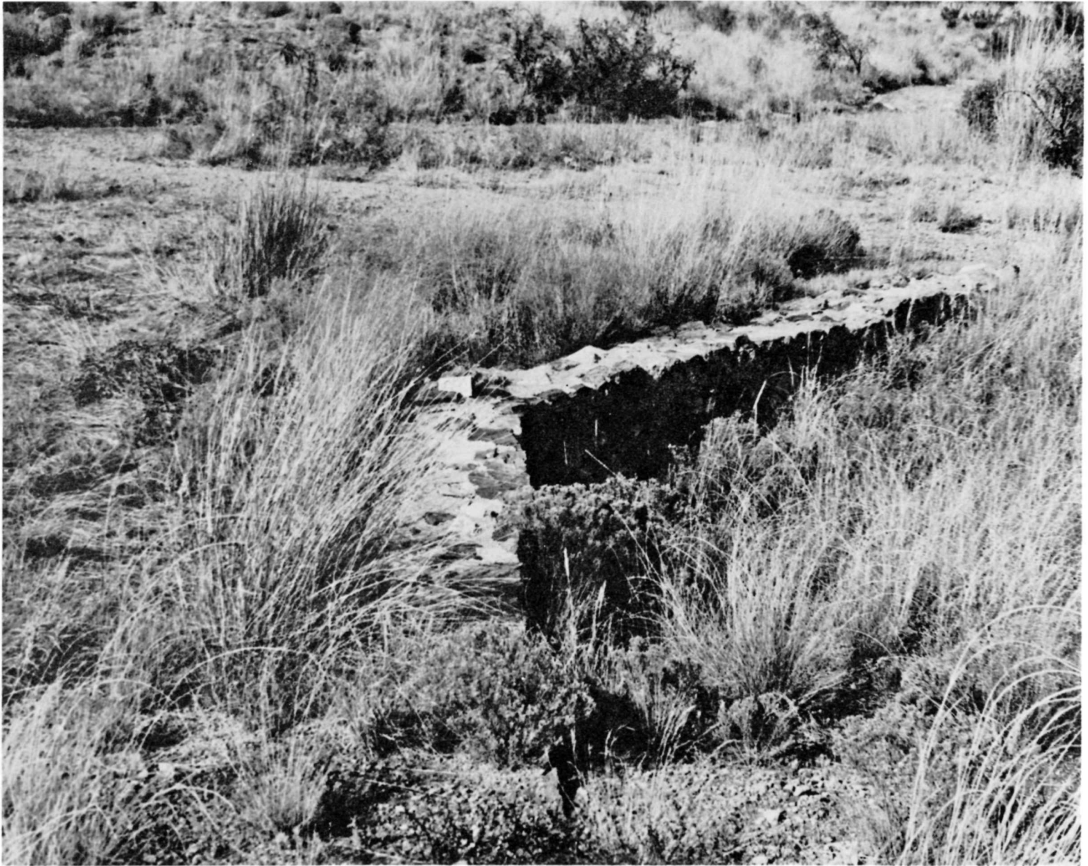
HS 060: View looking northwest.
