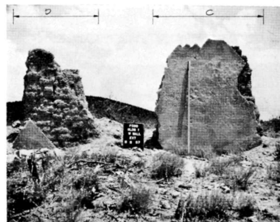
(C) HS 001 • WALLS D & C • WEST ELEVATION BEFORE 1967 STABILIZATION.
