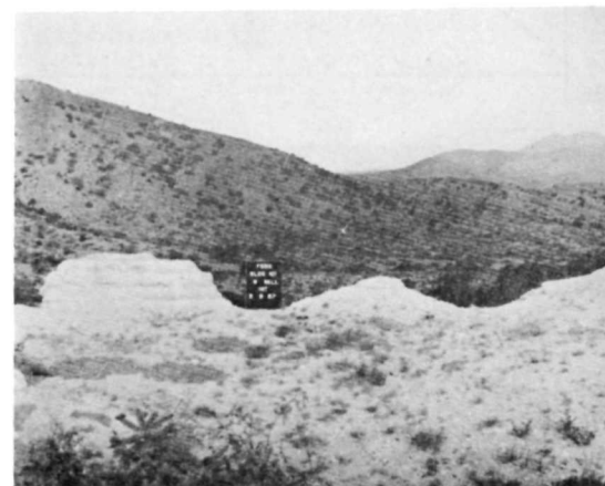
Ⓒ HS 101 • EAST ELEVATION BEFORE 1967 STABILIZATION. SAME VIEW AS Ⓐ
