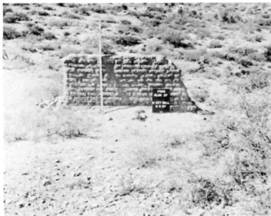
Ⓑ HS 037 • NORTH ELEVATION BEFORE 1967 STABILIZATION, SAME VIEW AS Ⓐ.
