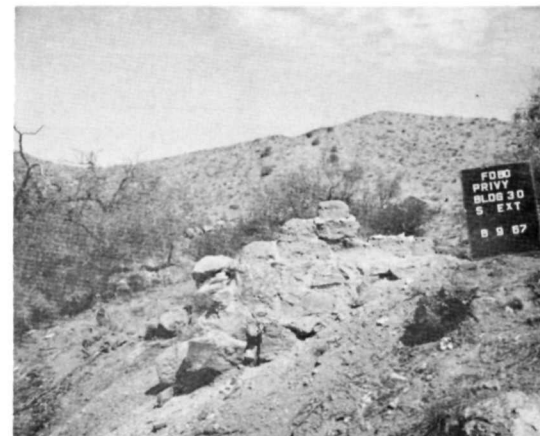
Ⓒ HS 030 • SOUTH ELEVATION BEFORE 1967 STABILIZATION.
