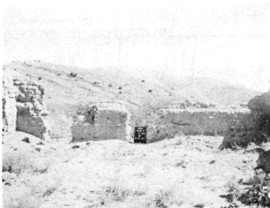
(A) HS 008 • SOUTH ELEVATION BEFORE 1967 STABILIZATION, SAME VIEW AS (B).
