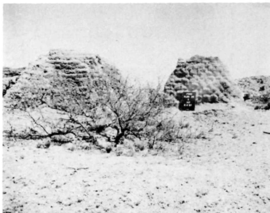
(B) HS 035 • WEST ELEVATION BEFORE 1967 STABILIZATION SAME VIEW AS (A)
