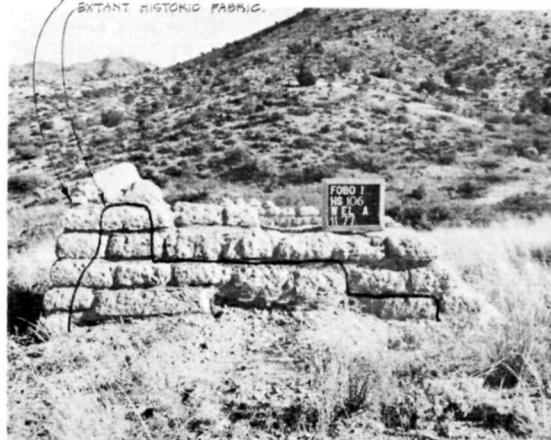
Ⓔ HS 106 • WALL A • WEST ELEVATION
