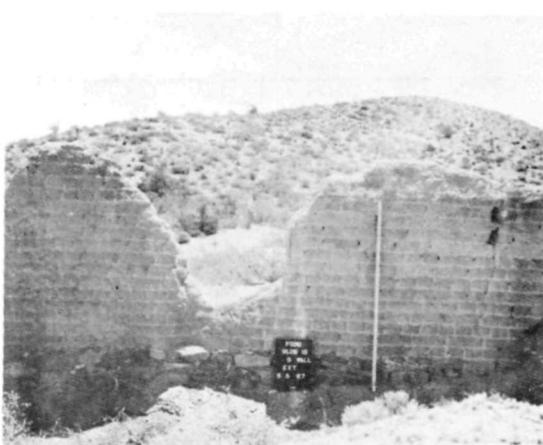
Ⓔ HS 010 • WALL A • WEST ELEVATION BEFORE 1967 STABILIZATION. SAME VIEW AS Ⓒ & Ⓓ
