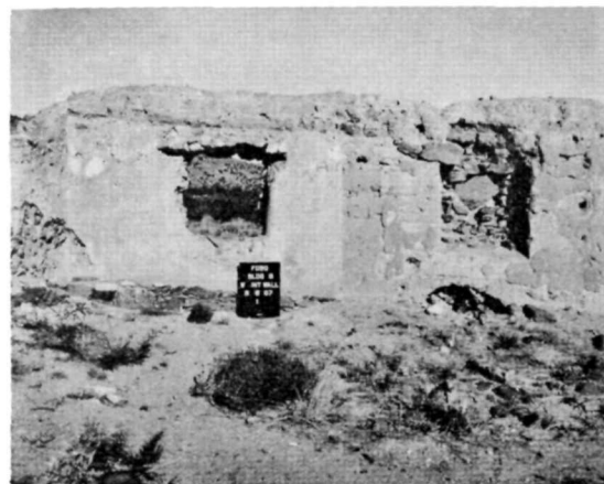
Ⓔ HS 008 • EAST ELEVATION BEFORE 1971 STABILIZATION. SAME VIEW AS Ⓓ.
