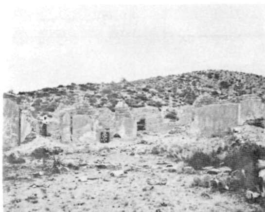
E HS 00B • WEST ELEVATION BEFORE 1967 STABILIZATION. SAME VIEW AS D , C & A .
