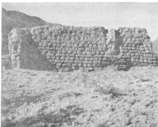
Ⓔ HS 01B • NORTH ELEVATION BEFORE 1967 STABILIZATION. SAME VIEW AS Ⓓ
