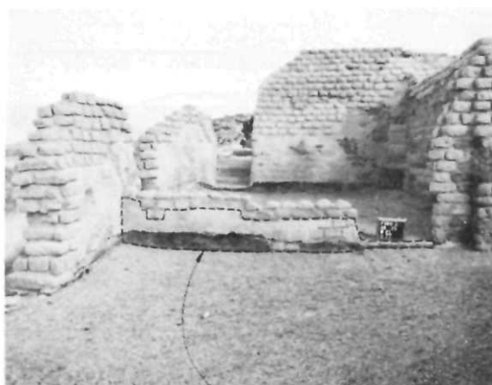
NON-HISTORIC SOIL CEMENT & CEMENT PLASTER REMOVED TO EXPOSE HISTORIC FABRIC, 1970.
