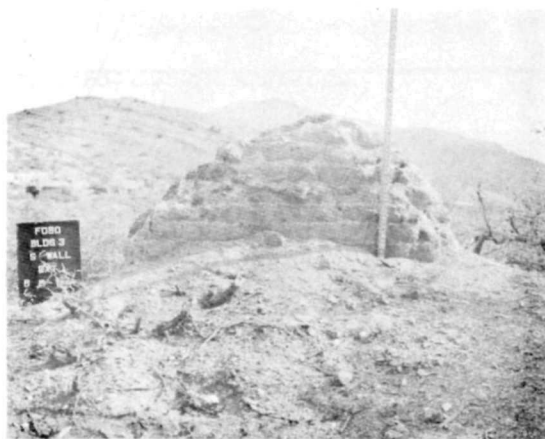
Ⓑ HS 003 • SOUTH ELEVATION BEFORE 1967 STABILIZATION
