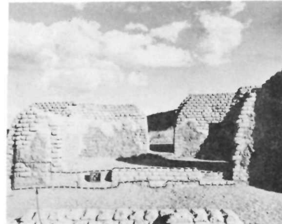
NON-HISTORIC SOIL CEMENT REMOVED & REPLACED WITH UNAMENDED ADOBE EXCEPT STAKES WHICH WERE REPLACED WITH NEW SOIL CEMENT ADOBE. Ⓕ HS 035 • WEST ELEVATION
