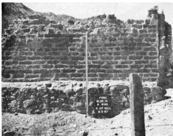
(A) HS 014 & 015 • WALL B • NORTH ELEVATION BEFORE 1967 STABILIZATION. SAME VIEW AS (B).
