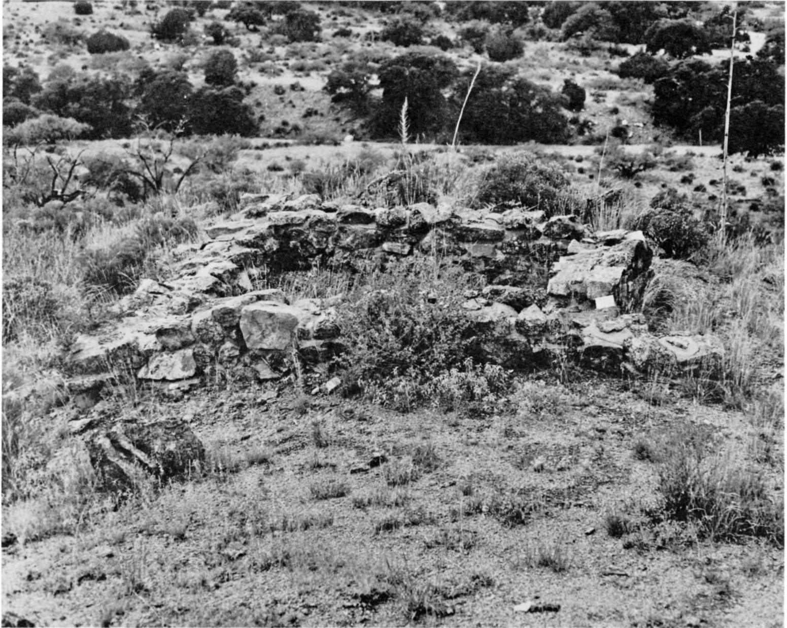
HS 102: View looking northwest
