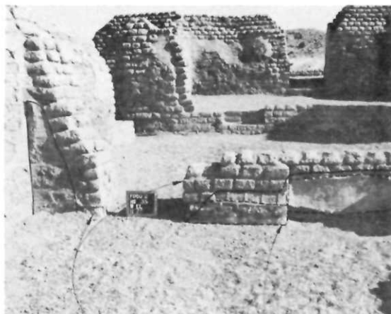
NON-HISTORIC SOIL CEMENT REMOVED TO EXPOSE HISTORIC FABRIC. NON-HISTORIC CEMENT PLASTER REMOVED, 1970.
