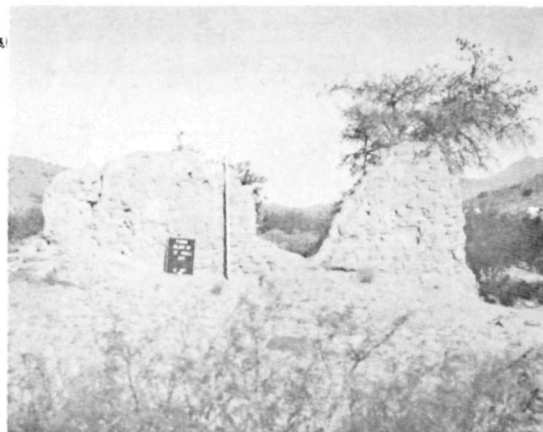
Ⓑ HS 010 • WALL A • EAST ELEVATION BEFORE 1967 STABILIZATION. SAME VIEW AS Ⓐ
