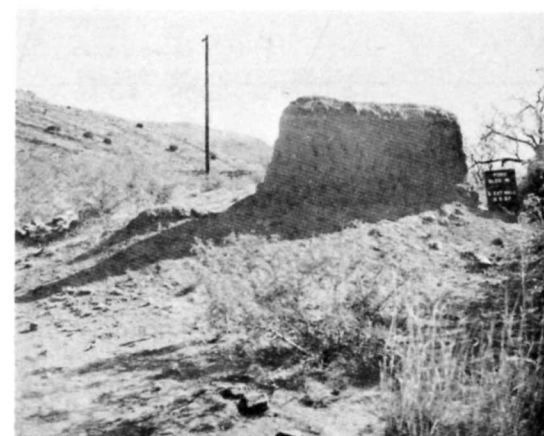
(F) HS 018 • SOUTH ELEVATION BEFORE 1967 STABILIZATION. SAME VIEW AS (B)
