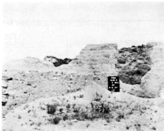
(B) HS 000 • WEST ELEVATION BEFORE 1967 STABILIZATION, SAME VIEW AS (C) 36
