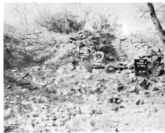
⑥ HS 043 • EAST ELEVATION BEFORE 1967 STABILIZATION.
