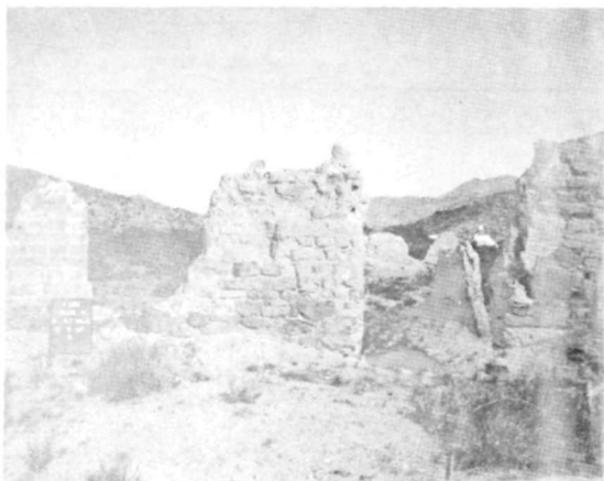
Ⓓ HS 008 • EAST ELEVATION BEFORE 1967 STABILIZATION. SAME VIEW AS Ⓒ & Ⓖ.
