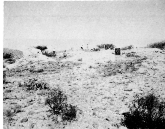
Ⓕ HS 106 • WALLS B & C • EAST ELEV. BEFORE 1967 STABILIZATION.
