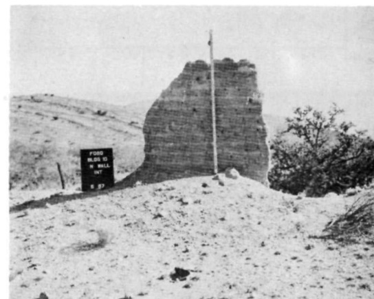
(C) HS 010 • WALL B • SOUTH ELEVATION BEFORE 1967 STABILIZATION, SAME VIEW AS (B)
