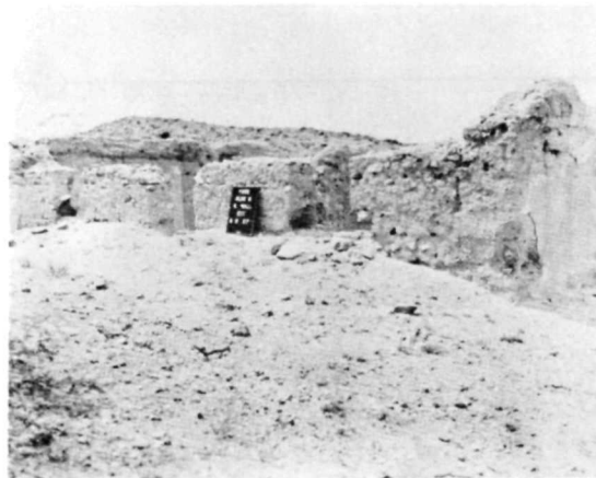
Ⓔ HS 008 • SOUTH ELEVATION BEFORE 1967 STABILIZATION,
