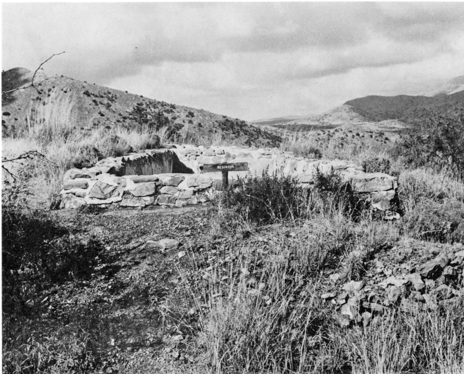
HS 069: View looking northwest.
