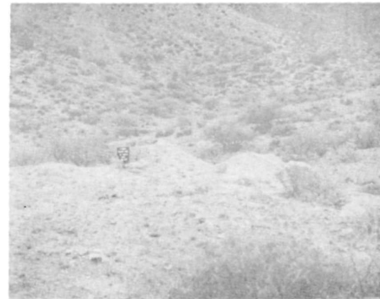
Ⓒ HS 106 • WALLS C & D • WEST ELEVATION BEFORE 1967 STABILIZATION.
