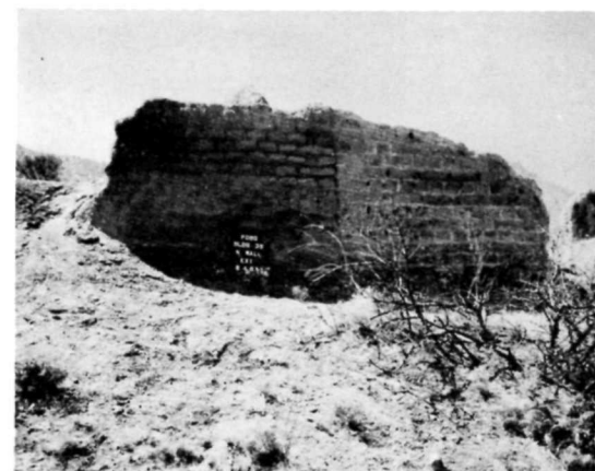
Ⓒ HS 035 • NORTH ELEVATION BEFORE 1967 STABILIZATION. SAME VIEW AS Ⓑ.
