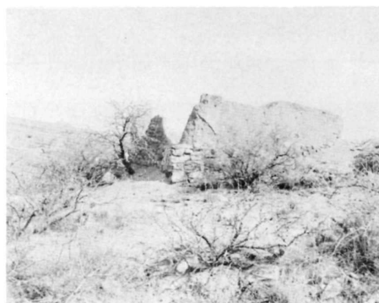
(C) HS 026 • SOUTH ELEVATION BEFORE 1967 STABILIZATION, SAME VIEW AS (A).
