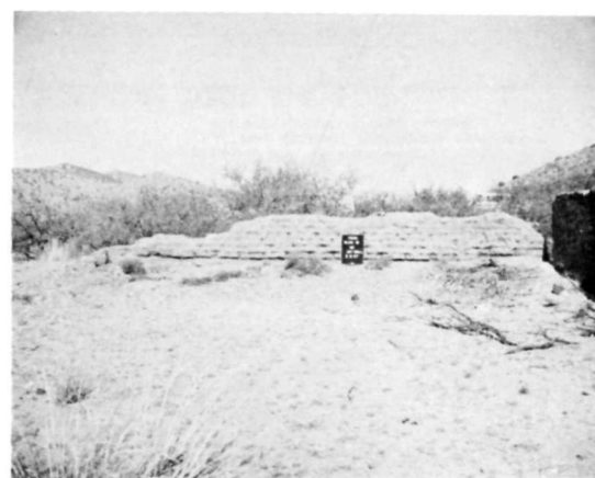
(F) HS 01B • EAST ELEVATION BEFORE 1967 STABILIZATION. SAME VIEW AS (E)
