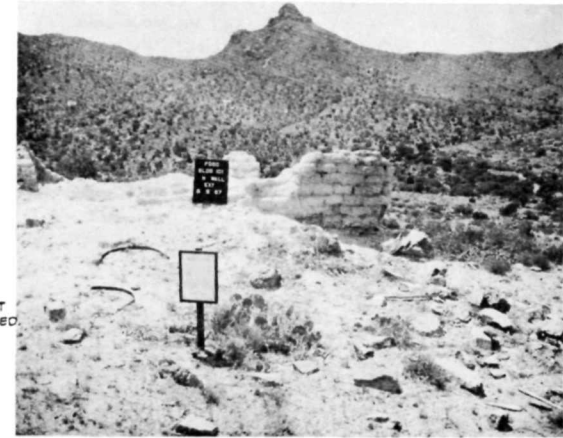
Ⓕ HS 101 • NORTH ELEVATION BEFORE 1967 STABILIZATION, SAME VIEW AS Ⓐ.
