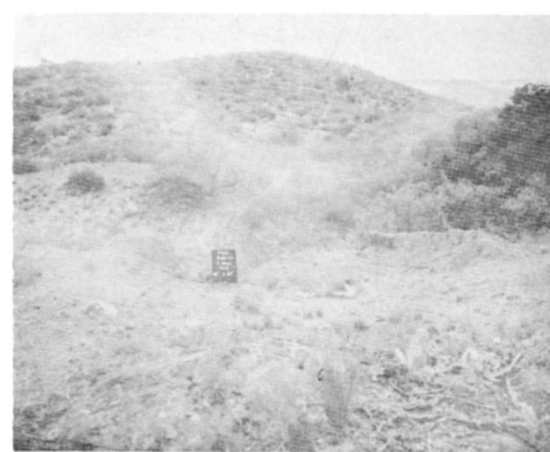
(F) HS 021 • WEST ELEVATION BEFORE 1967 STABILIZATION
