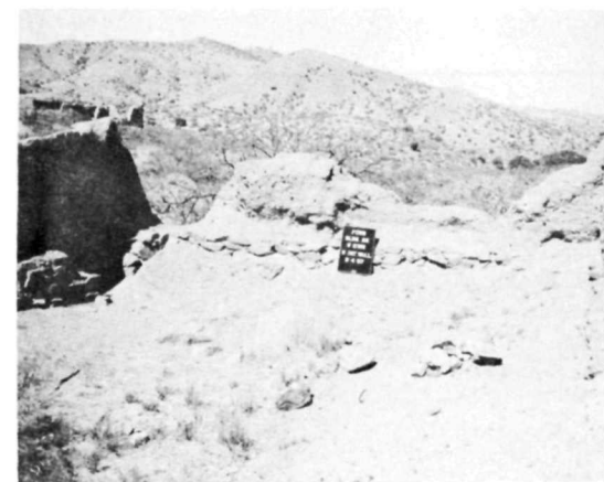
Ⓕ HS 026 • EAST ELEVATION BEFORE 1967 STABILIZATION, SAME VIEW AS Ⓔ.
