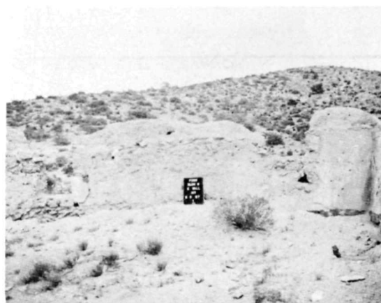
Ⓑ HS 008 • WEST ELEVATION BEFORE 1967 STABILIZATION. SAME VIEW AS Ⓓ & Ⓔ.
