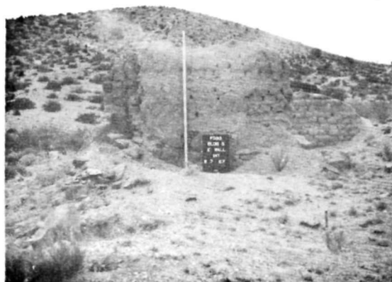
Ⓓ HS 004 & 005 • WEST ELEVATION BEFORE 1967 STABILIZATION. SAME VIEW AS Ⓒ.
