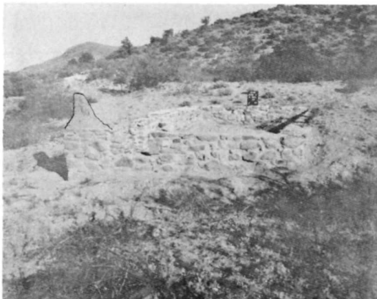
Ⓒ HS 011 • WEST ELEVATION AFTER 1967 STABILIZATION (ADOBES PORTION UNTOUCHED.)
