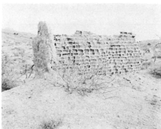
(E) HS 014 & 015 • WALL B • SOUTH ELEVATION BEFORE 1967 STABILIZATION. SAME VIEW AS (F).
