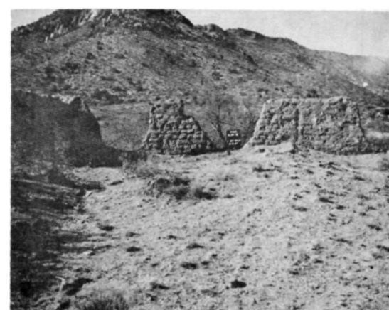
Ⓒ HS 01B • NORTH ELEVATION BEFORE 1967 STABILIZATION. SAME VIEW AS Ⓐ & Ⓑ.
