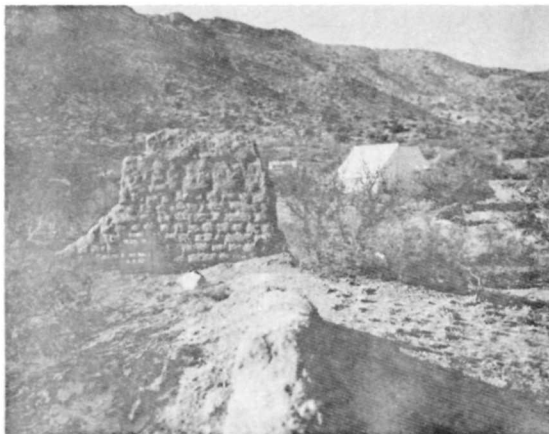
(A) HS 018 • NORTH ELEVATION BEFORE 1967 STABILIZATION. SAME VIEW AS (P 55)
