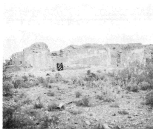
Ⓑ HS 008 • EAST ELEVATION BEFORE 1967 STABILIZATION. SAME VIEW AS Ⓒ Ⓓ Ⓔ
