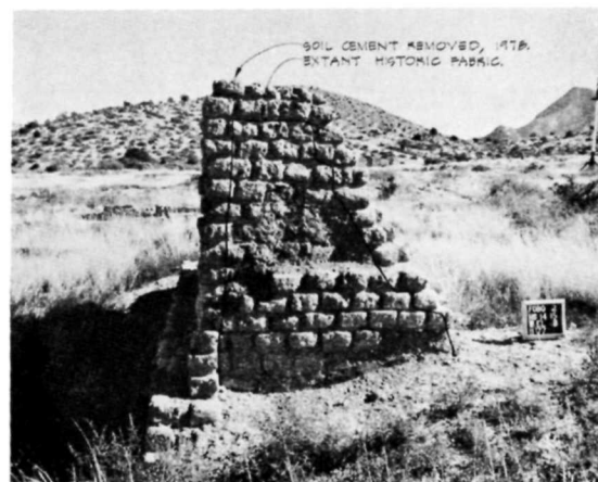
(F) HS 014 & 015 • WALL B • WEST ELEVATION
