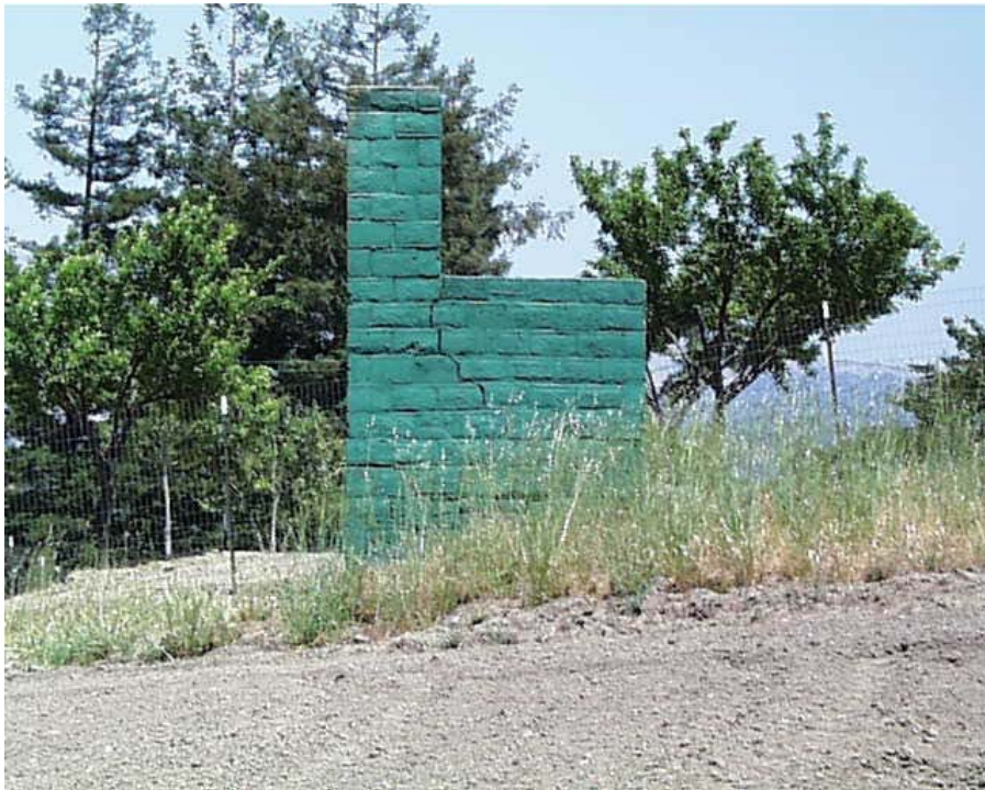
Photograph of the incinerator (PWR, Seattle 2003).
