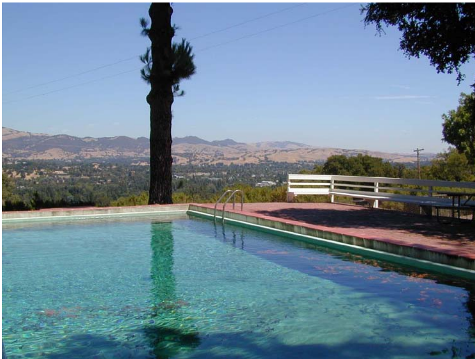
Photograph of the swimming pool. The pool is a contributing structure (PWR, Seattle 2003).
