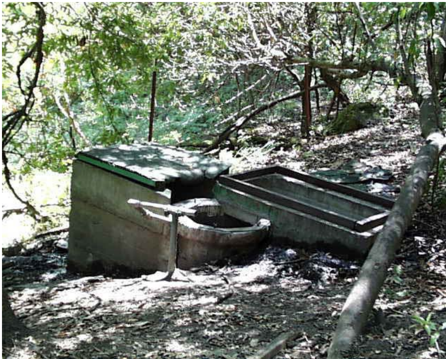
Photograph showing the water catchment system located at the naturally occurring spring west and uphill of the the Tao House (PWR, Seattle 2003).
