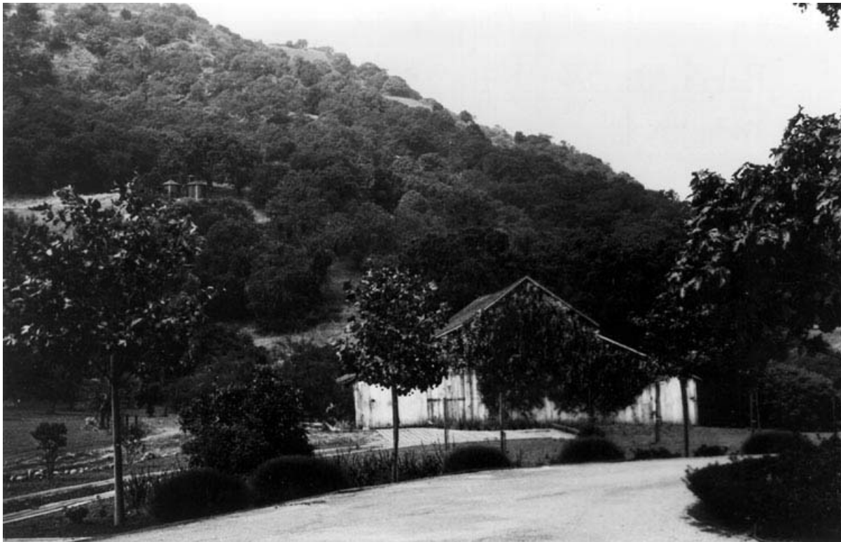
Photograph of the old barn taken from the turnaround, circa 1942 (EUON 1391 N).
