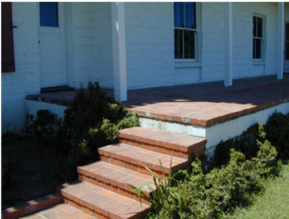
Photograph of the east terrace and the historic privet hedge, to the left and right of the staircase, which has been grazed by deer (PWR, Seattle 2003).
