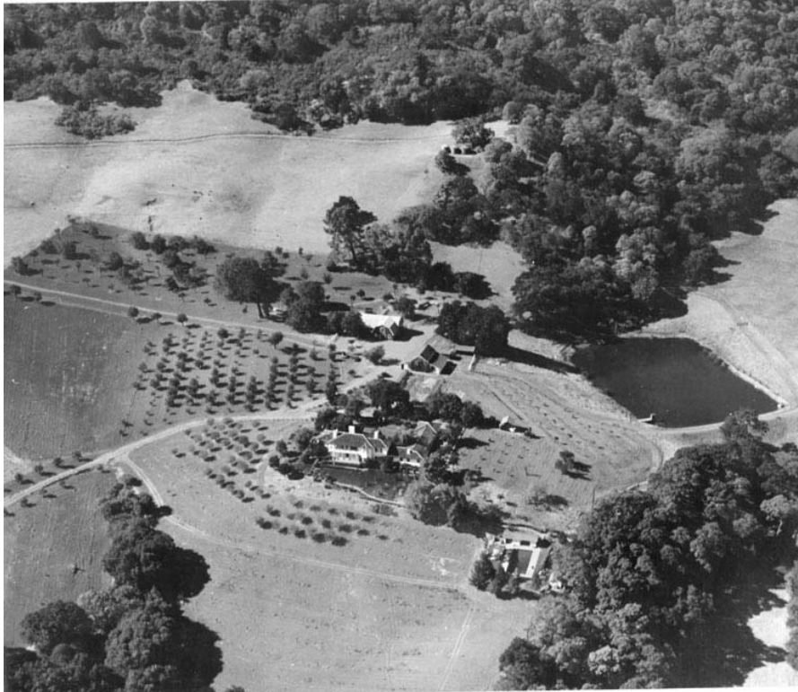
Oblique photograph, circa 1950, showing the Tao House, related outbuildings, and orchards approximately six years after the historic period (EUON collection).
