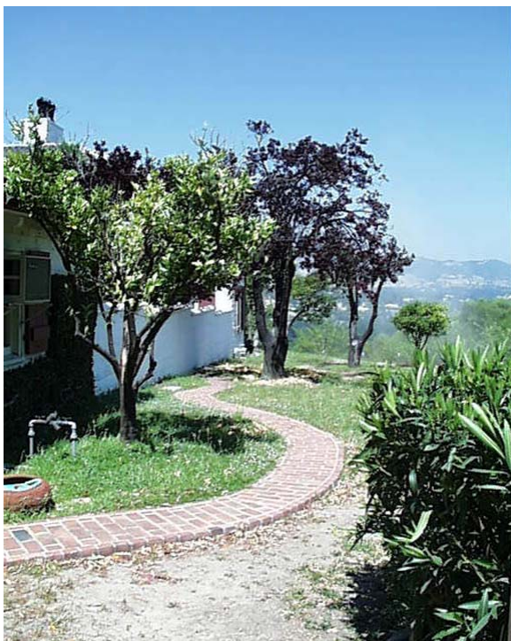
Photograph showing a typical curvilinear brick walkway, laid in a running bond pattern, on the south side of the Tao House (PWR, Seattle 2003).
