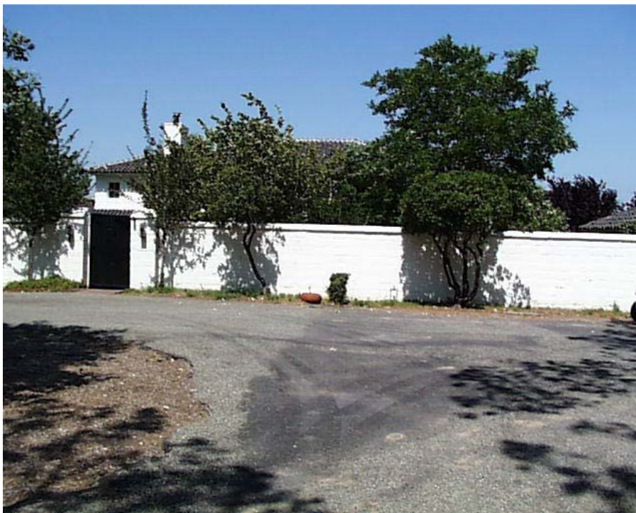
Photograph of the potting shed. It is undetermined how this building was used during the historic period (PWR, Seattle 2003).
