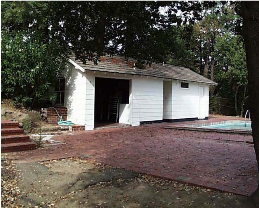
Contemporary photograph of the change house. This building was altered after the historic period when the Carlsons built an addition on the south side of the building (PWR, Seattle 2003).
