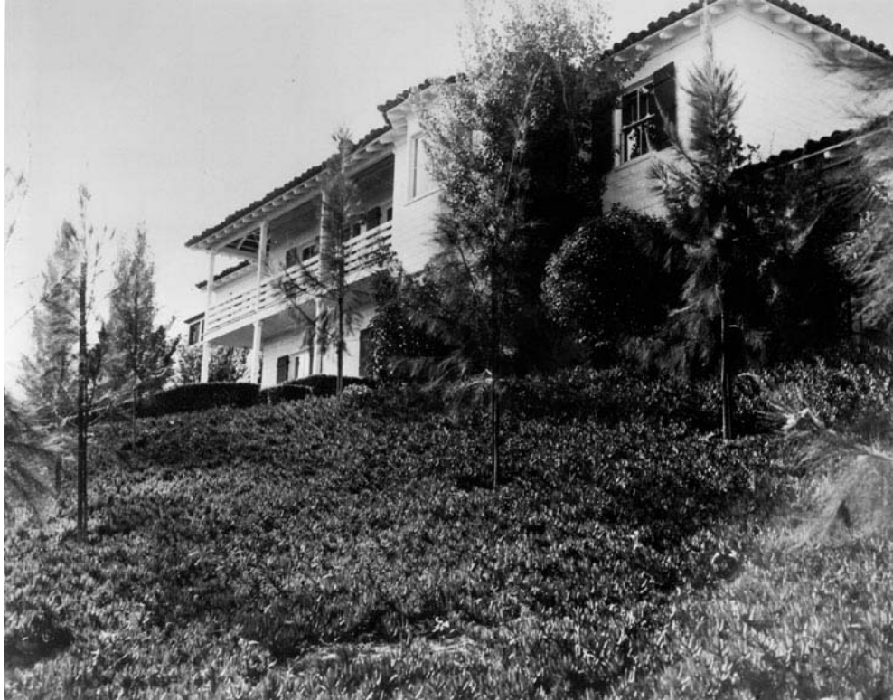
Photograph showing the east side of the Tao House, circa 1942 (EUON collection).
