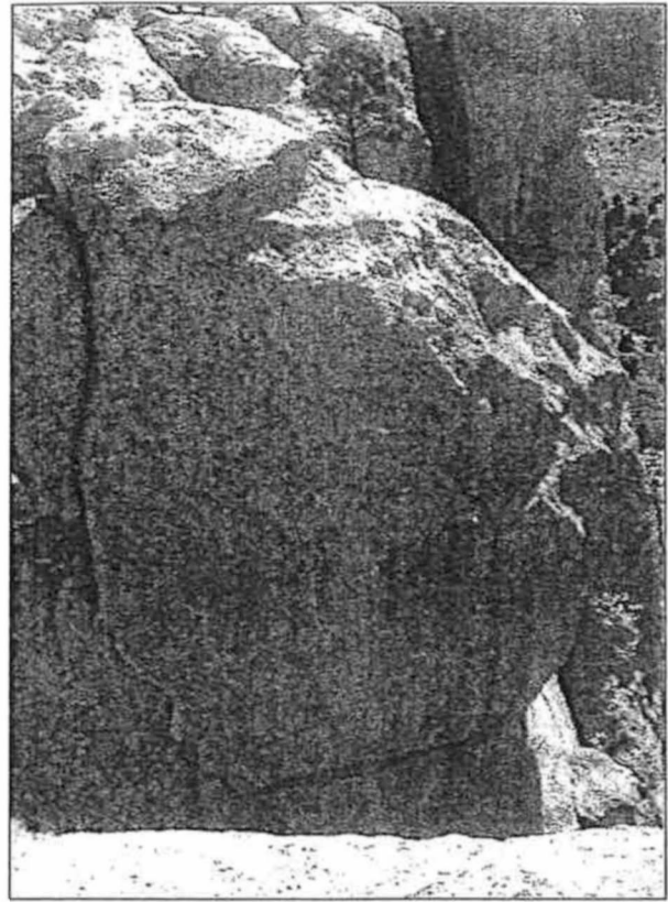
Figure 17. Section of overhanging mesa rim above pool area. Center of gravity of rock mass is well behind cliff face, indicating that topping failure is unlikely. Joint behind large section of rock shows no indication of recent movement.
