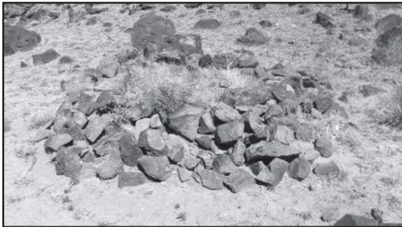
Coursed basalt stone foundation.
