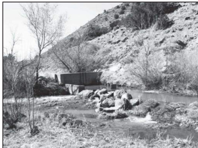
La Presa—main diversion structure from the Santa Fe River.
