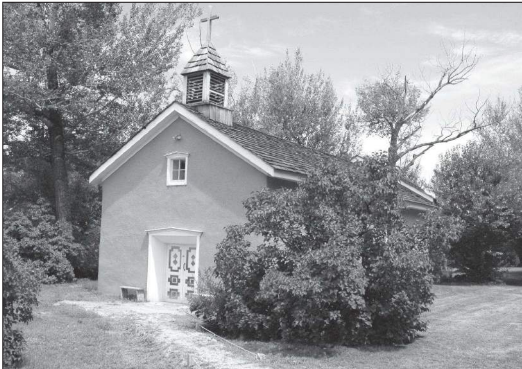
Los Luceros Chapel, "La Capilla de la Familia Santa," west façade. The hand-carved doors by master woodcarver Gregorio Ortega from Truchas, c. 1870, are from a demolished house in Peñasco.
