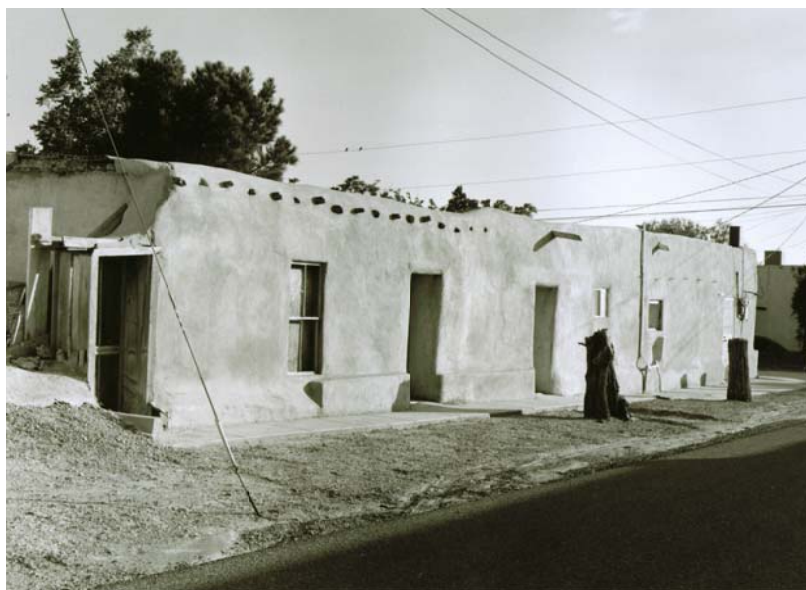
A rough-hewn adobe-based home in Doña Ana with irregularly sized windows and contours
