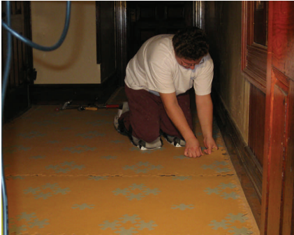
Installing Glenmont floor tile piece by piece.
