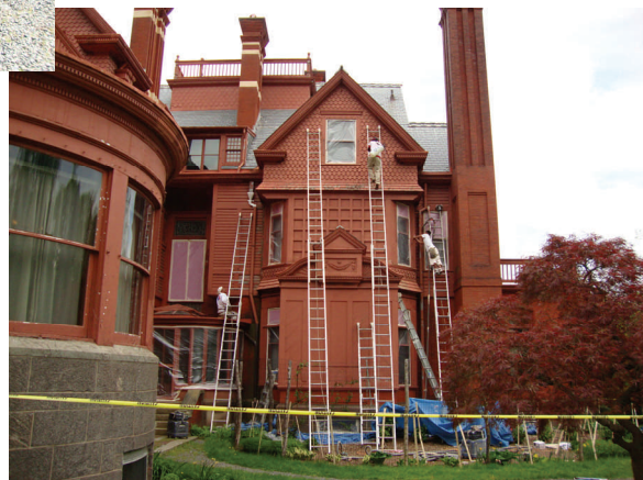
Workers start scraping and sanding the house exterior for the Glenmont painting project.
