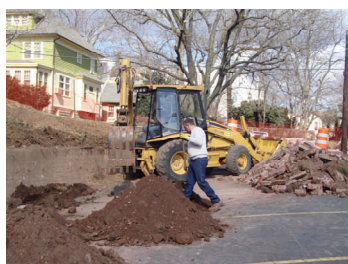
Work begins on the retaining wall.
