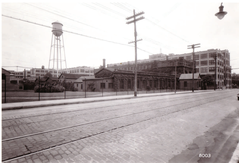
Historic view of Main Street, Edison Laboratories, 1939. The Black Maria, visible in the modern view above, now sits where the test circles are located in the left foreground.
