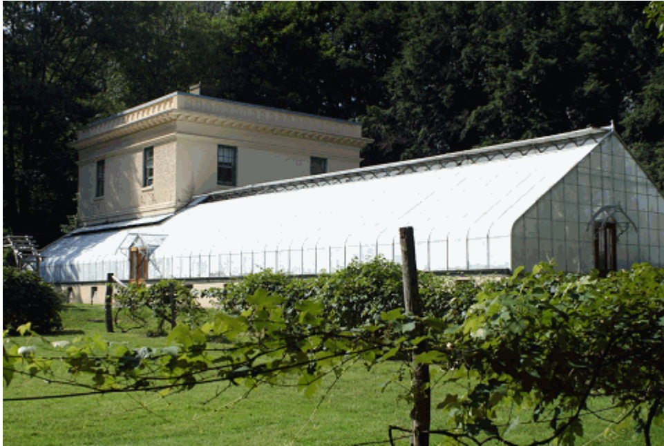
Figure 21. View looking north towards the gardener's cottage, potting shed, and greenhouse. The cottage and shed, built in c.1908, is one of the earliest examples of monolithic concrete construction developed by Thomas Edison (OCLP, 2009).
