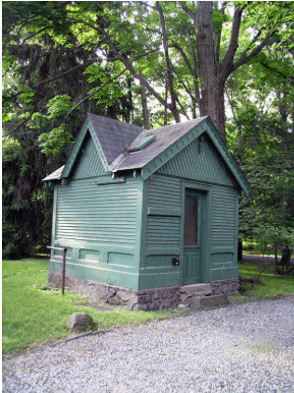
Figure 24. Similar in Victorian architectural design and construction as the house, the pump house built between 1882 and 1884, is a small wooden structure with a cross gable roof set on a fieldstone and mortar foundation (OCLP, 2009).
