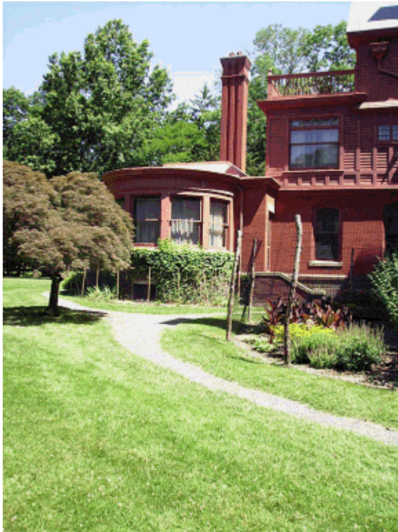
Figure 17. View looking north showing a pedestrian path. Pedestrian circulation within the grounds is limited to a small gravel path around the perimeter of the Glenmont house (OCLP, 2009).
