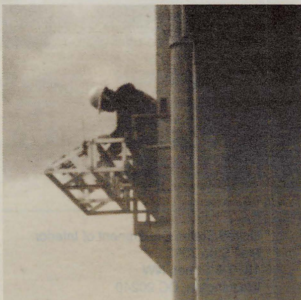
Bernie Covino installs a rack of coated samples on a coastal bridge in Oregon.
