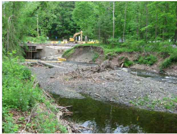
Figure 26. Photograph of repairs to U.S. 209 bridge over Raymondskill Creek. River channel migration and flooding are natural processes that impact infrastructure along or crossing the rivers. Note eroded and slumped banks along the creek. National Park Service photograph courtesy Leslie Morlock (Delaware Water Gap NRA).
