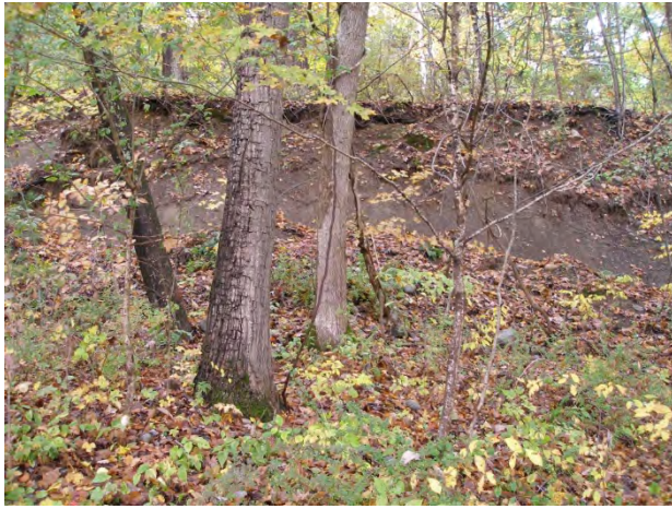
Figure 24. Photograph of slump along U.S. 209. Near mile marker 15, portions of the road collapsed in October 2011 as the slope was undercut by the Delaware River. National Park Service photograph courtesy Leslie Morlock (Delaware Water Gap NRA).
