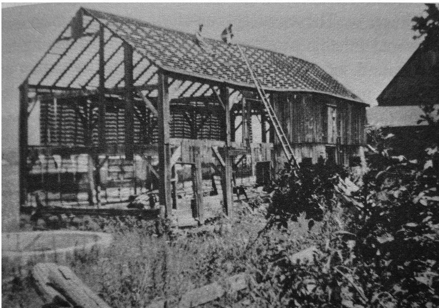
Figure 12. Dismantling the cow barn that stood beside the Van Campen-Dewitt Barn (background image right) in July 1939, when Nat and Hilda Ludwig were tenant farmers residing at the Van Campen Inn. (Hutson 1992: 95)
