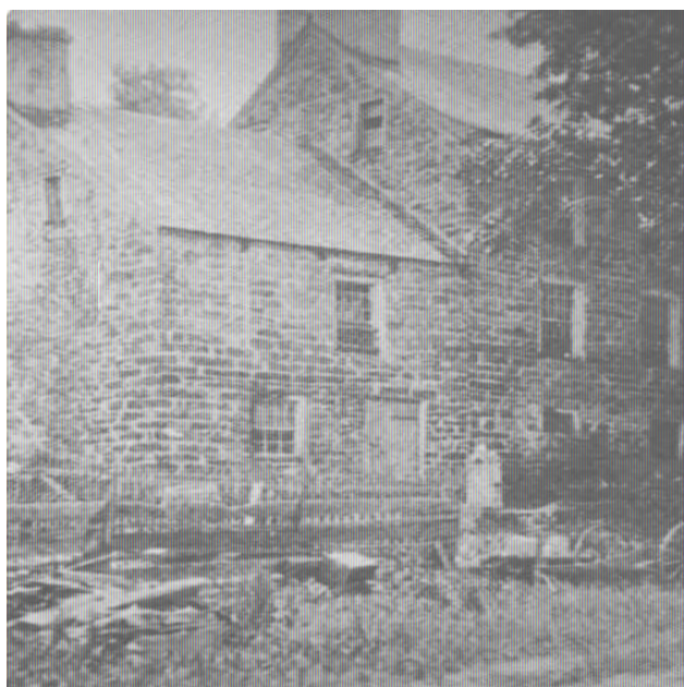
Figure 4. A 1903 photograph, taken by C.G. Hine, shows a portion of the northwestern (front) facade of the Van Campen Inn, looking southeast. (Snook 1974: 47)
