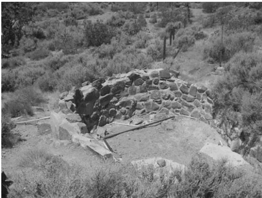
Buildings and Structures 7. The swimming pool is constructed with stone set in mortar and resembles the main residence in character (PWR 2005).
