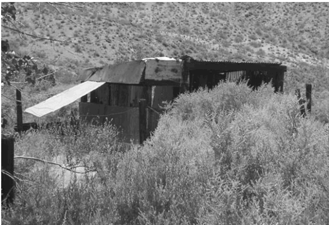
Buildings and Structures 6. The storage shed, located on the southwest corner of the property (PWR 2005).
