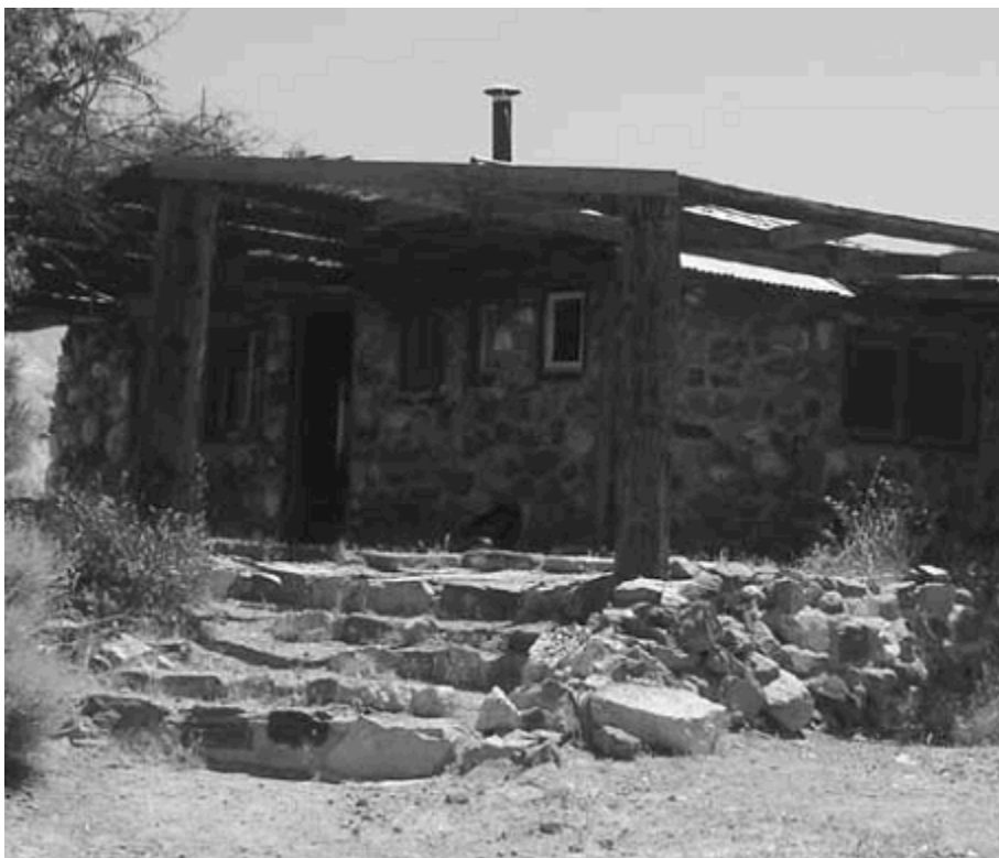
Circulation 2. Image showing the stone stairway near the front door of the main entrance. The stones are set in mortar (PWR 2005).
