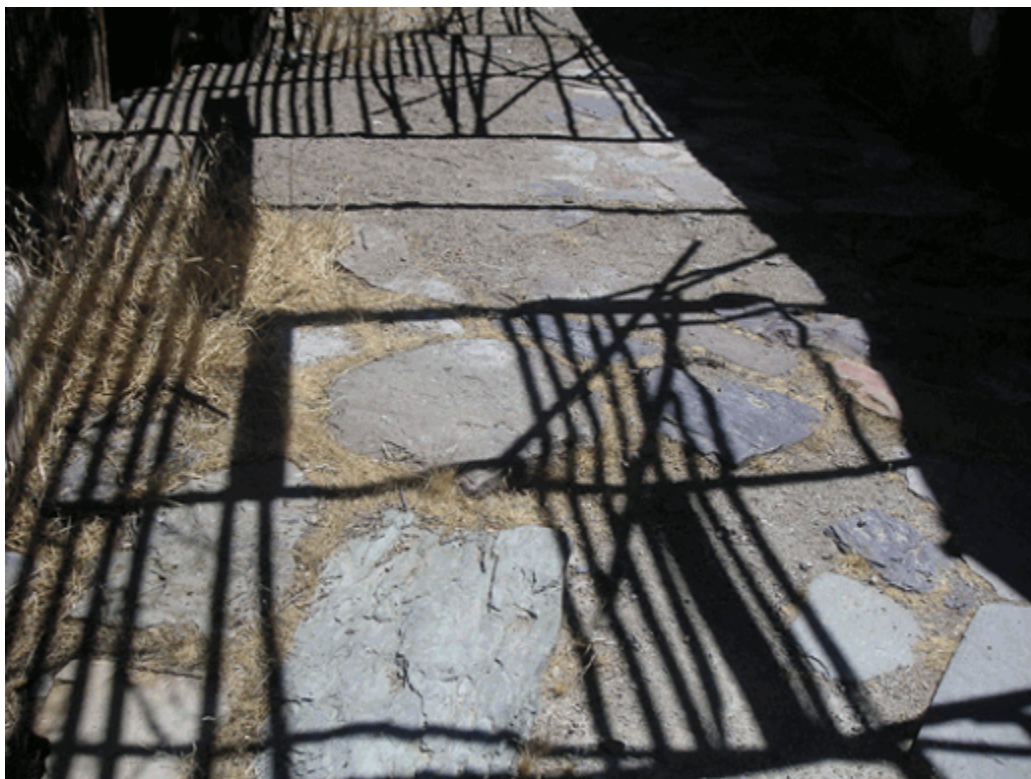
Circulation 3. The stone patio is located between the main residence and workshop. The large stones are set in earth and complement the masonry at the main residence (PWR 2005).
