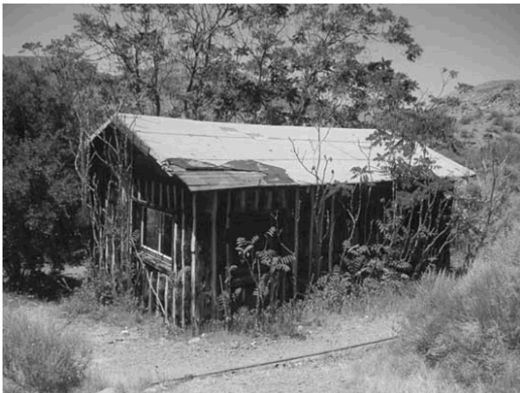
Buildings and Structures 4. Image of the east and north elevations of the bunkhouse. The architecture represents a departure in the use of materials. Instead of stone, this structure is constructed with vertical siding with chinking (PWR 2005).
