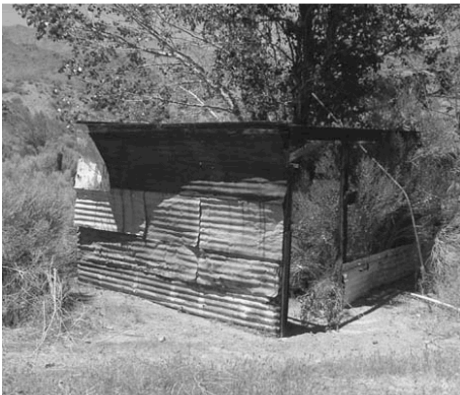
Buildings and Structures 5. The chicken coop is constructed with an eclectic mix of materials including corrugated metal, dimensional lumber, and chicken wire. View south and east elevations. (PWR 2005).
