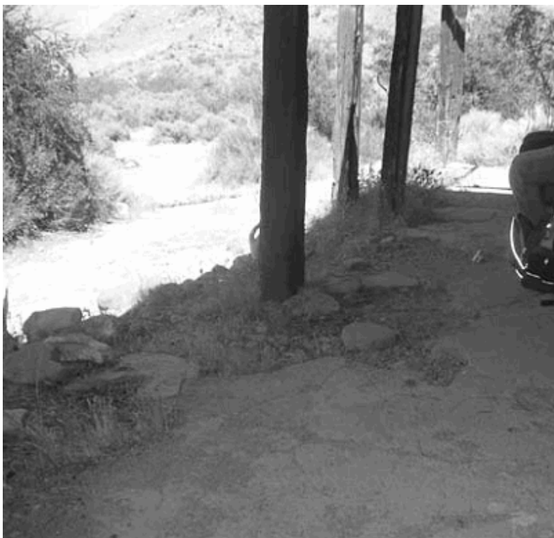
Circulation 4. The concrete surface of the front porch is located on the south elevation of the main residence (PWR 2005).
