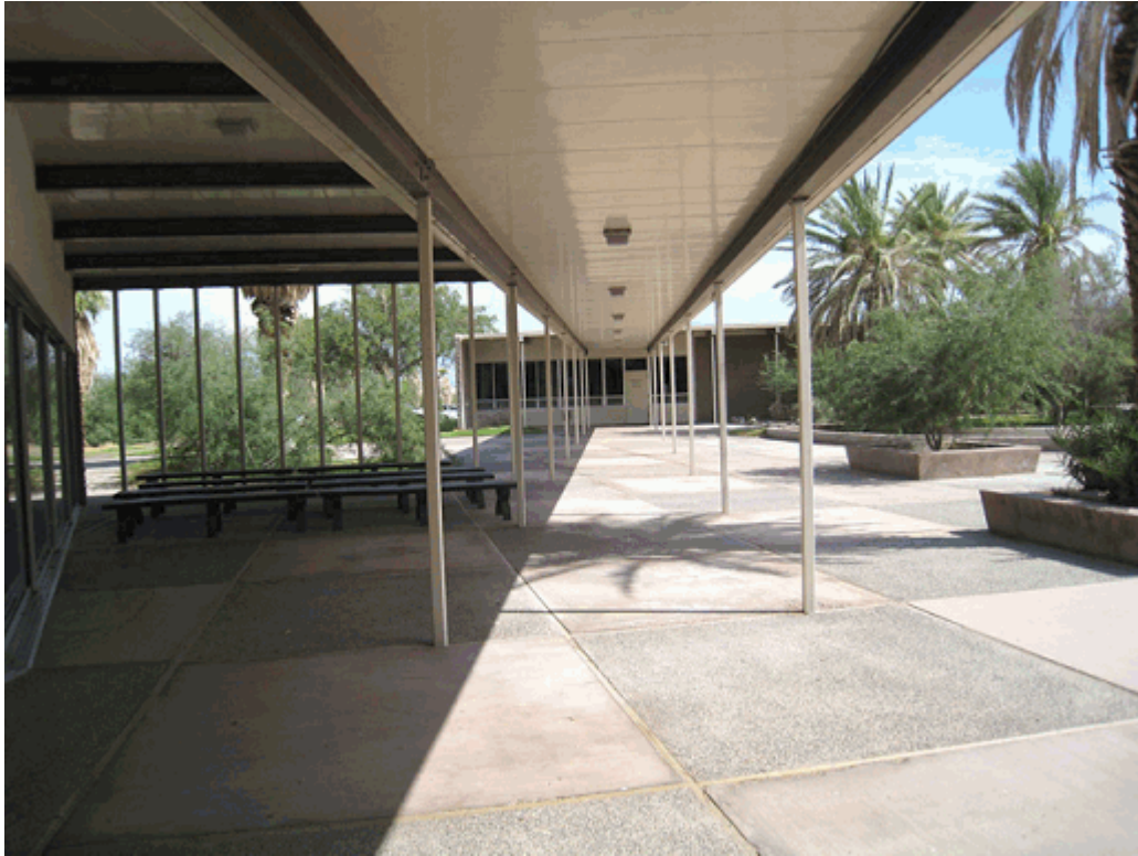
Photograph of the colonnade from the lobby to the administration Building south entrance, looking north. (PWRO 2009)
