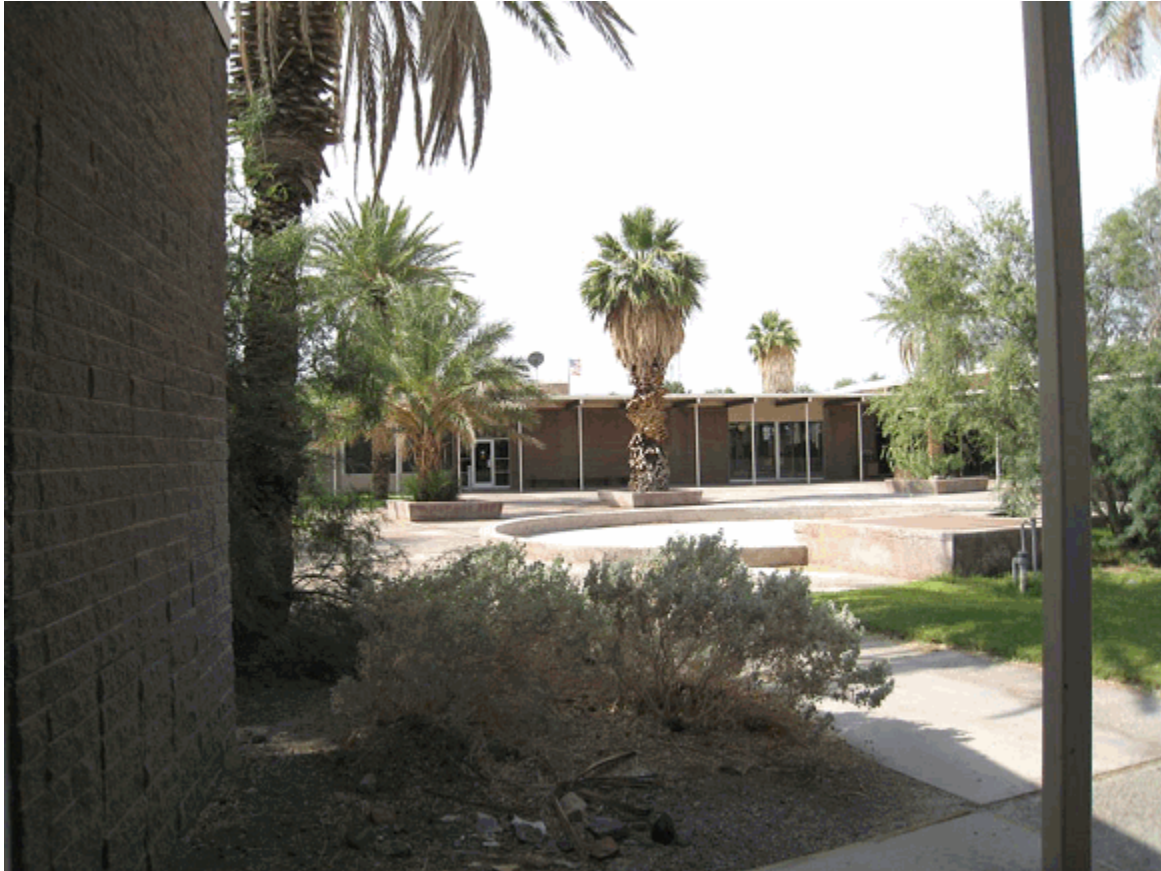
Photograph of the main courtyard, looking southwest toward the back of the lobby wing of the Museum. (PWRO 2009)
