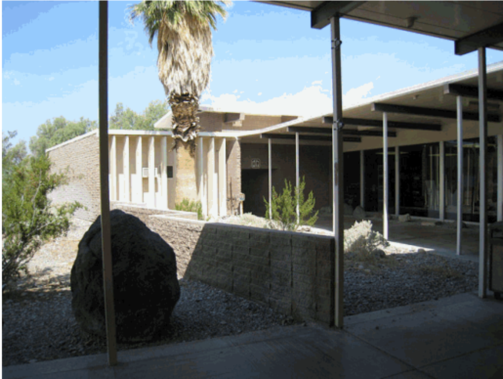
Photograph of small forecourt near lobby entrance of the Museum Building, looking northeast. The original lawn has been replaced with alluvial rock, but the wall and the palm still remain. (PWRO 2009)
