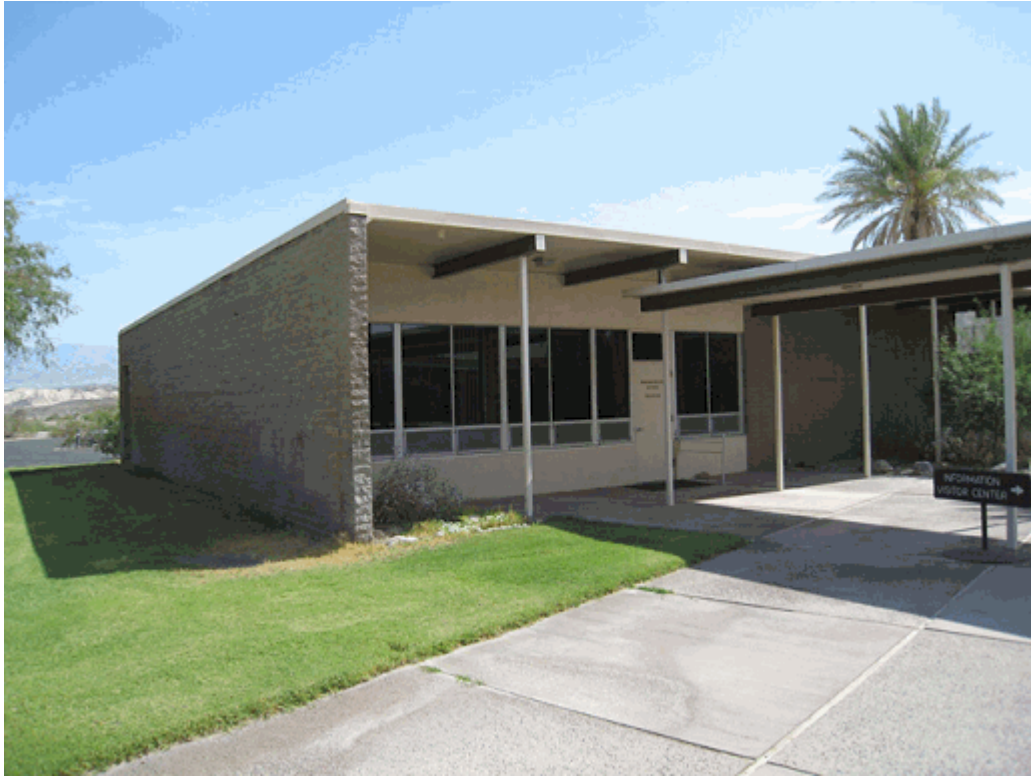
Photograph of the Administration Building south entrance, looking northeast. (PWRO 2009)
