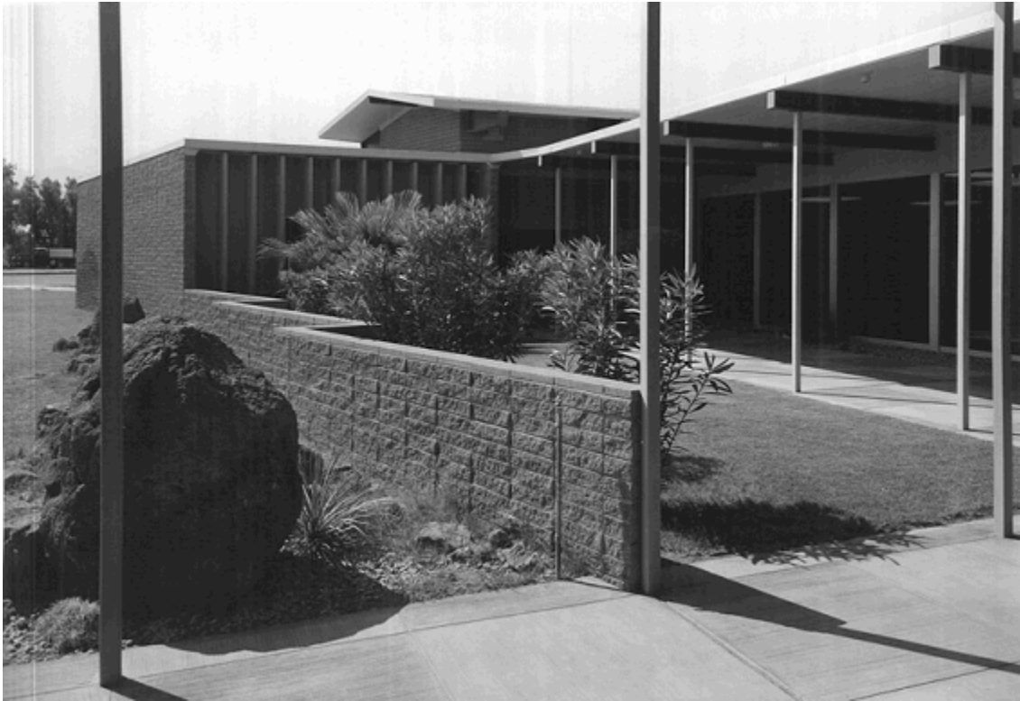
Circa 1960 photograph of the forecourt of the Museum near the lobby entrance, looking northwest. Note the rock garden to the left of the wall and lawn to the right. #143-008 located at the NPS Technical Information Center, Denver Service Center. (Denver S
