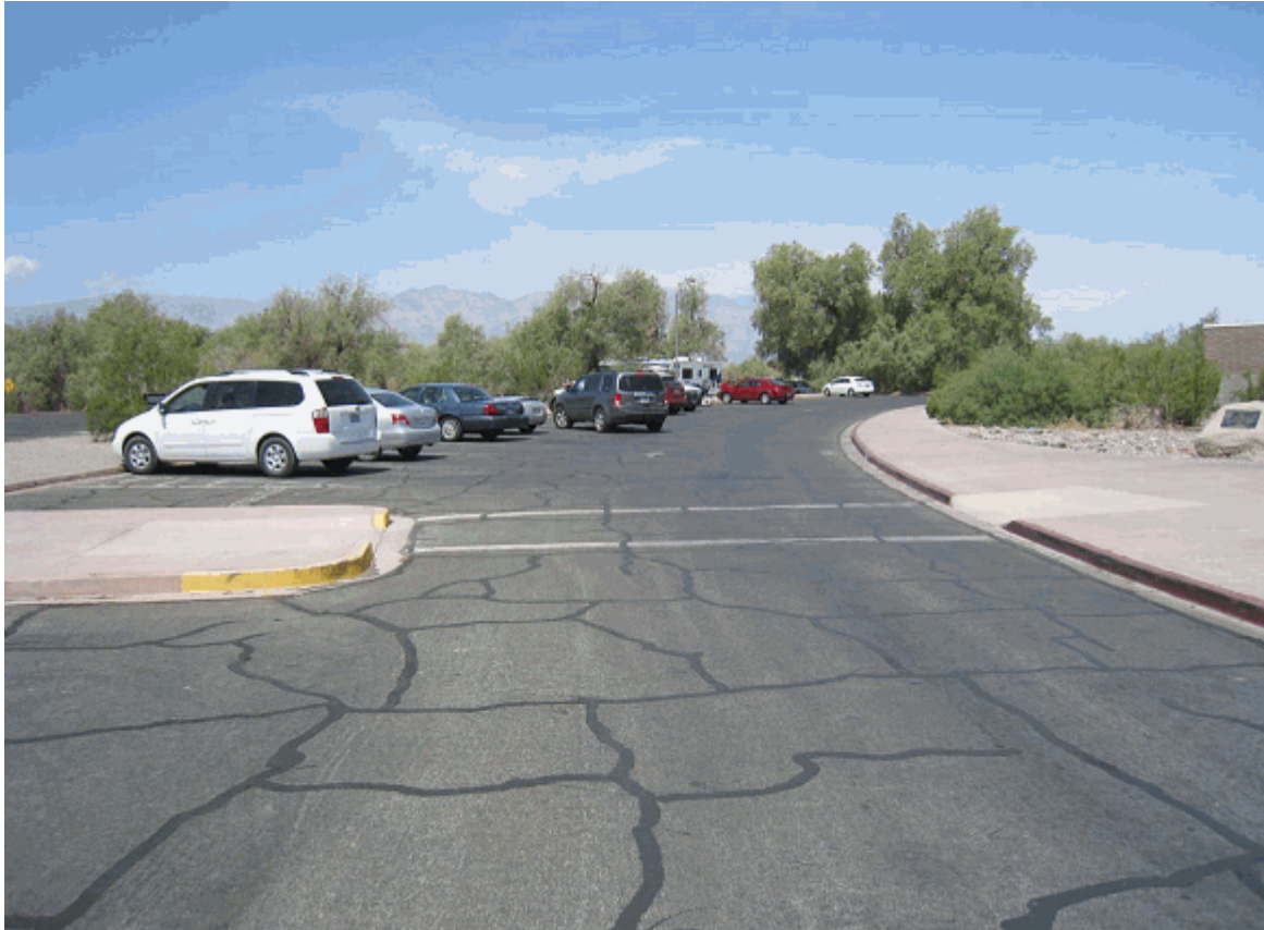
Photograph of visitor parking lot, looking northwest. (PWRO 2009).
