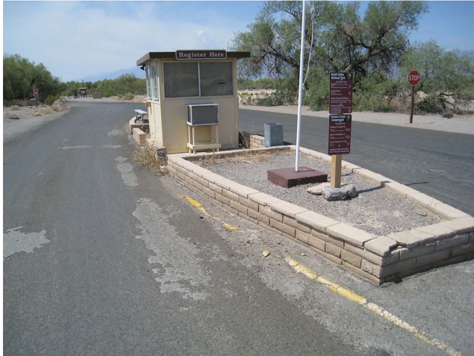
Figure 14. Furnace Creek Campground entrance station, looking southwest (Pacific West Regional Office, 2009). The northern entrance station was added after the period of significance.
