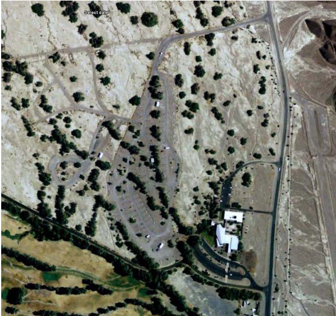
Figure 7. Aerial photograph of Furnace Creek Campground in 2005 (Google Earth website, 2009). The campground has been expanded with multiple loops, new campsites, and comfort stations.
