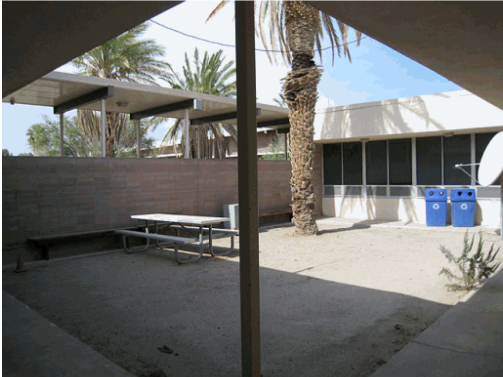
Photograph of the Administration Building courtyard looking southwest. (PWRO 2009)
