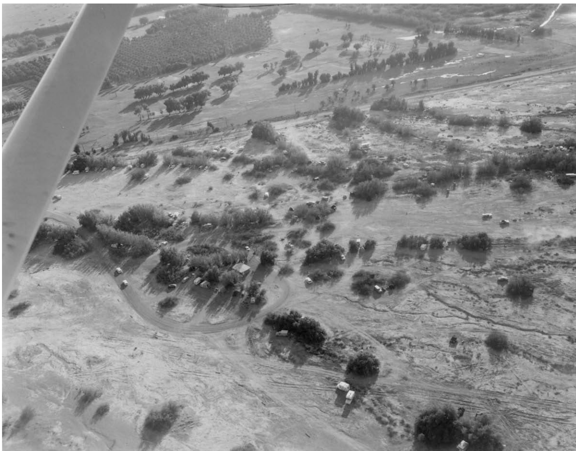
Figure 4. An aerial oblique photograph of Furnace Creek Campground in 1962, looking southwest (Death Valley National Park archives, NEG 2987). Loop A and the comfort station, constructed in 1960, are in the middle-ground.
