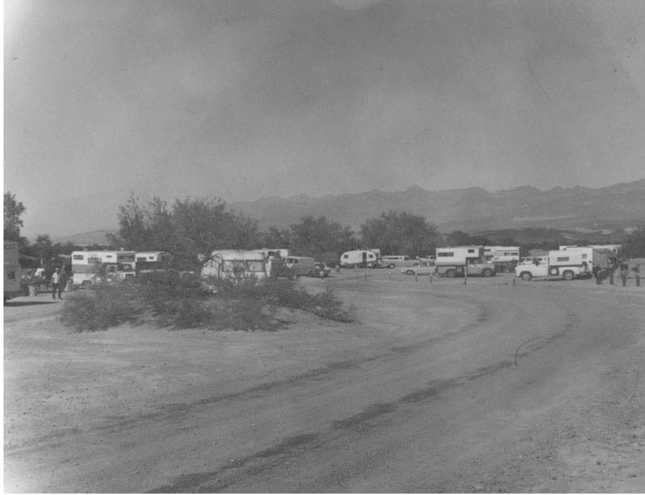
Figure 10. Furnace Creek Campground, looking northwest with Loop A in the foreground (Death Valley National Historic Park archives, NEG 5024, n.d. (circa late 1960s/early 1970s)). In the 1960s, the campground roads were surfaced with gravel. In the right-background, the non-historic outer loop built by this time is visible with its additional camping sites.
