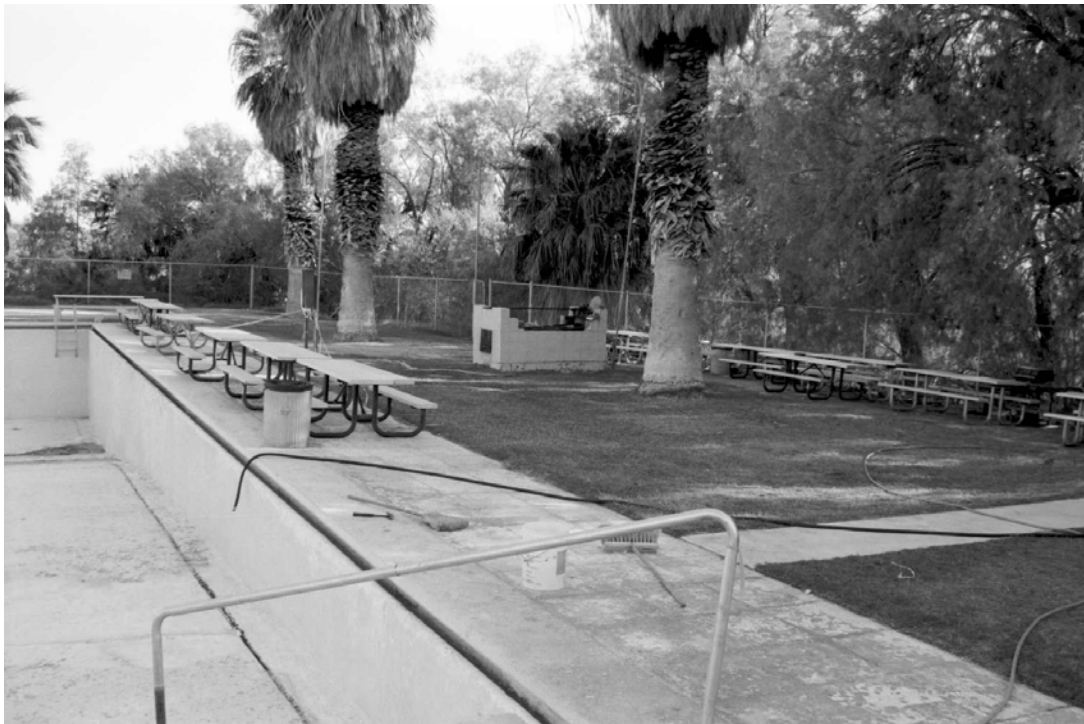
Small Scale Features #4: Pool patio area showing swimming pool deck and barbecue, looking south. (PGSO, CLI negative #DEVA-N-0006-17, 2000)
