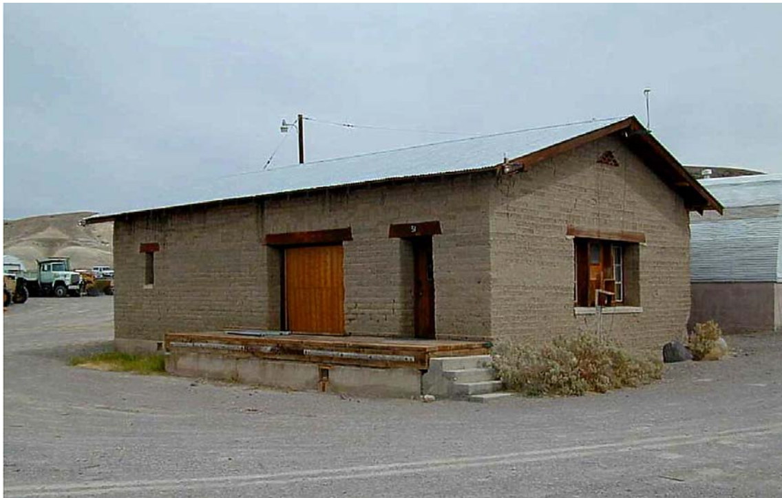
Buildings and Structures #5: Cow Creek warehouse with loading dock, looking east. (PGSO, LCS digital file #DEVA-18, 2000)
