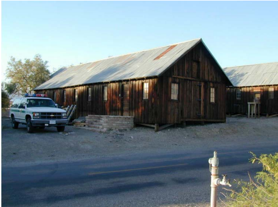
Buildings and Structures #3: Cow Creek warehouse with stone steps, looking north. (PGSO, CLI slide #DEVA-S-0001-12, 2000)
