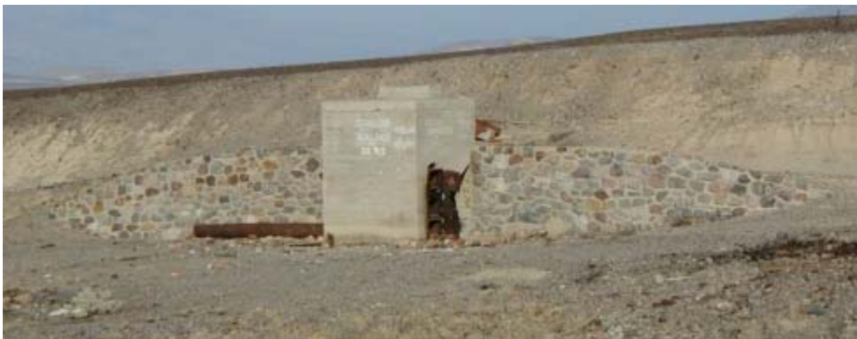
Small Scale Features #5: CCC Incinerator with wingwalls and graffiti, looking north. (DEVA, park digital photo, no identifier, 2001)
