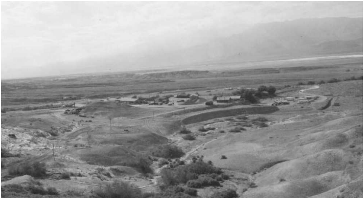
History #8: General view of utility yard area, looking west. (Death Valley National Park archives, Acc. #725.1, DEVA #1657, 1958)
