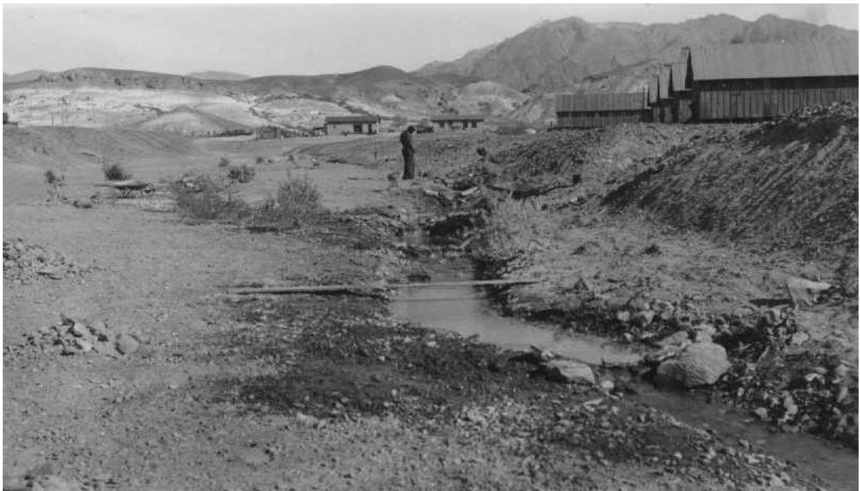
Topography #1: Leveling the wash between Camp Cow Creek and Camp Funeral Range, looking east. (PGSO, Death Valley National Park Archives, Acc. #1240, DEVA #30524, 1936)
