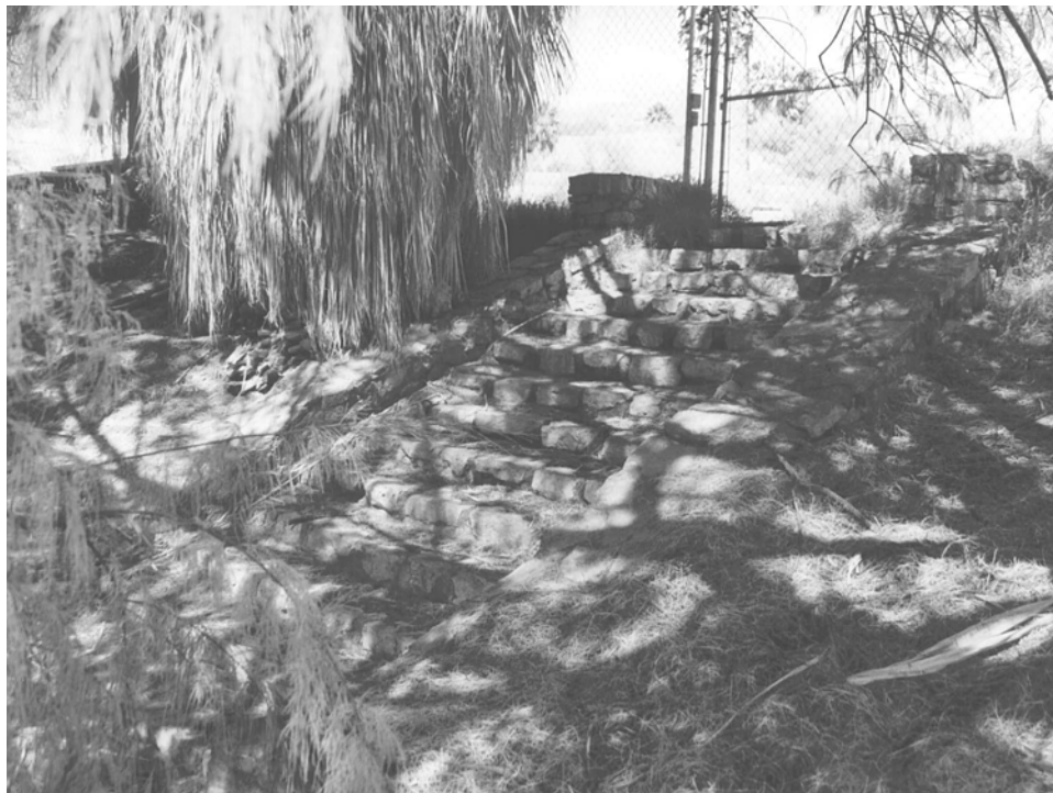
Circulation #5: CCC-era stairs leading to pool area, looking north. (PGSO, CLI print #DEVA-P-0007-2, 2000)
