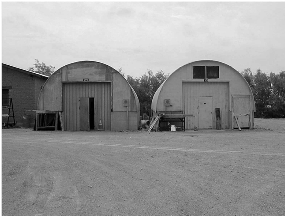
Buildings and Structures #8: Cow Creek quonset huts, looking south. (PGSO, LCS digital file #DEVA-11, 2000)
