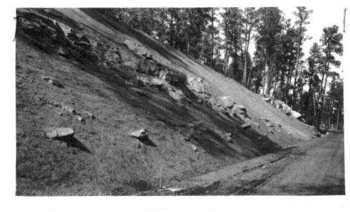
"Cut slope after flattening and rounding. Note all existing rocks strongly imbedded, not disturbed."
