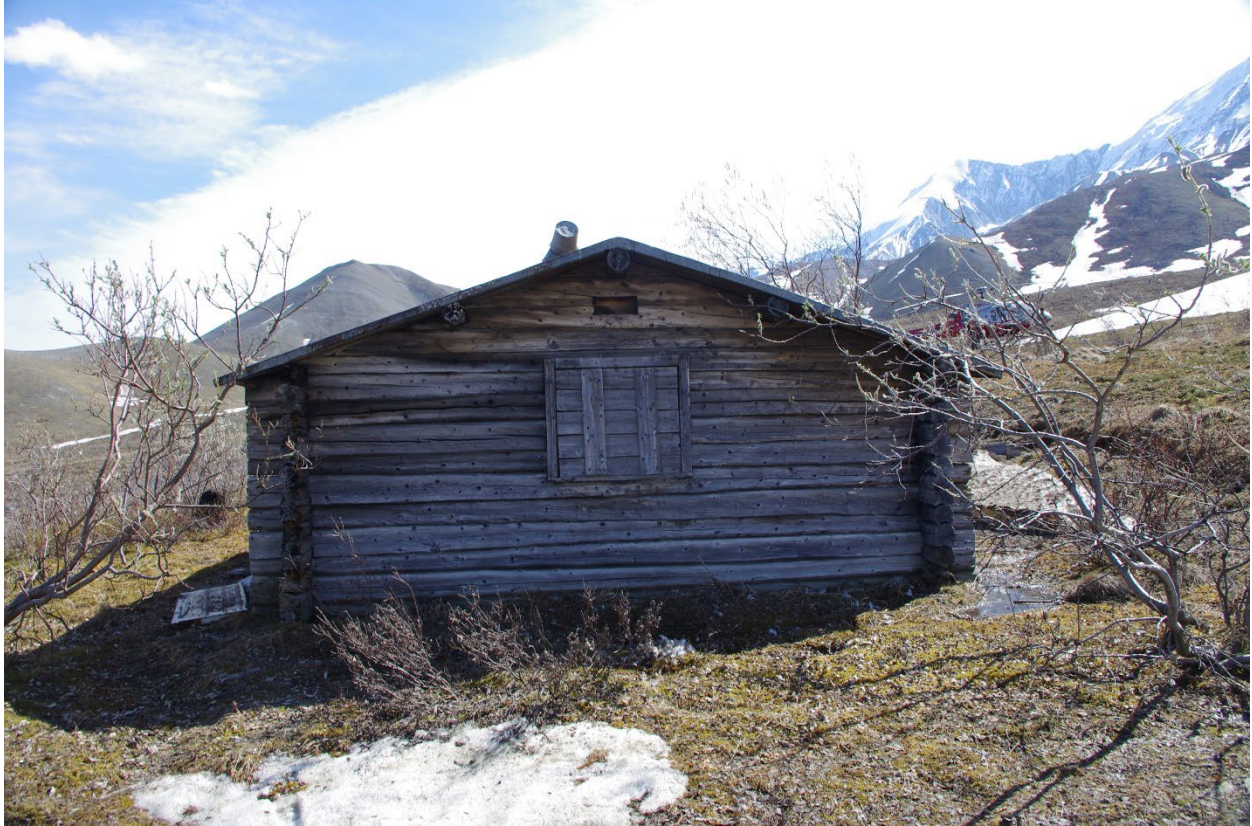
Photograph 3: East gable elevation of the Slippery Creek Mine Cabin, 2022.
