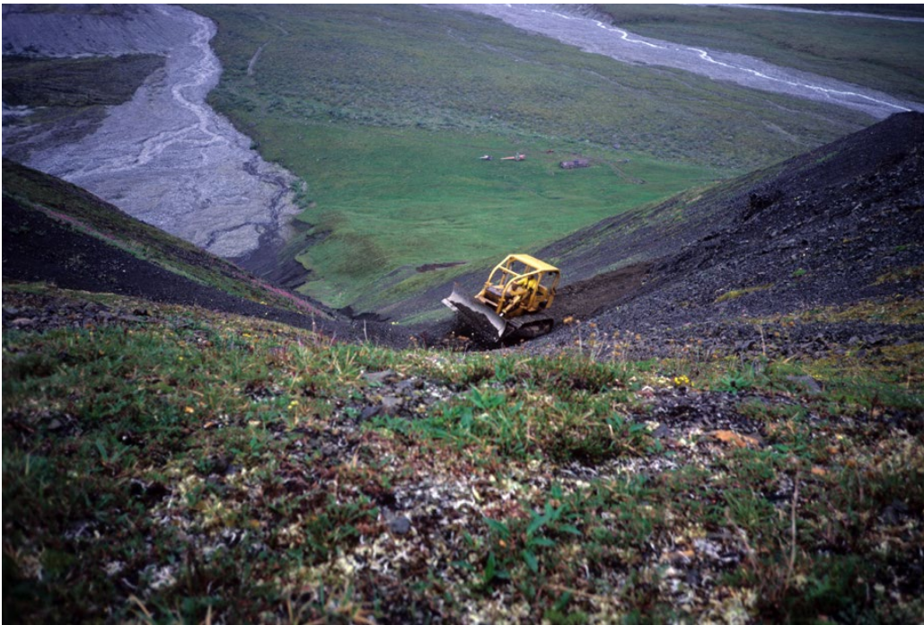
Figure 12: Second phase of Mineral Mountain road reclamation, using the D-6 cat. 1987; photographer unknown. DENA Archives
