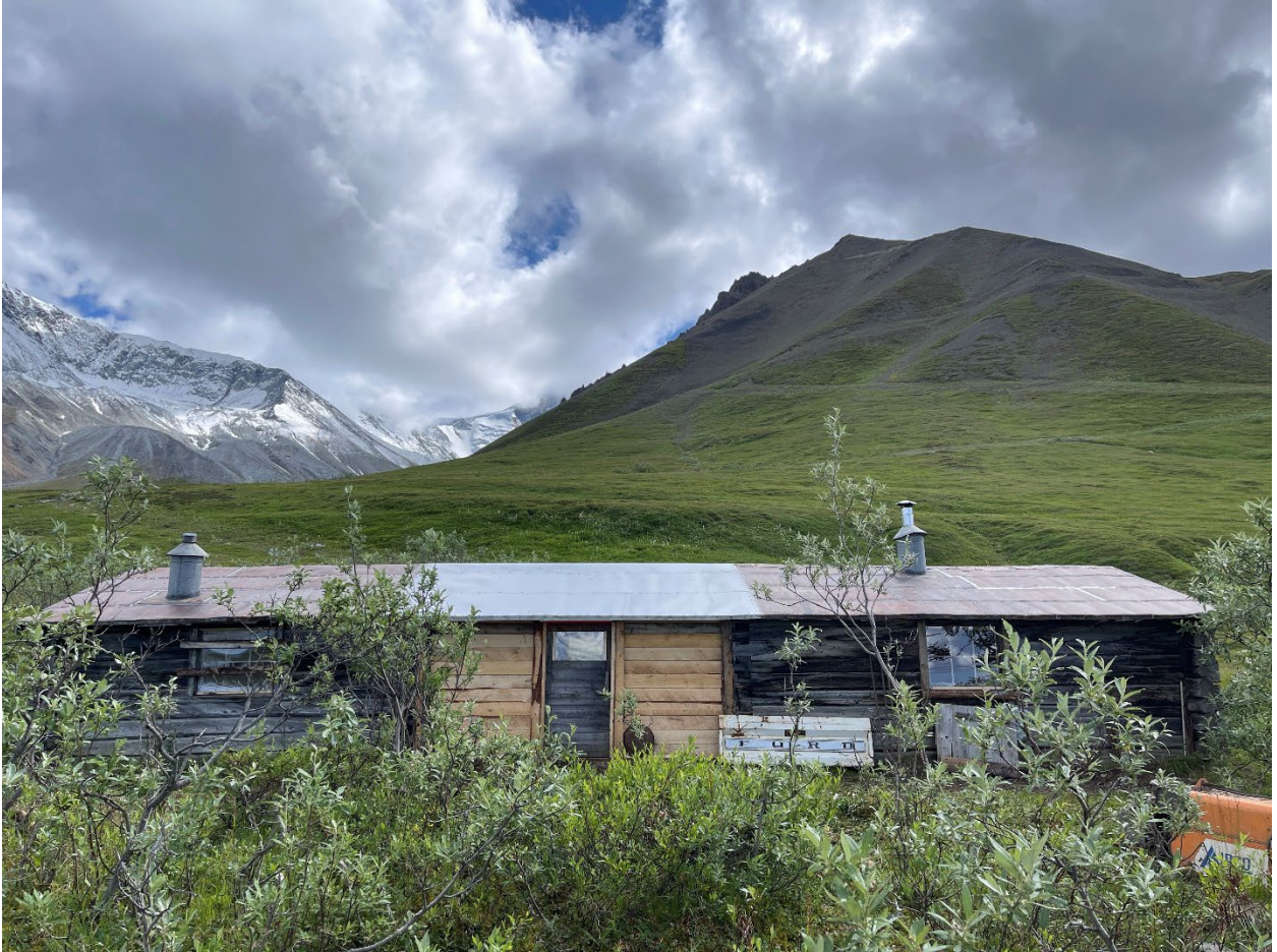
Photograph 2: Front elevation of Slippery Creek Mine Cabin after initial stabilization completed, 2025.
