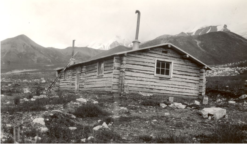
Figure 3: Slippery Creek Mine cabin, looking east. 1941; photographer unknown. DENA Archives
