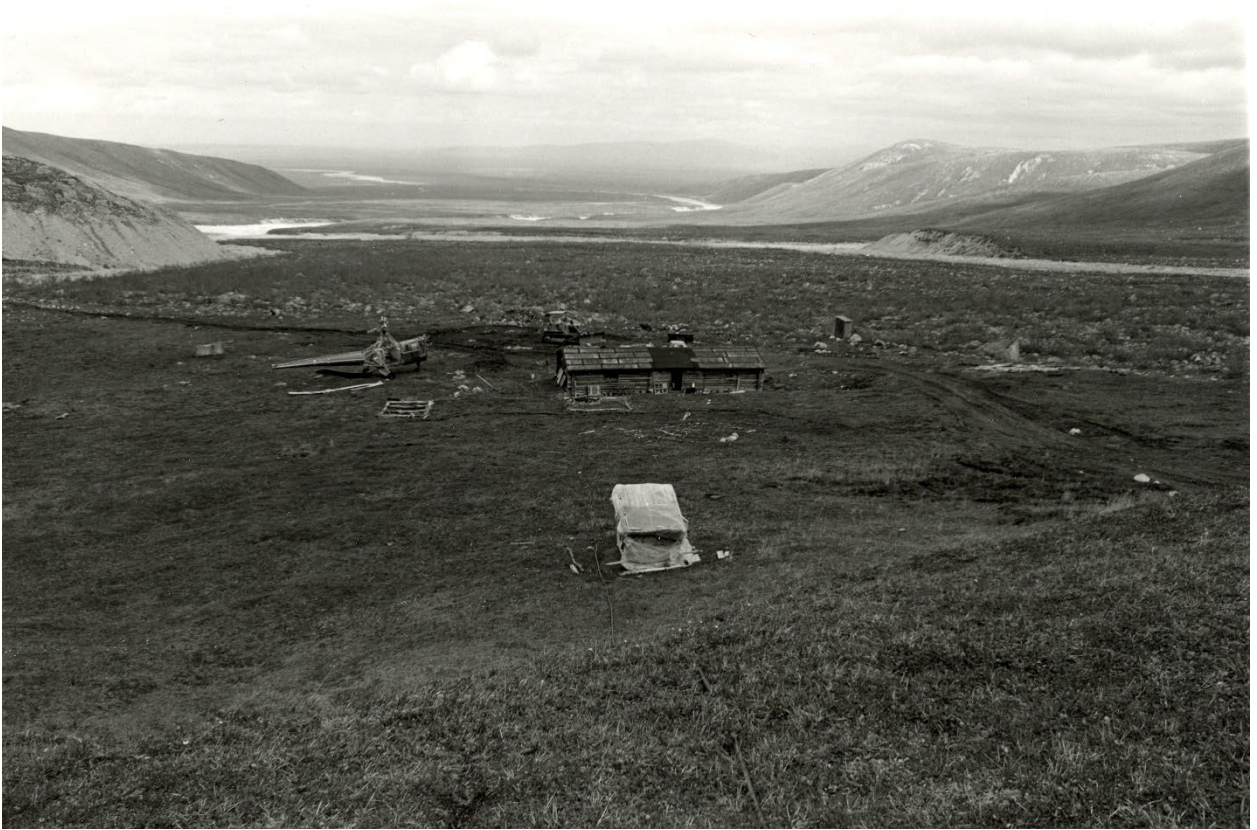
Figure 7: Cabin and site overview, looking north. Buskirk, 1976.
