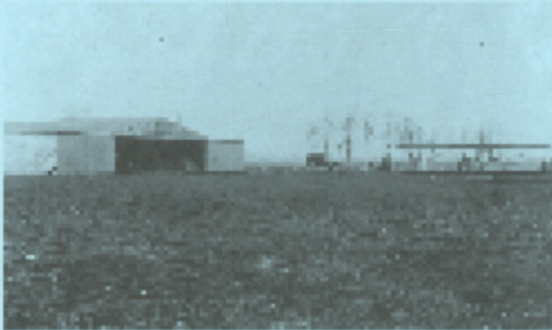
The 1910 hangar housed the Wright Exhibition Company and the Wright School of Aviation.
