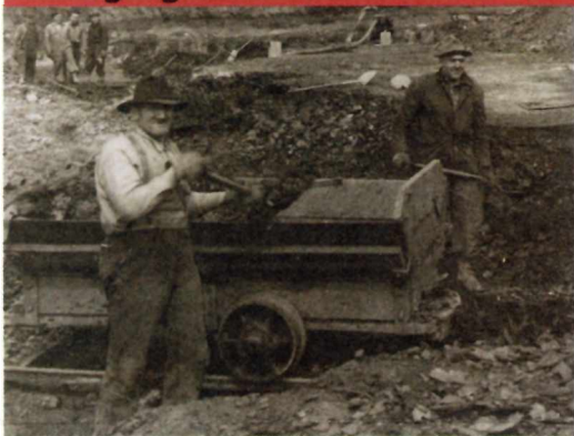
Coal Mining in Tuscarawas County, Ohio, 1930s.
