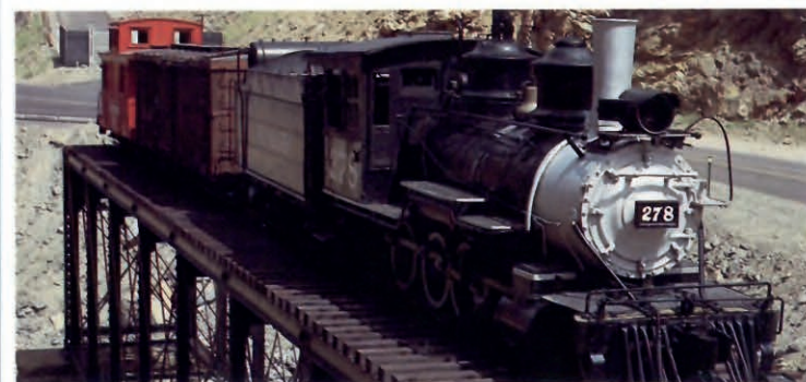
D&RG Engine 278, exhibited on the Cimarron Canyon trestle, recalls the railroad era.
