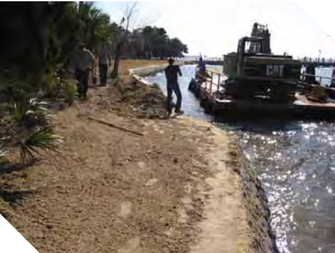
Contractors working to repair one of the Island's seawalls after damages sustained in tropical storms Beryl and Debby.
